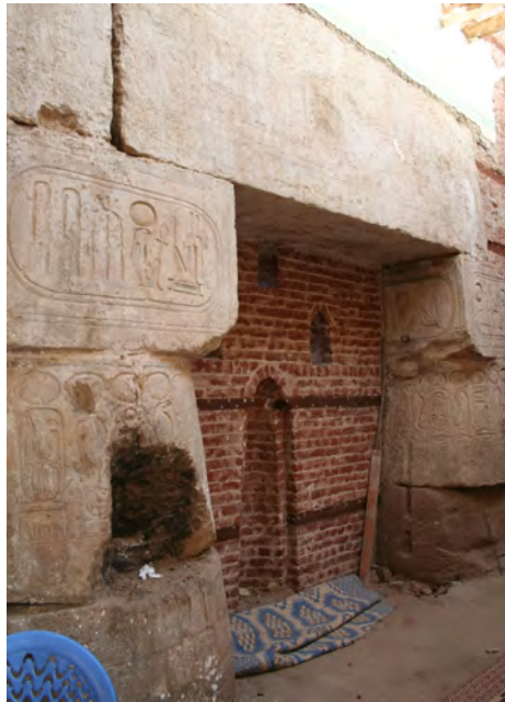
Figure 9.2 The interior of the Mosque of Abul Hajjaj during restoration works, showing the integration of part of the Luxor Temple structure within the structure of the mosque. Image: Hossam Mahdy
