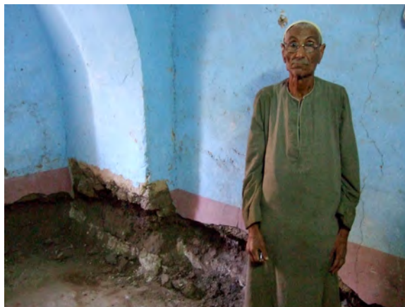
Figure 3.3 Loss of original earthen fabric due to groundwater conditions and poor foundations, as seen in the lower walls of this interior space, has contributed to the use of fired bricks and concrete in the village. Image: Community Consortium / World Monuments Fund
