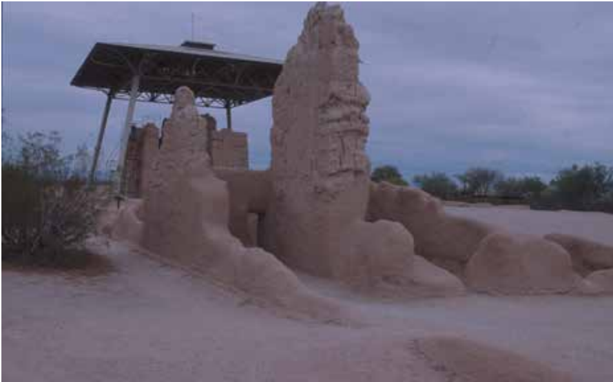
Figure 1 Great House, Casa Grande Ruins National Monument, Arizona. Since 1879 both preventive and remedial measures have been taken to preserve this earthen Hohokam site, including the 1902 and 1935 (present) shelters and a continual program of applying amended earthen shelter coats on the exposed low wall ruins. Reproduced by permission of the U.S. National Park Service
