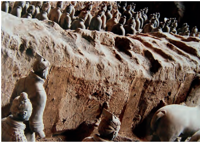
FIGURE 5 Condition of the earthen partition wall after use of steel plates for reinforcing. The imprint of steel plates can be seen on the wall.
