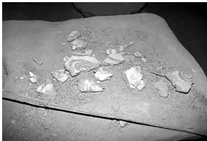
FIGURE 5 Detachment, followed eventually by collapse, is a widespread problem. Here, fragments of painted plaster lost from the west slope in 1996 near an anchor installed in the 1970s. Credit: J. Paul Getty Trust
