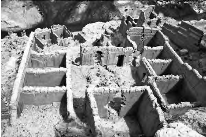
FIGURE 4 Building foundations and the mountainside eroded by rainwater.
