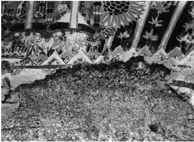
FIGURE 5 Large area of plaster loss in wall painting in cave 368, Mogao Grottoes, Dunhuang.
