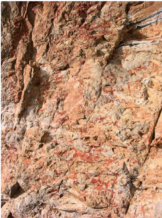
FIGURE 2 Weathering of the rock paintings on the Huashan cliff.
