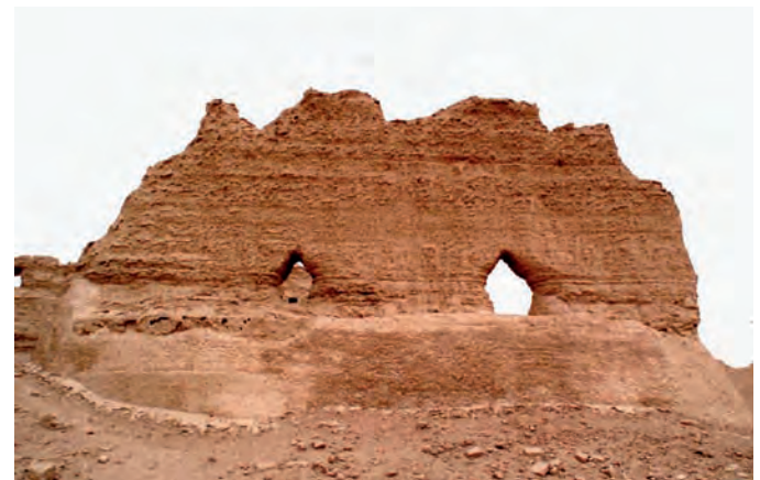
FIGURE 7 Hecang Fortress after consolidation.
