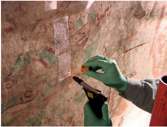
FIGURE 2 Salts being removed with the Preservation Pencil.
