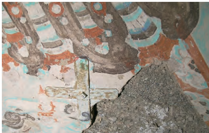
FIGURE 1 Detail of cave 85 showing where painted earthen plaster has separated and fallen away from the underlying conglomerate rock. A metal cross-brace was bolted into the rock by Dunhuang Academy conservators before the collapse but failed to prevent it. Photo: S. Rickerby
