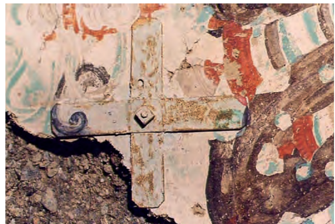
FIGURE 5 Example of the steel anchors used to secure areas of detached painted plaster in cave 85. The anchor was painted to match the decoration of the original painting.
