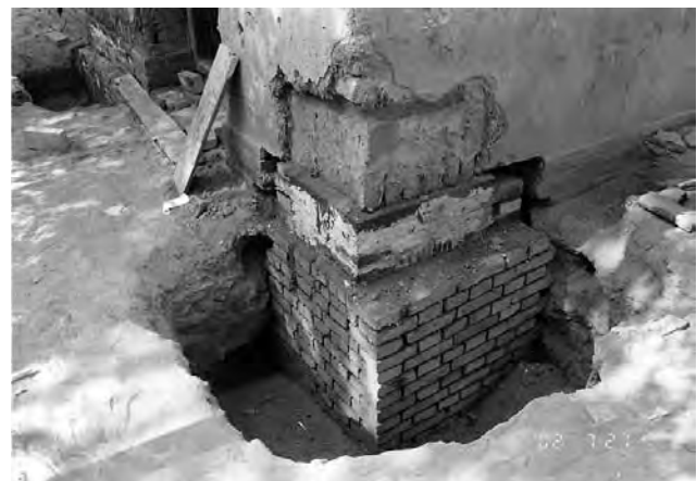
FIGURE 3 Wall stabilization with a brick footing.
