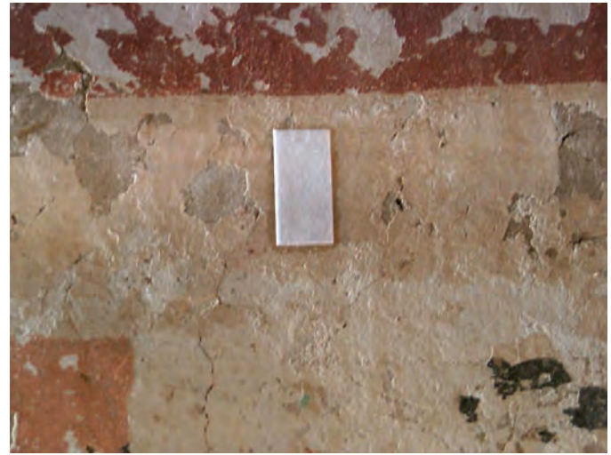
FIGURE 3 Prewettted paper strip applied to a wall painting in cave 85.
