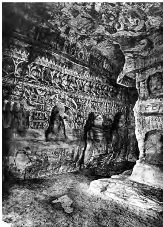
FIGURE 1 Weathering of the lower part of the west wall of cave 1 due to groundwater.
