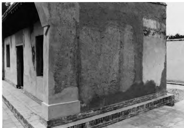
FIGURE 2 The north wall shown in figure 1 after restoration.
