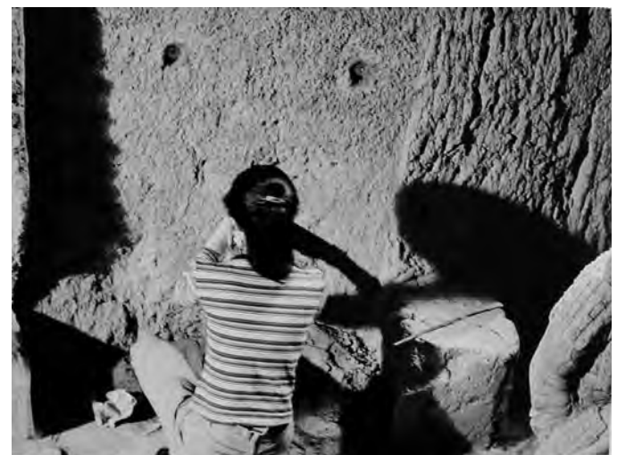
FIGURE 6 Reinforcing with the anchor bolts and grouting method.
