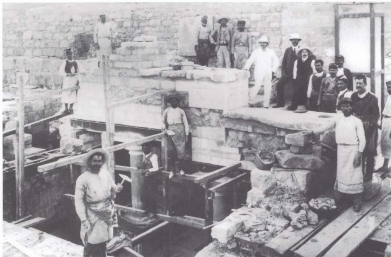
Figure 17 Grand Staircase during restoration, 1910. The wooden supports initially used to stabilize the structures (see Figs. 15, 16) were replaced a few years later by iron girders. Arthur Evans, dressed in white, is seen at the upper center right; next to him stand Duncan Mackenzie (wearing a pith helmet), Evans’s assistant and supervising field archaeologist, and the architect Christian Doll (wearing the wide-brimmed hat).
