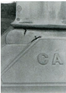
FIGURE 8. Detail of stress cracks, Fourth Ohio Infantry Monument, Gettysburg National Military Park, Gettysburg, Pennsylvania, sand-cast and sandblasted by the Monumental Bronze Company, 1887.
