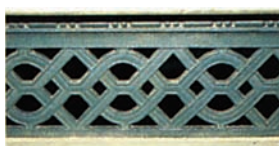
FIGURE 9. The Rookery, oriel stair riser. Cleaned original Bower-Barff finish.
