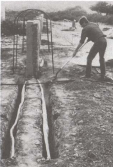
Figure 17. a) Close up of geodrain showing black plastic core and white geotextile fabric. Manufactured under the name Cordrain, by Nylex Corp., Australia. b) Photograph showing geodrains in place and being buried by author.
