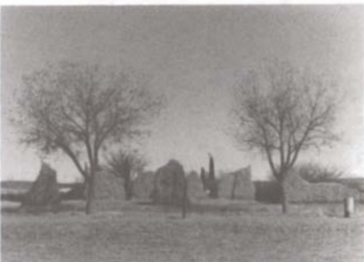
Officer's Quarters after stabilization, 1980. New Mexico State Monuments.
