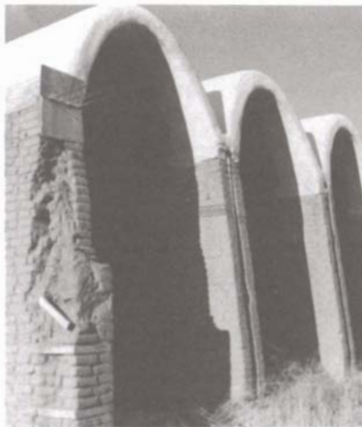
4. Barrel vaults. Photo: James Steele.
