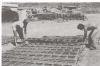
Figure 2. Adobe mud placed in 10-brick ladder forms at the commercial adobe yard of New Mexico Earth in Alameda, New Mexico.
