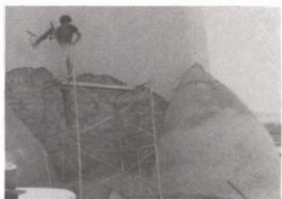
Figure 14 Removing Cement Stucco Before Mud Plaster San Francisco de Assisi Ranchos de Taos, New Mexico
