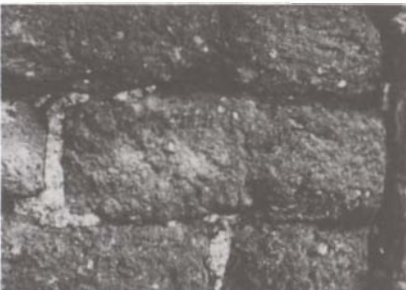
Figure 17. Detail of the same wall in 1969.
