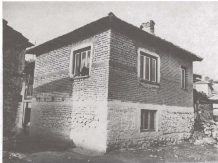
Fig. 7 - Modern reinforced concrete belt Struga (South Macedonia) - Application of reinforced concrete belts in adobe wall weight-bearing structures as a reflection of reinforcement new structures after Skopje 1963 Earthquake.
