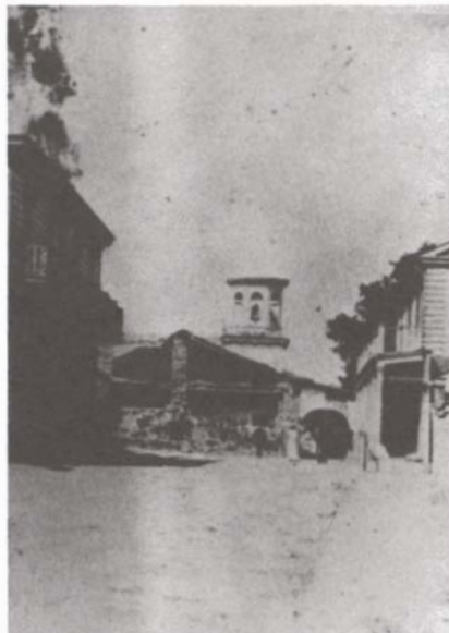
Figure 2. Mission San Juan Bautista, Convento Wing. View of damage after the 1906 earthquake. (Photograph from San Juan Bautista Historical Society)
