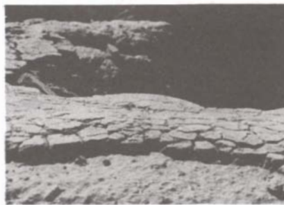
Figure 12. Detail of the soil-cement capping, partially detached and cracked. Besides damage due to temperature changes and water infiltration, it should be remembered that people walked on the capping.
