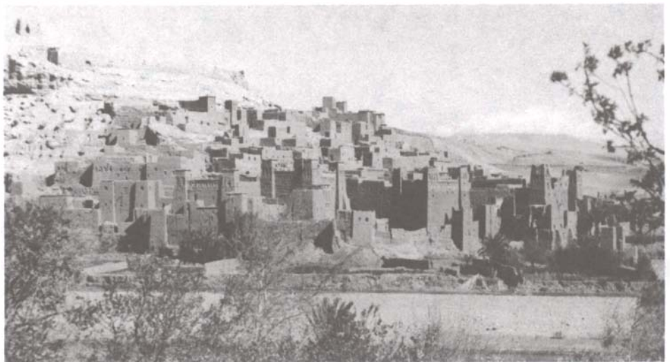
Figure 11. The ksar Ait Ben Haddou (25 km N-E from Ouarzazate) is threatened with destruction. Its rehabilitation is now being planned under the leadership of CERKAS (Photogr. Ministry of Culture/Baamri, 1975)
