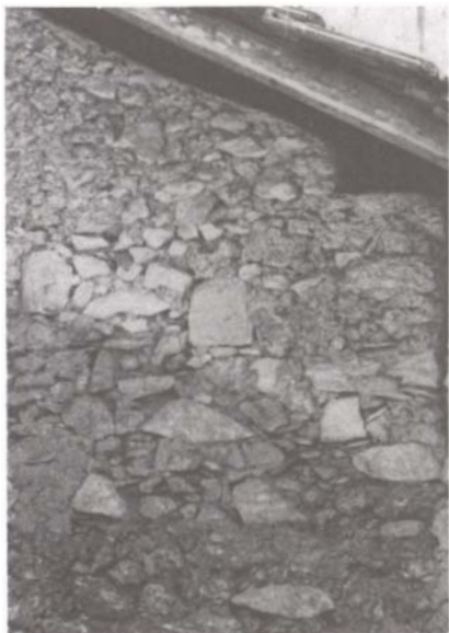
Figure 10. A wall made of rubble bonded with mud.
