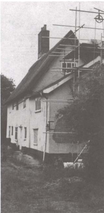
3. Pulham Manor Farm is a mediaeval timber and earth building with a nineteenth century earth block addition.
