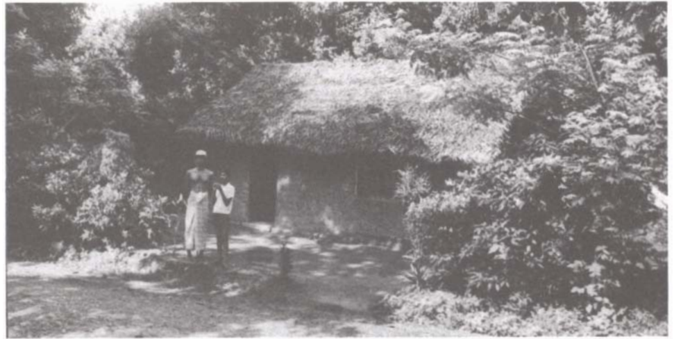
Figure 8. A house constructed with sun-dried bricks (adobe).
