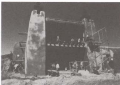
Figure 11 Mud Plaster Workday San Jose de Gracia Las Trampas, New Mexico Photo by Anita Rodriguez
