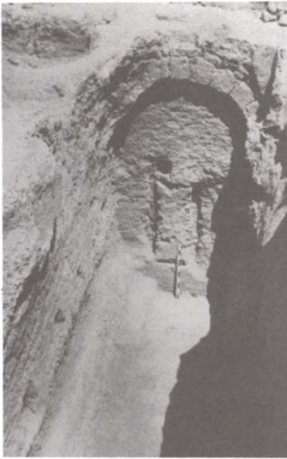
Fig.3. Ground floor room with its vault. Early 8th century.
