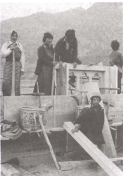
Fig. 4. Placing the windows.
