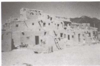
Figure 1. Five-story Taos Pueblo originally built of puddled adobe (made by patting mud into a wall-shape) before the introduction of Spanish adobe forms. Note mud plastering that is carried out each year to maintain the structure.
