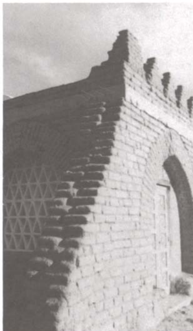
5. Buttress wall and concrete lintel beam. Photo: James Steele.
