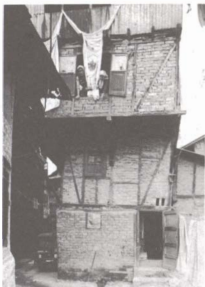
An example of Dhajji Dewari construction.
