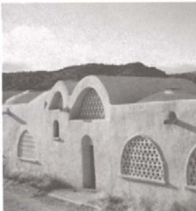
6. Cement plaster coating. Photo: James Steele.
