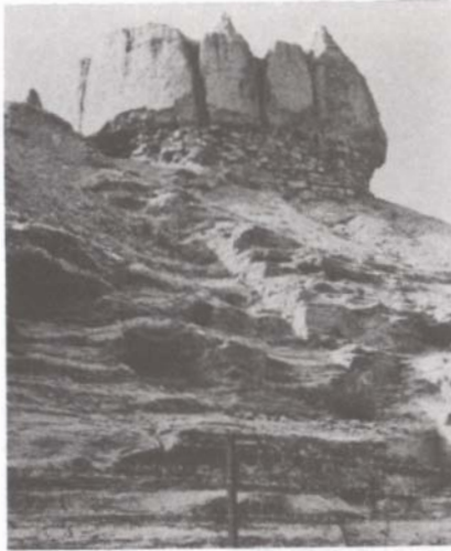
26. Faisal Tower prior to reconstruction as seen from the wadi below.
