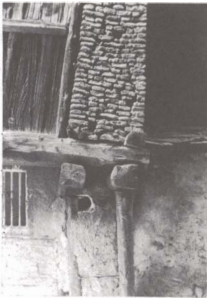
Above: A masonry pier resting on a timber cantilever bracket on a ca. 18th century house. The beams extend across the width of the house, tying it together, while the weight of the masonry holds the wood in place in an earthquake.
