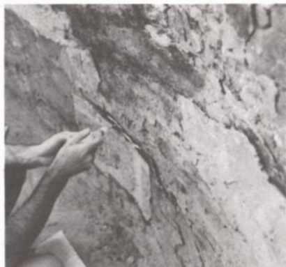
8. On-site pilot conservation treatment. Injection of adhesive after facing with Japanese tissue.
