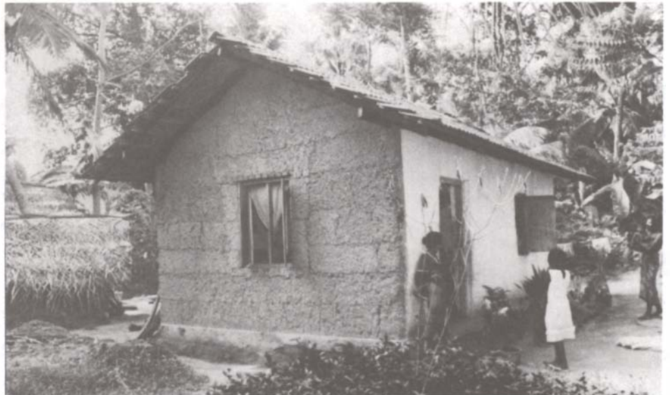
Figure 7. A completed house with rammed earth-walls and a tile roof with the front wall plastered and white-washed; the side-wall shows how the work progressed.
