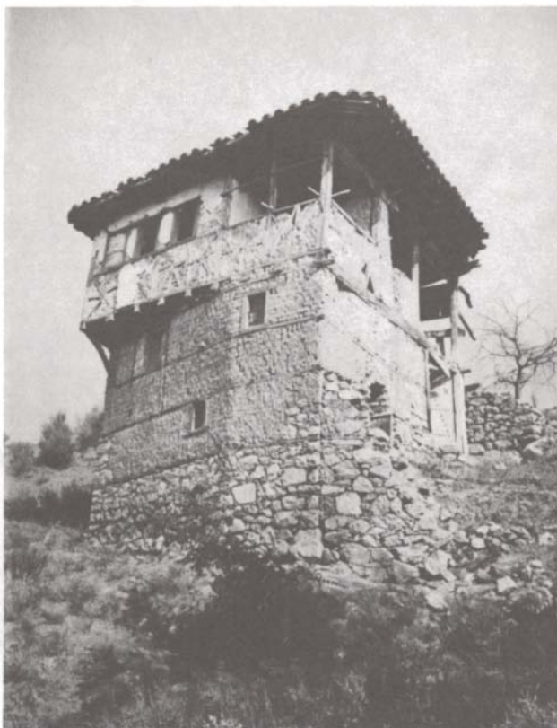
Fig. 2 - Typical traditional aseismic elements v. Cucer (Skopje region)
