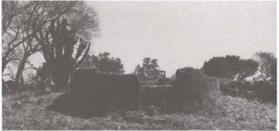
Fig. 3: Prehistoric structure-exterior decay. Note flaking towards base of wall
