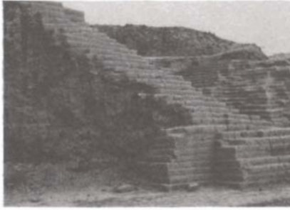
Figure 7. On the north side, the unprotected wall has suffered an enormous loss of material, due to the rain. (Tell 'Umar).
