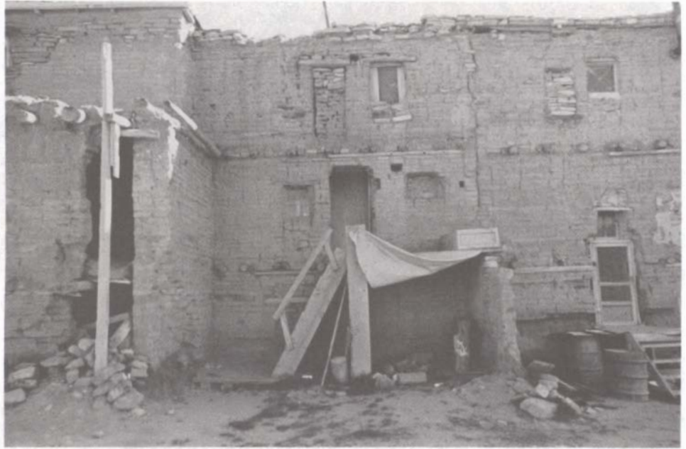
Area "C" north side, before rehabilitation.
