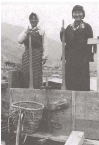
Fig. 2. Bhutan, process of constructing "pisé de terre".
