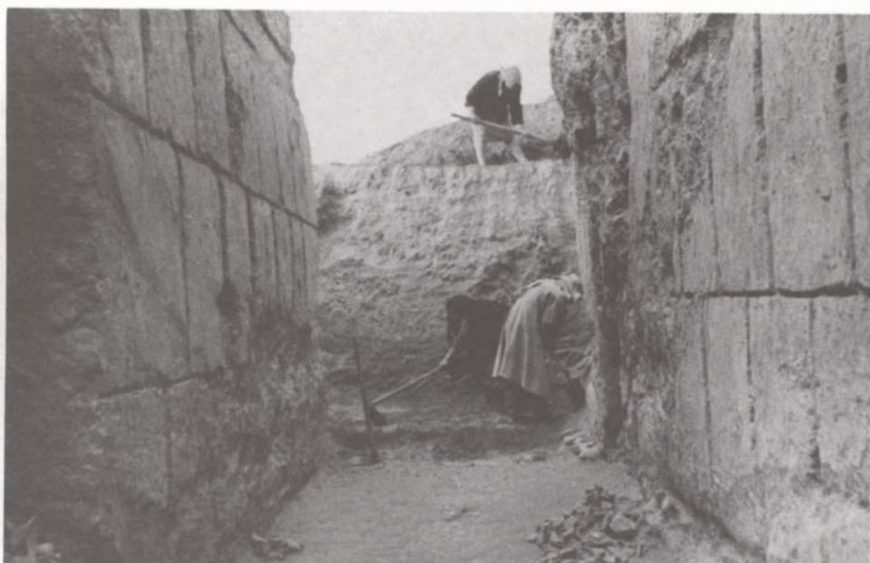
Fig.2. Vaulted alley with the walls from pisé divided into large blocks.
