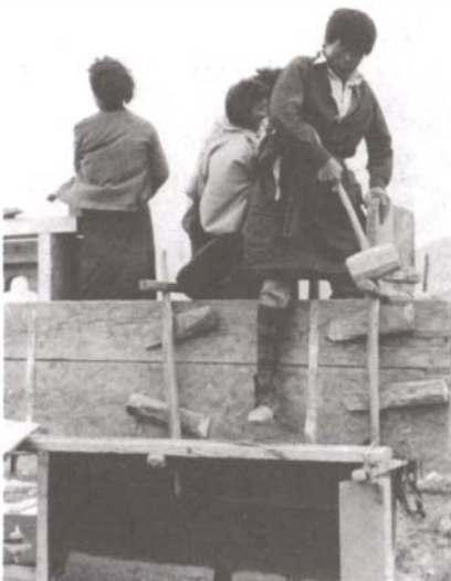
Fig. 3. Setting the planks.
