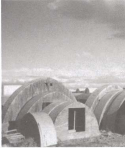
3. Plywood forms for arches. Photo: James Steele.
