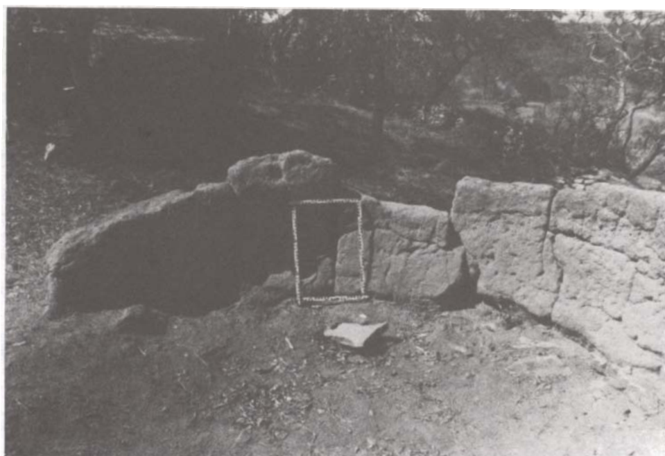
Fig. 2: Prehistoric structure-interior decay.
