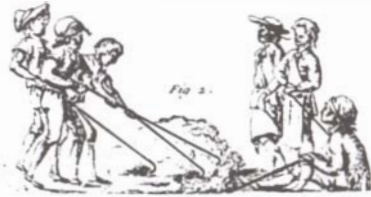
Fig. 6. Plate XII from Cointeraux's Second Cahier , showing workers mixing soil.
