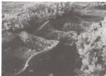
Figure 13. Rooms at "Via Porticata", in the Seleucia area, without any conservation work.
