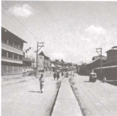
The new road constructed during the 1970's which replaced the picturesque 14th century Mar Canal which used to penetrate the heart of Srinagar. The sewerage line which was supposed to replace the canal was deleted in a budget cut, so now the sewerage which used to flow out of the city through the canal now backs up into Dal Lake.
