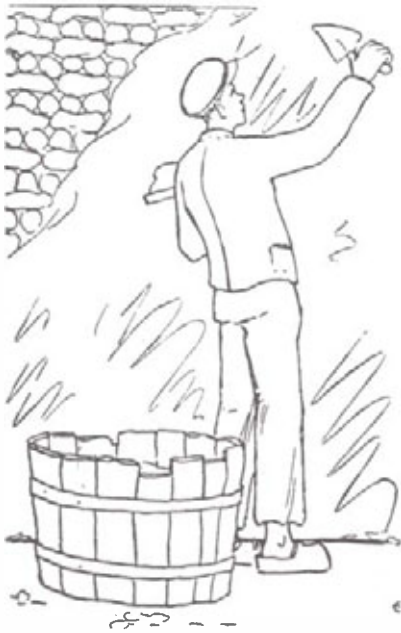
Plastering a wall made of clay-loaves.
