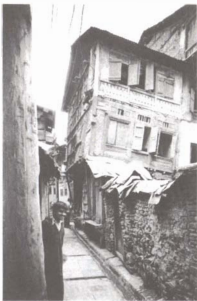
Many of the houses in Srinagar remain radically askew from weak soil and past earthquakes.
