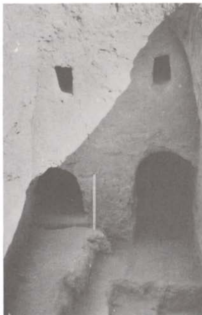
Fig.4. Lobby with two doors and two windows for the stair-case. Early 8th century.
