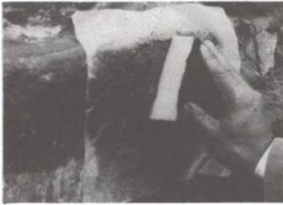
Figure 3. Application of moistened rice paper: the pressure allows adhesion to be reestablished.
