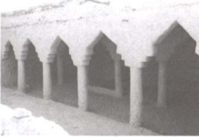
7. Example of stone keel arch construction typically used in mosque and public building construction.
