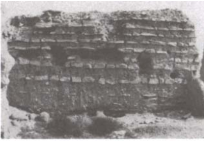
6. Example of horizontal coursed stone used in wall construction.
