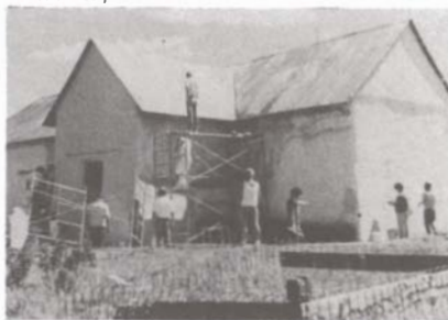
Figure 10 Lime Plaster Workday La Capilla de San Antonio Chacon, New Mexico
