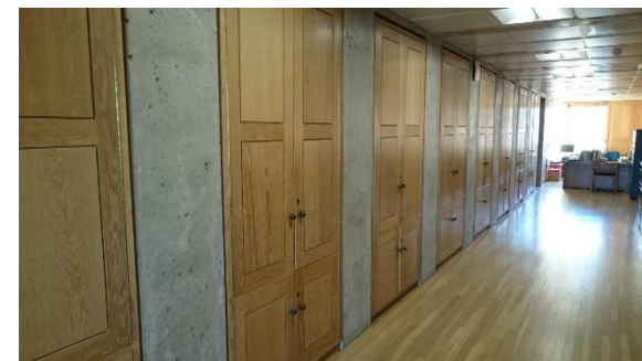
White oak strip flooring in North Office Wing, installed 1965.
