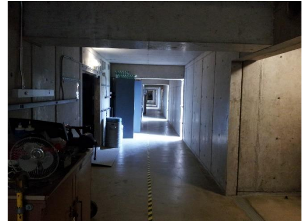
North Laboratory building, circulation adjacent to pipe floor, 2015.
