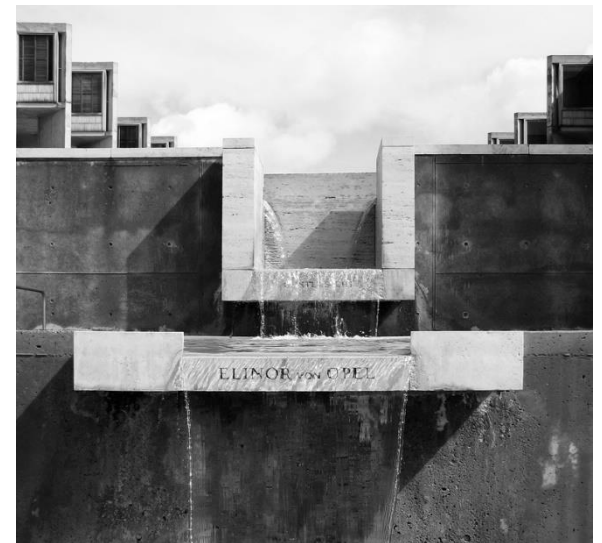
Top: Construction of cistern below West Court, 1965. Bottom: Cascade from West Court.
