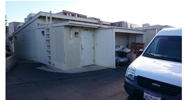
Temporary Buildings No. 4 and 5, 2015.
