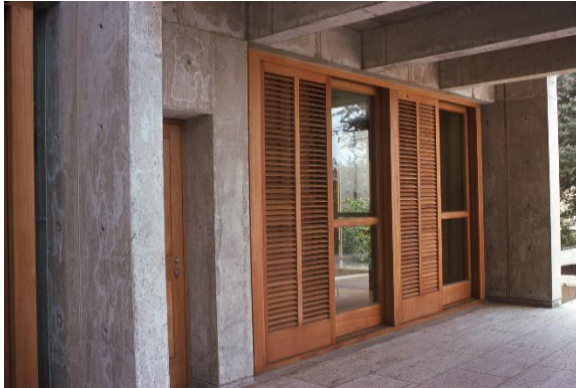
Millwork within arcade, North Office Wing in 1977.
