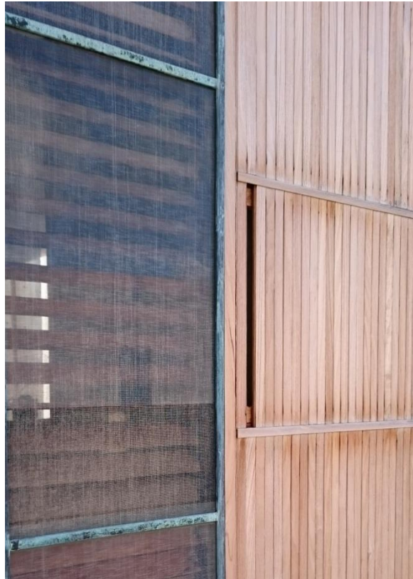
Failure of teak siding, as a result of weathering due to ultraviolet exposure over time, revealed concealed nailing and reduced the cross-sectional area of the wood.
