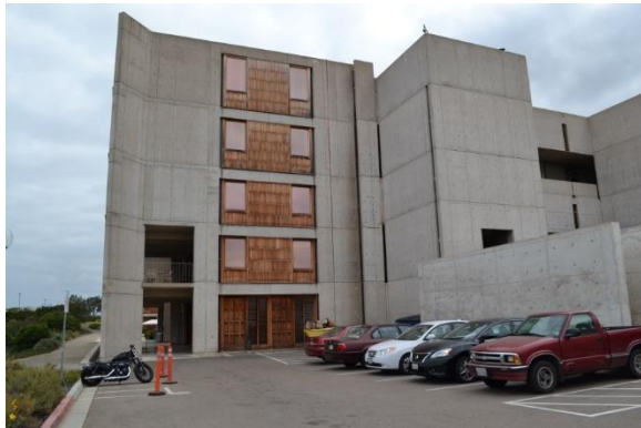
Top: Walls edging the south garden. Bottom: The south parking area.
