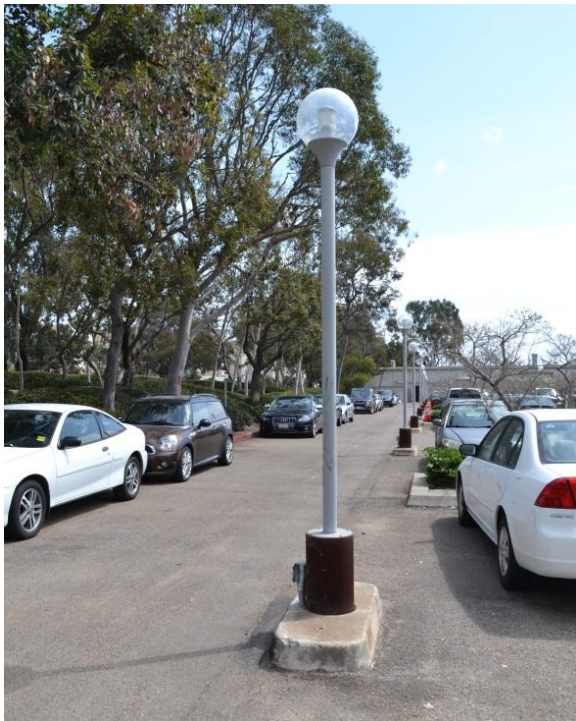
Top Cracks in the pavement caused by Chinese fringe tree roots.
