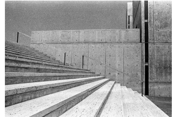
Travertine steps at Northwest Entrance.
