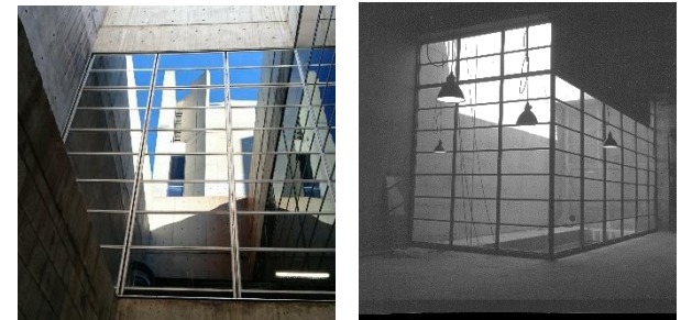
Top left: Slot windows to service towers. Top right: Later mesh to blank openings to pipe spaces. Bottom left: Demountable glass wall giving plant access to mechanical wing. Bottom right: Mechanical wing light well in 1965.
