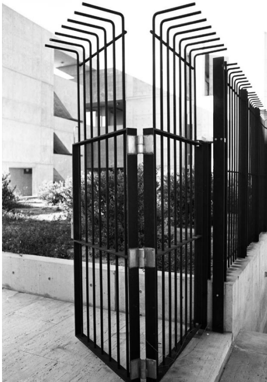
Top: East Gate Corten gates and railings in 1967. Travertine parapets not yet added to the steps. Bottom: Corten folding gates and railings to the East Gate in 1967.
