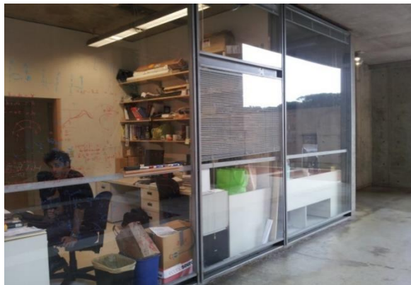
Top: Tempered glass produces different reflections to the original polished plate. Bottom: Kahn likely never suspected glazed walls would become “chalkboards.”
