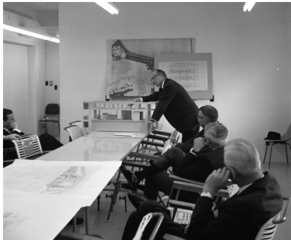
Top: Temporary Building No. 1 under construction, 1963. Bottom: Dr. Salk explaining the Third Design to Trustees in the temporary buildings, 1964.
