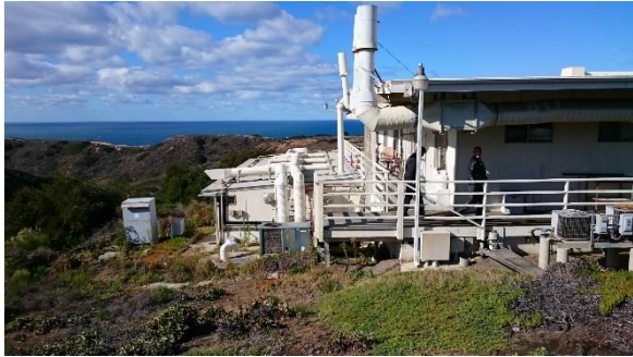
Temporary Building No.1 with later modifications, 2015.
