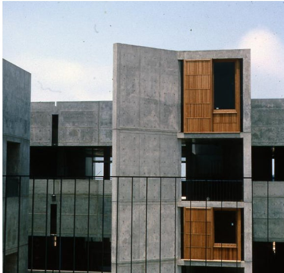
Stainless steel railings to porticos of the study Towers.
