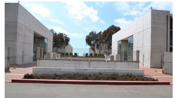
Top View of the East Building (north). Middle: View of the East Building (south). Bottom: The east gate is composed of a central concrete wall edged by stone blocks inscribed with quotes, and a steel fence that is framed on either side by pedestrian gate openings. Low shrub plantings occur within a planting bed in front of the wall.
