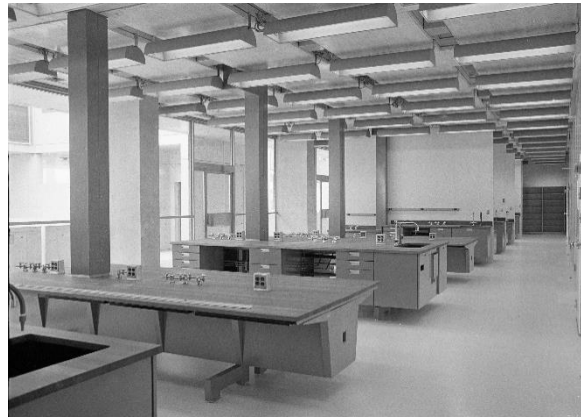
Top: Typical shell of North Laboratory in 1965. Bottom: Fit-out of North Laboratory underway but not yet complete in 1966.
