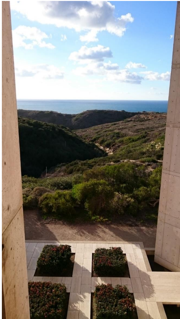
North Building: View from Study Stair over the canyon to the ocean, 2015.
