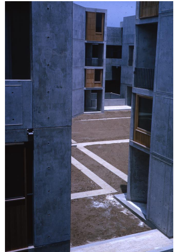
Plaza left with earth infill between channels, 1965.
