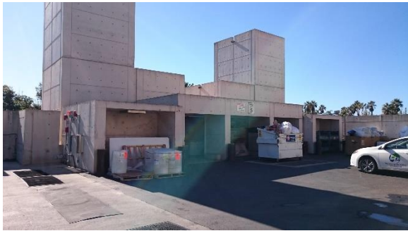
Service Yard: the service towers were introduced in 1975.
