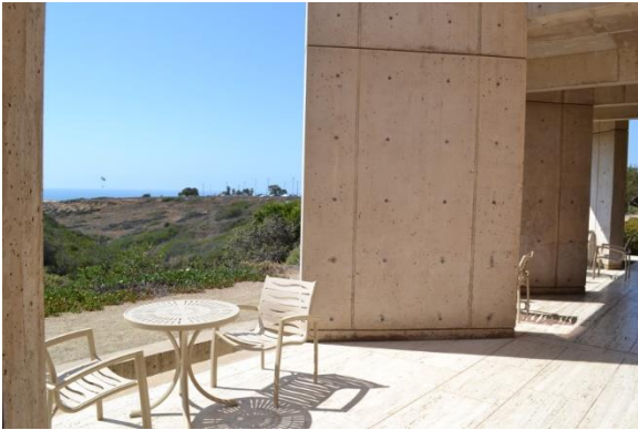
Top: The upper and middle pools. Bottom: Tables and chairs associated with the makeshift cafeteria.
