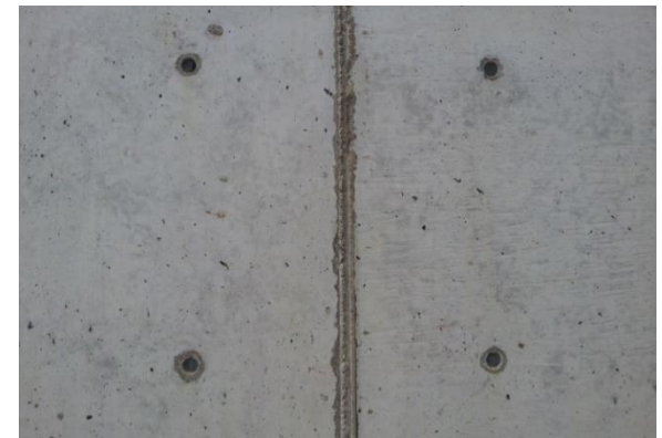
Top: Dr. Salk reviewing concrete samples in the excavation for the Mechanical Wing. Bottom: Typical concrete fins and lead plugs.
