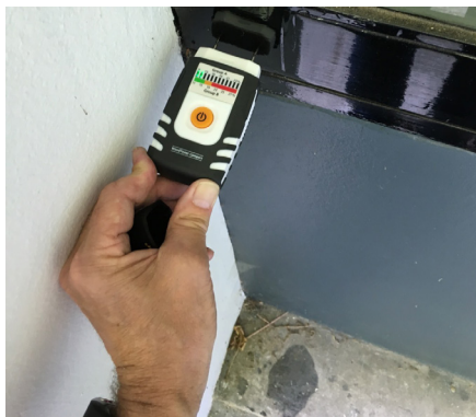
Figure 6: Indicative measurement of moisture content in timber window frames
