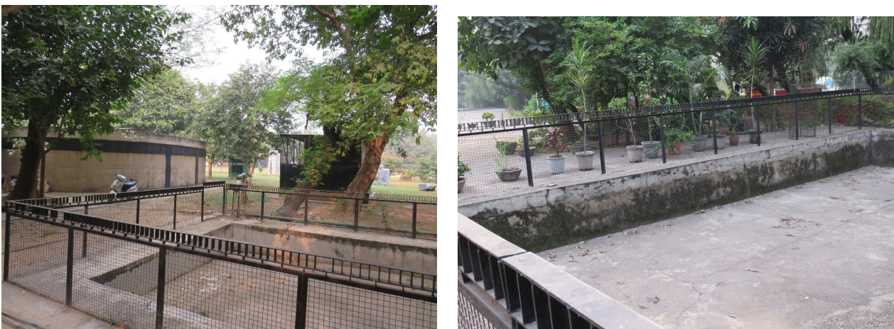
Fig. 127: Addition of metal railing around - Rear pool (L); Auditorium pool (R)
