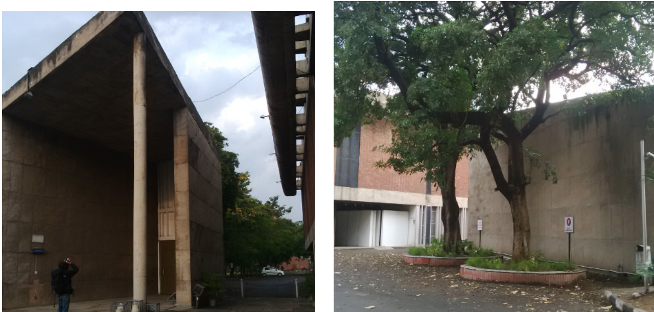
Fig. 129: Damaged litterbin and cluster of uplighters near auditorium (L); Inefficient signage and other utilities
