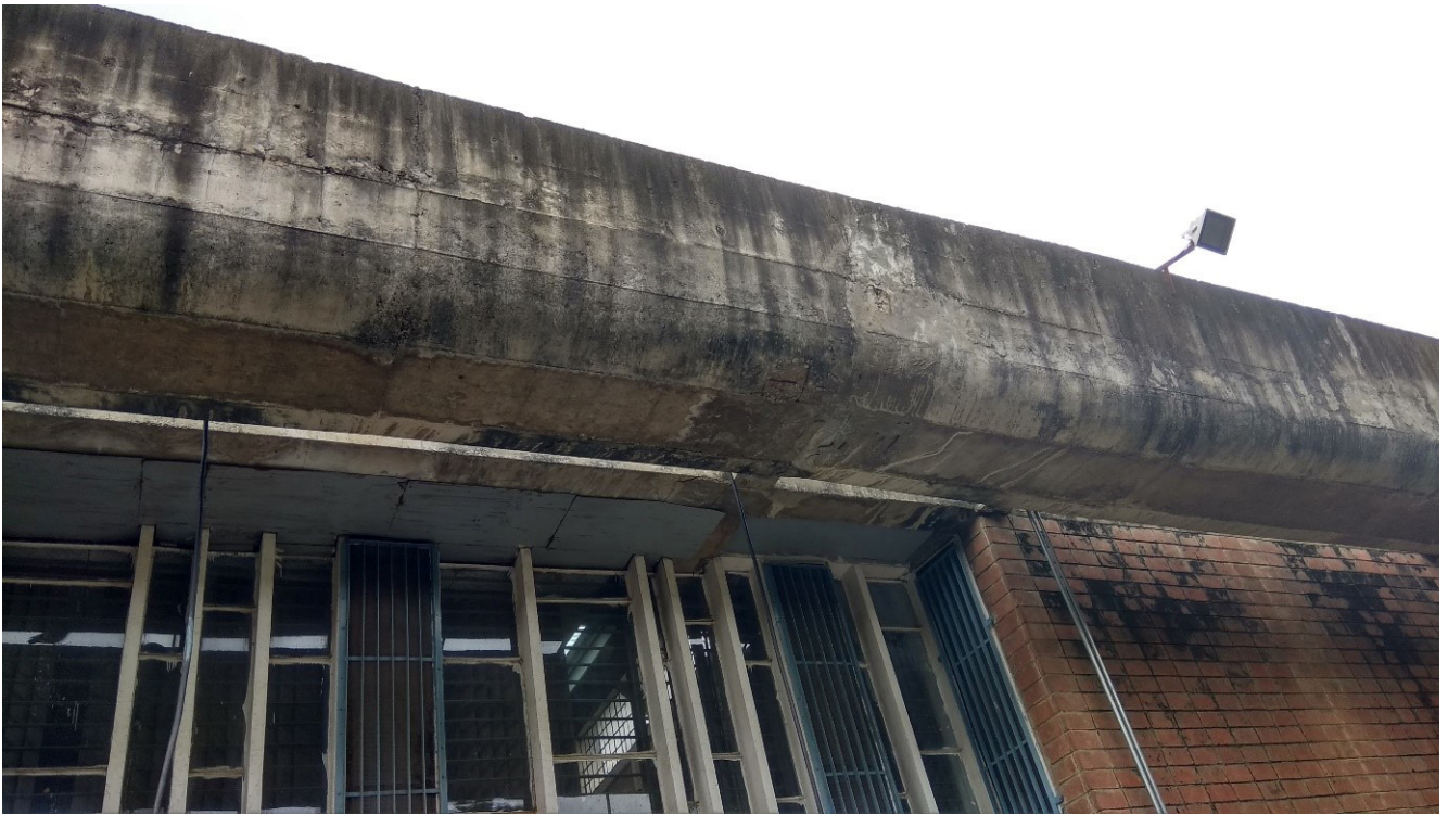
Fig. 124: Patch repair of concrete drains
