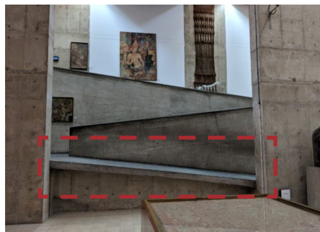
Fig. 234: Open edge of the ramp should be provided with railing
