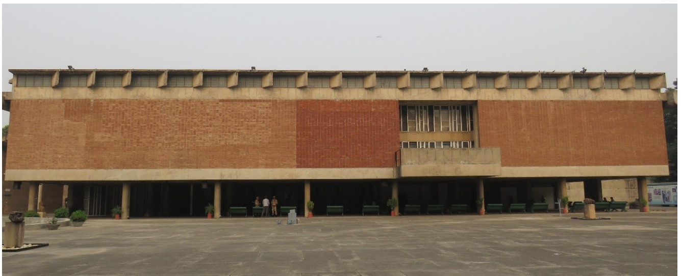
Fig. 101: South-west façade of the building with sun protection system. Source: DRONAH
