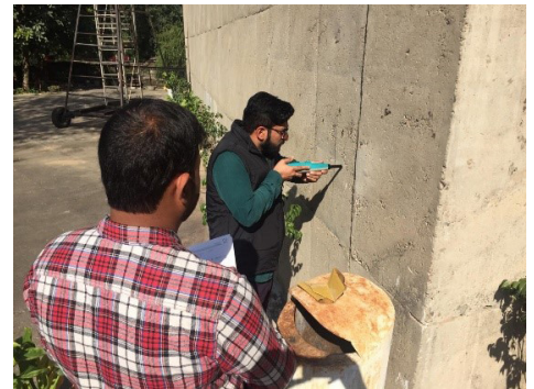
Fig. 163: Core Rebound Hammer testing
