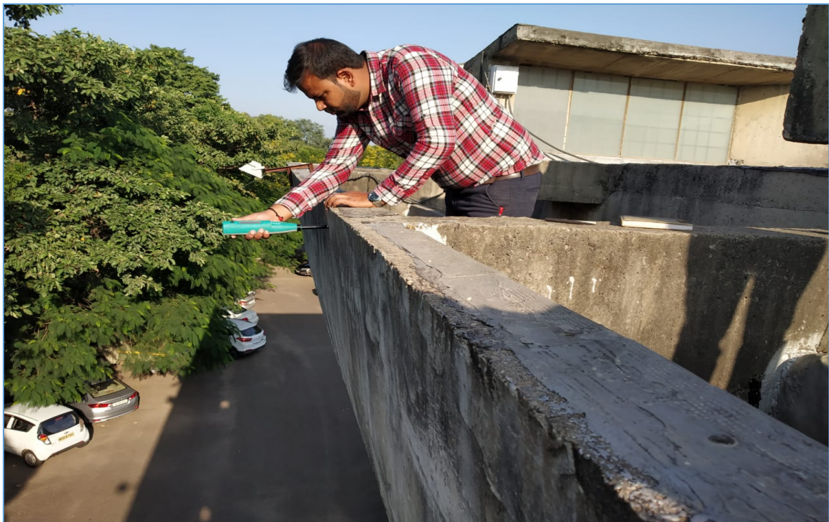
Figure 4 Rebound hammer Test at wall of Gargwell (rainwater drain at roof).
