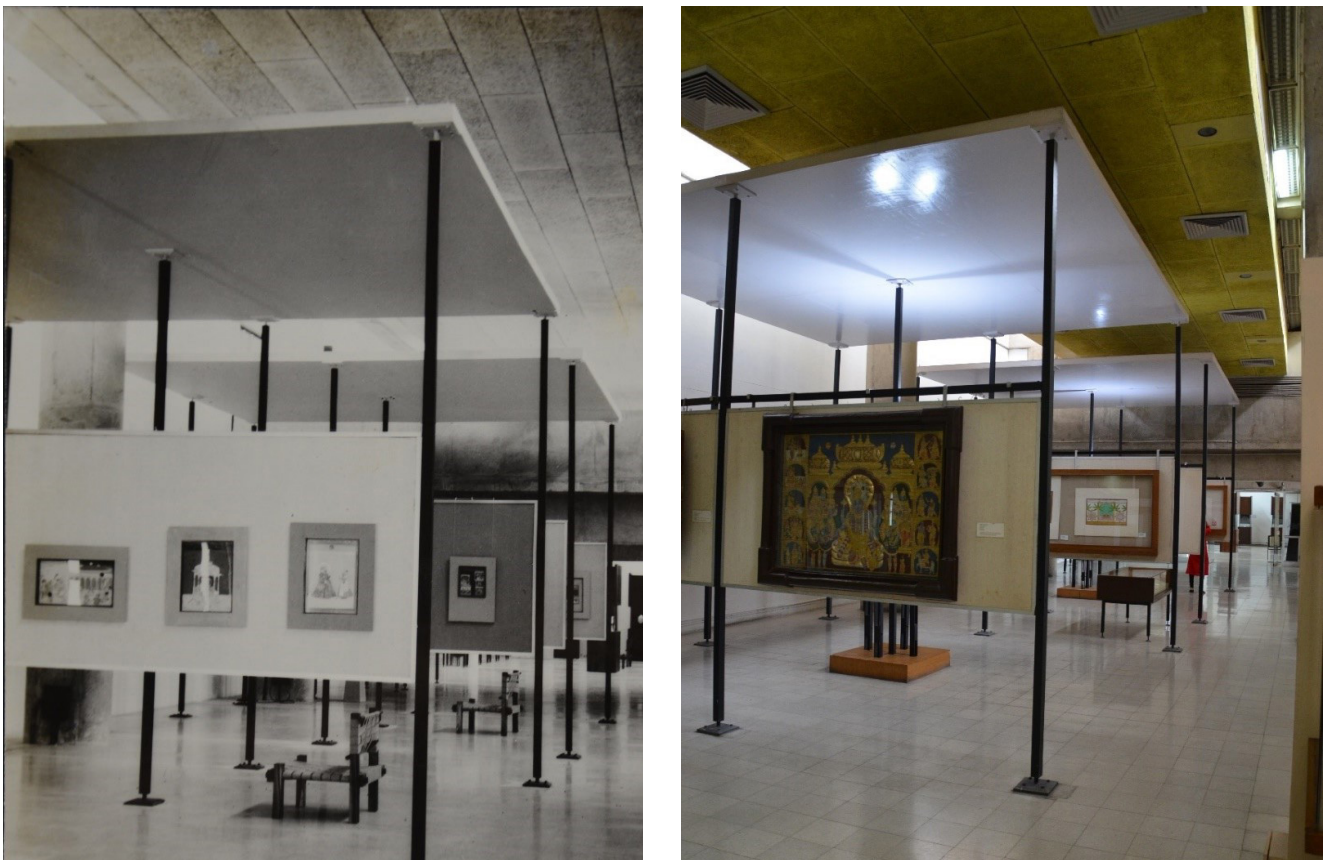
Fig. 113: Addition of air conditioning units has brought down the ceiling level in the gallery dampening the spatial quality.
