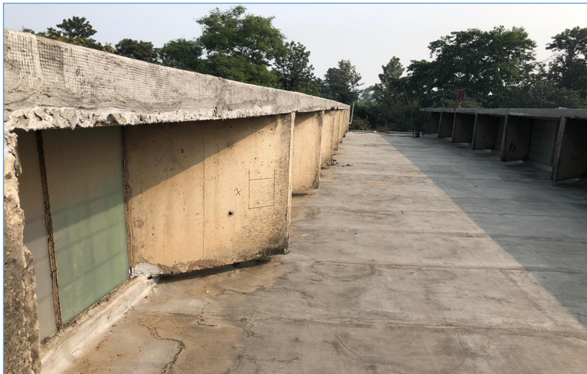
Figure 2 Extended fins at roof top of the building.
