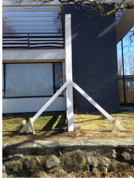
Figures 3 and 4: West trellis: failing timber (left) and new stabilization techniques (right), 2016 RS ID #263883 and RS ID #263888
