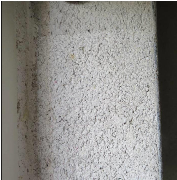
Figure 35. MasonRE test patch, post-treatment.
