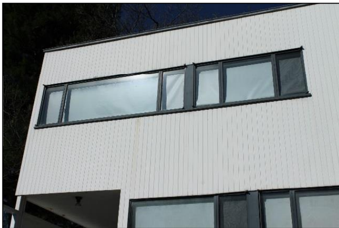
Vertical board siding on east elevation
