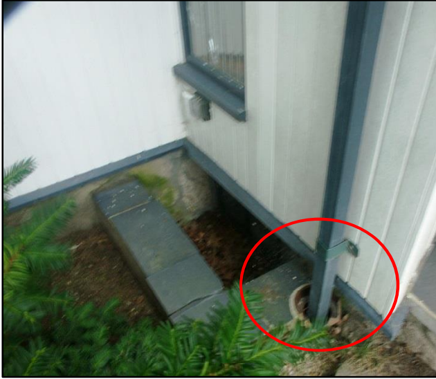
Downspouts of front entry porch draining to underground clay tile pipes
