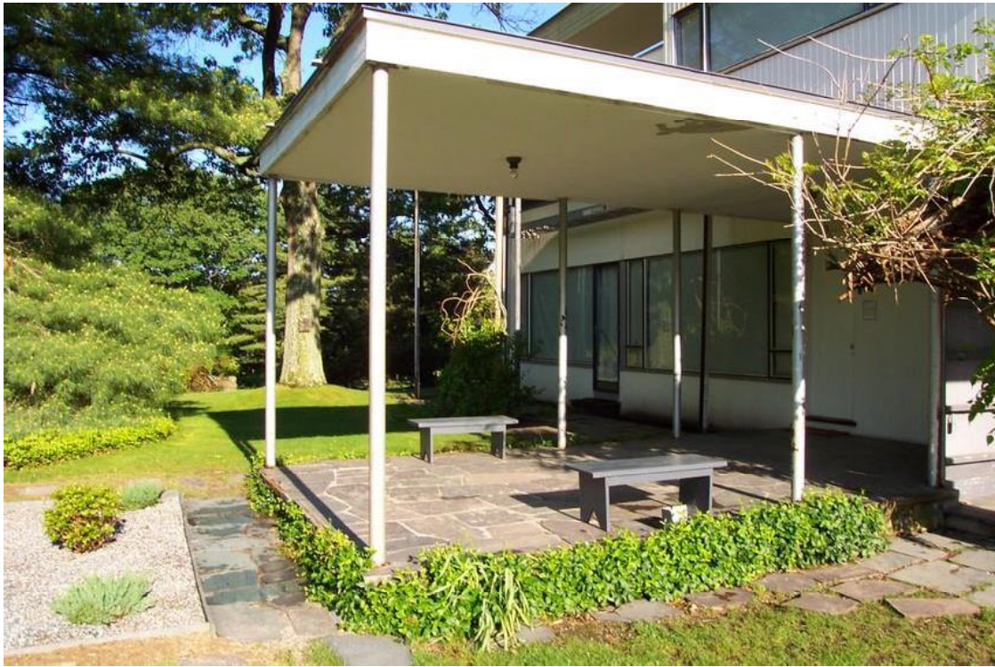
Figure 7: Screen porch during 2001 repairs RS ID #57137
