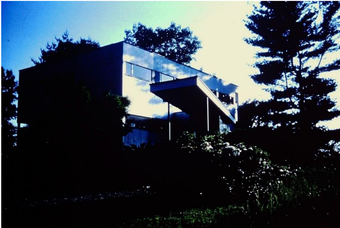
Figure 3: North façade, including the flat marquee roof, 1965
