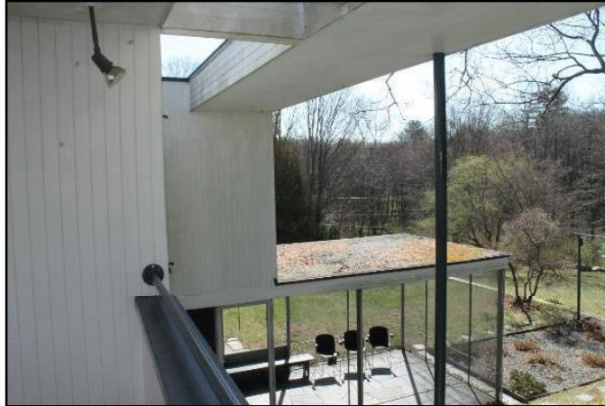
Roof over south elevation screen porch
