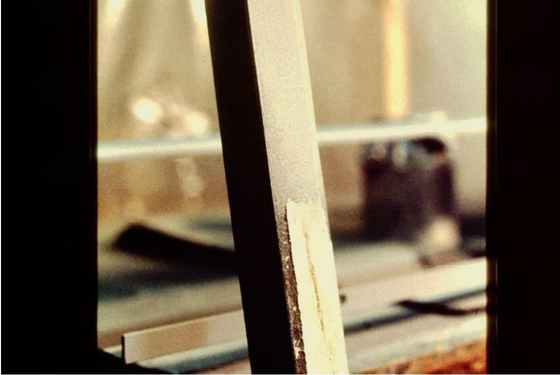
Figure 6: Steel window frame during grit blasting, 1995 Historic New England Property Care Binder, Lyman Estate
