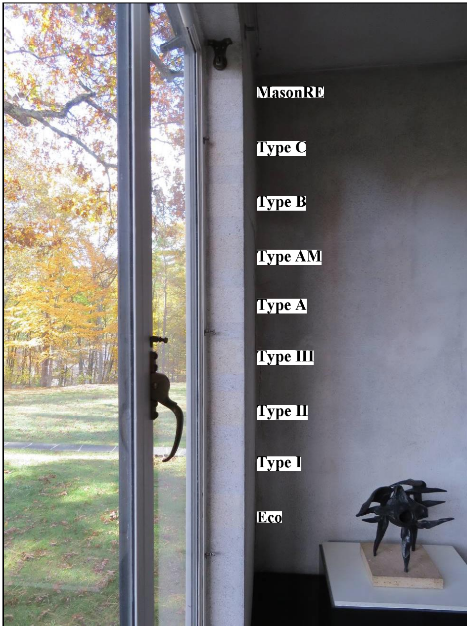
Figure 36. Poultice test area, post treatment (product names positioned next to test patch location).
