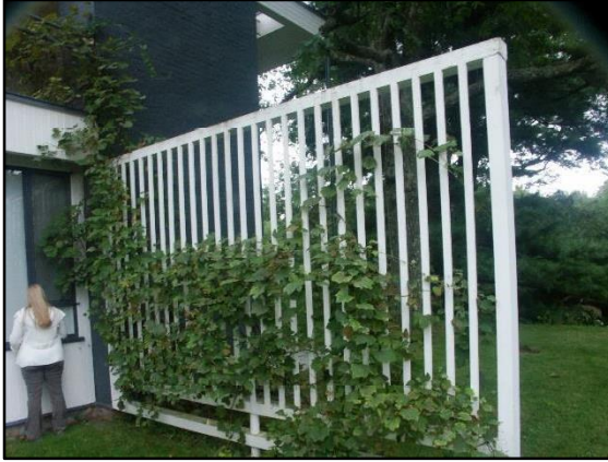
Trellis at western elevation
