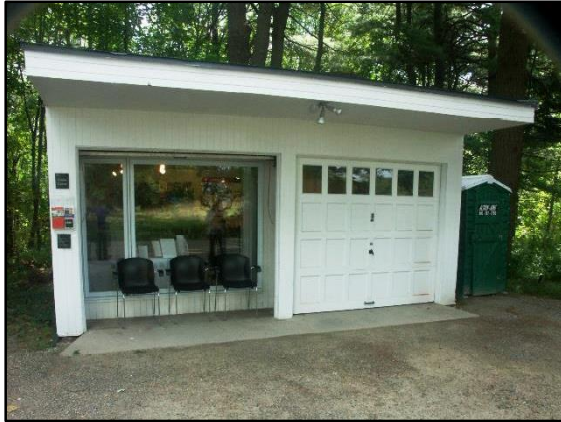
Window arrangement on front elevation
