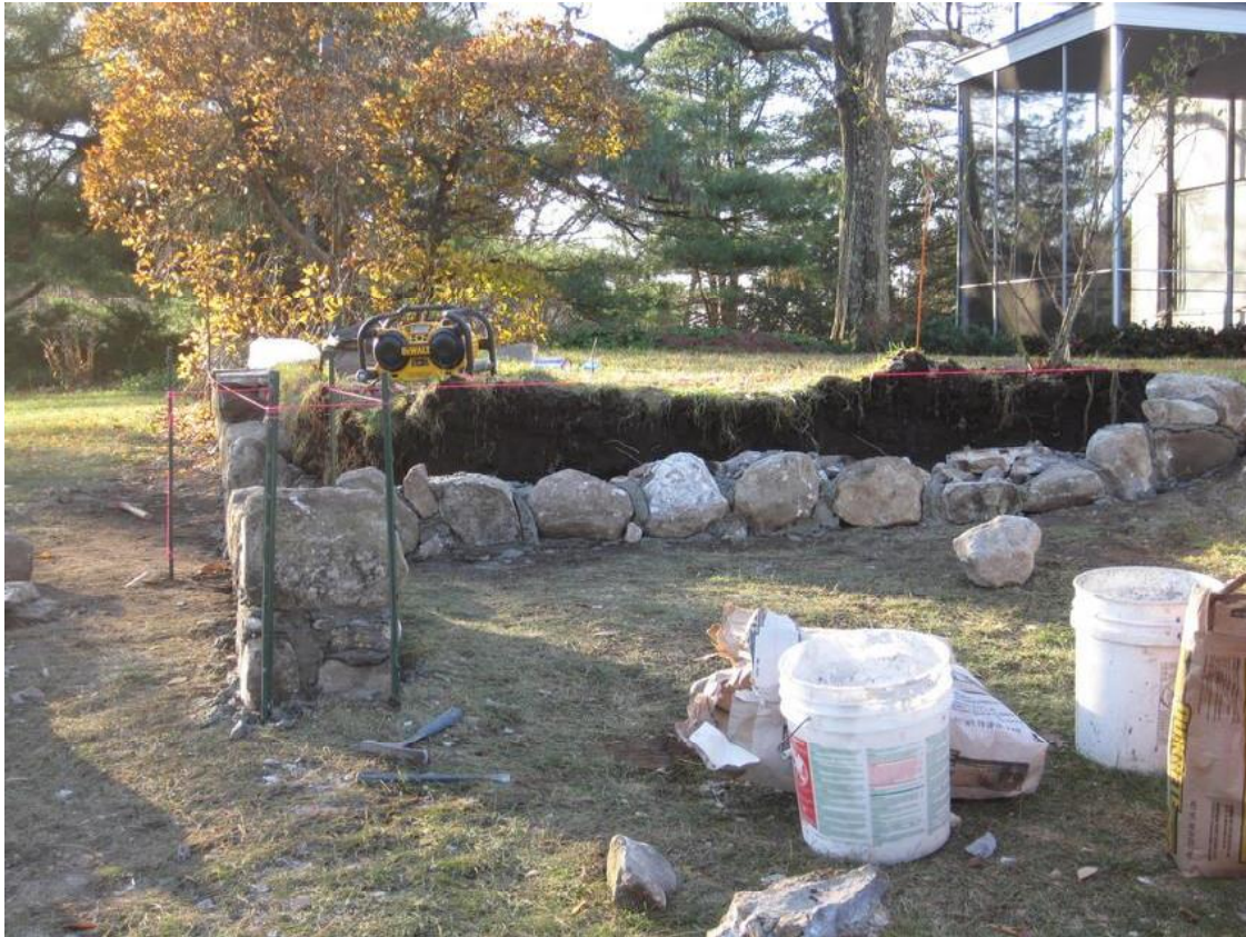
Figure 6: Stone wall repair, 2009 RS ID #46978
