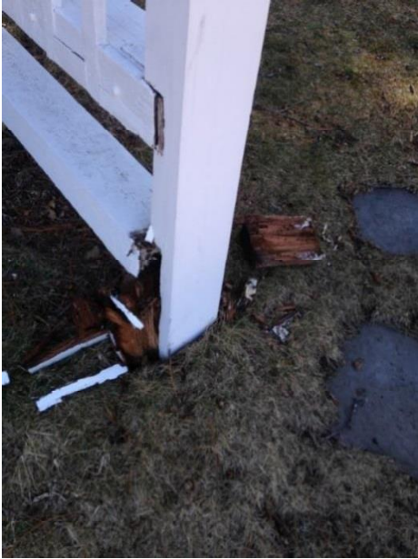
Figures 3 and 4: West trellis: failing timber (left) and new stabilization techniques (right), 2016 RS ID #263883 and RS ID #263888
