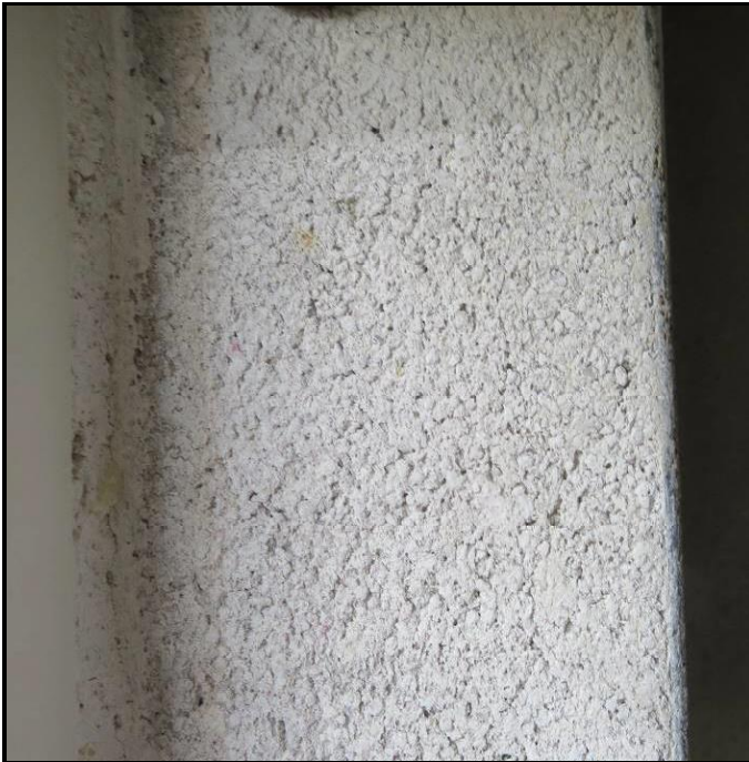
Figure 35. MasonRE test patch, post-treatment.
