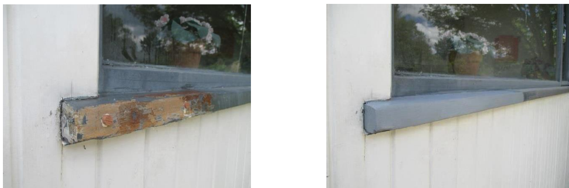
Figures 9 and 10: Sill repair, 2015 RS ID #249326 and RS ID #249330
