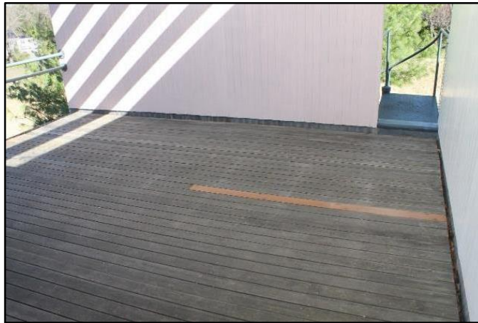
Decking of roof porch; Built-up asphalt and gravel roof underneath
