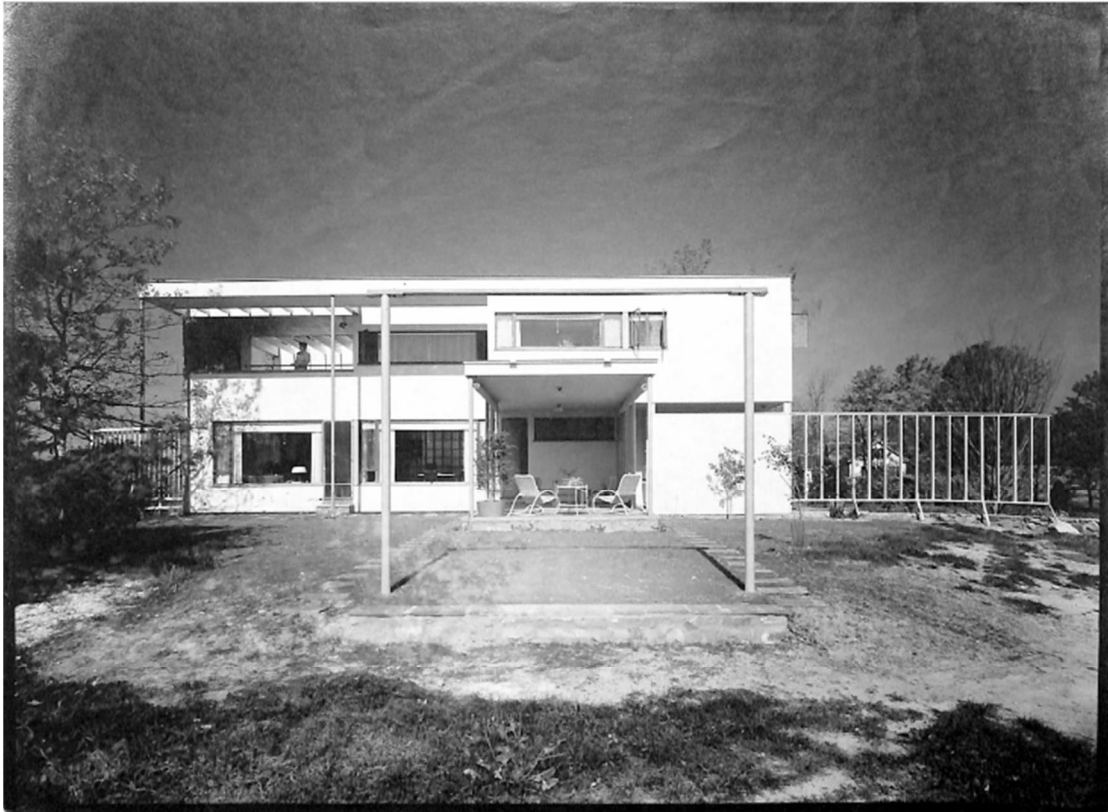
Figure 3: Steppingstones around porch and perennial garden bed, Paul Davis, 1939-40 Historic New England Archives
