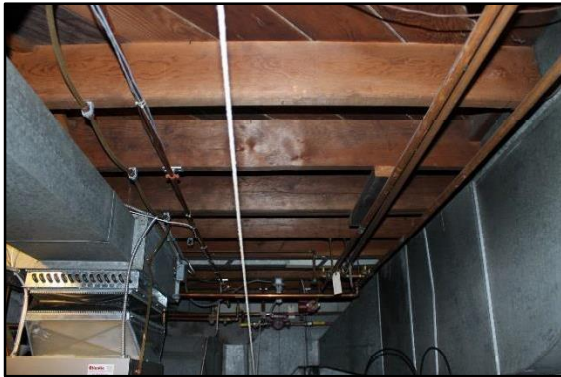
Nominal 2" framing stock as visible in the basement
