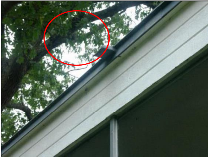
Scupper on south elevation of screen porch
