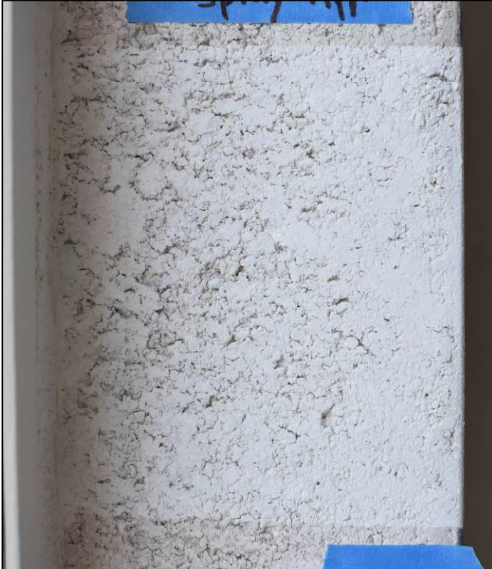
Figure 43. Spray-applied Acrylic-modified Type S limewash test patch.
