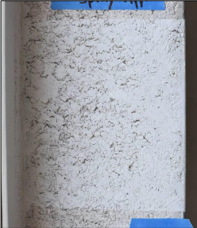
Figure 43. Spray-applied Acrylic-modified Type S limewash test patch.
