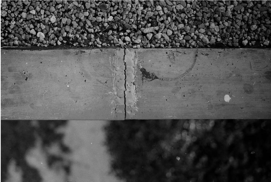
Figure 6: Solder joint of flashing, circa early 1990s Historic New England, Property Care Files
