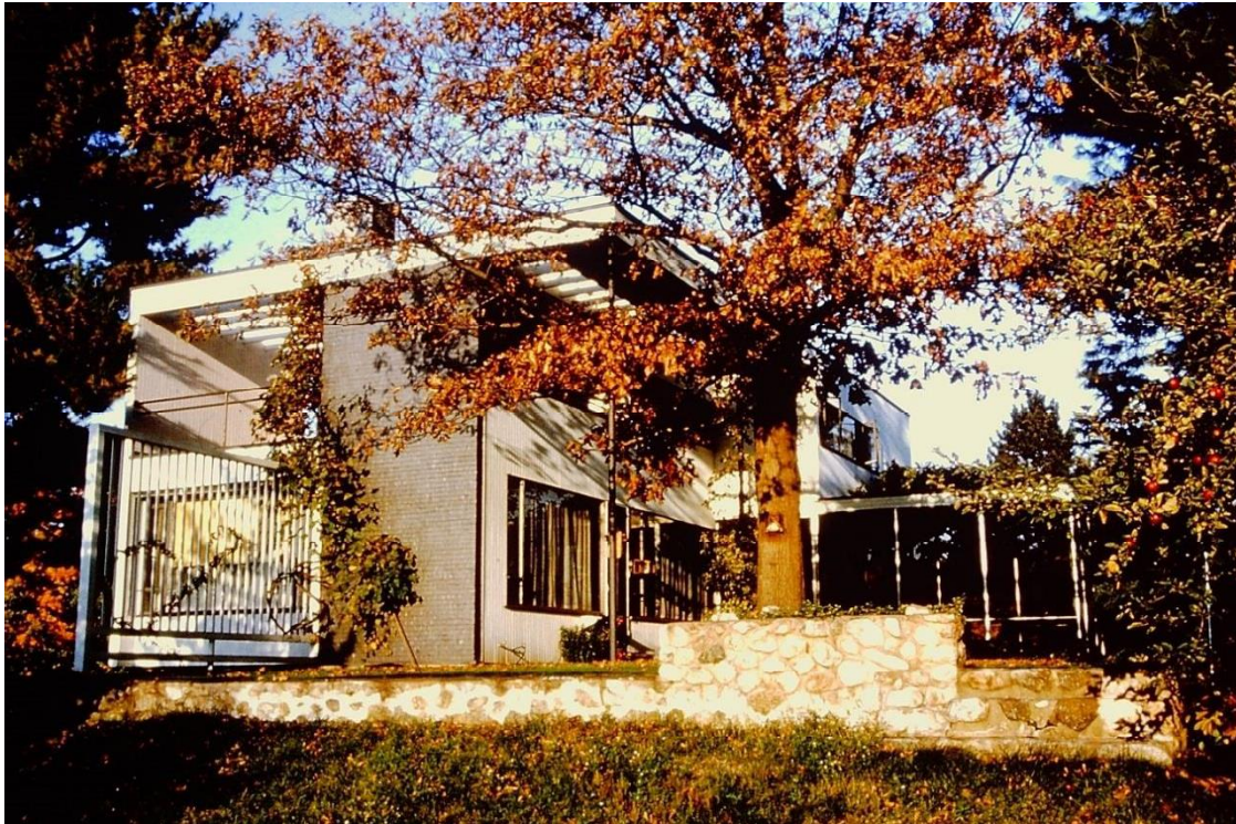
Figure 4: Gropius stone wall with mortar and flagstone clapping, circa 1967-68 Historic New England Archives, Binder of Slides
