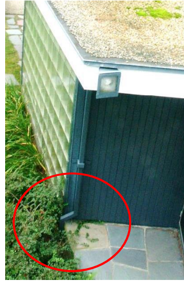
Downspouts of front entry porch draining to underground clay tile pipes
