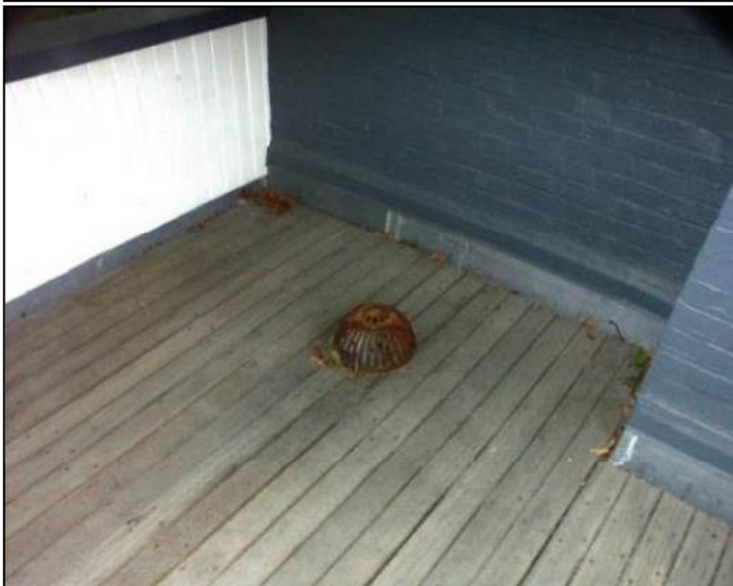
Drain on second floor porch deck
