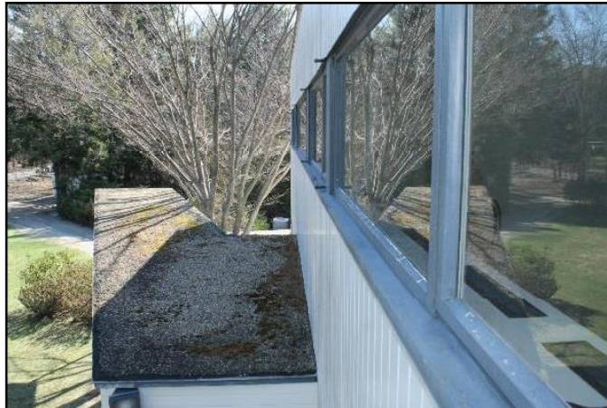
Roof over front entry walk way
