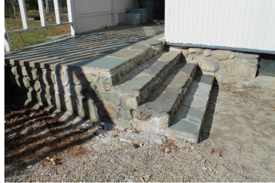
Rear entry steps – general conditions
