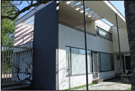
Column supports on south elevation
