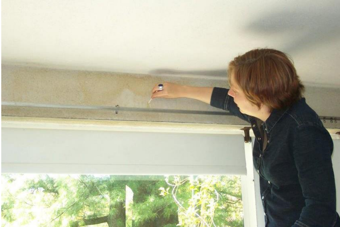
Figure 4: Acoustical plaster is treated with paint layers, 2002 RS #57099
