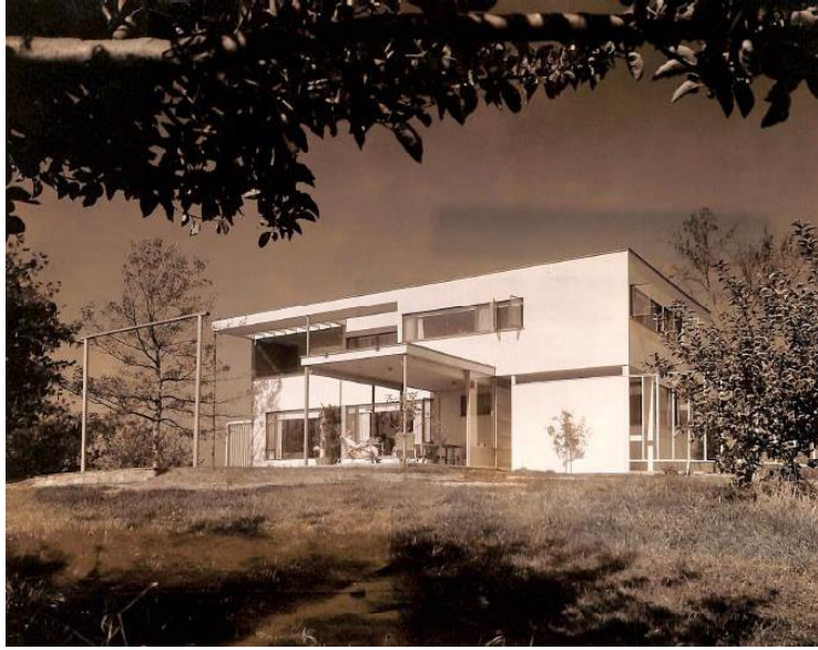
Figure 2: Gropius House south elevation, Paul Davis, 1938 Historic New England Archives
