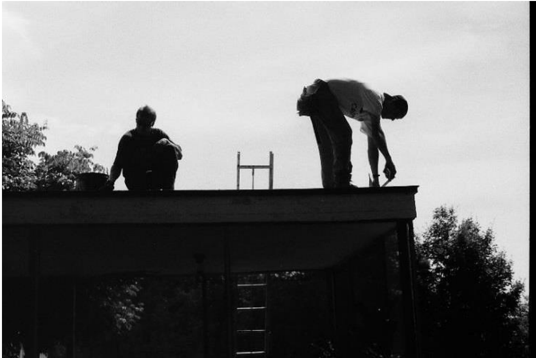
Figure 6: Screen Porch Roof testing, 1996 Historic New England, Property Care Binders
