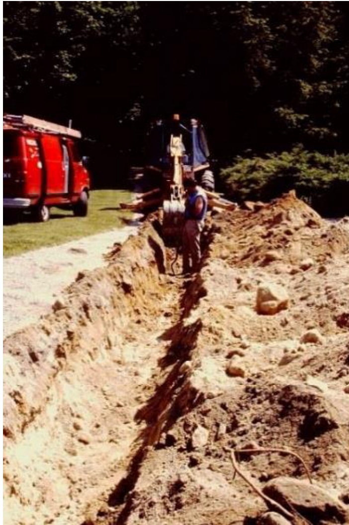
Figure 9: Trench dug in the driveway, 1997 Historic New England Property Care Binders
