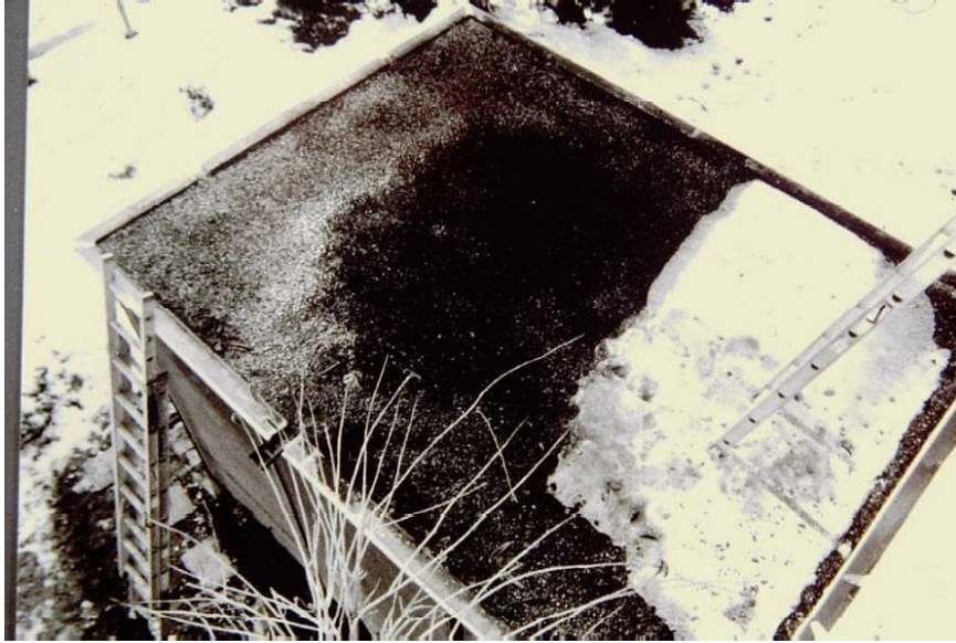
Figure 5: Porch roof, 1990 Historic New England, Property Care Files
