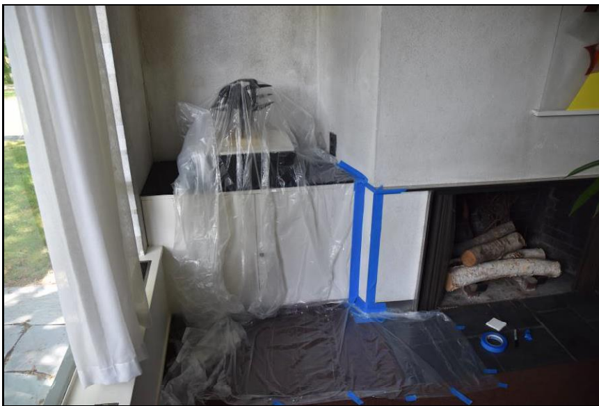
Figure 26. Location of pigmented limewash test patch (outlined in blue tape) adjacent to living room fireplace.
