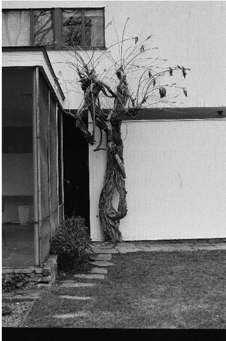
Figure 8: Flagstones along the porch and south façade, 1994 Historic New England Property Care Binders
