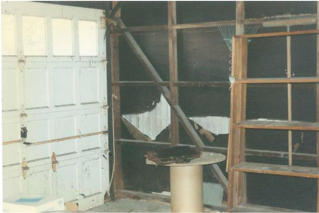
Figure 3: Garage framing, circa 1990s Historic New England, Property Care Binders
