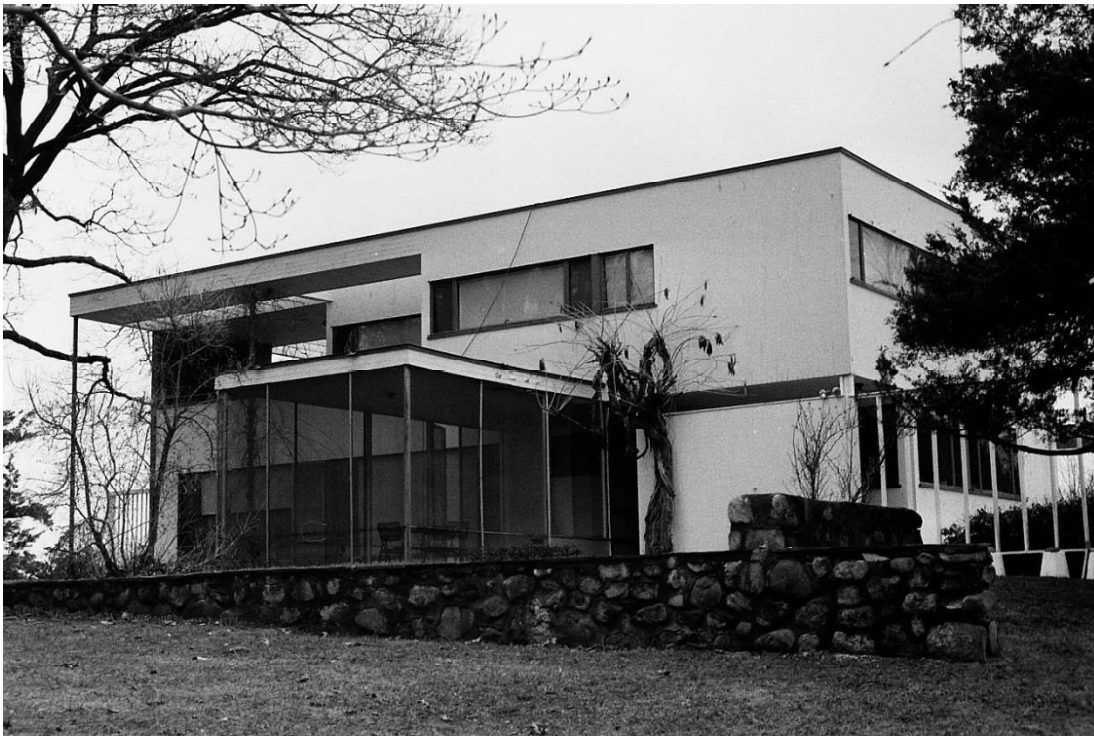
Figure 3: Retaining walls reflecting edges of house, 1994 Historic New England Property Care Files
