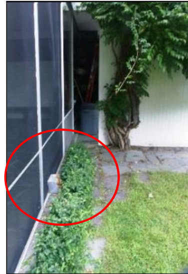
Water deflector on east elevation of screen porch
