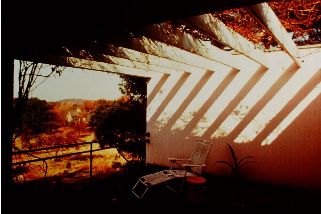
Figure 4: Roof deck, 1977 Historic New England Archives, Binder of Slides
