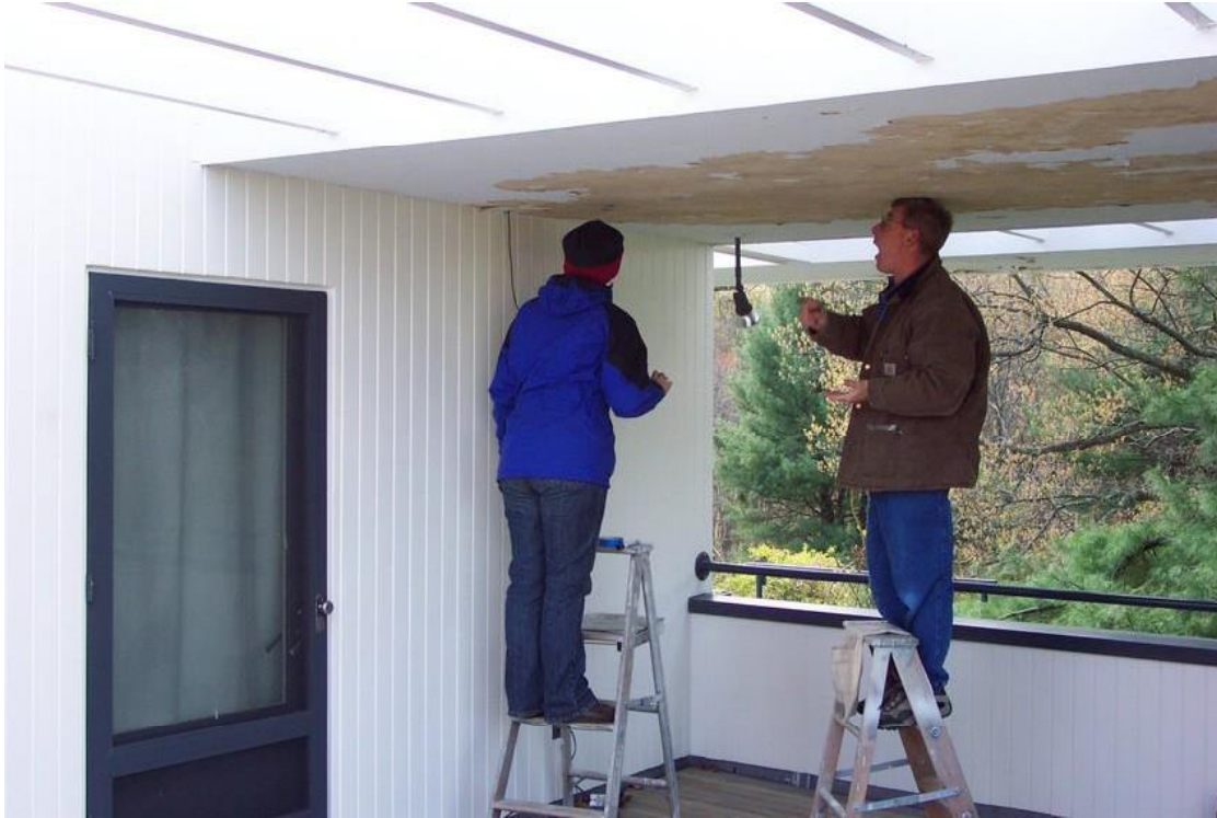
Figure 5: Roof deck ceiling repair or replacement, 2002 RS ID #57056
