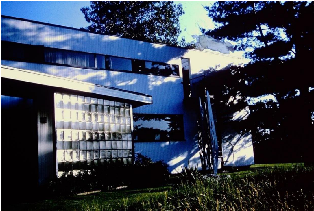
Figure 2: Exterior glass block wall, 1965 Historic New England Archives, Binder of Slides
