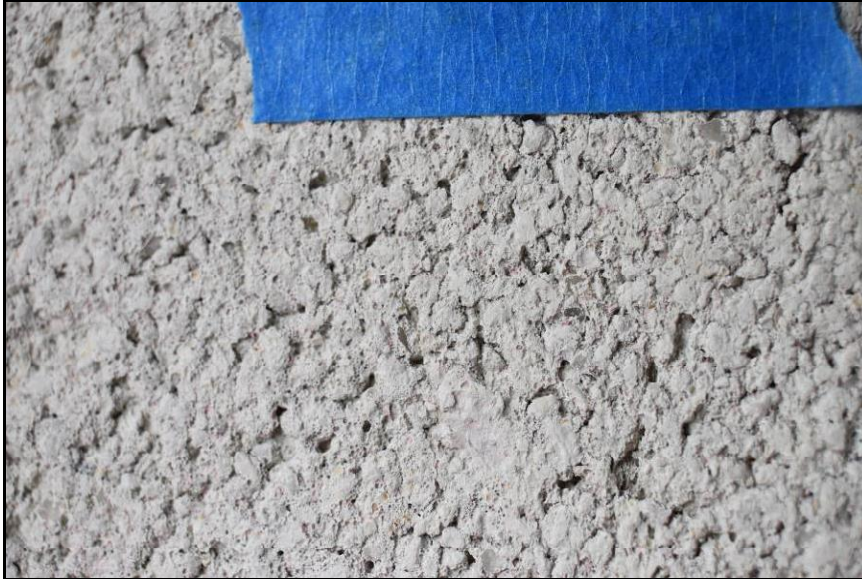
Figure 19. Close-up of plaster in living room showing typical surface texture.
