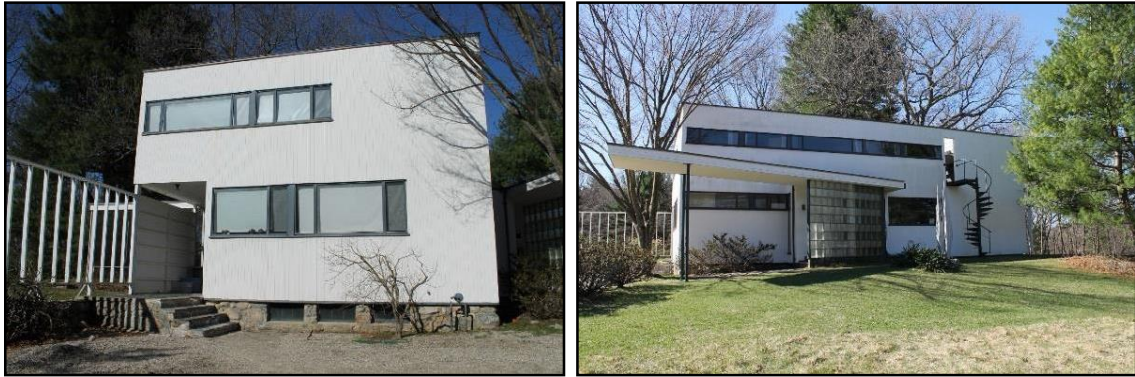
Windows on the east and north elevations
