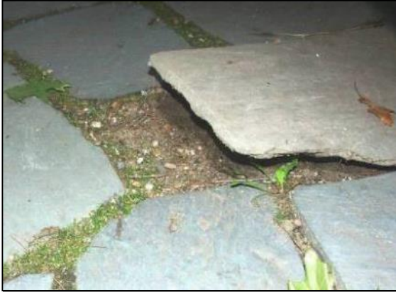
Shifting paving stones
