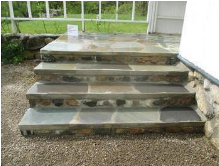
Figure 4: Kitchen steps after nosing repair, 2016 RS ID #278687
