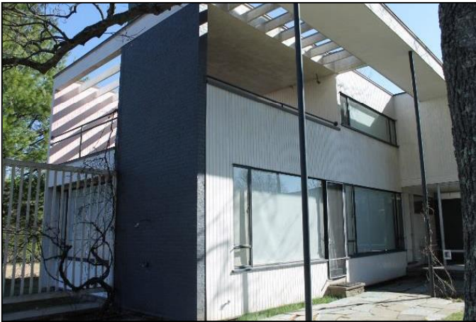
Brick fireplace wall on west elevation
