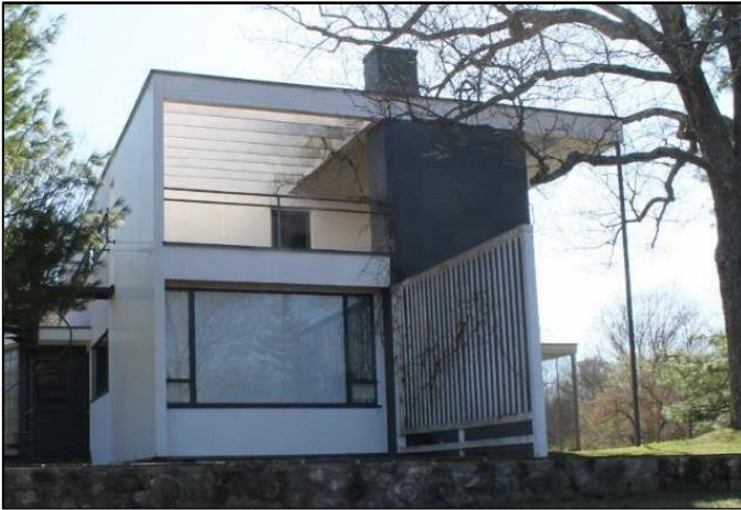
Brick and glass west elevation
