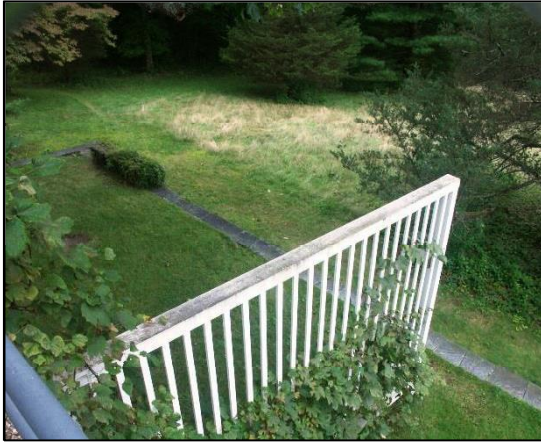
Trellis on western elevation
