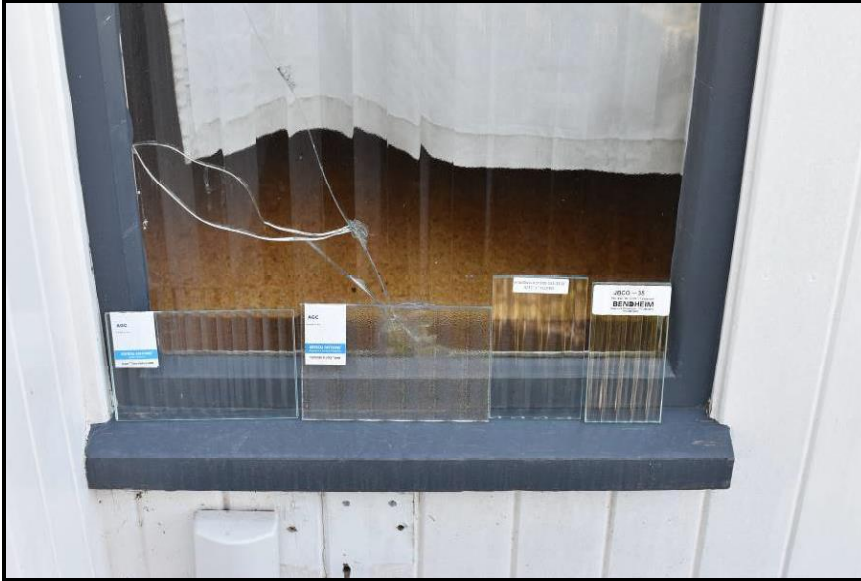
Figure 17. Samples of replacement glass compared to original Louvrex glass in Window 109 (east elevation). Samples (left to right): AGC “Flutes” Clear Pattern, AGC “Textured Flutex”, Gray Glass “1-inch Fluted”, Bendheim’s JBCO-35.
