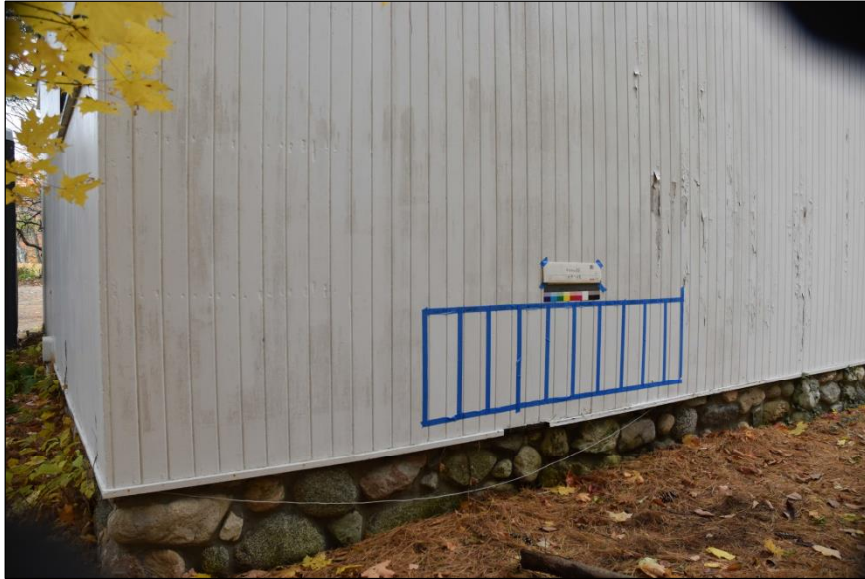
Figure 12. Cleaning test location on east elevation of the detached garage.
