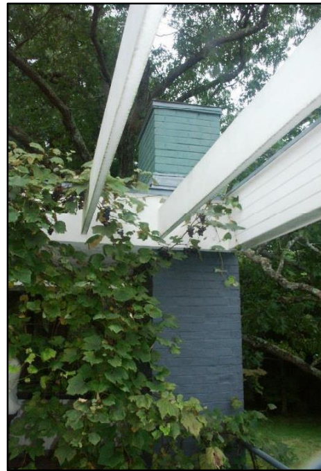
Inactive chimney on west elevation
