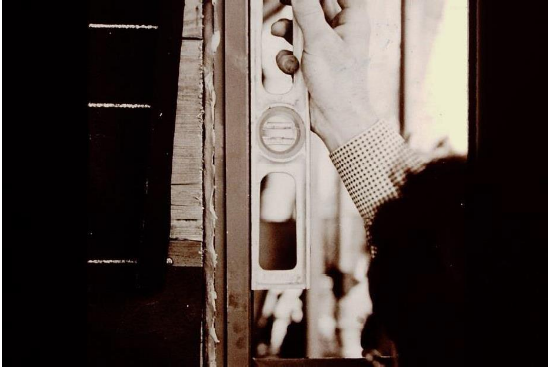
Figure 2: Installation of the windows, 1938 Historic New England Archives, Binder of Slides
