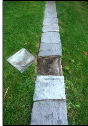
Stone capped walls (above)
