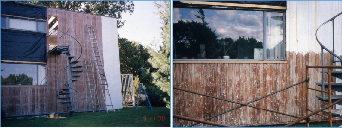
Figures 5 and 6: Exterior paint is stripped, 1998 Historic New England, Property Care Binders
