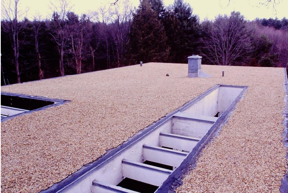
Figure 7: New roof from west, 1999 Historic New England, Property Care Files
