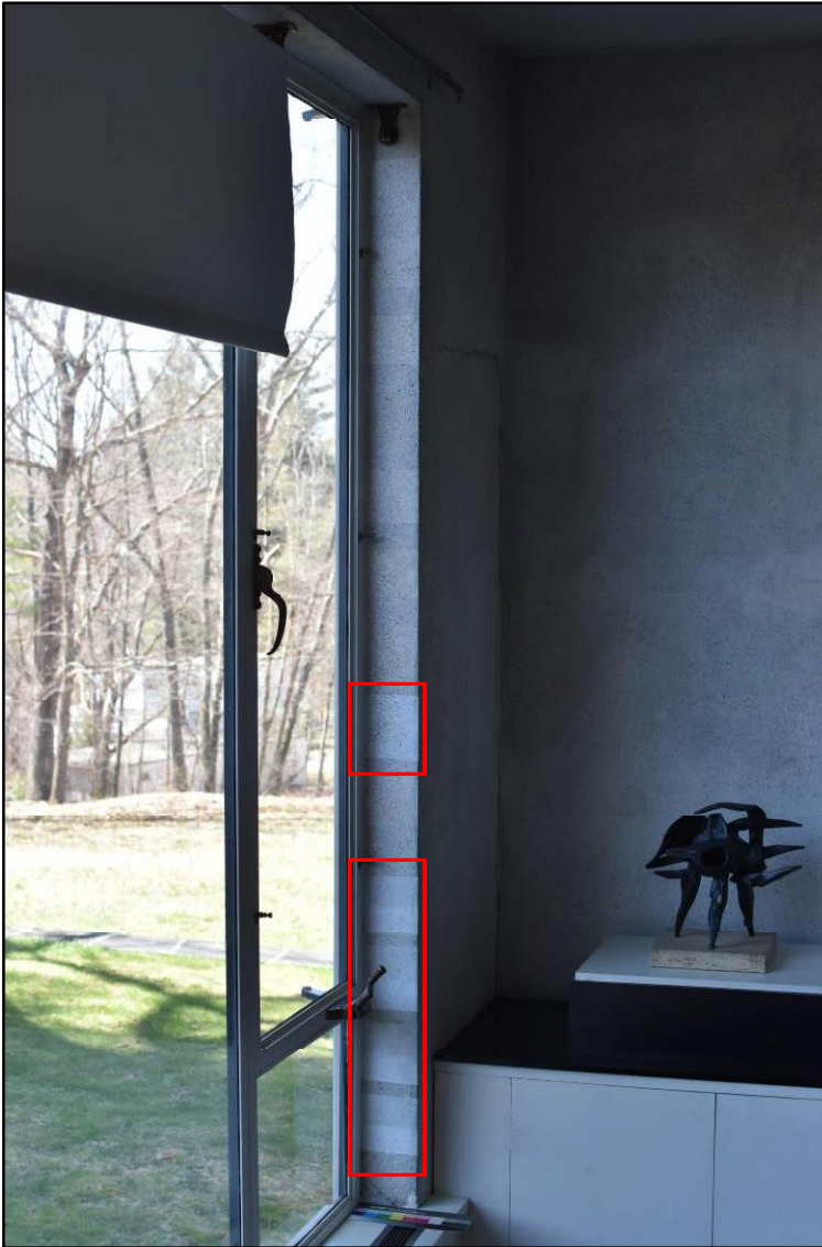
Figure 25. Location of limewash test patches (outlined in red) on window return in living room.
