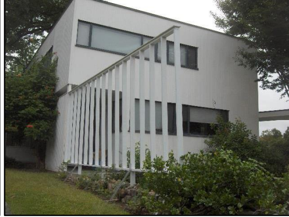
Trellis at eastern elevation
