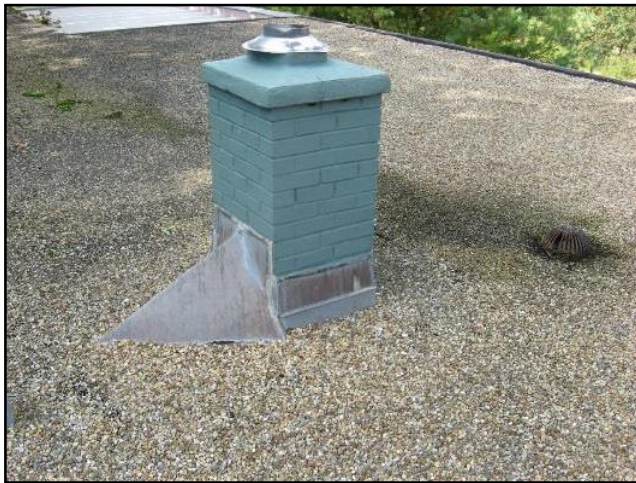
Active chimney in center of building
