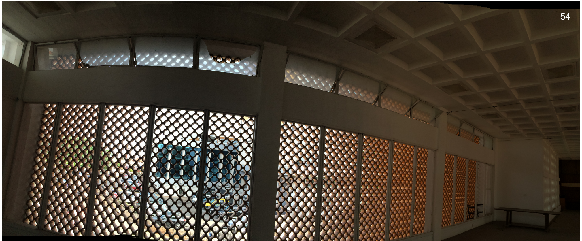
54 Photo of the louvre sections to be replaced (Tuuli Saarela)
