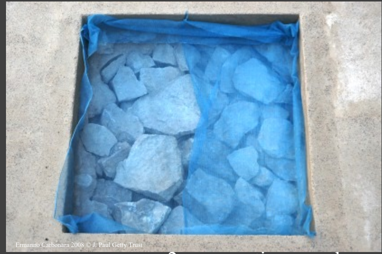
2 – separation membrane
