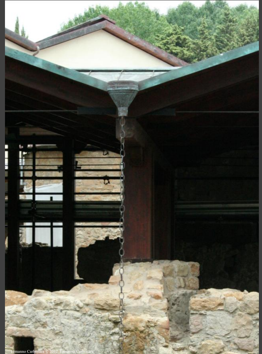
Rain water chain
