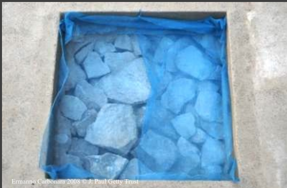
2 – separation membrane
