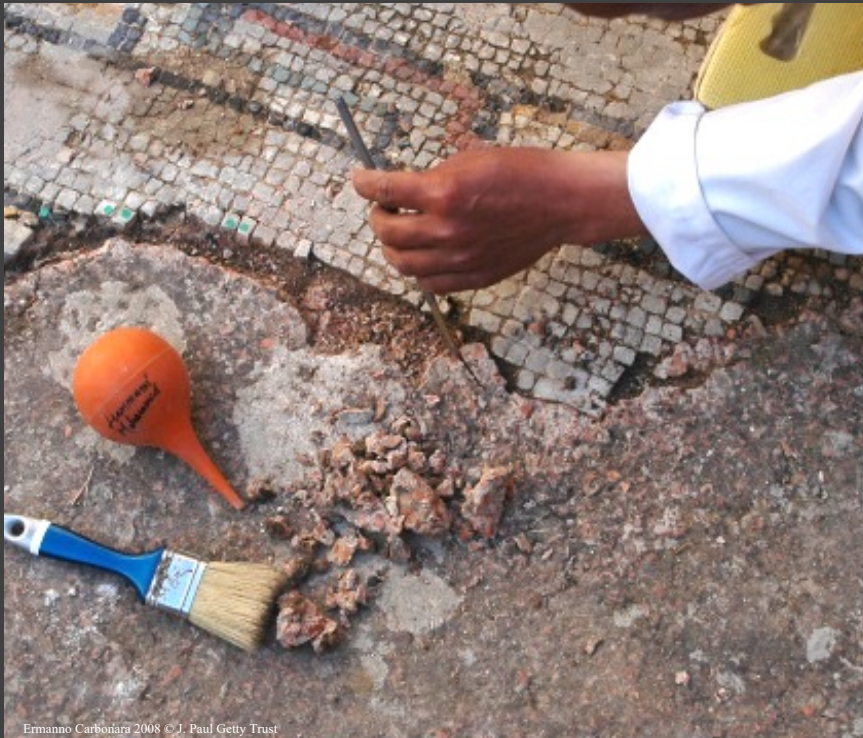
Removal of modern repair mortars with a chisel and small hammer
