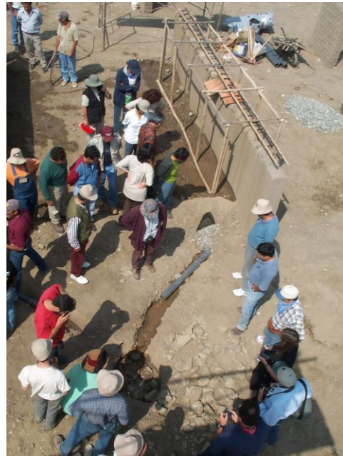
Figure 5.1.3 View of French drain installation PAT course, 1999 © J. Paul Getty Trust
