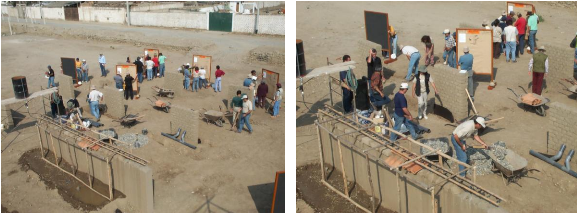
Figure 5.1.4 (left) and 5.1.5 (right) PAT students working on different drainage installation systems at test walls PAT course, 1999 © J. Paul Getty Trust
