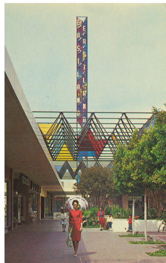
Eastland Shopping Center, about 1957, A. C. Martin and Associates. Photo by David M. Mills. Chris Nichols Collection
