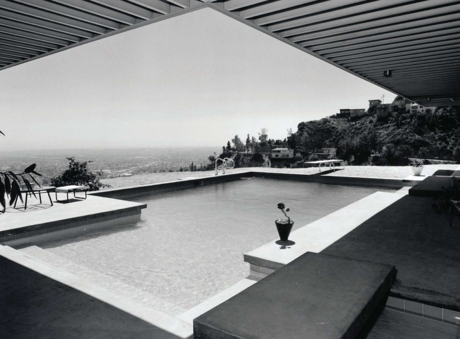
Case Study House No. 22, Los Angeles, 1960, Pierre Koenig, architect. Black and white negative. Used with permission. Julius Shulman Photography Archive. The Getty Research Institute. © J. Paul Getty Trust. One of the 6,500 Shulman images in the Artstor Digital Library.
