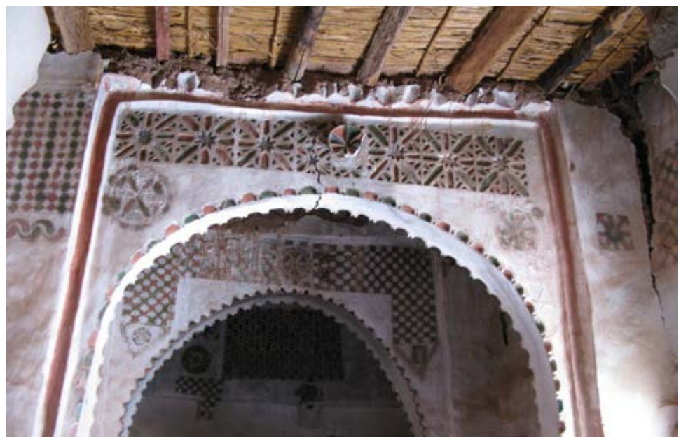
FIGURE 4.43 Detail of sagging arches leading to structural cracks separating the painted arches from the walls. Photo: Lorinda Wong, 2013.
