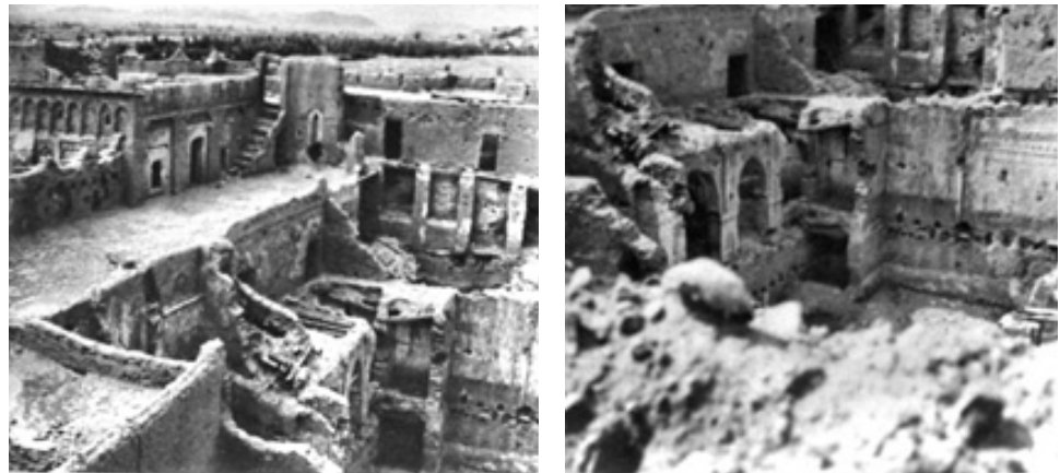
FIGURES 4.33 AND 4.34 The area of collapse to the south and southwest is revealed by photographs taken ca. 1970. Photos: CERKAS collection.
