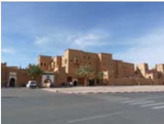
FIGURE 1 North view of Kasbah Taourirt. Photo: Susan Macdonald, 2011.
