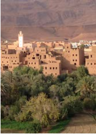
FIGURE 1.2 Ksar Aït Boujane, Todgha Valley. Photo: Elena Macchioni, 2013.
