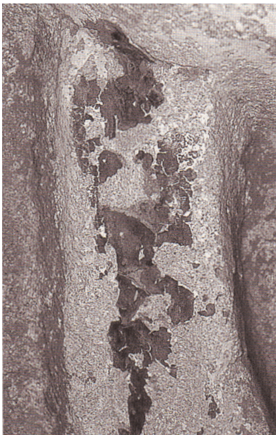
Figure 7 Cave 6, stupa pillar, east face, lower story, lower part of third figure from west, enlarged detail showing traces of paint layer flaking from the stone support. Large amounts of dust are deposited at the feet of the figure and also behind the flakes of the paint.
