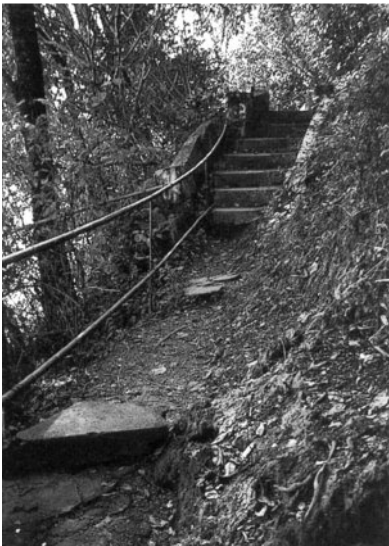
Figure 9 Eroded pathway joining the two caves.
