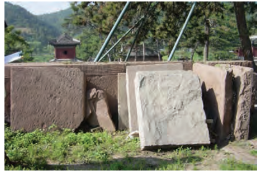
28、槛墙陡板 vertical sill wall ashlars
