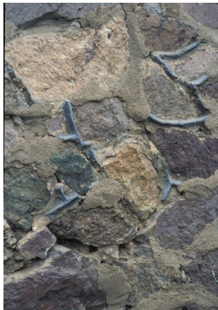
39. 下层月台护坡墙中的水泥和原始青灰勾缝 Cement and original lime mortar of retaining wall, Lower Terrace
