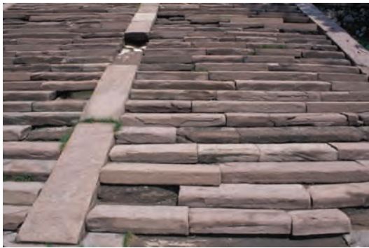
34. 台阶和垂带的近景 Close-up of stairway and splay
