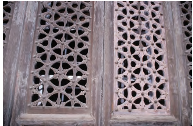
62. 隔扇棂心 Detail of lattice on doors
