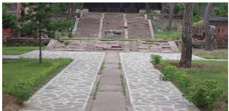
13. 第一进院落内用水泥重新铺的冰纹甬路 Crazy-paving re-laid with cement in Courtyard 1
