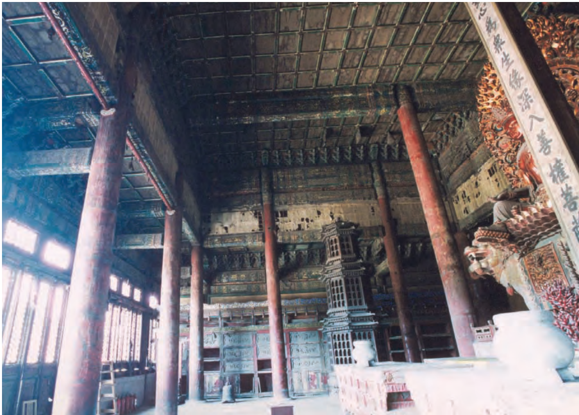
71. 从殿内朝西；天花板 Interior, looking west and at ceiling
