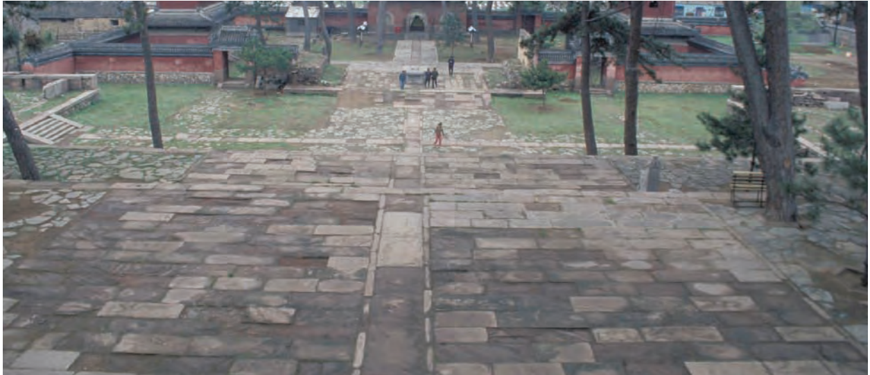
46. 上层月台铺石埧地（朝南） Paving of Upper Terrace, looking south
