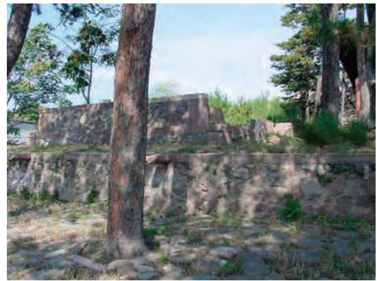
48. 下层月台松树树池Edging stones for trees on Lower Terrace
