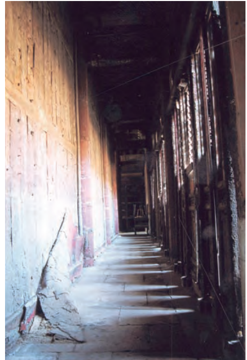
73. 殿内北面小通道 Corridor along north side of interior
