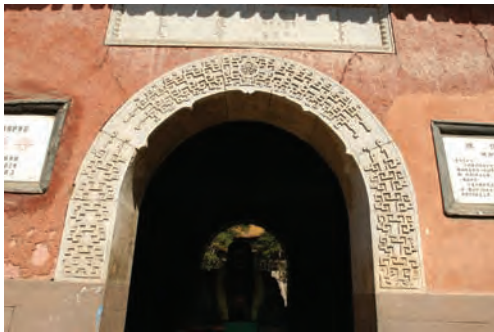
5.石半圆盲窗（上边），石卷门（下边） Details of stone window (above) and door surround (below)
