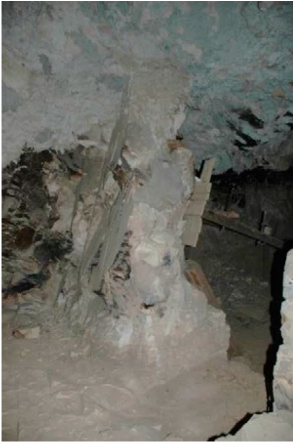
Shoring supporting fragile remains of heavily fractured rock of wall between chambers (C) and (E), west of doorway (D).
