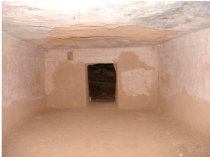
General view of burial chamber (C) and doorway (D), looking south toward rear chamber (E). There are large plaster losses throughout the main chamber that have been repaired with plaster fills.
