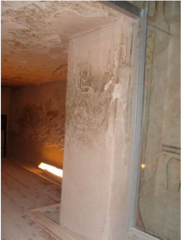
The jambs of doorway (J) leading into the rear chamber (K) are unprotected and show signs of visitors touching the walls. This area should be protected.
