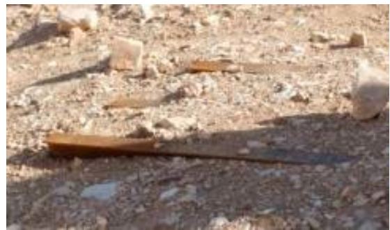
Detail of exposed, steel cross-braces supporting masonry surround and requiring attention.
