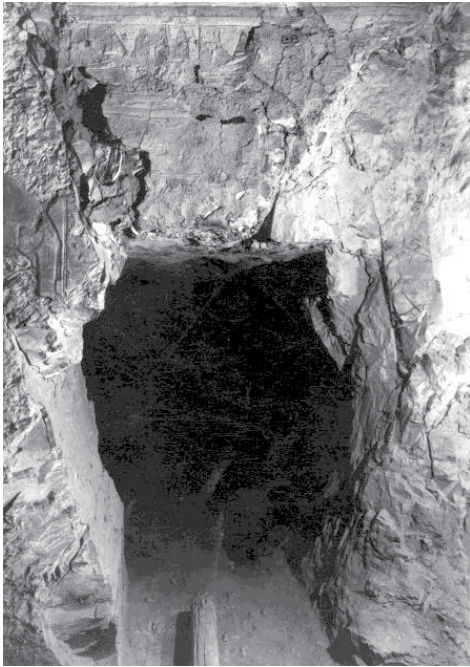
A photograph from 1986 shows rock loss in doorway (H) which may be related to flood damage. The photo at right shows the reconstructed doorway as it appeared in 2006 (Image: CEDAE).
