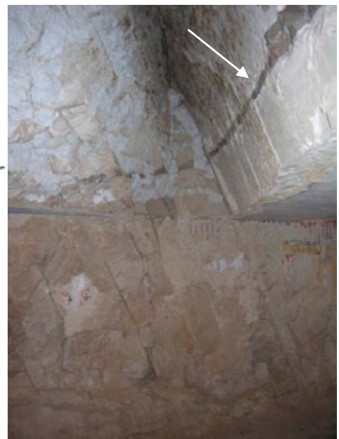
Large fracture at apex of wedge-shaped area of rock loss in ceiling of main chamber (C) shown on isometric plan and in photo, above Note dark diagonal band of chert across area of loss (arrow).
