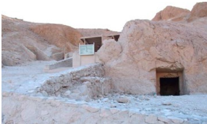
Approach to tomb and retaining wall along visitor path with entrance and shelter for QV 44 left and above.
