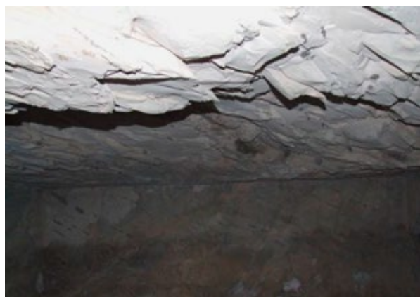
Fractured ceiling rock in chamber (K).
