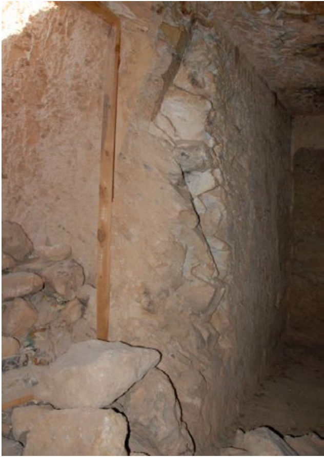
Rock loss and some adjacent loose fragments at doorway (B) west jamb. (Image: CEDAE 2009).
