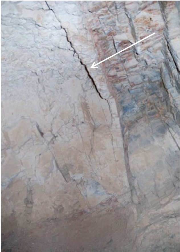
East wall of rear chamber (E) has vertical and diagonal open fractures in the marl which follow the orientation of the shale layer below.
