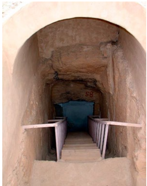
Entry ramp (A) with arched cover and masonry walls, wooden stairs with handrails installed over the original stepped ramp, and exterior metal door without ventilation holes.
