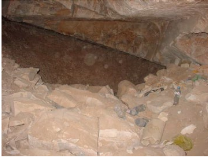
Rock from ceiling collapse in chamber (C).
