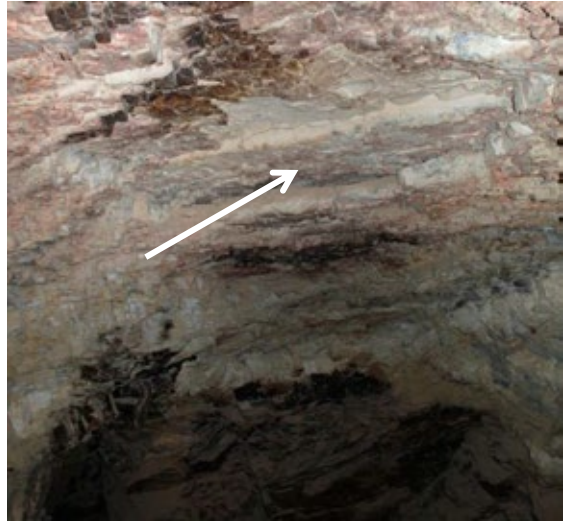
Delaminated shelf (arrow) in the ceiling of QV 15 chamber (C).
