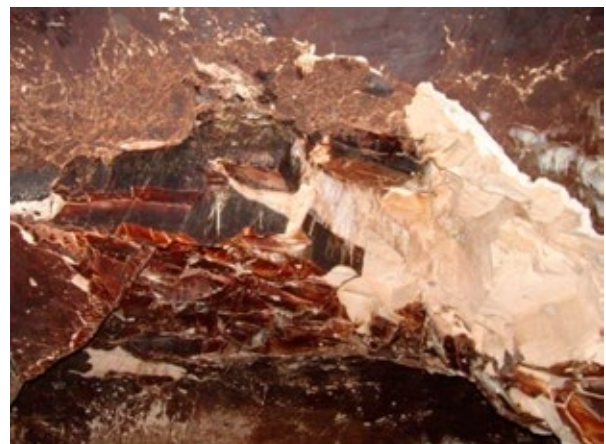
Post-fire rock loss in ceiling of chamber (E) above Pillar III.
