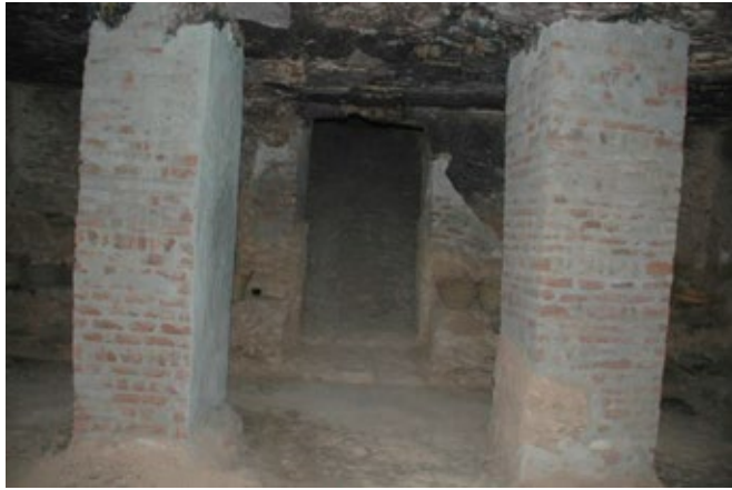
Reconstructed pillars in burial chamber (G) and door jambs of doorway (F) built using modern fired bricks.
