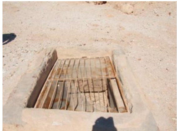
Shaft entrance prior to the installation of the prototype shaft cover in 2008.
