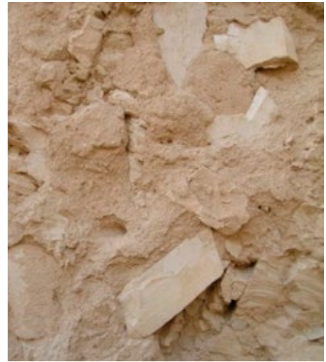
Exposed infill plaster with rock shards on walls of entrance ramp (A).
