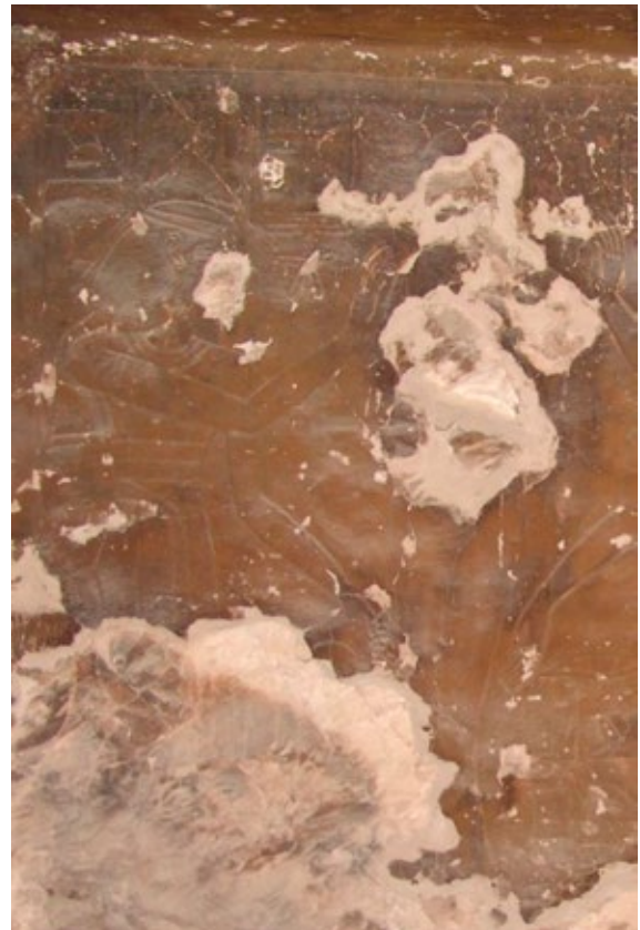
Chamber (I) in 2008 showing same area with 1989/1991 edging repairs.
