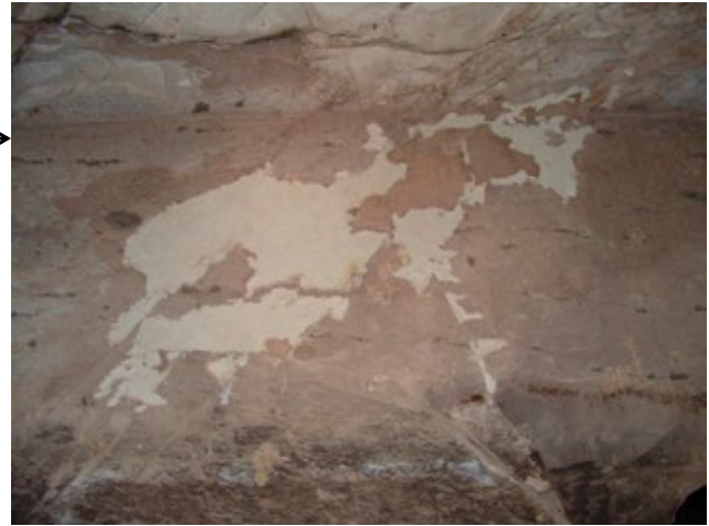
Chamber (E): Detail of surviving area of plaster. The light gray areas are repair plaster.
