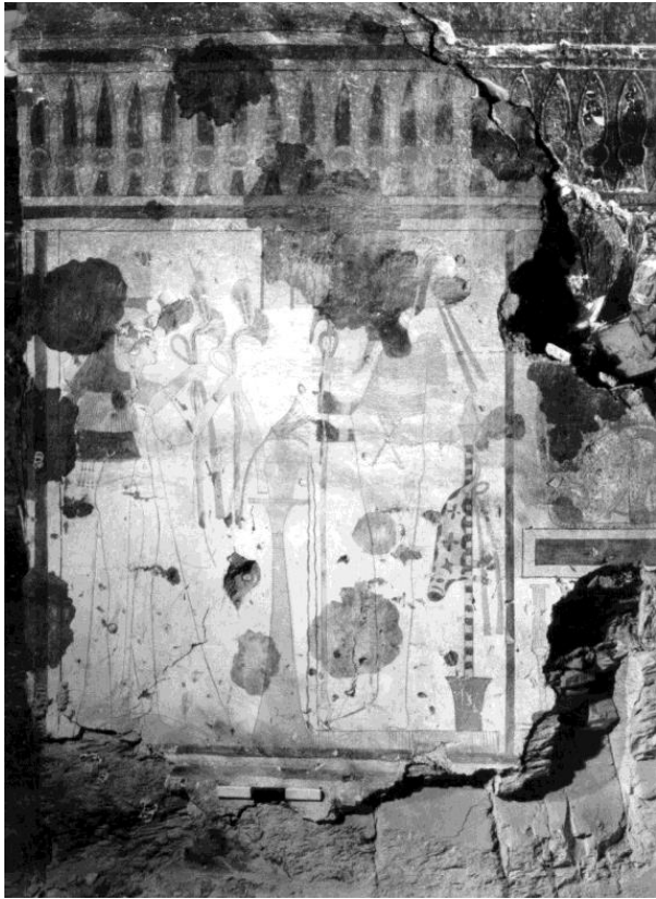
East side of north wall of burial chamber (E) that features depiction of the queen. Unlike most of the decoration in the tomb, this area is painted on a constructed masonry wall support. The painting differs in this area with no relief work and a slightly cruder painting style. Note large diagonal crack and losses of the painted plaster, already evident in the 1977 photo, left (Image: CEDAE).
