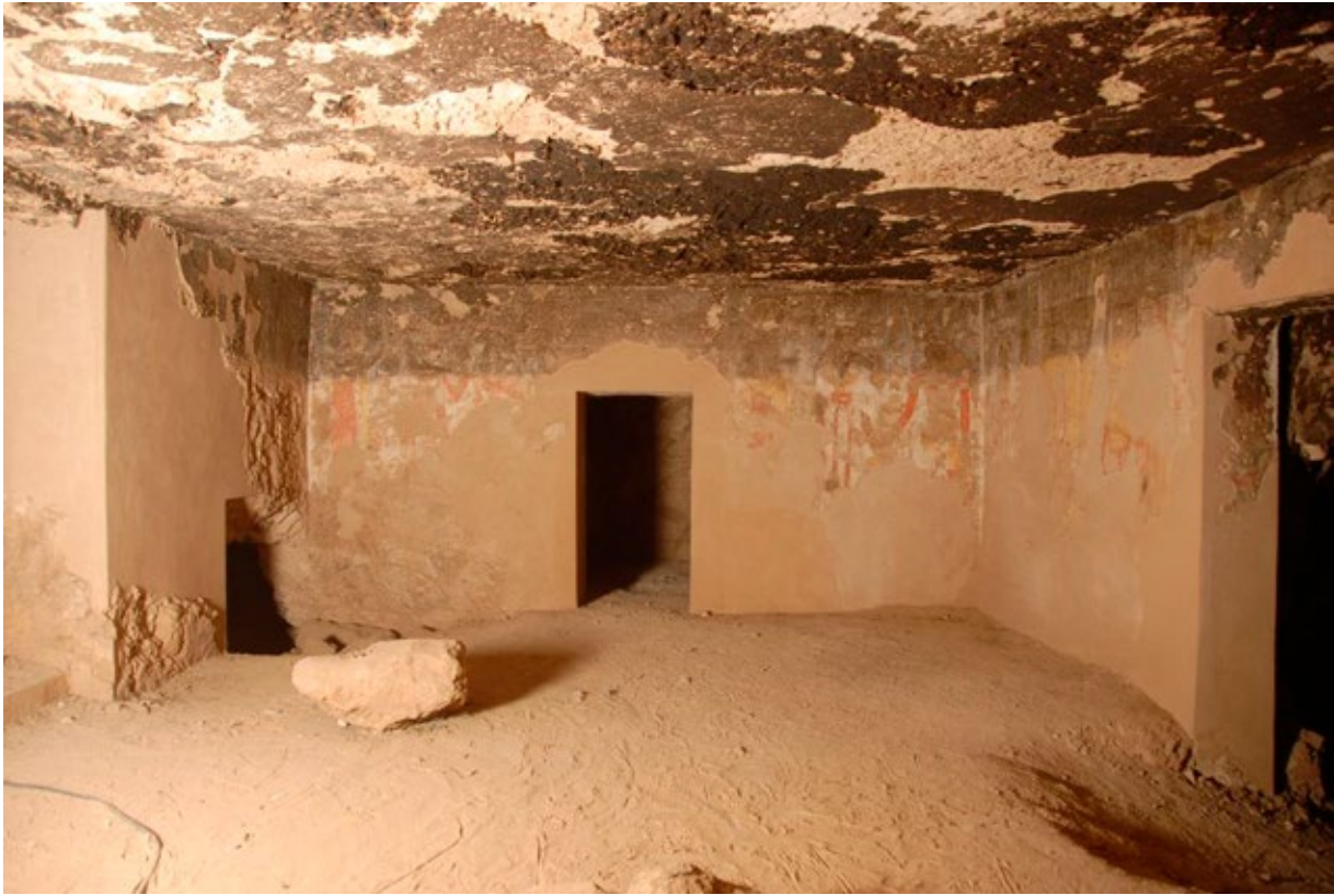
Chamber (C) looking east toward side chamber (G). Only the base of the easternmost pillar and fragments of painted plaster survive. Note blackening on ceiling and upper third of walls. The lower parts of walls were presumably protected from fire by debris. (CEDAE 2009)
