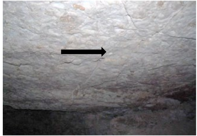
Ceiling fracture in chamber (B) near arrow.
