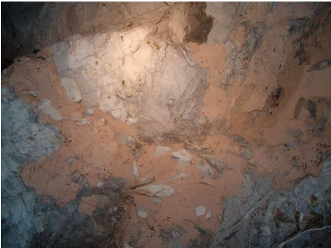
Packing out of walls and ceiling with plaster and rock shards was necessary in areas. Traces of this infill material still remains.
