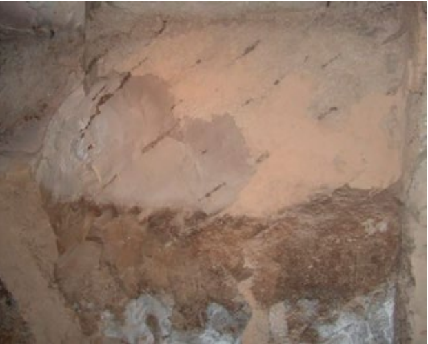
Chamber (K): White efflorescence can be seen on the rock in the flood zone at the base of the walls. Traces of painted original plaster survive above. It is pink in color possibly indicating heat-related damage.
