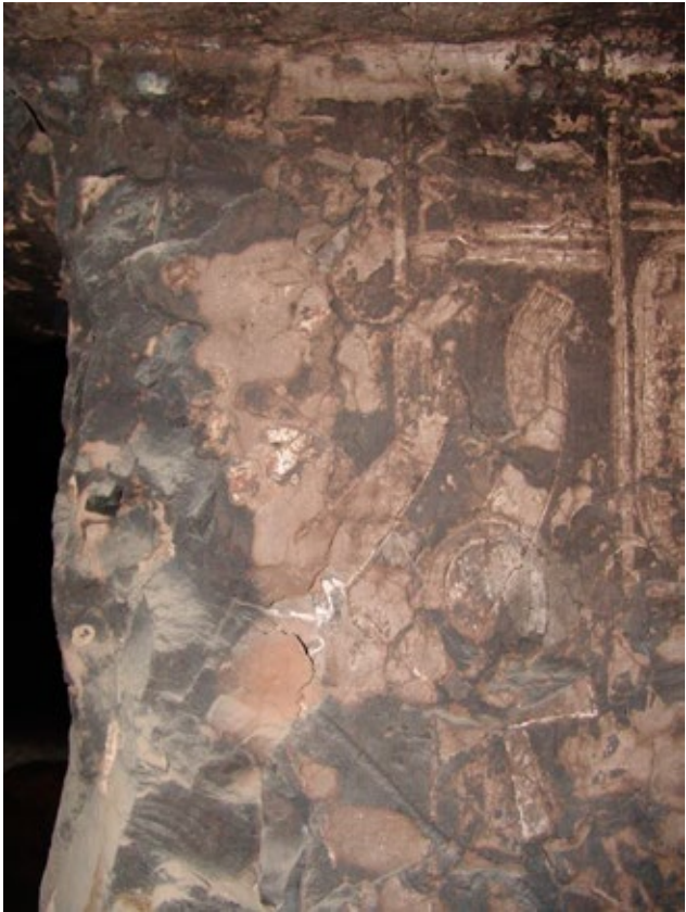
The fire in side chamber (G) caused loss of the upper plaster leaving behind a "negative effect" of the raised decoration. The figure now appears unblackened (as upper plaster layers were lost) while the background is still fire-blackened.
