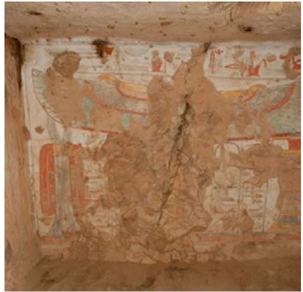
Bird nest on ledge of ceiling fracture and micro-fractured ceiling rock.
