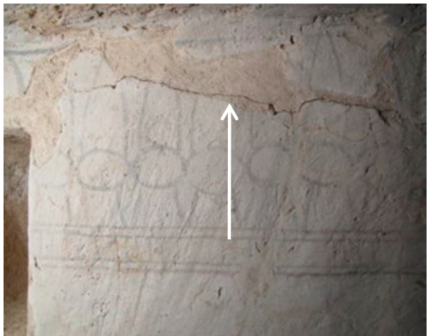
Crack has reopened where a previous plaster repair existed.
