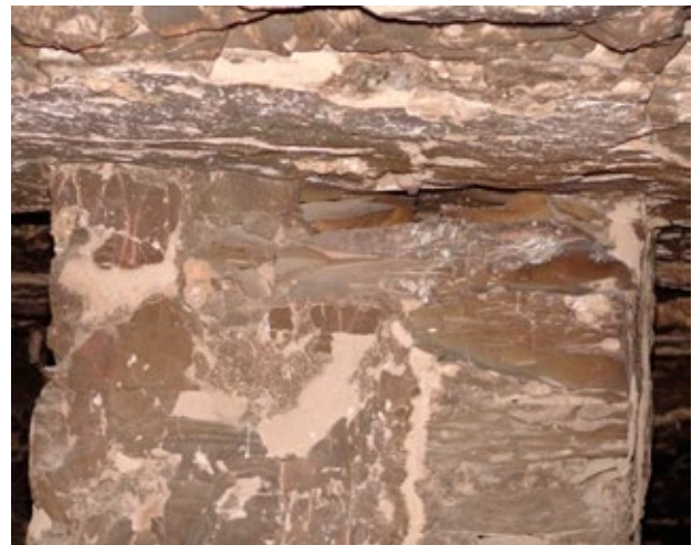
Detail of one of the masonry-constructed pillars in chamber (C).
