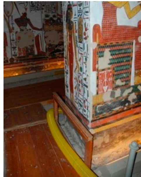
Narrow doorway (F) has no barrier to prevent visitors touching the walls.
