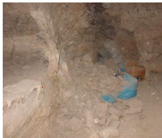
Shale deteriorating in main chamber, adjacent to entrance of side chamber.
