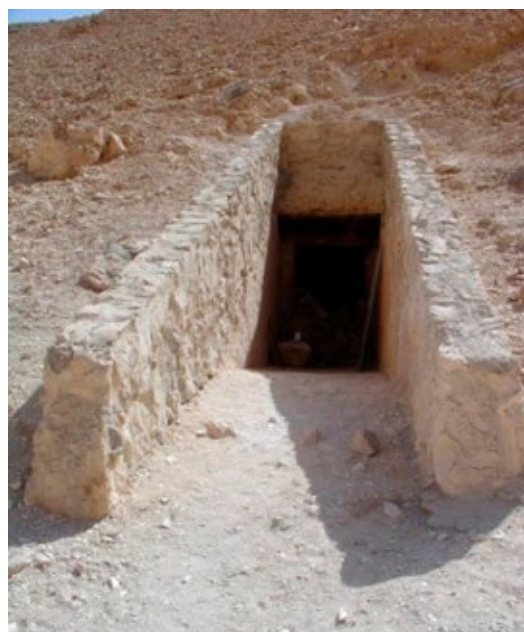
Entrance ramp (A) and entrance (B) in 2007. Modern masonry walls have been constructed along the ramp.
