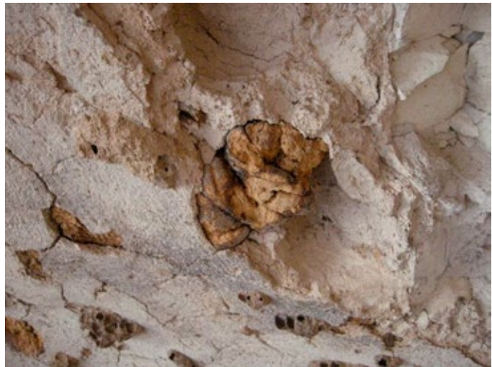
Detail of ceiling plaster in chamber C of tomb QV 31 showing the addition of animal dung.
