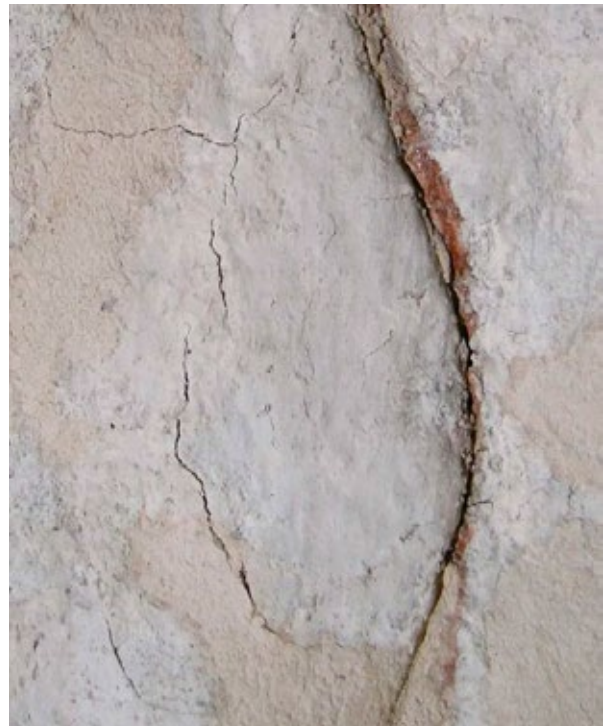
Minor cracks in both original and repair plasters are typically interpreted as evidence of ongoing deterioration. In most cases, cracks in the original plaster already existed, but photographs did not allow this to be properly assessed. These cracks do not represent a serious risk.
