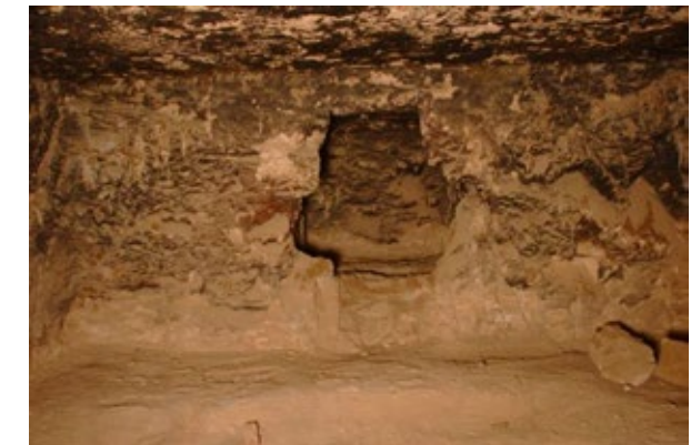
Lower part of the north wall of burial chamber (I) has area of rock loss around doorway (J) leading to niche (K) but otherwise appears stable. This area has not been previously treated.
