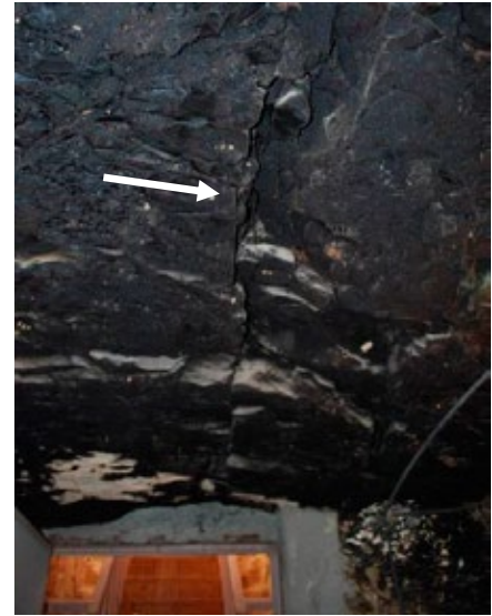
North-south fracture (arrow) in blackened ceiling of entrance chamber (B), with area of recent loss near door.
