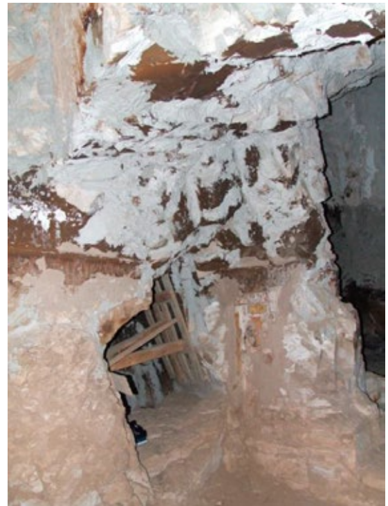
Shoring in niche (F) of east wall of Chamber (C) with plaster repairs of fractured and blackened rock of upper part of wall and ceiling above. In upper left part of wall, post-fire loss of ceiling rock is visible.
