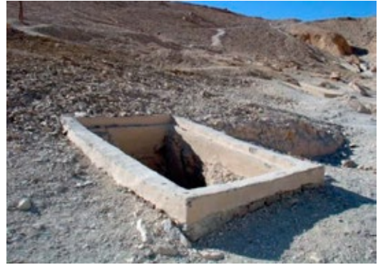
Shaft entrance with masonry surround.
