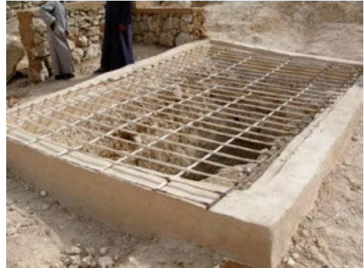
Masonry surround installed by the SCA as of December 2009
