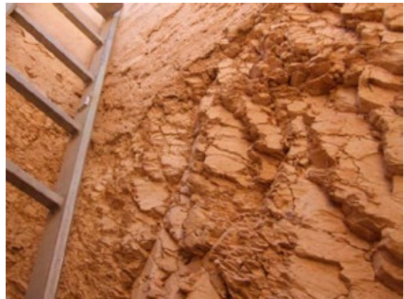
Heavily fractured rock in shaft.
