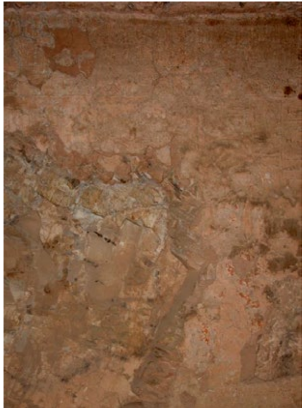
Same area in 2009. Little change in rock condition can be noted.
