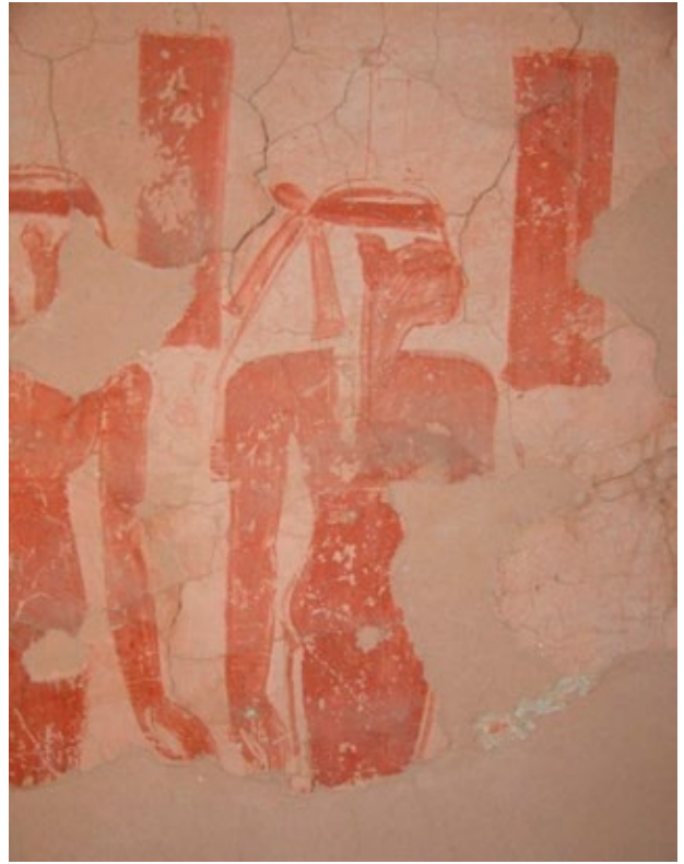
The paintings in chamber (K) are highly fractured and detached in areas.
