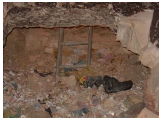
Debris and trash have accumulated at bottom of shaft.
