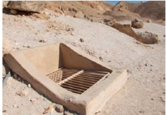
Shaft entrance with masonry surround.
