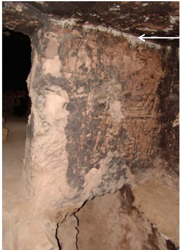
East wall of side chamber (E); note white crystalline material at tops of walls from bat urine.
