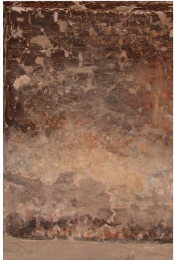
Chamber (C) in 2008 showing same area with 1989/1991 edging repairs.
