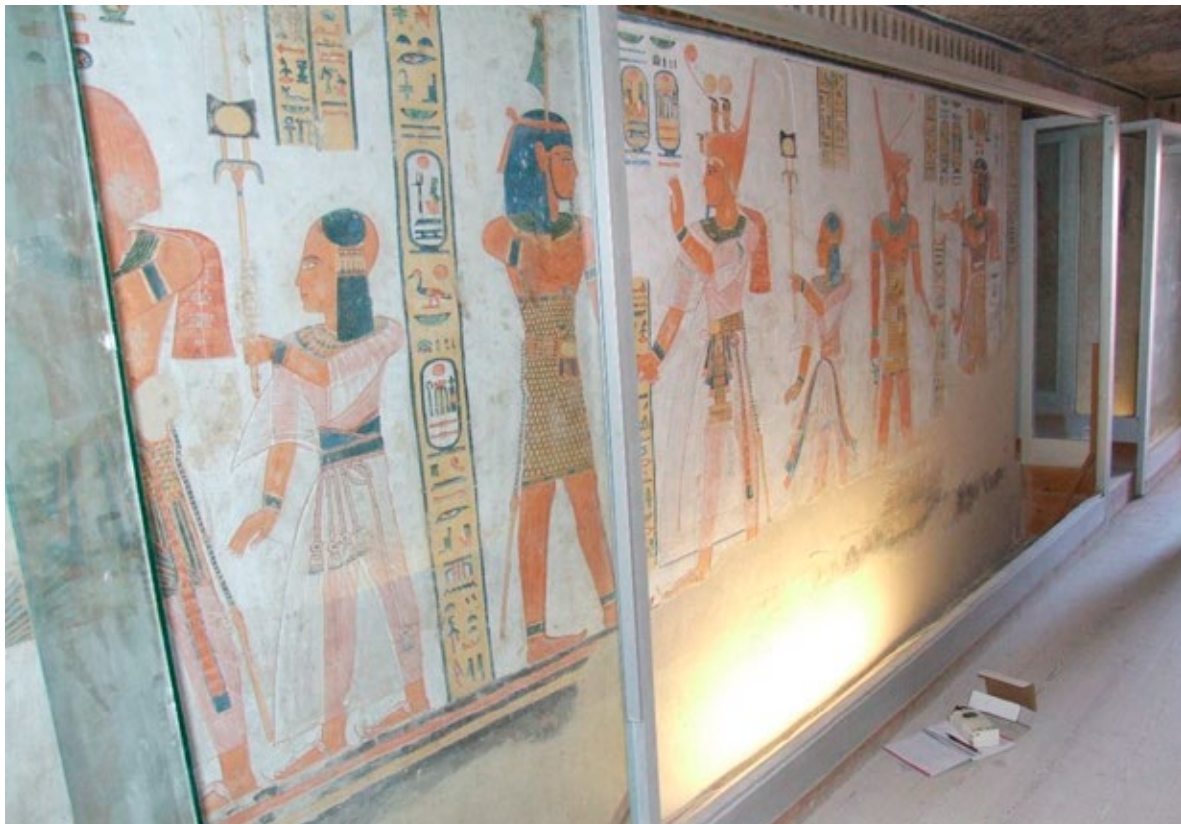
Panel of glass missing in first chamber corridor (C) (above and right), leaving the paintings unprotected.
