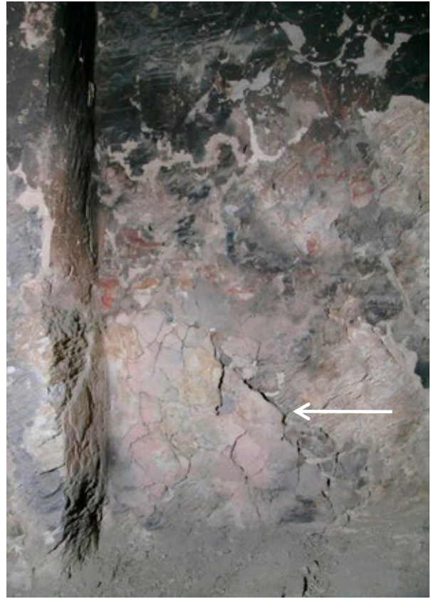
Fragile, cracked and detached areas of plaster on east side of ramp (E).
