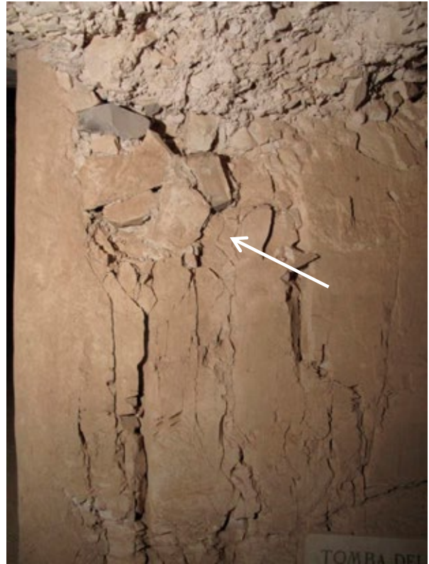
Above right: Image showing rock infill needed to rebuild door jamb of doorway (D) taken from chamber (E) looking north toward entrance (above left). Adjacent rock presents severe open vertical fractures.
