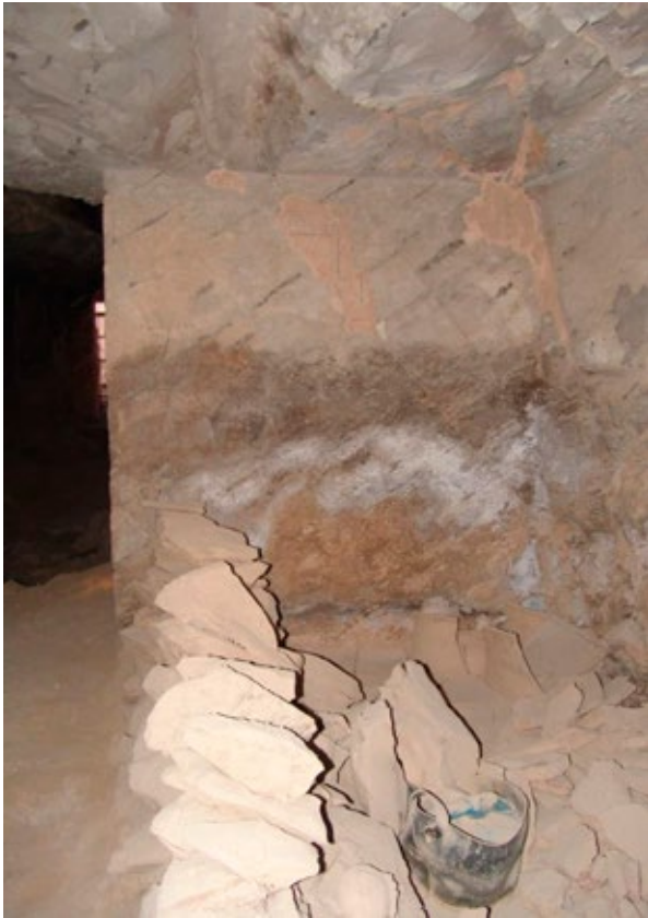
Chamber (K): White efflorescence can be seen on the rock in the flood zone at the base of the walls. Traces of painted original plaster survive above. It is pink in color possibly indicating heat-related damage.
