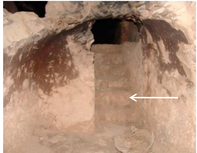
Lower chamber (N) of side chamber (E). The ceiling of the chamber, once vaulted, is now partially collapsed.
