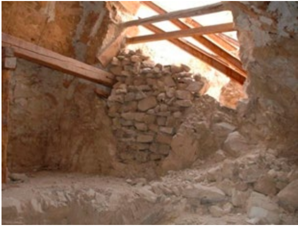
Side chamber with existing wooden and metal shoring and dry masonry wall between chambers to prevent access to the side chamber.
