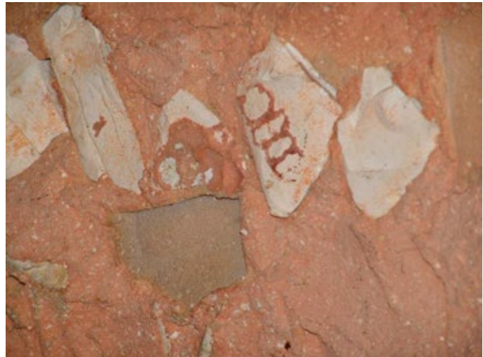
The ceiling of chamber E in tomb QV 51 was plastered and rock shards pushed into the plaster to minimize shrinkage.
