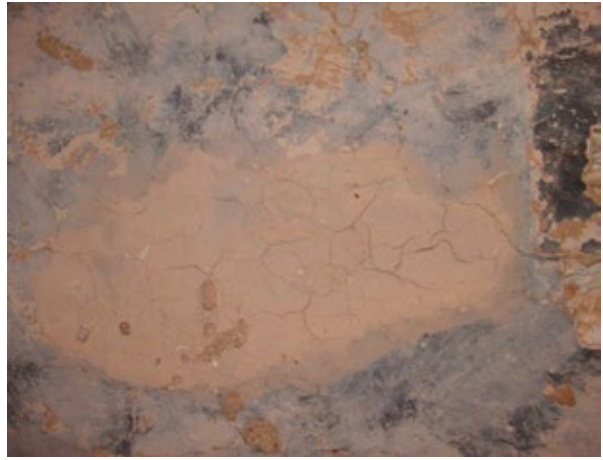
Area of repair on ceiling of chamber (C) is possibly an early repair from antiquity.
