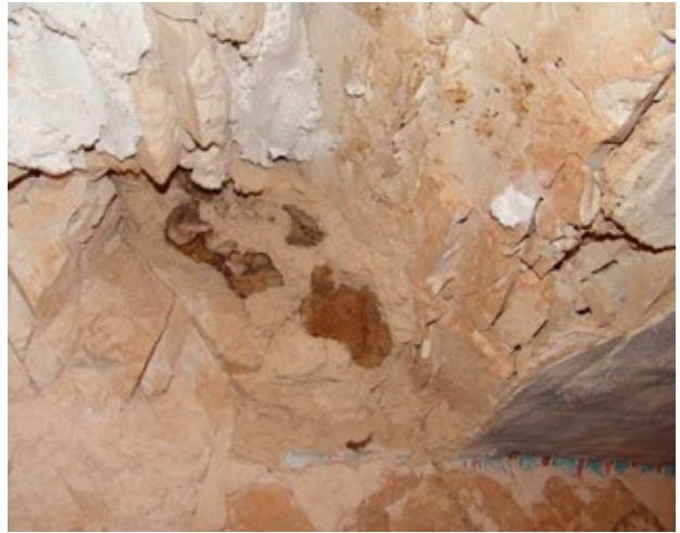
Detail of ceiling of chamber (C) showing traces of infill plaster that might indicate that the ceiling in this area was either never flat or that large amounts of infill material previously filled this space. It also indicates that some of the rock collapse had occurred in antiquity before the tomb was decorated.
