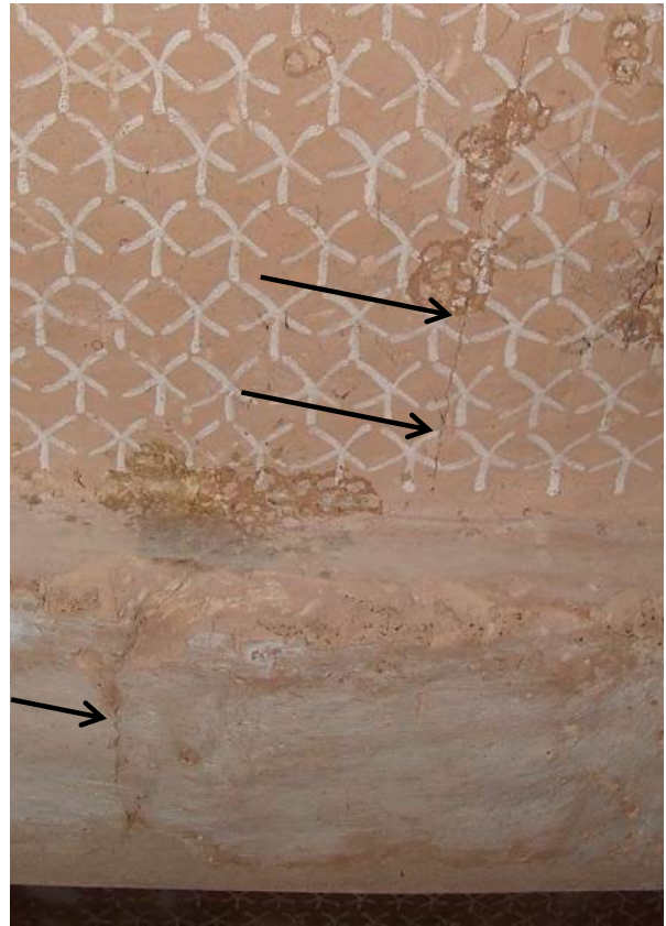
The small crack observed in lintel of doorway (D) should be monitored.
