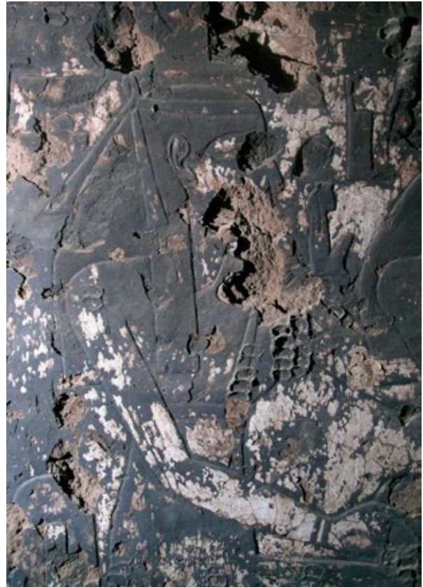
Decoration on north wall of chamber (C) suffered severe fire damage, which has led to both heavy blackening of the surface and complete loss of the paint layer; remains of insect nests also apparent.
