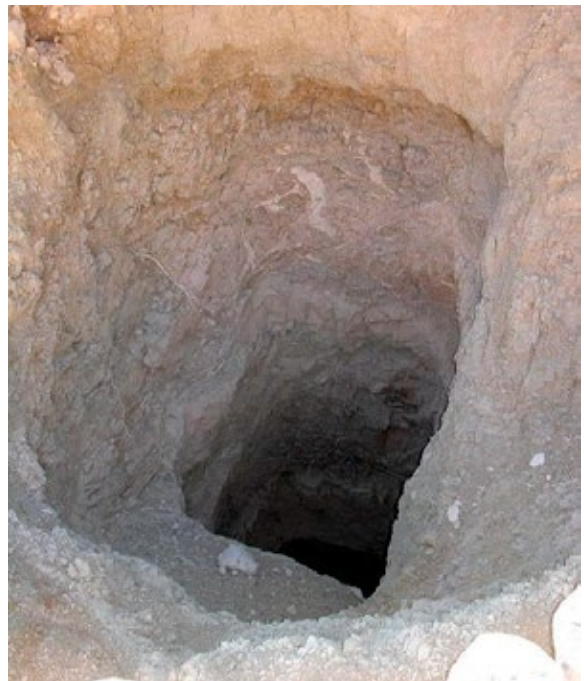
The shaft from above. Note friable shale throughout length of shaft.
