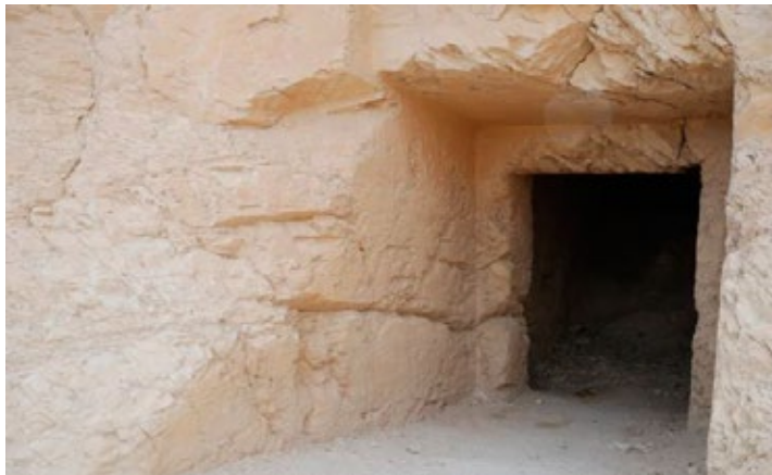
Horizontal crack on south wall in ramp continues to the corridor wall through south door jamb. Areas of loss occur along the crack.
