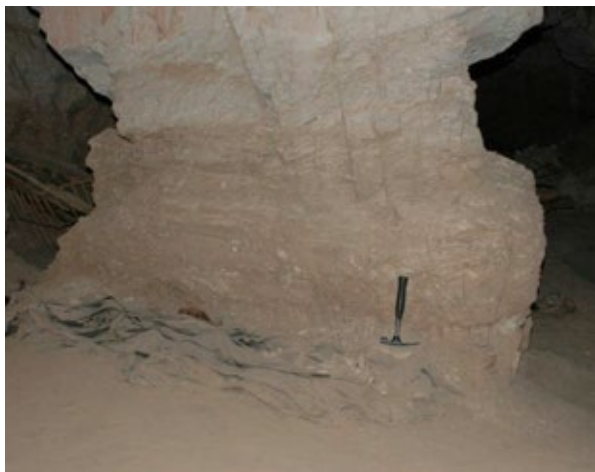
Lower part of wall shows weakening and deterioration by retained moisture in the clay-rich marl.
