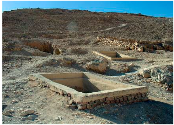
Shaft entrance with masonry surround.
