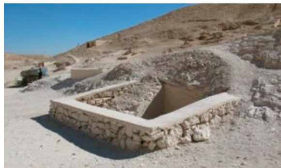
Entrance to QV 50 before (above) and after (below) rebuilding of masonry surround with cement capping.
