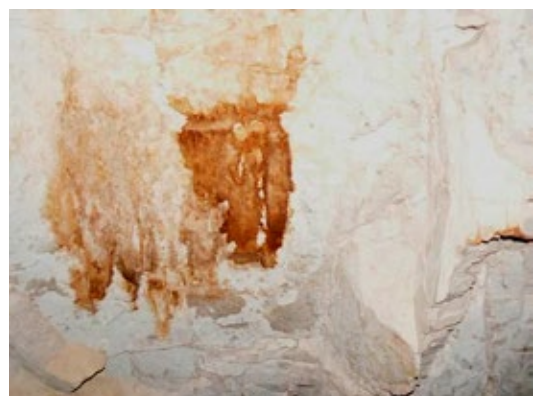
Brown staining on rear wall, perhaps due to bats.
