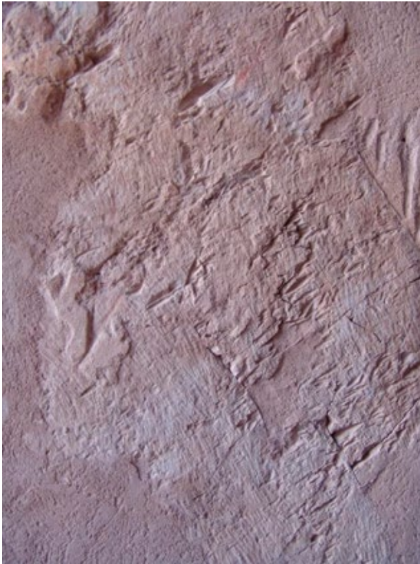
Good quality rock support, with little fracturing, in entrance corridor (C) that enabled fine chiseling and a flat wall surface. Only a thin skim of plaster was needed to prepare the surface for painting.
