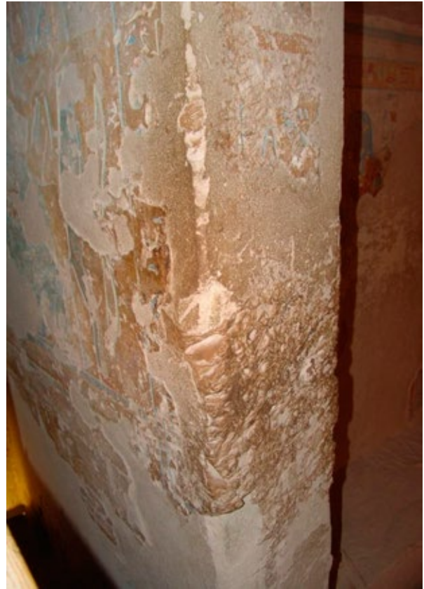
The jambs of doorway (H) show the result of visitors touching the painting. This area should be protected.
