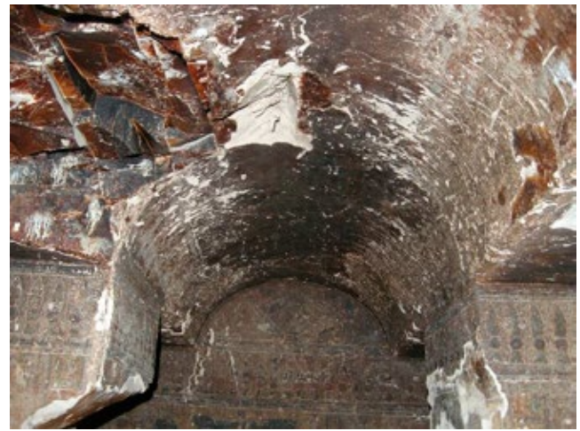
Post-fire loss of ceiling rock in barrel arch that appears more recent.
