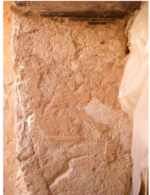
Area of decoration survives on the exterior and jamb of doorway (B).
