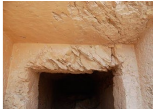
A fracture continues through the ceiling of the ramp to lintel at doorway.
