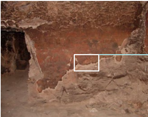
Comprehensive campaign of edging repairs was carried out throughout the tomb in 1991 to secure areas of surviving painted plaster.
