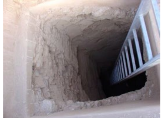
Deep shaft, as seen from above.
