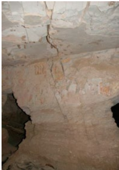
Basal erosion and fracturing of the two remaining piers within tomb. Basal rock is fragile and is incapable of supporting upper portion of rock.
