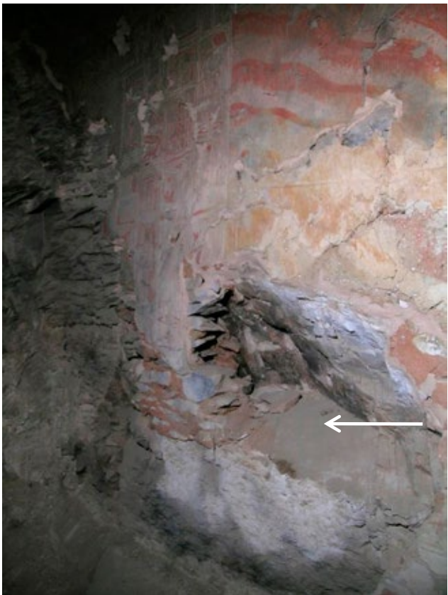
Substantial packing was necessary to fill large voids in the walls. A large amount of this infill material has been lost in chamber (G).
