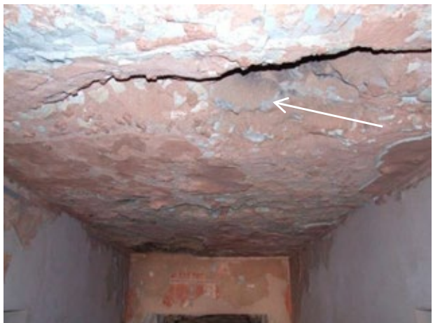
The rock quality worsens toward the rear of the tomb. The large area of rock loss on the ceiling of chamber (E) is historic (from the time of the tomb construction) and shows evidence of rock and plaster infill still remaining.
