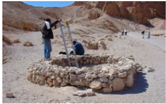
Low rubble wall surrounds shaft entrance during initial assessment (2007).
