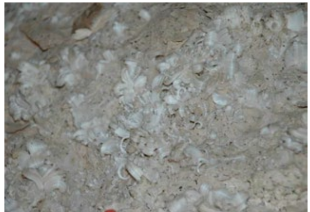
Substantial salt efflorescence and large crystal growth on east wall in chamber (G).
