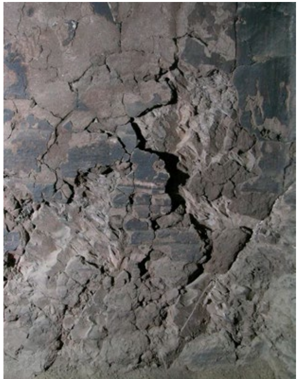
Some areas of decorated plaster are cracked and detached.
