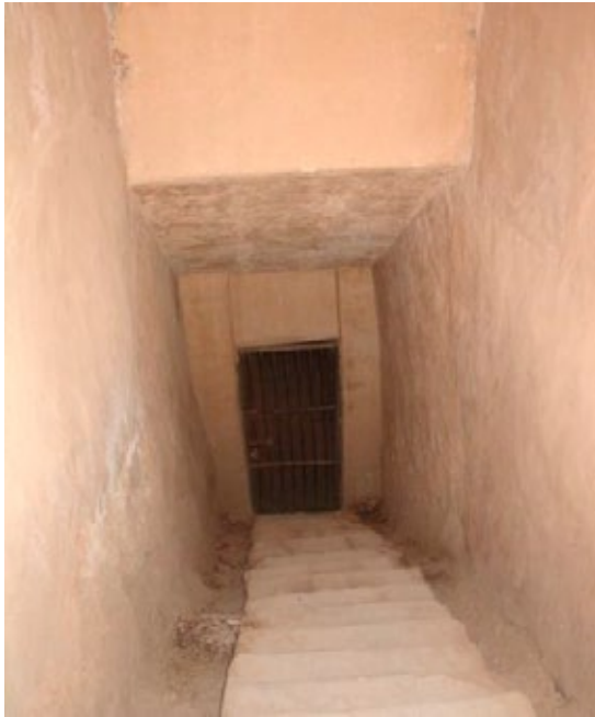
Reconstructed entrance and stepped ramp (A).
