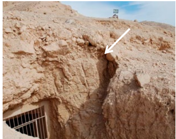
Detail of east wall of ramp (A): a large area of rock loss where boulders in the overlaying debris have been undercut by water erosion is now at risk of falling.
