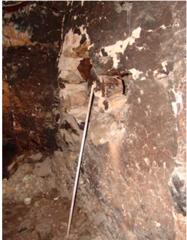
Constructed masonry wall of niche (O) (see also image below).
