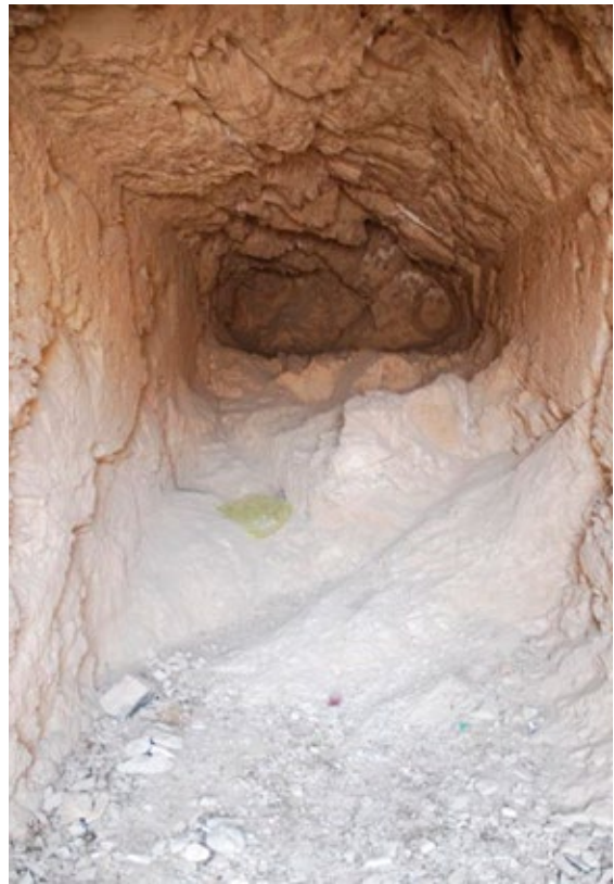
Previous ceiling loss is documented in TMP (1981) and CNRS (1988) mapping.
