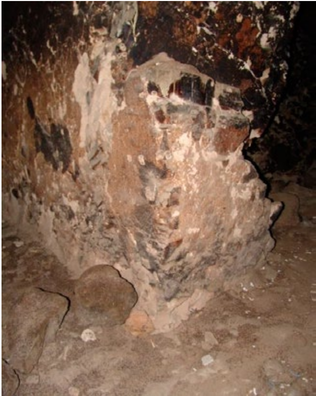
Areas of the tomb such as this doorway were constructed out of masonry and then plastered.
