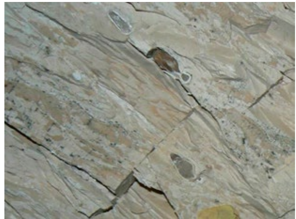
Chert nodules in marl of chamber wall.
