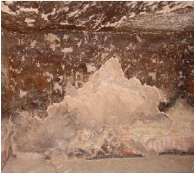
Large post-fire loss on east wall of chamber (C). Some stabilization of rock is necessary in this area.
