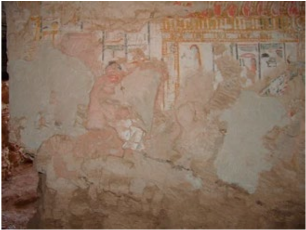
Plaster repairs on south wall of chamber (C).
