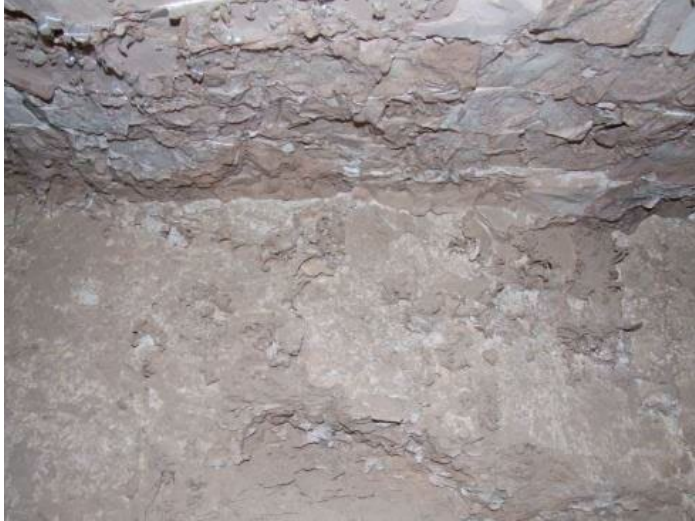
Fibrous halite salt growth in area of ceiling and wall.
