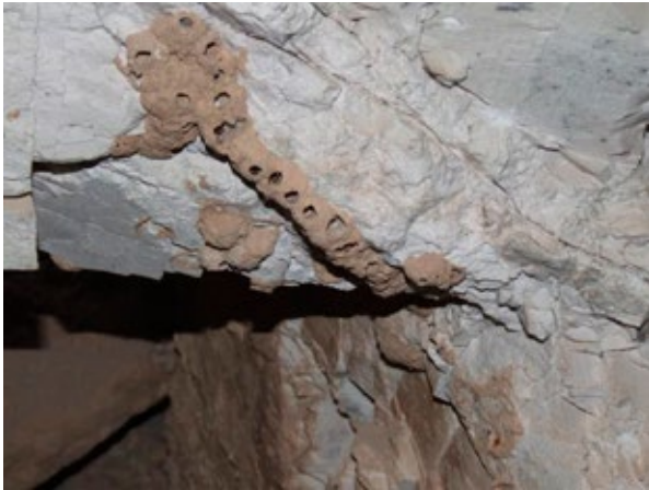
Wasp nest adhered to wall near entrance.
