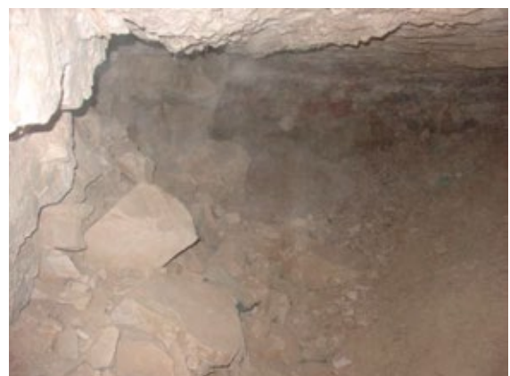
View of main chamber (B) with rock collapse on left.
