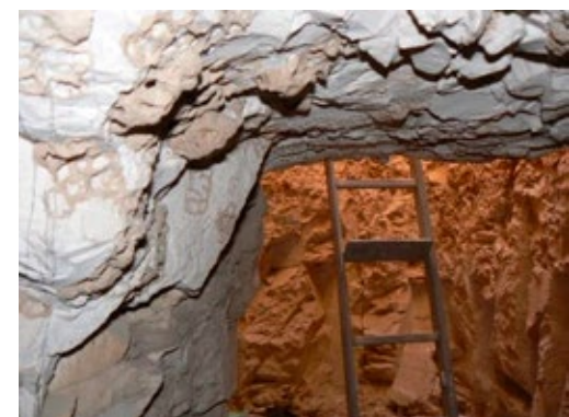
Shaft with ladder and remnants of wasps nests in foreground.
