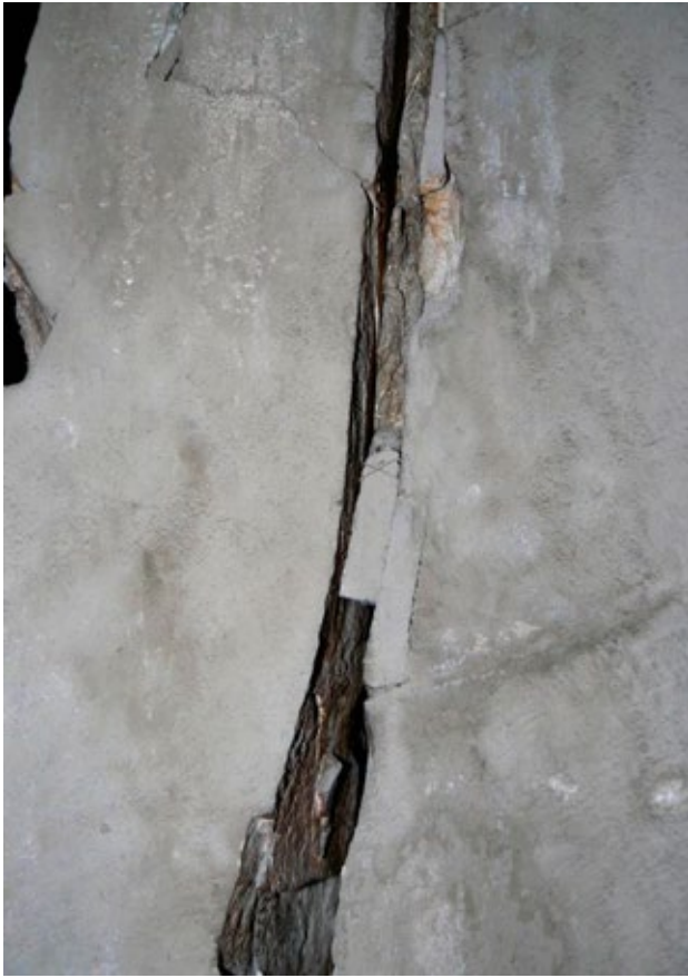
An early attempt in modern times at rock stabilization of pillar using gauze and adhesives.
