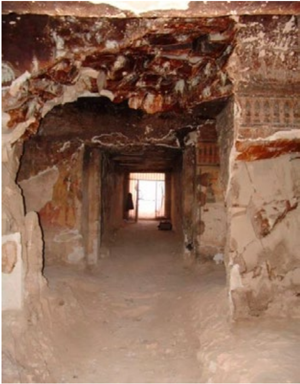
Interior view, looking towards entrance showing pre-fire loss of rock in pillar I (right) and in ceiling between the pillars.
