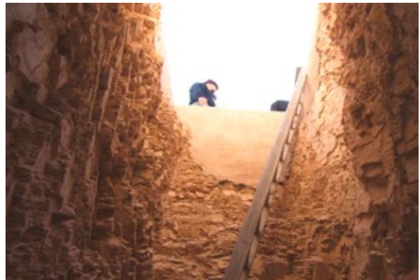
Fractured rock in shaft.
