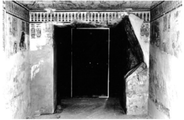
Early plaster repairs are already visible in 1980 photographs. However, not all areas have been treated. Doorway shows large loss that was later filled. (Image: CEDAE)
