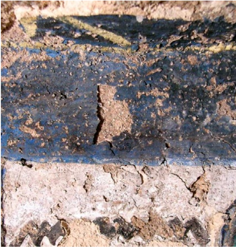
Detail of severe salt-related deterioration on the south wall of chamber (O). Although in a fragile condition, monitoring of such areas has indicated little or no change since 1997.
