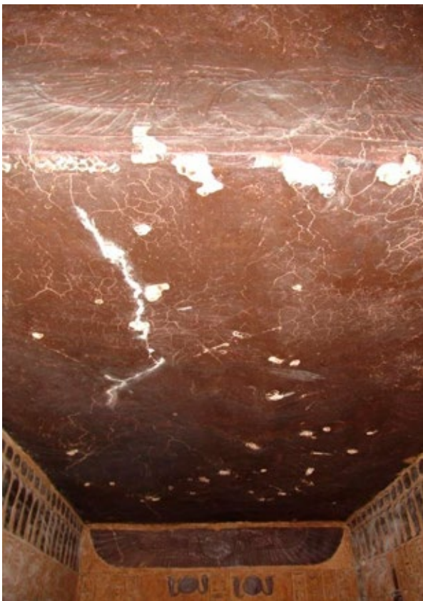
Note extensive cracking on ceiling of rear chamber (I) though very little loss has occurred.
