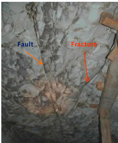
Shored ceiling area in antechamber (C) with fault to the left and fracture to the right.
