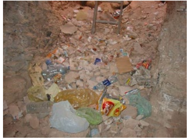
Accumulation of trash at bottom of shaft.
