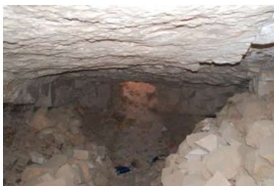
Rock piles associated with collapse of interior walls.
