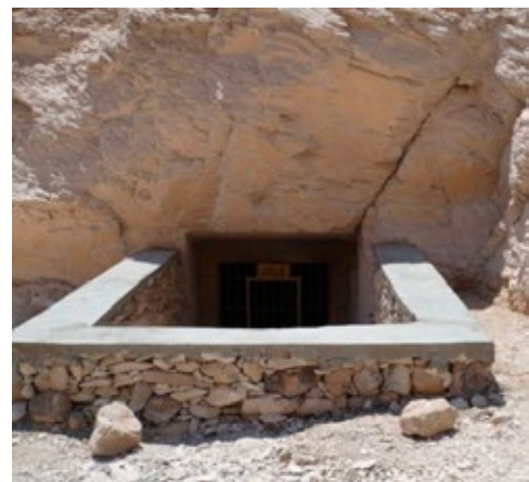
View of entrance surrounded by cement capped dry masonry wall.
