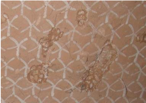
Insect nests on ceiling have been removed.
