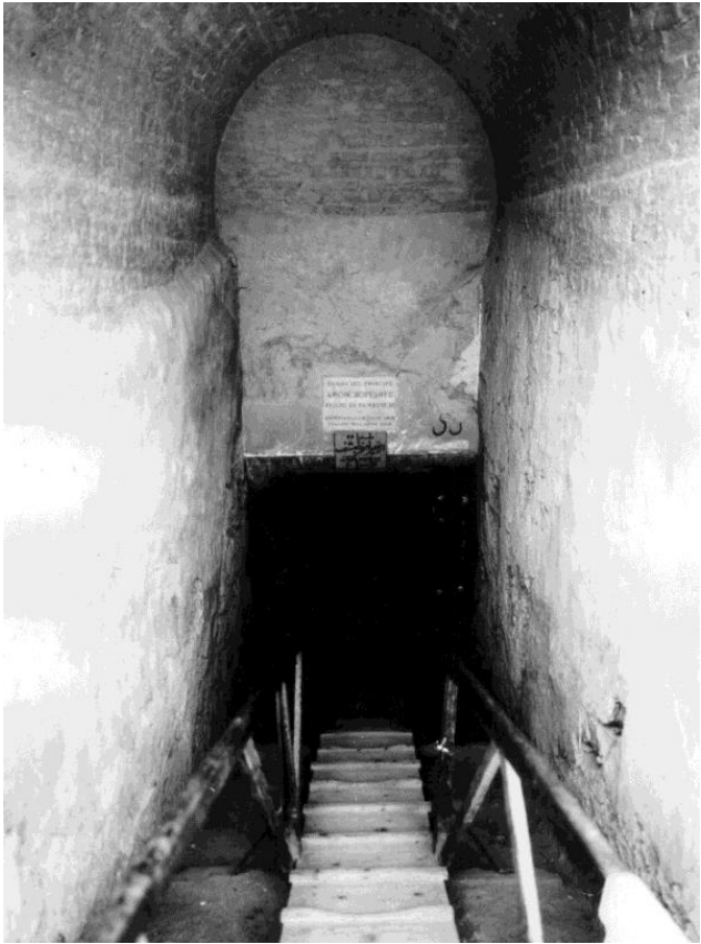
Wooden steps with handrail were installed at ramp (A) [to protect the original surface. They were later replaced with masonry steps (Image: CEDAE 1974).
