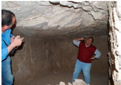
Area of substantial ceiling collapse in chamber (C).
