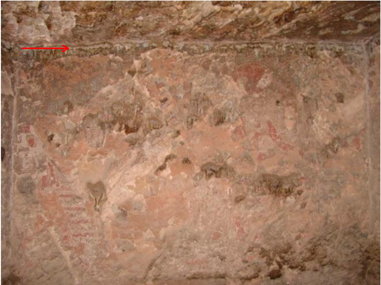
Fragmentary survival of painting in chamber (E). Though the lower plaster survives, the upper painted layer has suffered much loss. Bats also appear to roost on the edges of surviving plaster on this wall leaving staining and a line of white crystalline material at the tops of walls (indicated by red arrow).
