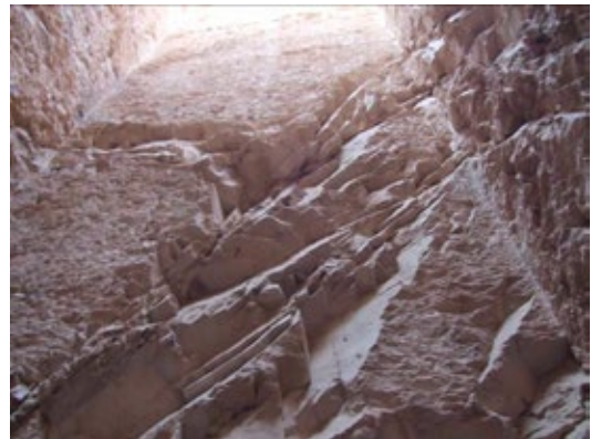
View of shaft from below, with visible fractures.
