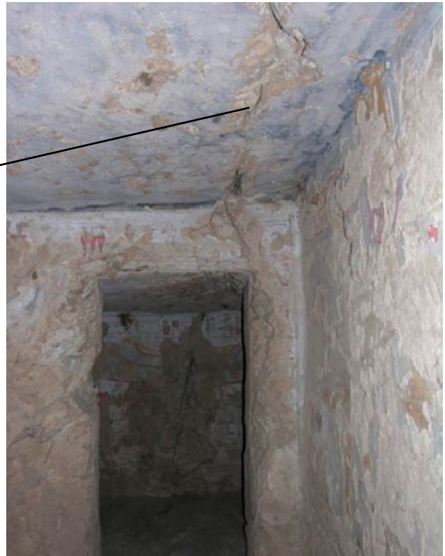
Open vertical ceiling fracture running laterally across the tomb and continuing into the east wall of chamber (G). Presence of original mortar packing in the fracture indicates little movement has occurred since the tomb was excavated in antiquity.
