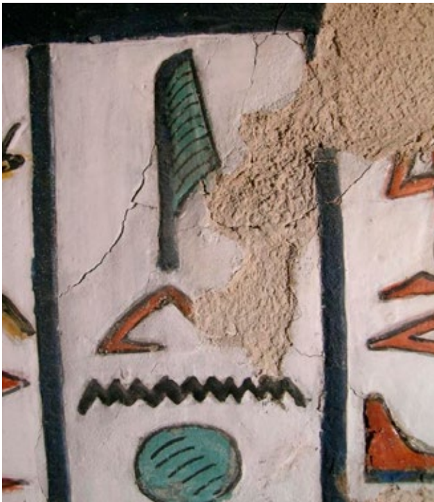
Minor cracks in both original and repair plasters are typically interpreted as evidence of ongoing deterioration. In most cases, cracks in the original plaster already existed, but photographs did not allow this to be properly assessed. These cracks do not represent a serious risk.
