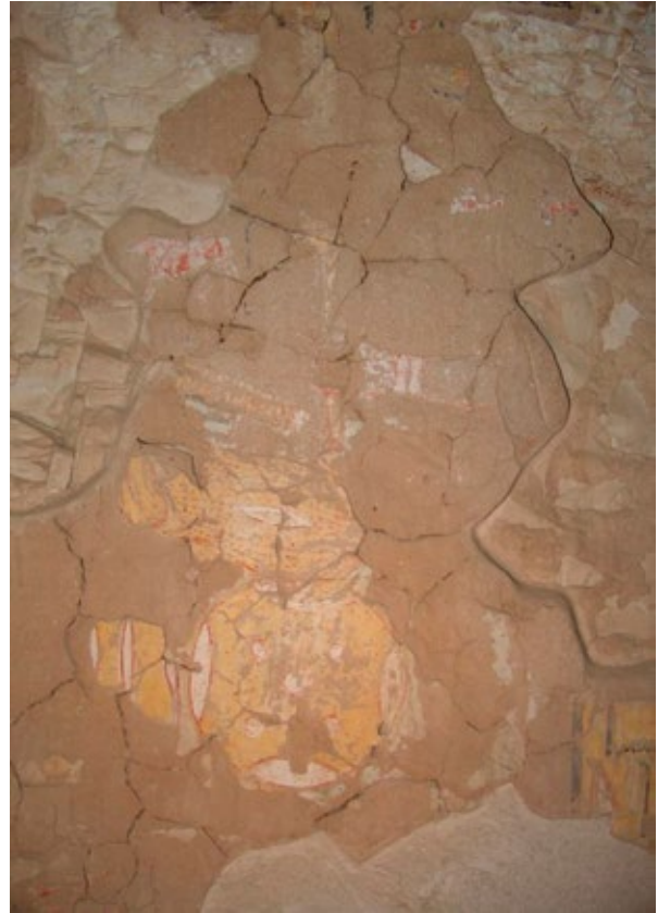
The treatment in side chamber (E) consists of edging repairs used to stabilize surviving areas of plaster. The repairs are quite minimal allowing areas of the rock to be left exposed and leaving the cracks of the plaster untreated.
