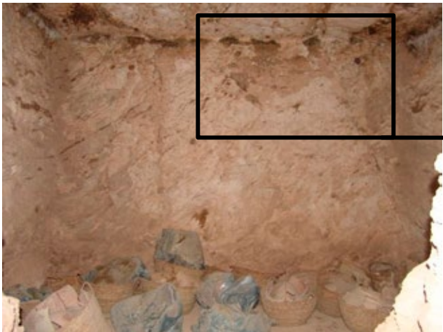
Right upper side chamber (M): small fragments of painted plaster appear heat damaged; paint layer looks to have been carbonized. In some areas the upper plaster layer has been lost which could be due to the fire damage.
