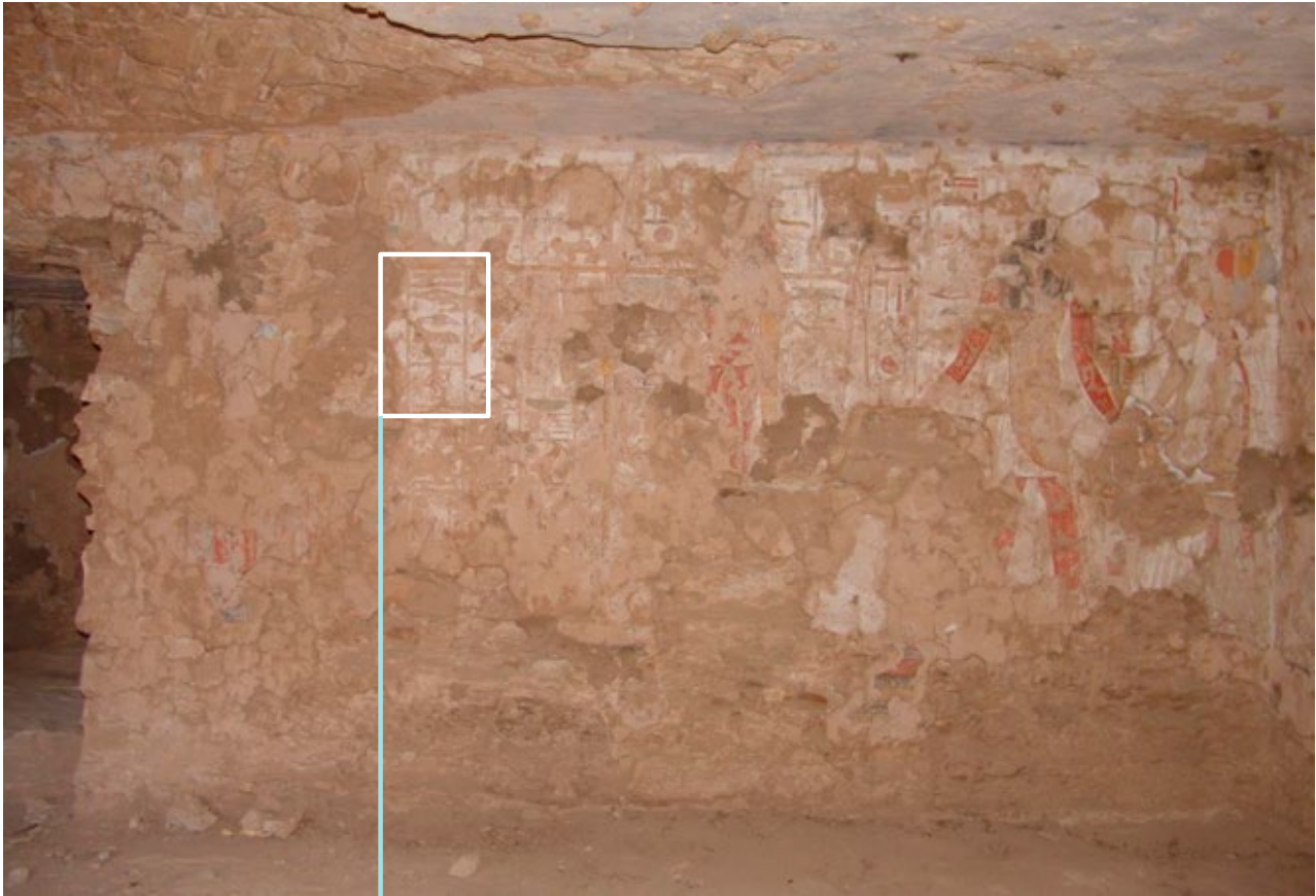
North wall of pillared chamber (C). Note fragmentary survival of painted plaster in this area.
