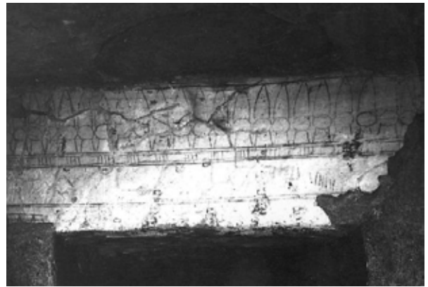
1988-89 CEDAE photograph shows crack already present.
