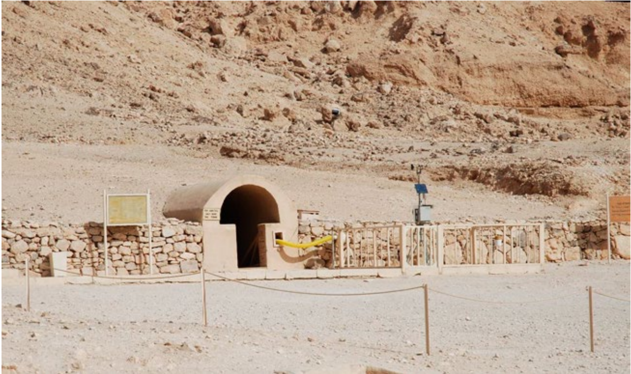
Entrance with overburden above the tomb, sloping upward. An environmental station was installed in the gated area to the right of the entrance.
