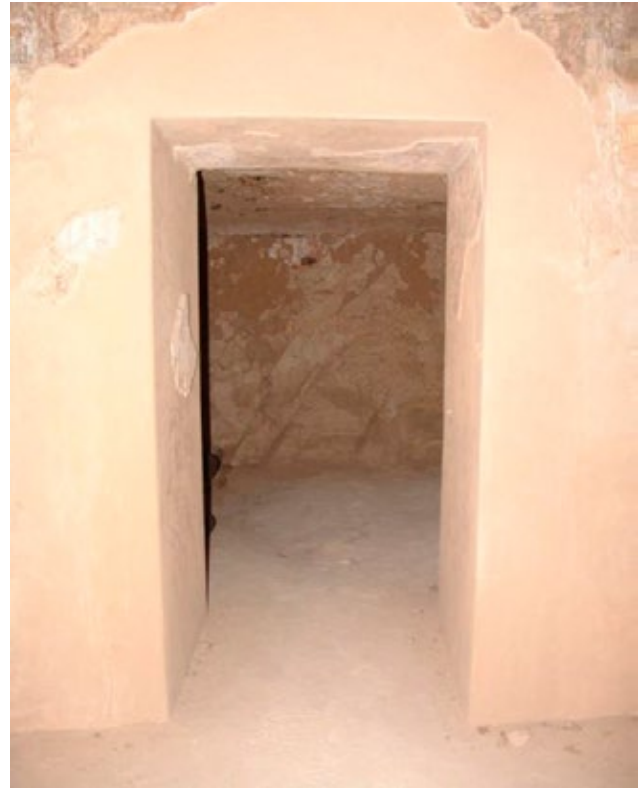
Doorway to side chamber (E) was reconstructed with a substantial amount of repair plaster. The extent of loss in this area suggests that the rock suffered extensive damage possibly caused by flooding.
