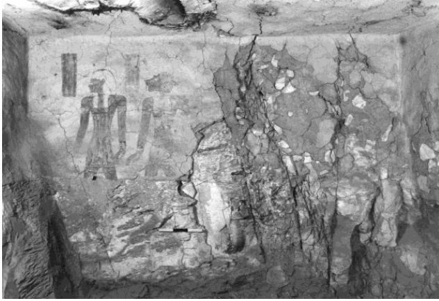
The walls and floor of side chamber (I) were never fully excavated during the tomb construction. The paintings appear unfinished. The image above left shows the area before treatment in 1986 (Image: CEDAE). Image above right shows the area after plaster repairs.
