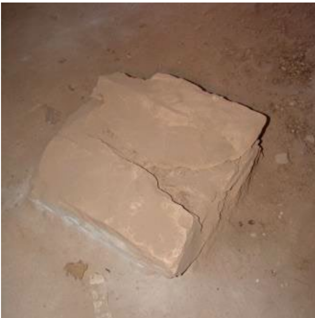
Pillar base (above left) and painted square on ceiling in chamber (C) directly above it (above right), indicating that the pillar was constructed at a later date (after the ceiling was already plastered and painted) and is now largely lost.
