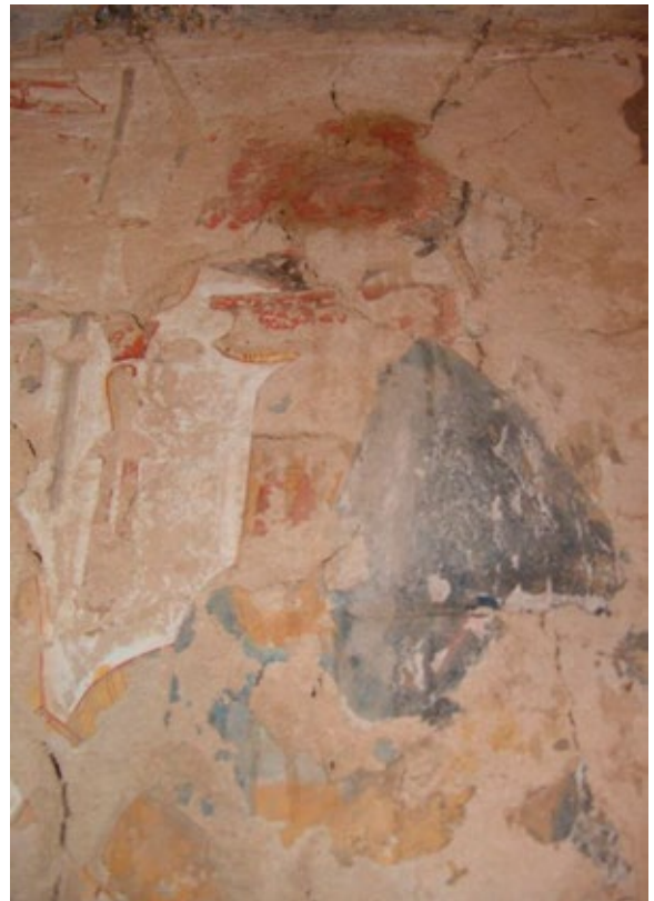
Drips from previous treatment are visible on the painting in chamber (C), north wall, east side.
