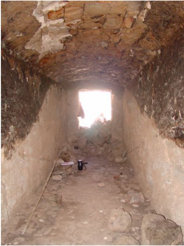
Corridor C: Fire damage rose upwards toward doorway (B), left. Looking from doorway (B) toward doorway (E), right. The lower part of walls of corridor (C) were protected from fire by debris.
