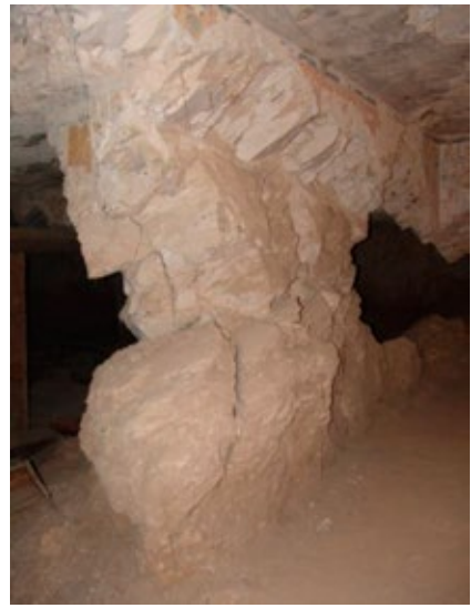
Basal erosion and fracturing of the two remaining piers within tomb. Basal rock is fragile and is incapable of supporting upper portion of rock.
