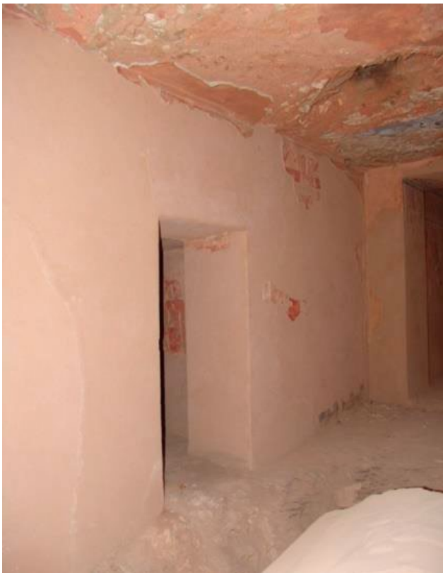
Walls in chamber (E) are largely reconstructed with plaster. Little painted plaster survives.
