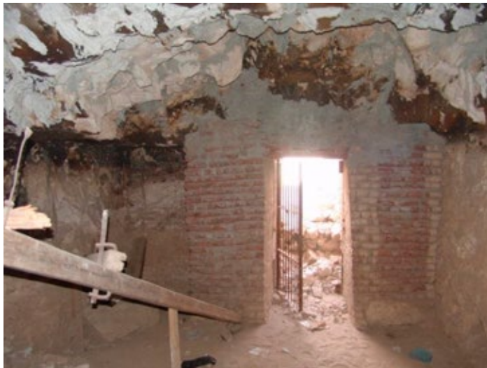
Reconstructed entryway (B) and extensive plastering on ceiling to prevent rock loss in chamber (C)
