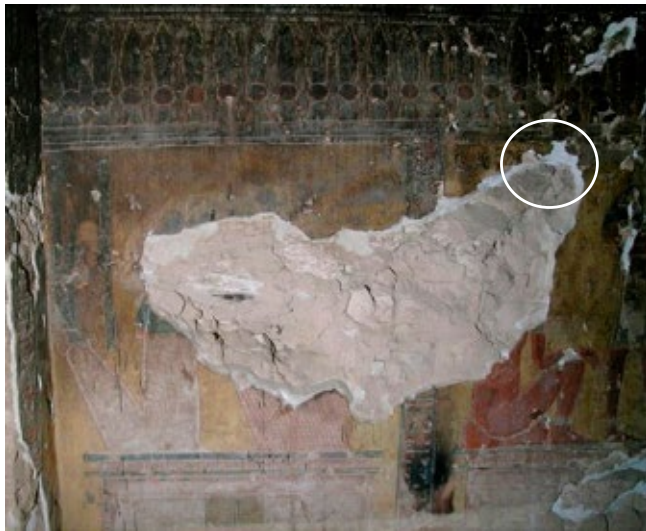
Losses of area of painted plaster since 1977 photograph (right, Image: CEDAE) in burial chamber on north wall, west side.
