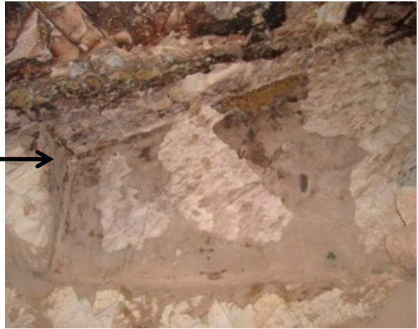
Surviving area of decoration in corridor (E).
