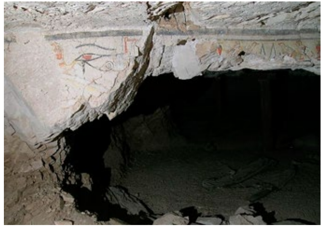
At risk area around doorway (K) between chambers (L) and (I). Loss of walls has resulted in large unsupported spans of rock throughout the tomb and localized loss of hanging rock.
