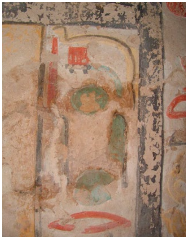
Area of green paint in chamber (G) looks as though it has been consolidated with an adhesive resulting in darkening of the surface.
