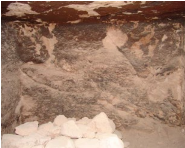
Side chamber (G) has heavy soot blackening and post fire losses.
