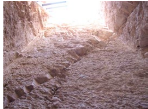
Shaft from below, with visible open fracture.
