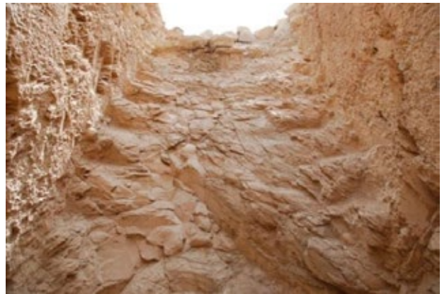
Heavily eroded steps of QV 56.
