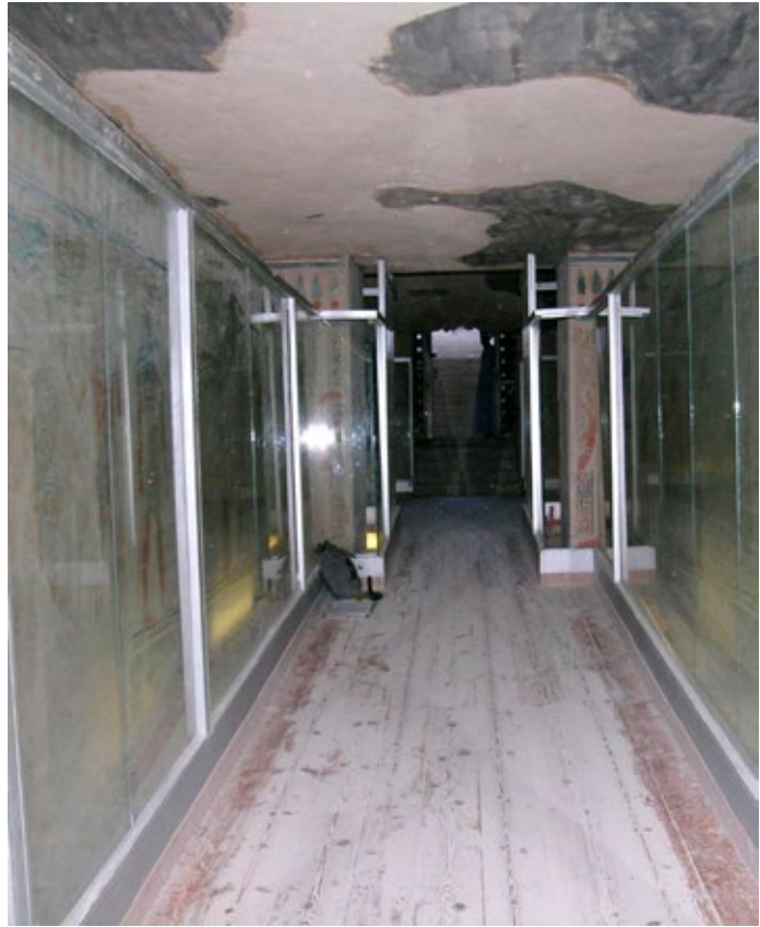
The ceiling losses have been filled with a modern repair plaster.
