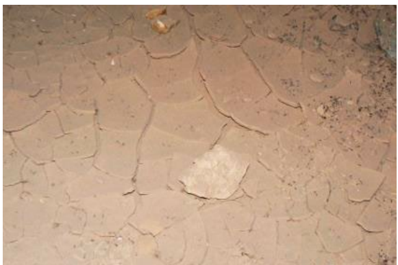
Dried mud layer on floor in chamber (C).
