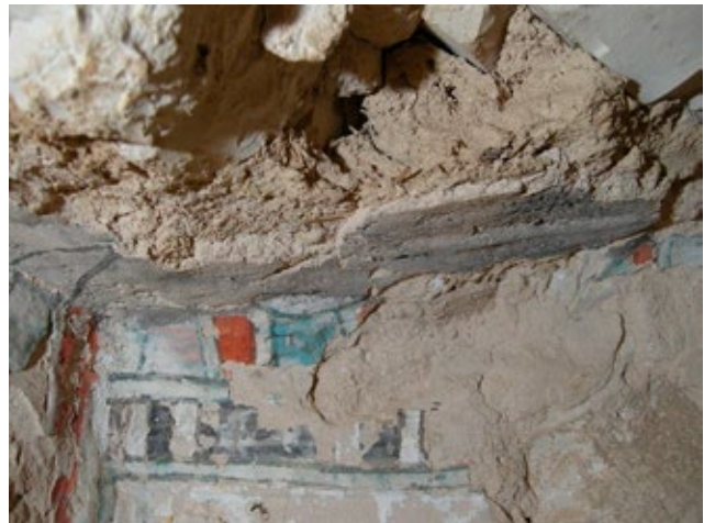
Example of hiba plaster used on the ceiling of chamber C of tomb QV 36. The lower plaster is an earthen plaster with a high fiber content.
