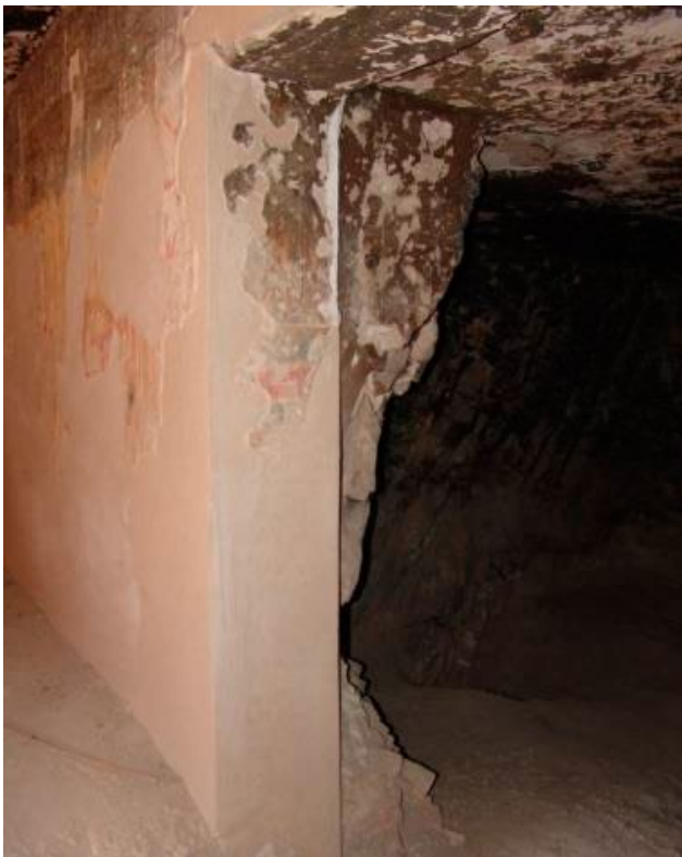
Area of rock loss at lower part of doorway (H) and partial reconstruction.
