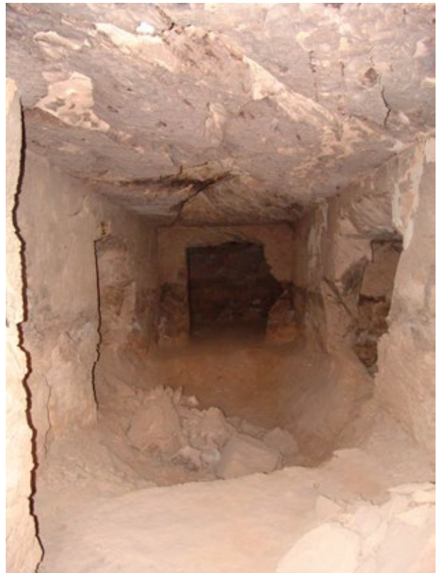
Overview of the tomb interior in corridor (E) with heavily fractured ceiling and local rock loss; water staining visible along wall.
