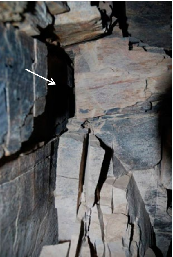
Detail of wide detachment of surface rock layer in rear wall of chamber (E). Areas of surface rock layers threaten to fall.
