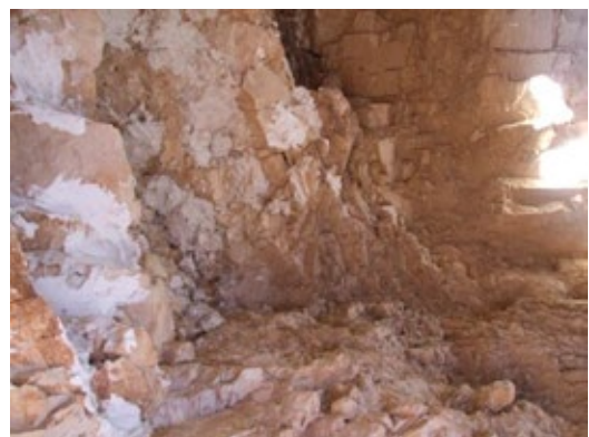
Detail of shale and white cement patches on walls.
