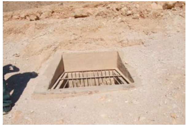
Shaft entrance with masonry surround and metal grill.
