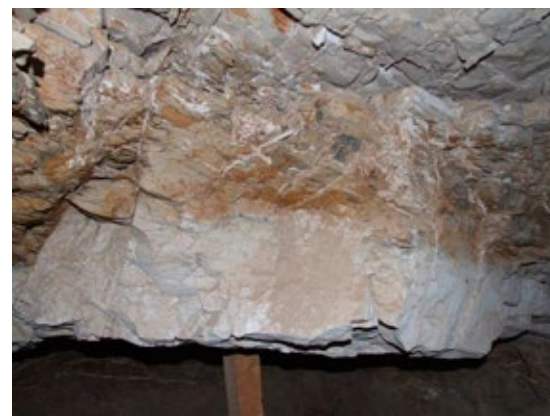
Rock overhang in south with shoring below.
