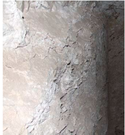
Salt efflorescence and related deterioration in main chamber.
