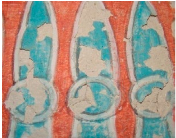
Detail of the flaking paint.
