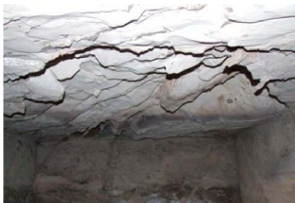
Fractured ceiling rock in side chamber (I).
