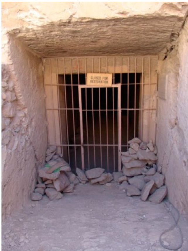
View of entrance (B) in 2006 with Schiaparelli plaque on right and "Closed for Restoration" sign above door.
