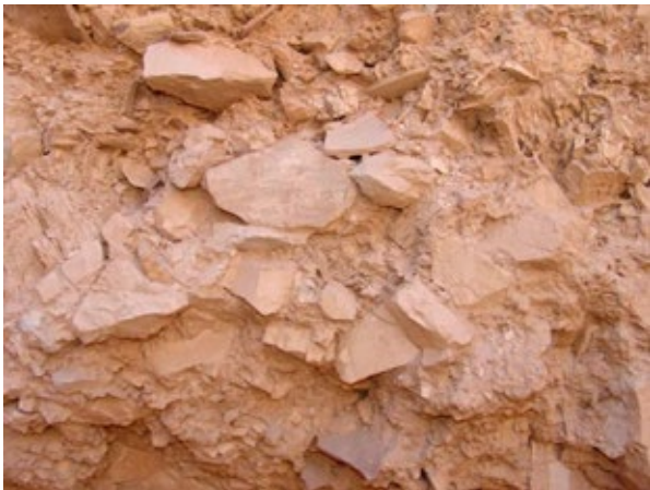
Substantial infill material used to pack out walls. Note large amount of rock and pottery shards mixed with plaster.
