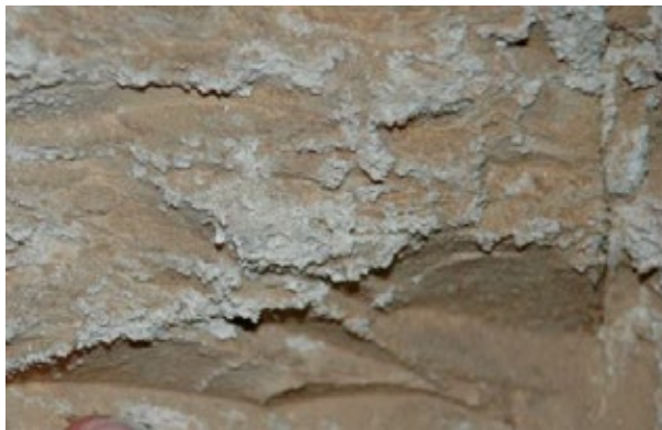
Detail of surface salt efflorescence.
