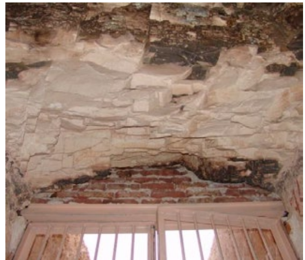
A large post-fire rock loss above doorway (B).
