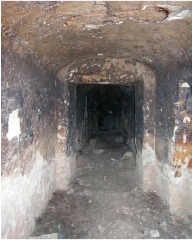
General view of the corridor (C) and doorway (E) with vaulted ceiling. Localized area of rock loss and basal erosion of walls and doorway are present.
