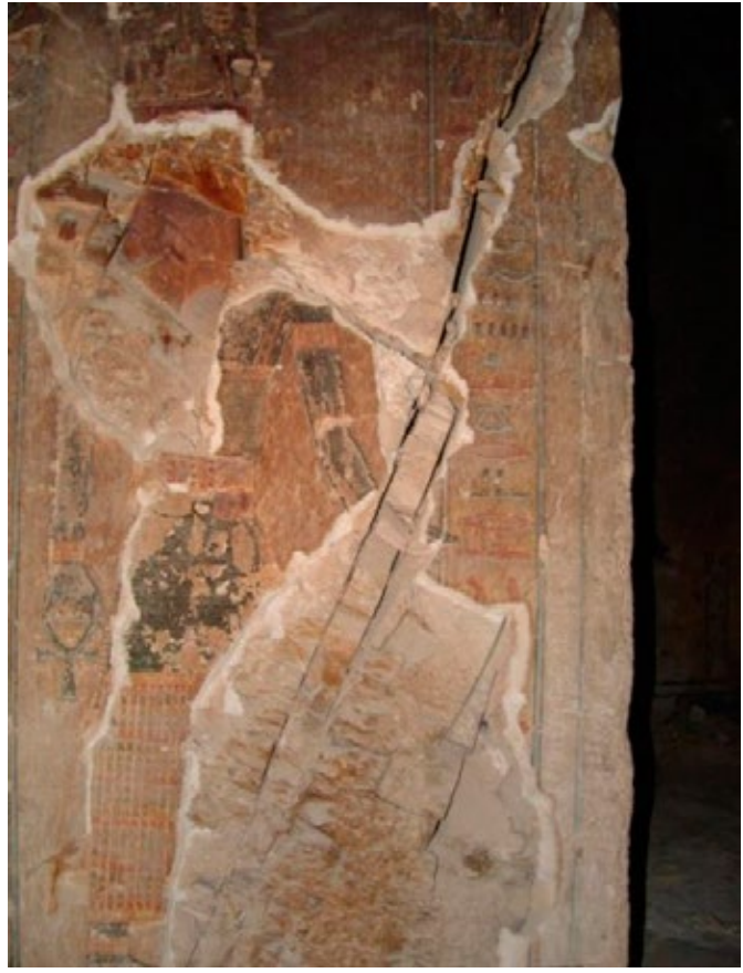
West face of pillar IV showing recent (likely 1989-91) edging repairs of wall paintings, but no change in rock fracture since 1977.
