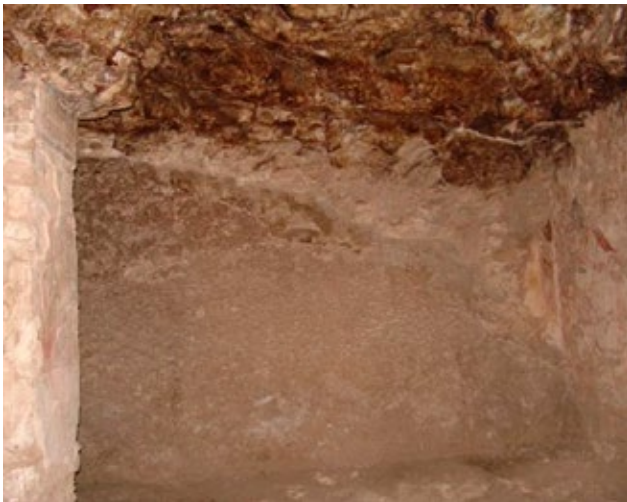
Rear wall of burial chamber (G) has salt accretions and there is almost no surviving decoration on this wall.
