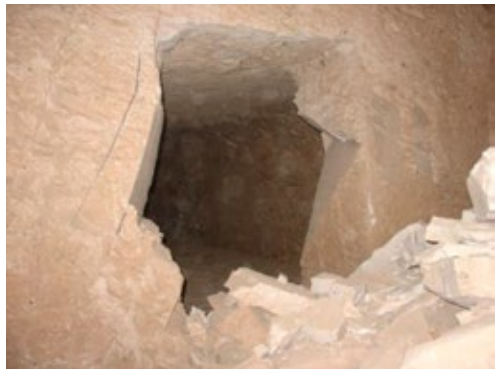
Partial collapse of door jamb between chambers (C) and (E).
