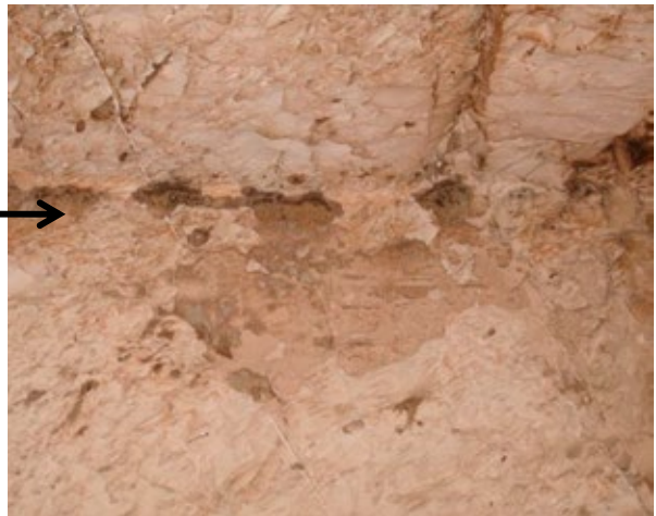
Right upper side chamber (M): small fragments of painted plaster appear heat damaged; paint layer looks to have been carbonized. In some areas the upper plaster layer has been lost which could be due to the fire damage.
