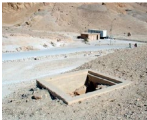
QV 81 entrance with masonry surround.
