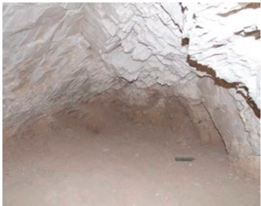
End of chamber with notable staining/discoloration along base of wall.
