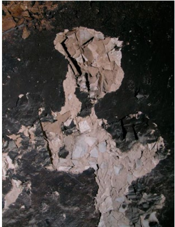
Post-fire loss in corridor (F) exposes areas of packing plaster and rock shards used to create a flat wall surface.
