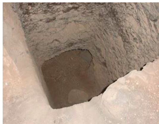
Interior shaft in side chamber, leading to lower chamber where bats were heard roosting.
