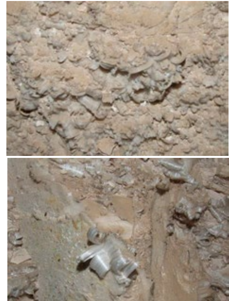
Above: Salt crystallizing on surface of rock in chamber (C). Below: fibrous salts.
