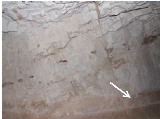
Water staining at base of wall (arrow); a line of chert nodules indicates the orientation of the bedding planes.
