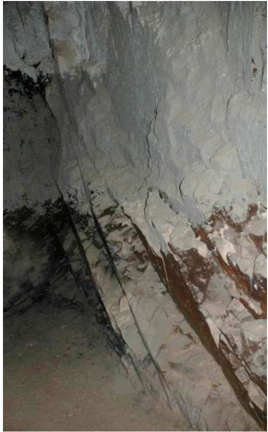
Steep joint planes in rear south wall of chamber (E) with recent rock plastering to prevent loss in upper part of the wall.
