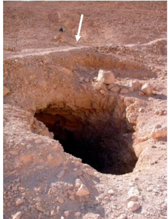
Shaft entrance, adjacent to footpath (arrow).
