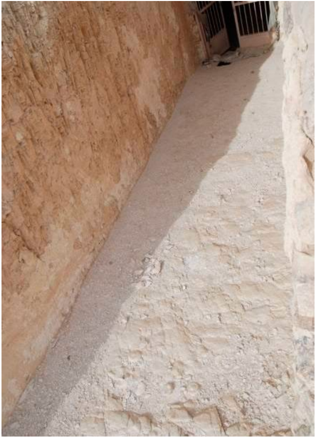
Ramp (A) once had steps, no longer extant. Plaster survives on lower part of ramp walls.
