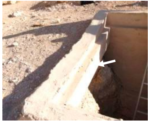
Detail of tomb surround. Arrow points to absence of rock beneath edge of surround.
