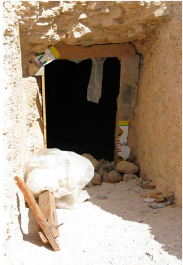
Above the entrance (B) are hanging fragments of rock.
