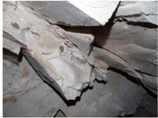
Detail of fractured ceiling rock with areas of salt efflorescence.
