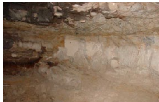
Overview of chamber (E) showing fractured and blackened rock.
