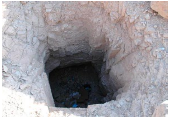
QV 3 shaft with trash accumulation at bottom.
