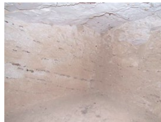
Fault visible in corner of tomb, with salt infill.
