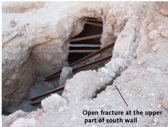
Overview of main chamber collapse, with view of shoring in side chamber. Open fractures at ground surface behind the area of collapse is evident.
