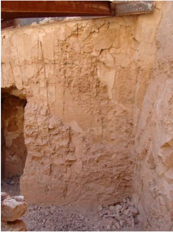
Area of painted plaster survives below steel, raking shoring on south wall of main chamber (C). This area of painting is in fragile condition as the rock support is highly fractured and susceptible to loss.
