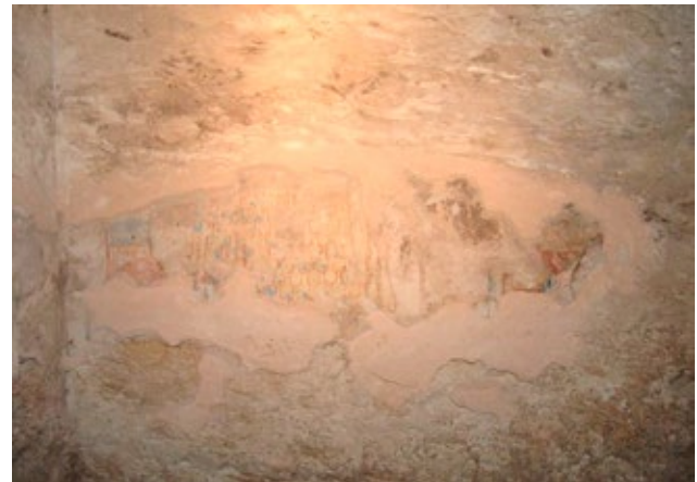
Same area in 2008. Significant areas of painted plaster have been lost.
