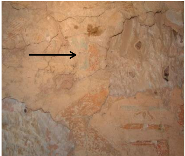
Only small traces of green paint survive.
