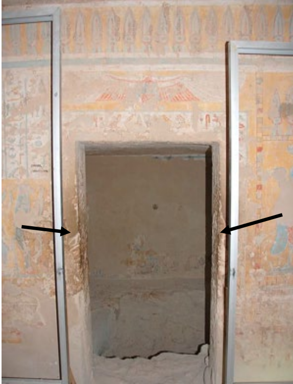
The sides of doorway (H) are unprotected and show staining caused by visitors touching the plaster.
