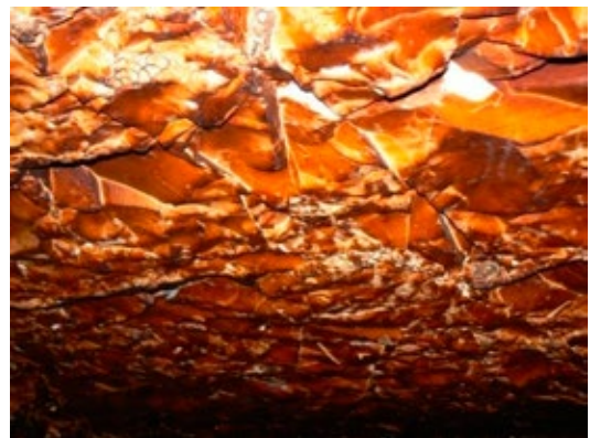
Detail of discolored rock ceiling in chamber (C).
