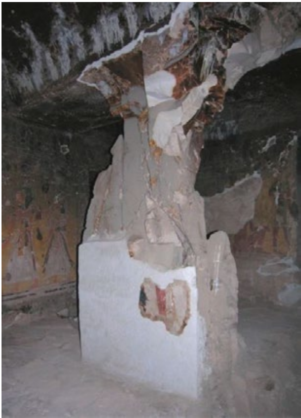
Fractured remains of pillar III in burial chamber (E) with recently reconstructed base of the south face, and post-fire loss on upper right side.
