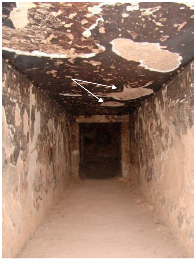
Corridor (C) looking south. Note line of blackening that rises up toward exterior door. Plaster loss on rear part of ceiling (arrows) occurred after Schiaparelli's mission, while loss near front of corridor (in foreground) was already present, based on photographic evidence (see D'Amicone and González 2008, fig 14).
