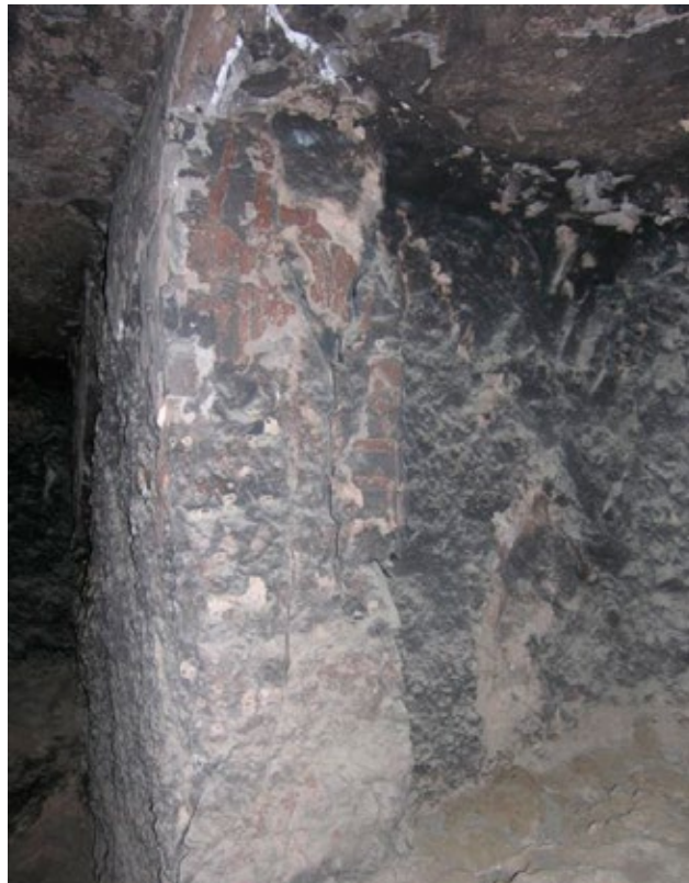
West jamb of doorway (K) to rear niche (L) has a large fracture but this is pre-fire and no adjacent loss has occurred.
