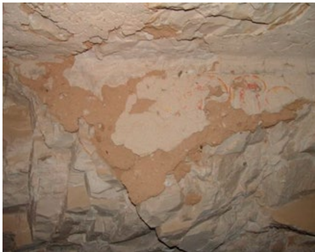
Multiple plaster layers are visible in chamber (L). Walls were filled with plaster and rock shards in preparation for painting.
