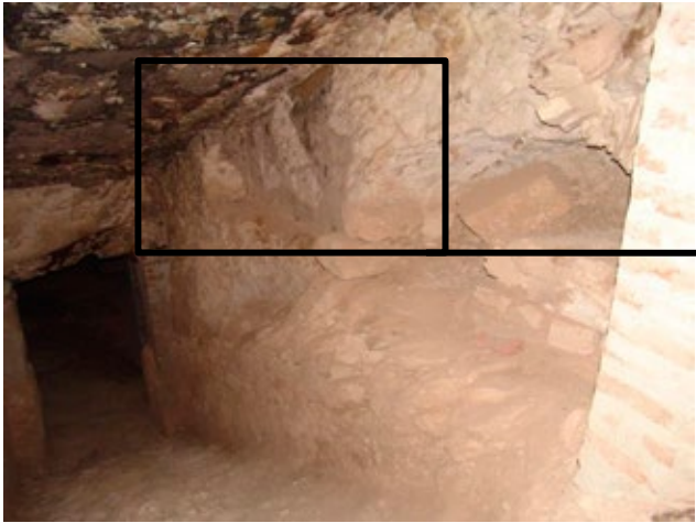
East side of corridor (E). Lower parts of the walls were built up with rocks.
