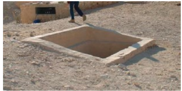
Shaft entrance with masonry surround.
