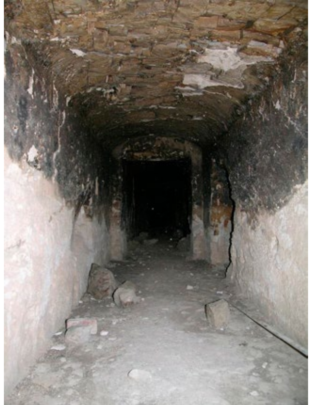
Corridor C: Fire damage rose upwards toward doorway (B), left. Looking from doorway (B) toward doorway (E), right. The lower part of walls of corridor (C) were protected from fire by debris.
