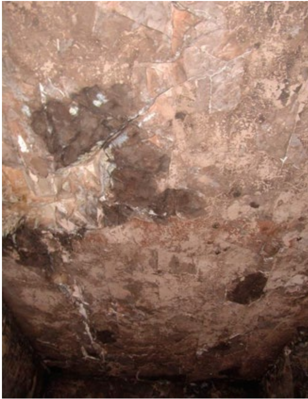
The ceiling of burial chamber (J) shows loss of rock along a fracture.
