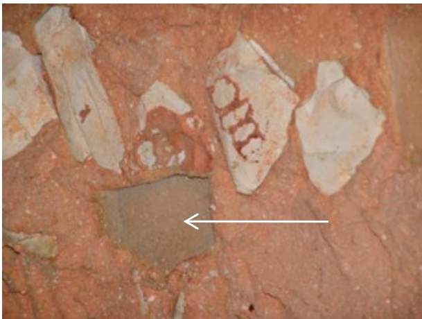
Stone shards are set into the plaster as filling material. Note area where stone shard has been lost. Plaster below this has been protected from the heat and has remained unaltered. It does not have the same pinkish color of surrounding areas where the plaster has been fired.
