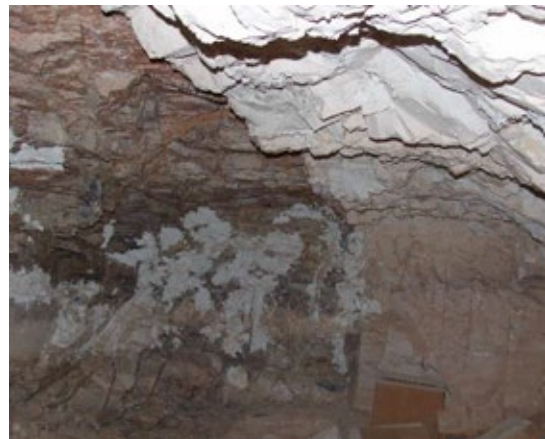
Chamber (E) showing relatively vertical interface between two rock types: dark shale on the left (with mortar interventions) and lighter marl on the right.
