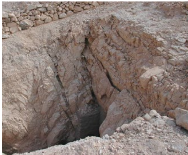
Open joints and related rock detachment above entrance.
