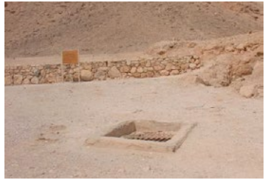
Shaft entrance and masonry surround.
