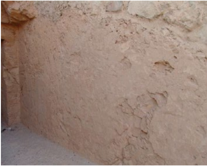
Side walls of entrance ramp (A) retain some original plastering.
