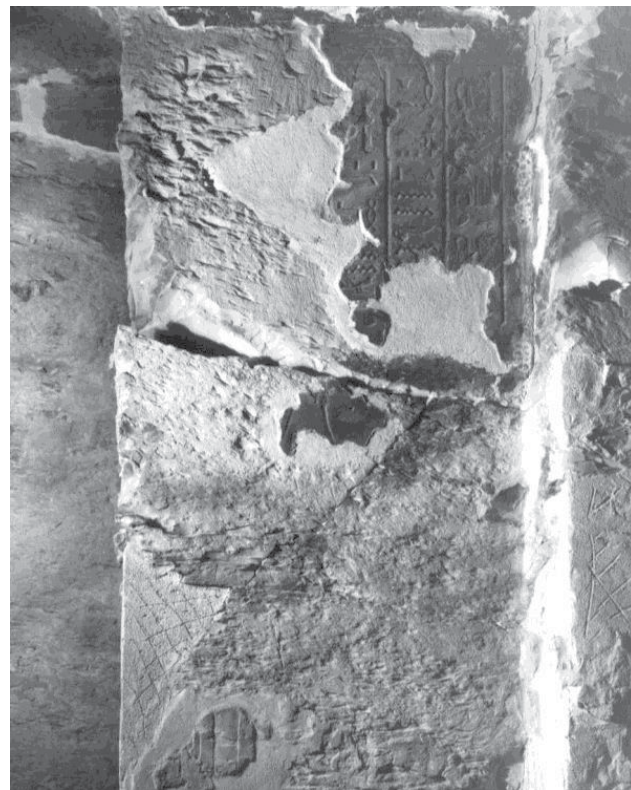
1987 CEDAE photograph of Doorway (D) showing area before loss.
