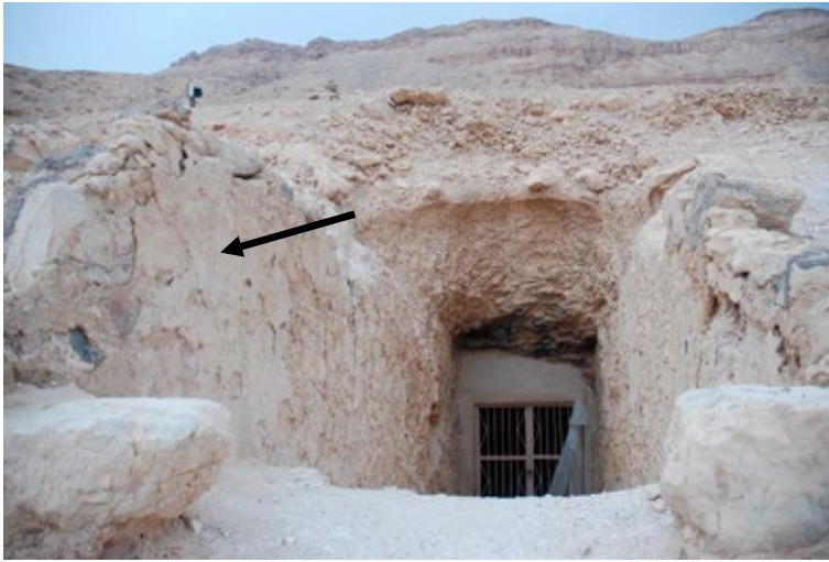
Rock overhang extends approximately 1m in front of entrance with some precarious large boulders in the debris fan located near the edge. Extensive surviving plaster on walls of left side of ramp (arrow).
