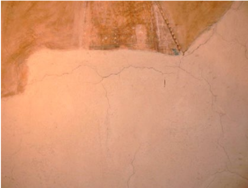
There are cracks visible in the substantial plaster repairs. As they conceal the condition of the underlying rock support these areas should be monitored to assess whether there are ongoing problems.
