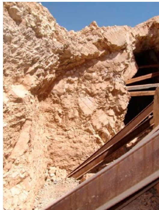
Evidence of ceiling vault on east side of main chamber.
