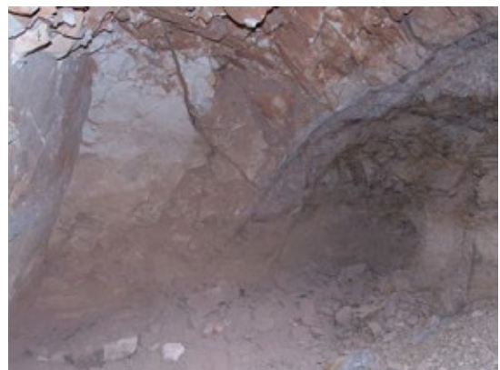
General view of chamber with piles of debris on ground.
