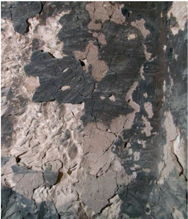
Surviving plaster in chamber (I) is fragile. Post-fire losses have occurred.
