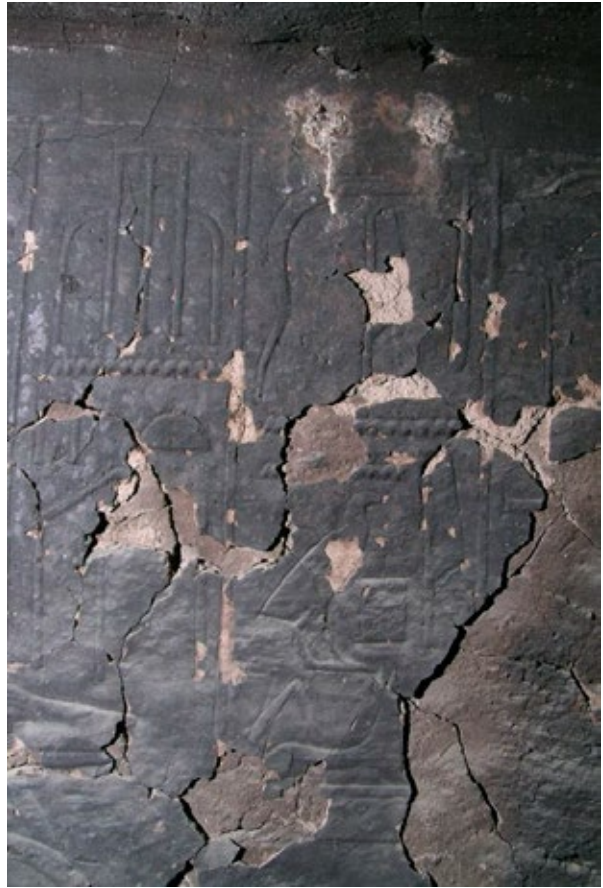
Post-fire losses have occurred throughout the tomb.
