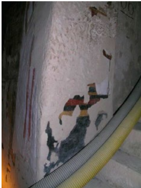
Doorway (B) has no barrier to protect painted surface. The ventilation ducts are in contact with the wall surface at bottom.
