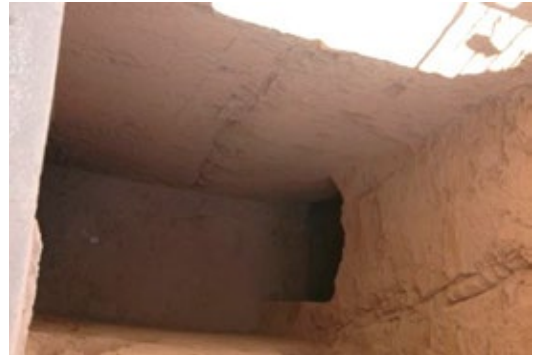
View of shaft from above.
