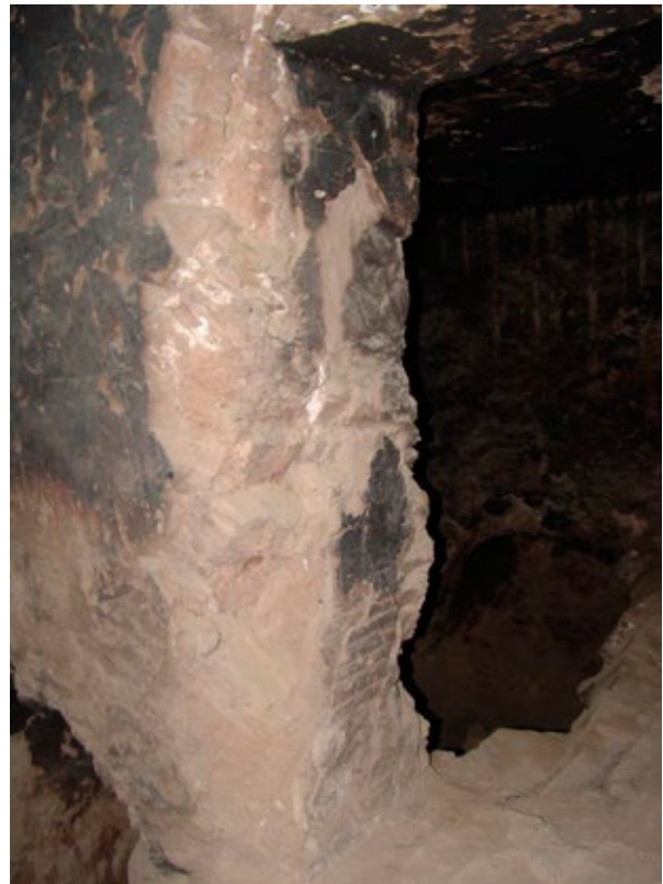
Large post-fire losses have occurred around doorway (D) of both rock and packing material
