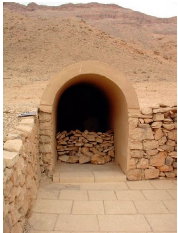
Arched cover and retaining walls on either side of entrance, with dry rubble wall at top of ramp as a barrier (later replaced by SCA with an iron gate).
