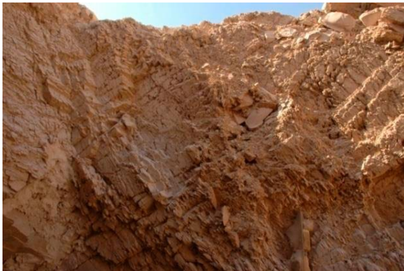
Fractured and friable rock above entrance.
