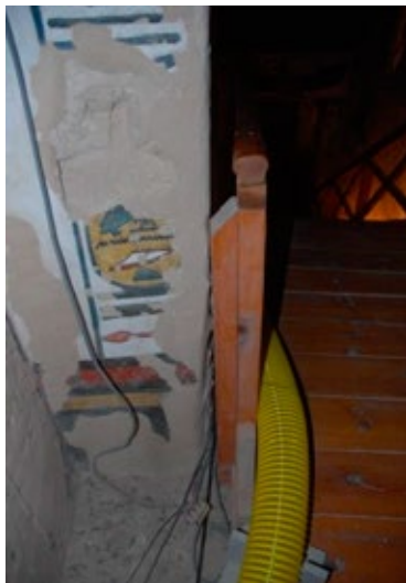
Handrail at doorway (H) is installed too close to the wall.
