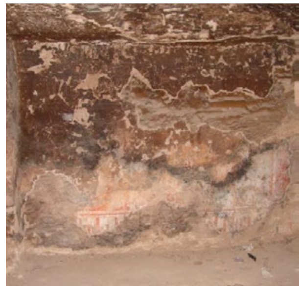
Lower parts of the walls in chamber (C) are not blackened having been most likely protected by sand and debris. Note mustard brown color of fire-related darkening in this chamber.
