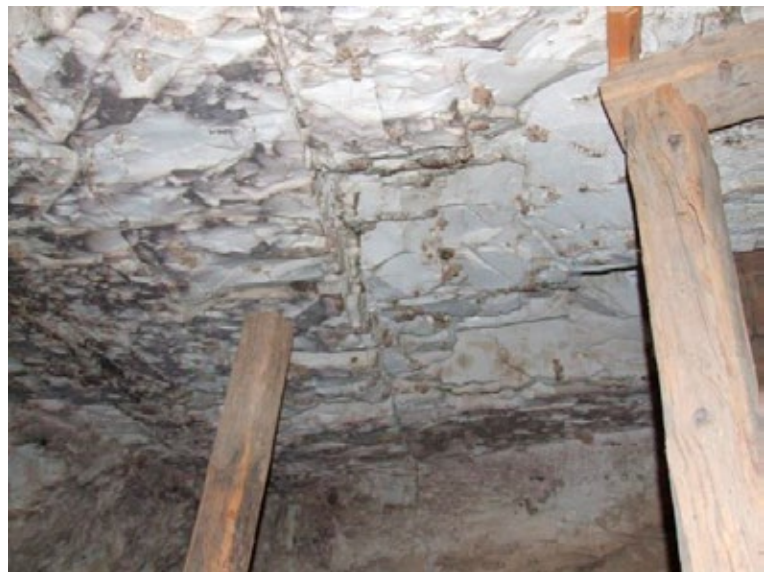
Fracture in ceiling of antechamber (C).
