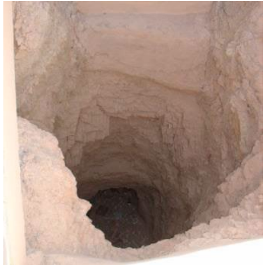
Shaft from above with shale along its length.
