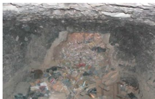
Chamber interior with blackened surface and trash on floor.
