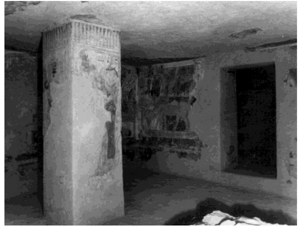
Chamber (C) in 1970 (CEDAE) showing plaster repairs already present. The extensive repairs did not allow for direct observation of the rock condition.
