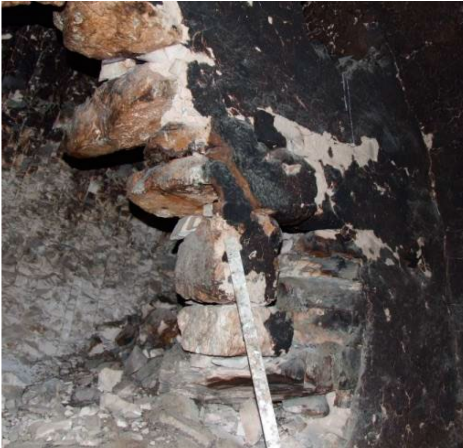
Detail of masonry wall of niche (O). This area requires stabilization to prevent further loss. Localized treatment of plaster may be needed in conjunction with this structural work.
