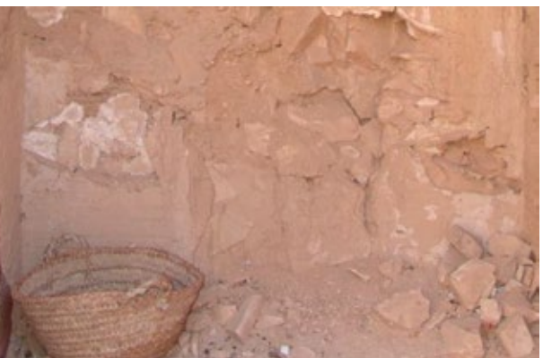
Detail of south wall of niche (G) in 1989 CEDAE photograph (above, left) compared with losses noted during 2007-8 inspection (above, right).
