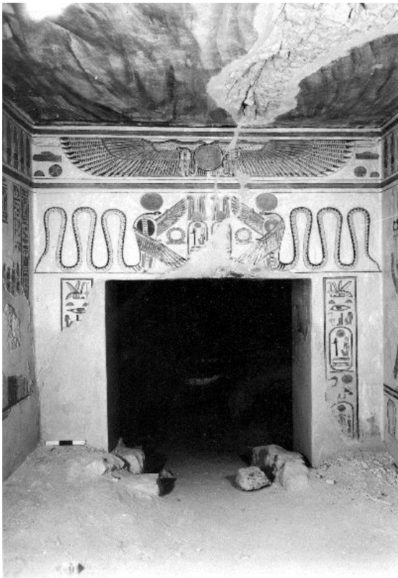
Fracture continues from corridor (G) to doorway (J) in 1974. Plaster on ceiling has been lost along the fracture (Image: CEDAE).
