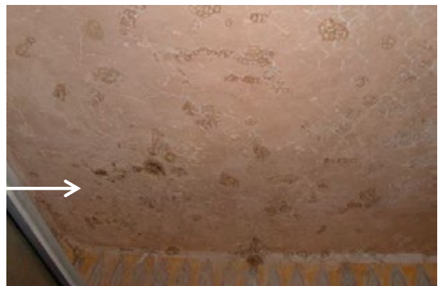
Detail of corner of chamber (E) showing concentration of deterioration and loss of painted plaster, possibly due to bats.
