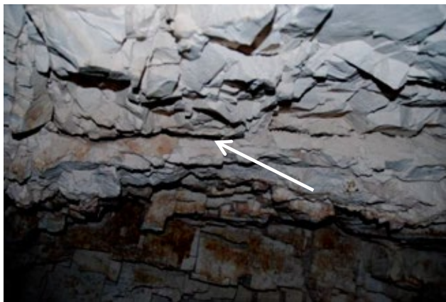
Ceiling of rear chamber (E) is heavily jointed and fractured with areas of detachment.
