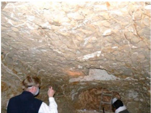
View of the fractured ceiling of chamber (C) facing the tomb opening (background).
