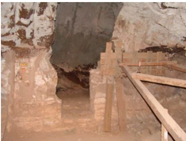
South wall of main chamber (C). Current wooden shoring is covering areas of painted plaster. Substantial amount of original fill plaster also survives on this wall.
