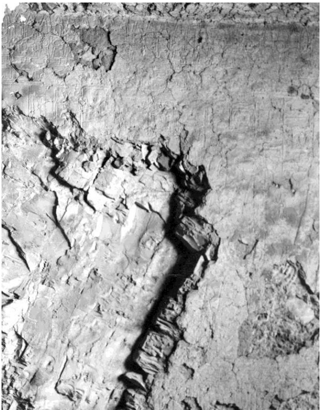
A large area of loss on the west wall in chamber (C) in 1985 (Image: CEDAE).
