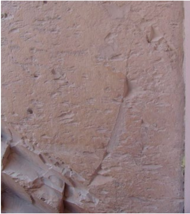
High quality of rock allowed for extremely fine working of the surface. Only a very thin layer of plaster was needed to cover the walls.
