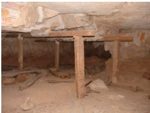
Existing wooden post and beam shoring in rear chamber (N_P).
