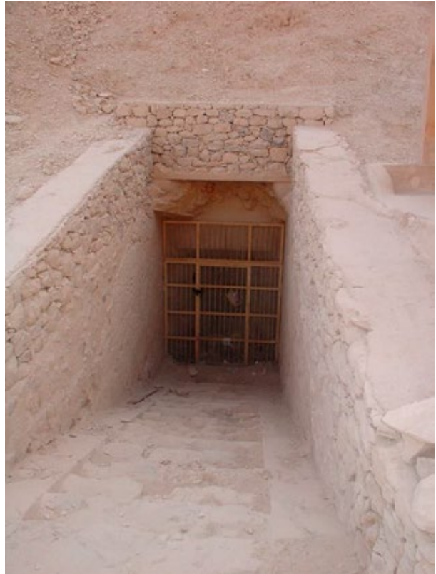
View of tomb entrance with modern masonry retaining walls lining ramp and above entrance.
