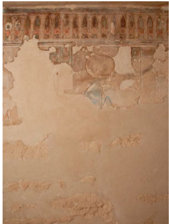
Repair plaster was applied to all areas of rock loss. The exact date of this work is unknown (Image: CEDAE 2009).
