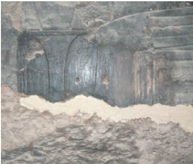
Localized edging repairs and a small cleaning test on the north wall of chamber (C).
