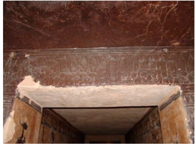
There is cracking around doorway (F) though very little post-fire loss of plaster.
