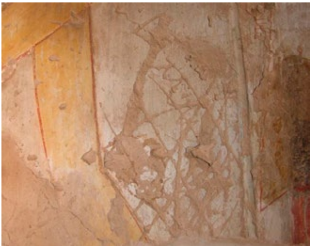
Image above left: Small losses and intentional scratching of painted surface contributes to an overall fragmentary appearance of the painted plaster in antechamber (C).
