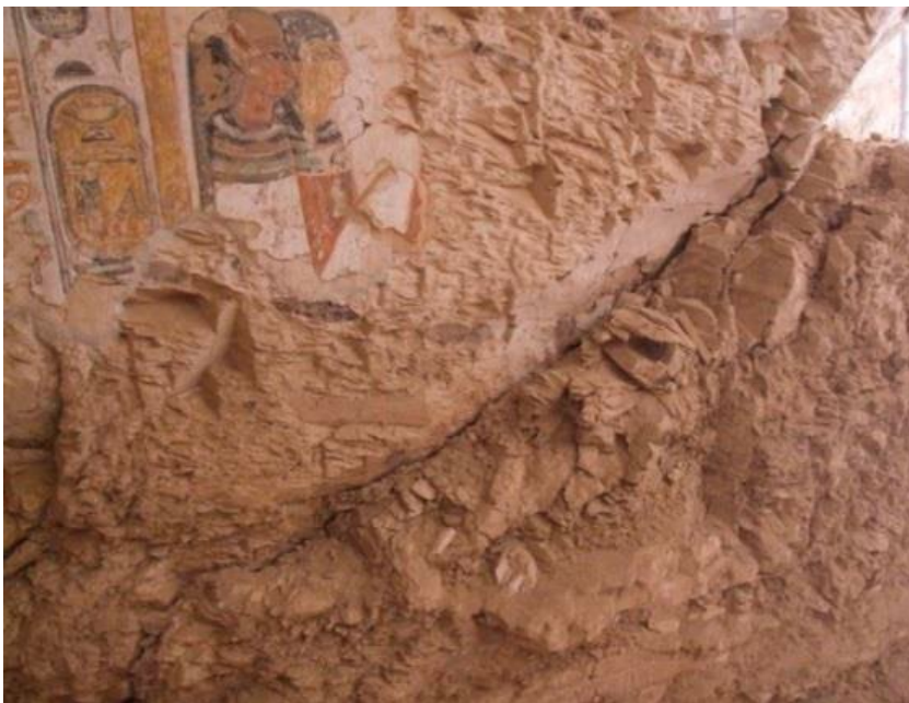
Area of rock fracture and loss adjacent to basal deterioration of wall
