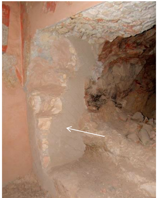
Niche (G) showing gray cement repair plaster. The repair has been scored in preparation for the final pink-colored finishing plaster that was never completed in this area.
