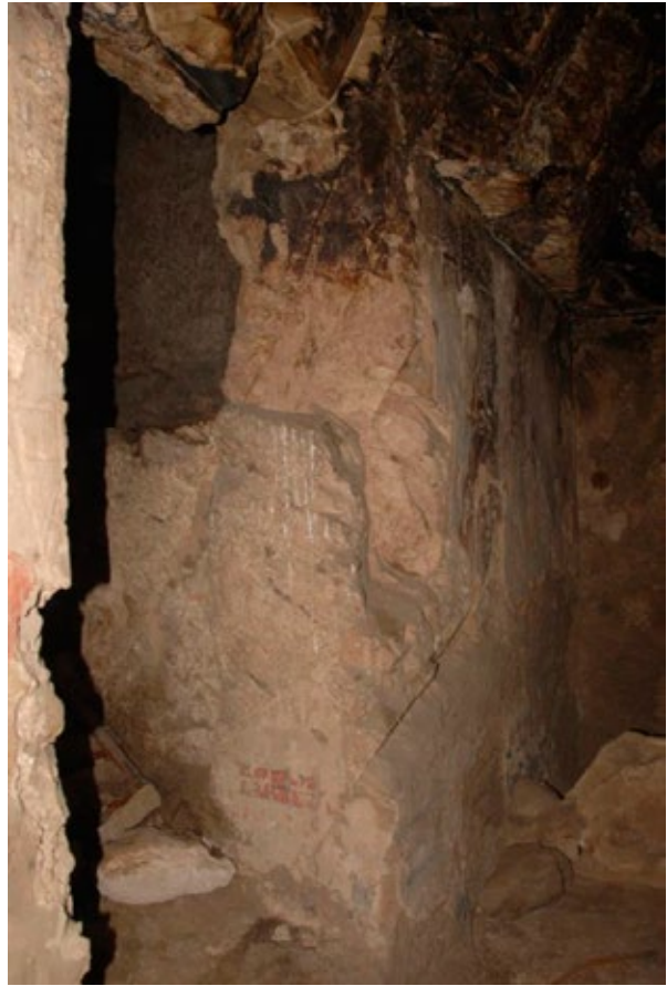
Localized loss and fracturing can be seen on doorway (F) (Image: CEDAE 2009).
