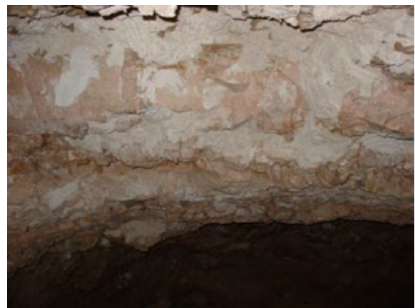
Cement mortar applied to ceiling.
