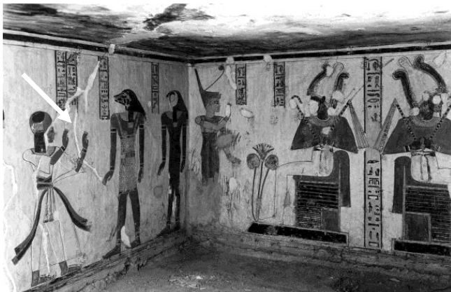
Large cracks can be seen in side chamber (G) that extend across ceiling and walls (Image: CEDAE).
