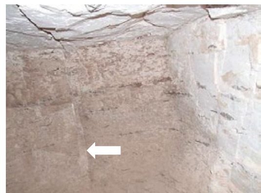
Corner of tomb with fracture running through ceiling and wall.
