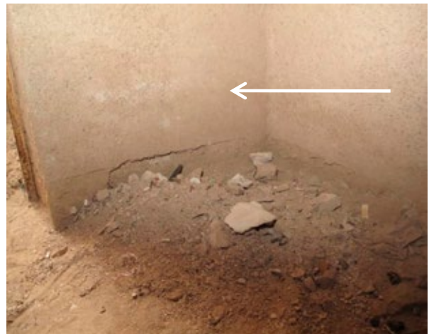
Staining (0.15m high from the ground) at the base of the wall in chamber (C) on repair plaster most likely from the 1994 flood.
