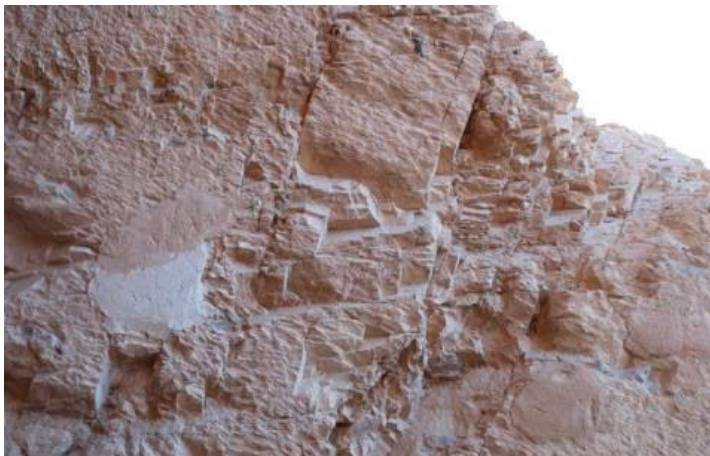
Patches of modern plaster tests.
