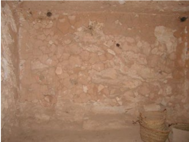
South wall, side chamber (E). Almost all of the upper painted plaster is missing. Note the network of cracking in the plaster. There is no straw in this plaster and it is possible that this could be the reason for the drying cracks.
