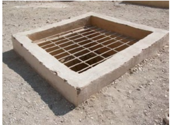
As of Dec. 2009, the SCA had installed a masonry surround with a metal grate.
