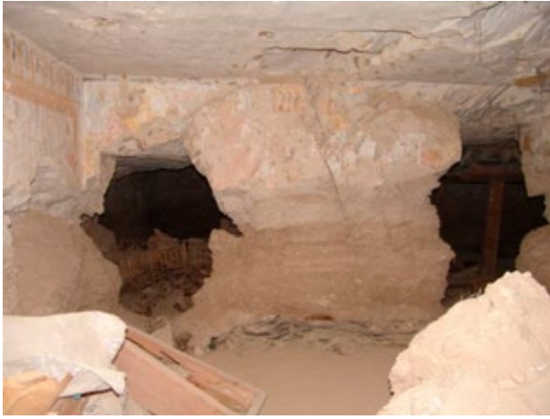
At risk area around doorway (D) between chambers (C) and (E) and doorway (H) between chambers (C) and (I).
