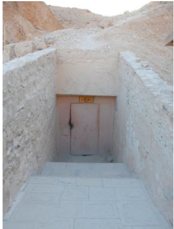
Ramp (A) with modern constructed steps and entrance (B). The retaining walls were re-built after the 1994 flood. (CEDAE 2009)
