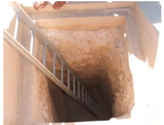
View of shaft from above.
