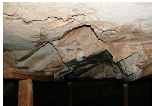
Large block at risk of collapse.
