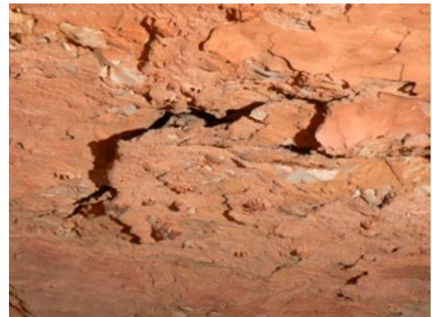
Areas of detached plaster on ceiling of burial chamber (E).
