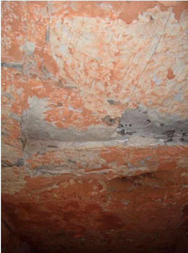
Heat-related damage of ceiling plaster of burial chamber (E) shows a firing of the earth-containing plaster. Rock loss has also occurred here some of which may be recent.
