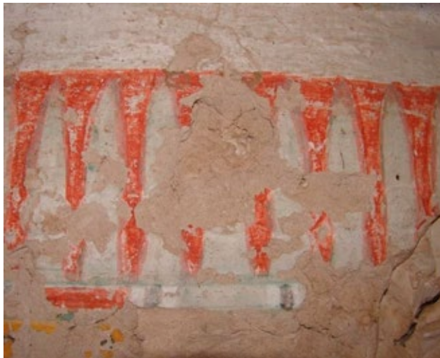
Image of the top band of decoration in main chamber (C) showing the fragile nature of the surviving painting. Note general losses in the paint layer and the cracked and unstable edges of the painted plaster around area of loss.
