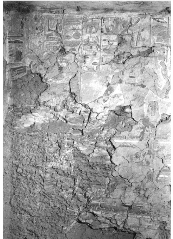
North wall of pillared chamber (C) before treatment in 1987 CEDAE photograph.
