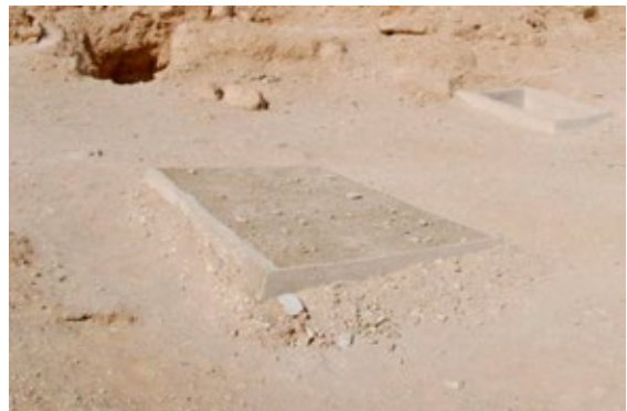
Shaft opening after the installation of the prototype shaft cover.
