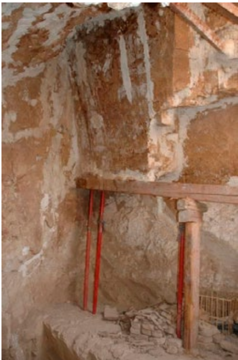
Existing shoring in side chamber (E).
