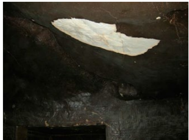
Recent area of plaster collapse in chamber (G) in 2009. This area was then treated by the SCA. Other areas of plaster cracking should be further investigated as it might indicate remaining areas of plaster instability.
