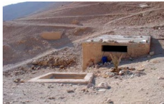
Proximity of entrance to old generator building (since removed).
