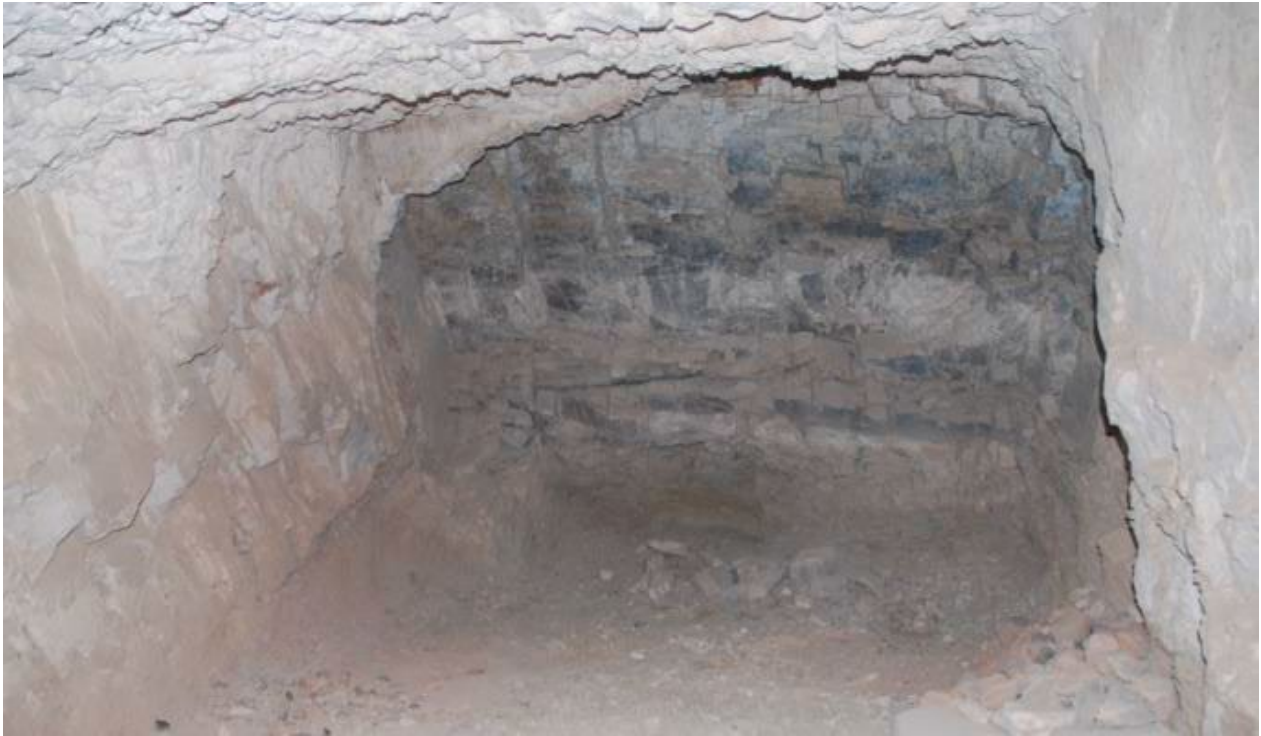
The rear part of chamber (E) is cut out of a shale stratum that is heavily jointed. Fallen fragments on the floor are evidence of recent rock loss from the walls and ceiling.
