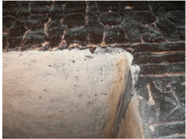
The area around doorway (F) has been whitewashed as part of the previous treatment interventions in the tomb. Note how the whitewash was applied over areas of original blackened plaster.
