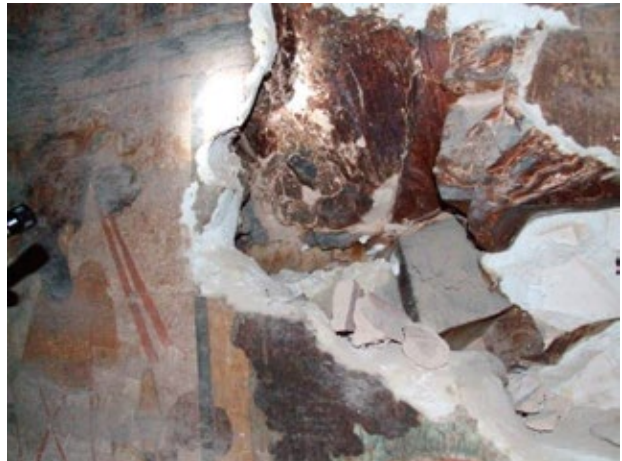
Detail of area of loss on the north wall of burial chamber (E). A gap exists behind the wall plaster.
