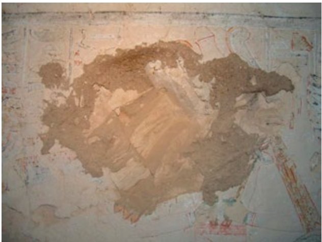
Mud plaster, thought to be Coptic period, was used to fill holes in chamber (G).
