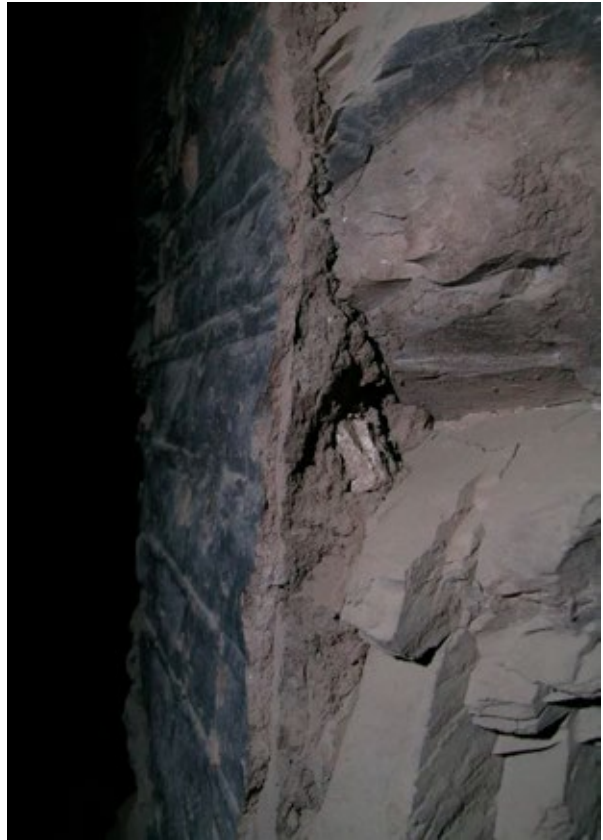
Note irregular surface of rock wall and the rock shards and large amount of infill plaster used to create a flat surface for the decoration.
