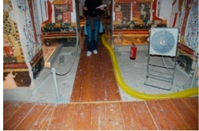
Wooden walkways, fans, fire extinguishers and ventilation ducts are installed in the tomb. Walkways are narrow and too close to walls allowing visitors to touch the walls.
