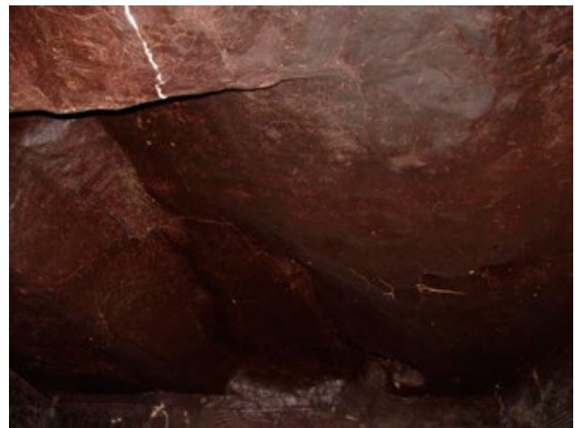
Irregular ceiling of chamber (G) with surviving plaster indicates that ceiling was never flat.
