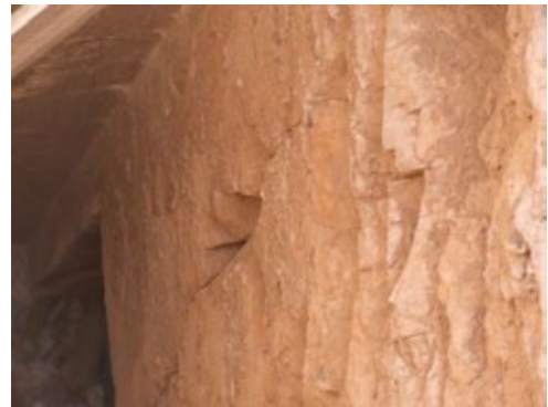
Vertical fracture running down south side of shaft as seen from above.
