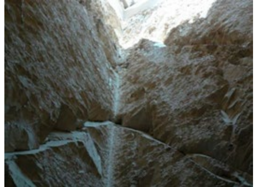
Shaft walls with open diagonal fractures.
