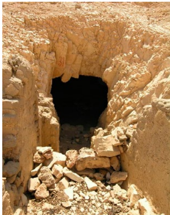
Ramp and Entryway in 2007. Fractured and falling rock along ramp and outside entryway; mudbrick walls lining the ramp; dry rubble wall in foreground placed in recent times as a barrier.
