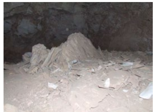
Evidence of ceiling collapse in center of chamber (C).
