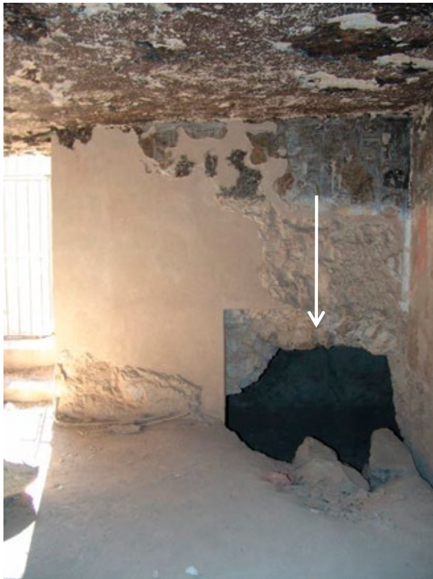
Opening (L) in the southwest corner of chamber (C) leads to lower chamber (M), thought to be a later addition.
