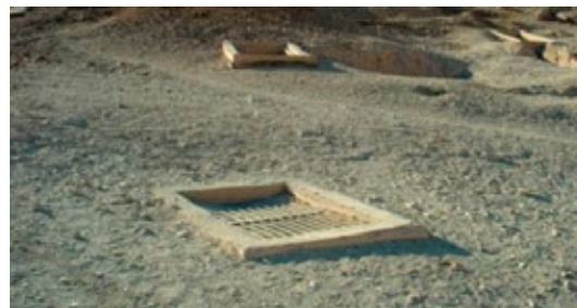
Shaft entrance with surround.
