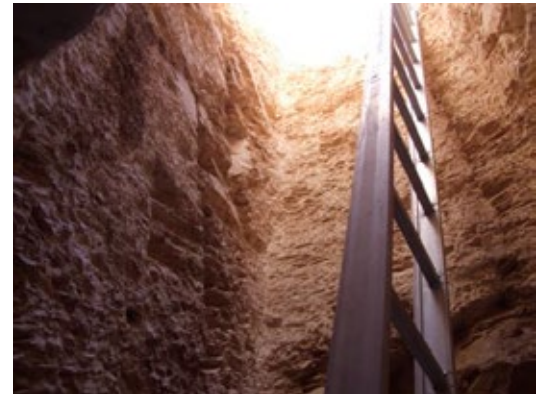
Shaft in relatively good condition.
