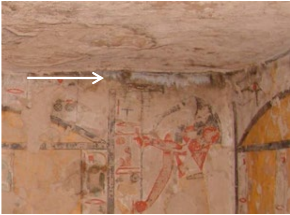
Evidence of bats on the upper part of walls and ceilings in the side chamber (G), in the form of crystalline deposits (salt residues) and staining. The problem is already evident in the 1973 CEDAE photographs (right).
