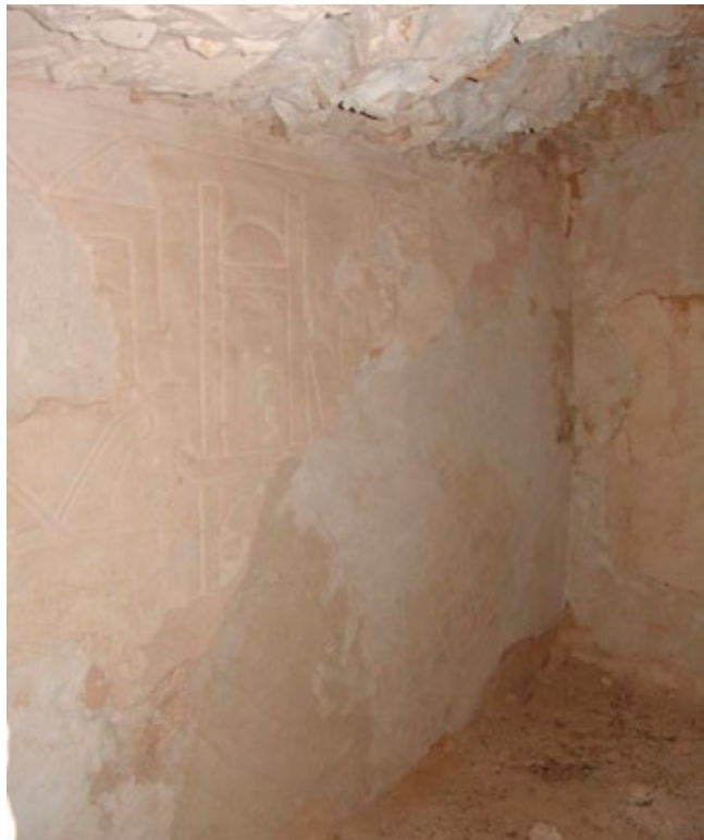
1984 CEDAE photograph (left) shows a large and deep area of loss. The 2008 photograph (right) shows same area with large repair plasters and areas of the ceiling rock secured with plaster.
