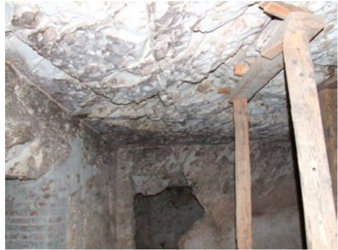
Fault plane in ceiling of antechamber (C) continuing to doorway (L) with adjacent rock loss.
