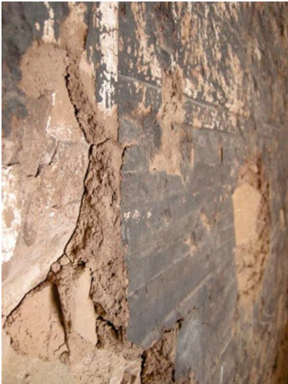
The ceiling of chamber E in tomb QV 51 was plastered and rock shards pushed into the plaster to minimize shrinkage.
