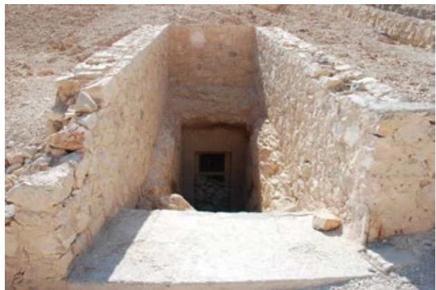
Stepped ramp (A) and entrance (B) in 2008. The irregular overhang of rock over entrance (B) indicates some rock loss has occurred in the past. Stone ramp walls were repaired and plastered in 2010 by SCA.
