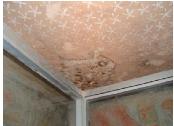
Bat-related damage in the corner of ceiling of chamber (K).
