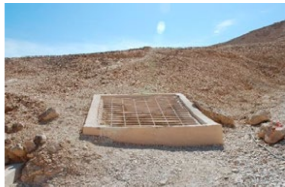
QV 6 shaft entrance with surround installed in 2009.
