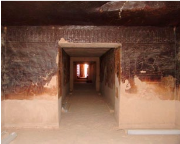
There is cracking around doorway (F) though very little post-fire loss of plaster.
