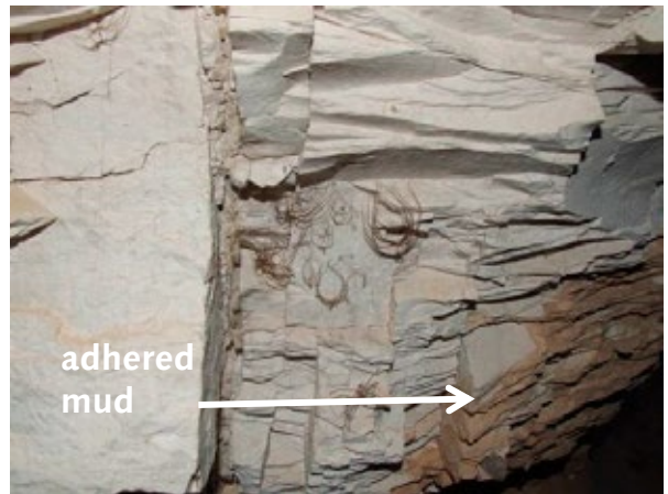
Detail of wall with an area of adhered mud on the lower right, evidence of past flooding.
