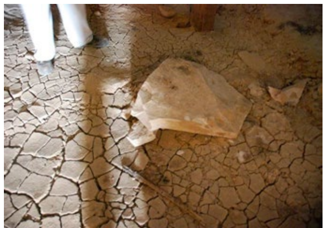
Thick layer of mud brought in by the 1994 flood in chamber (I).
