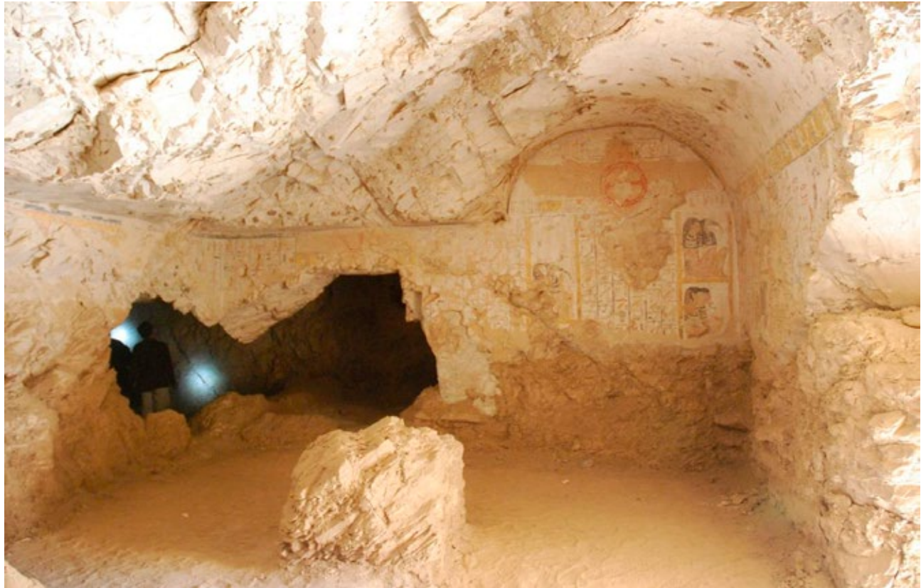
View of main chamber (C), east wall, with partial pillar, basal wall deterioration, ceiling loss, and rock fracturing.
