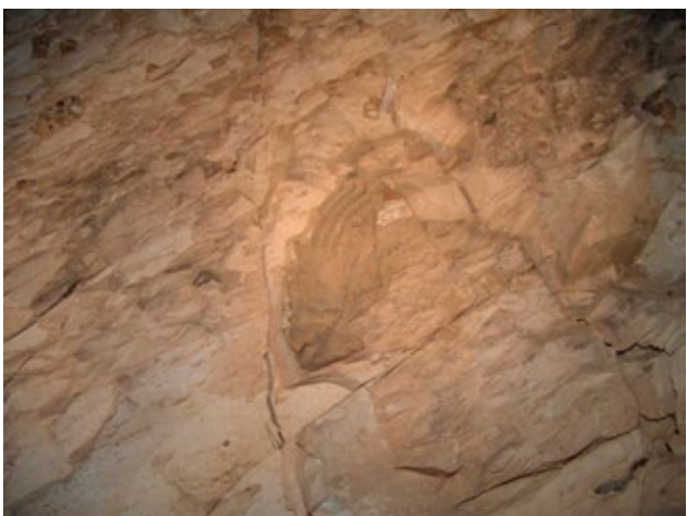
Upper parts of the walls in antechamber (C) have only small patches of surviving plaster that are blackened and heat damaged from fire.
