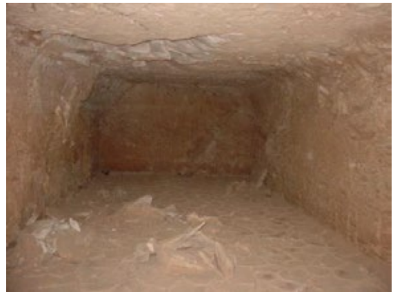
Third chamber (on CNRS sketch below) with localized ceiling rock collapse.
