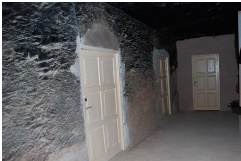
General view of blackened tomb interior of chamber (B) and modern doors to storage areas, looking east (2009).
