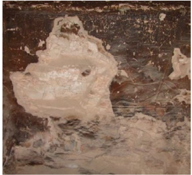
Large post-fire loss on north wall of side chamber (I)
