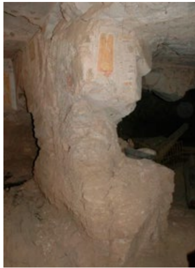
Basal erosion and fracturing of the two remaining piers within tomb. Basal rock is fragile and is incapable of supporting upper portion of rock.
