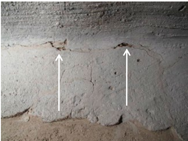
Other small loss along crack.
