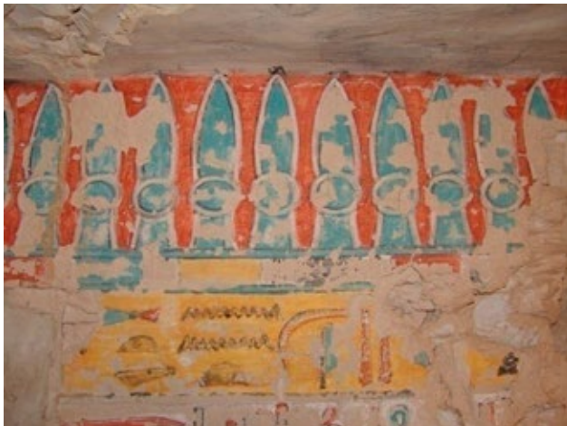
Flaking of the paint layer has led to substantial losses that expose the underlying plaster layer.
