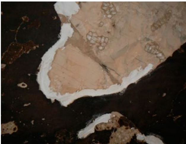
Edging repairs stand out starkly against the heavily blackened ceiling of the corridor. Note that this loss in the plaster is post fire.
