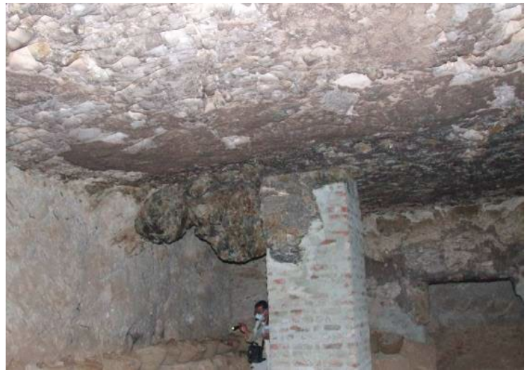
NW pillar in chamber (G), showing surviving top of the rock pillar and reconstructed part below. Thick chert concretion on fire-blackened ceiling indicates major fault zone. Areas of plaster survive at tops of pillars and on ceiling.
