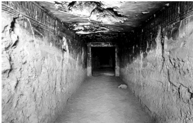
1977 photograph of corridor (C) shows the tomb before any treatment (Image: CEDAE). Note large voids in rock on ceiling and walls. Note also line of blackening that rises up toward the entrance of the tomb.
