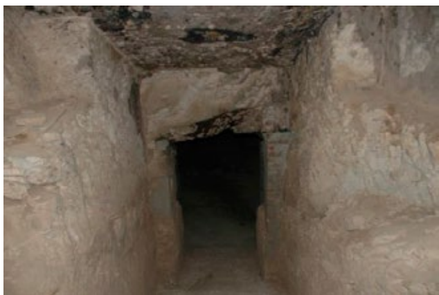
Ramped corridor (E) showing carved ledges of side walls and areas of loss, and rebuilt doorway (F).
