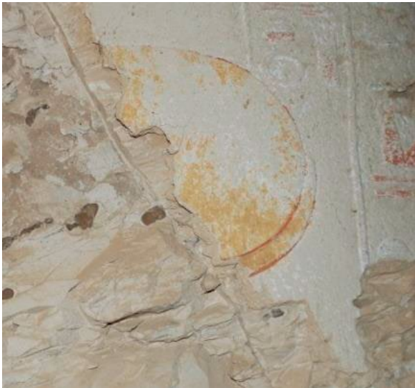
Detail of area of loss on the east wall of chamber (I) showing rock suffering from salt-related deterioration and pitting of the painted surface, also possibly caused by salts.
