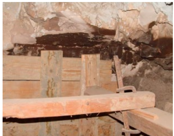
Detail of shoring that is covering areas of painted plaster.
