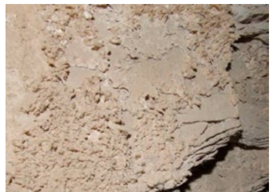
Fibrous halite crystal growth on rear wall of chamber.
