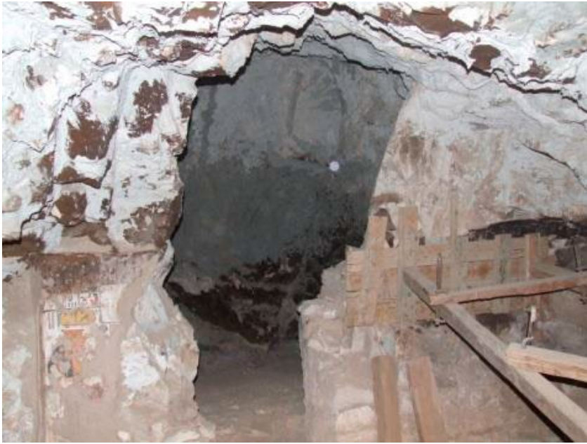
View into burial chamber (E) from main chamber (C). Wooden shoring on the right supports fragile internal wall; white plaster was spread liberally over ceiling rock in an attempt to prevent rock fall.
