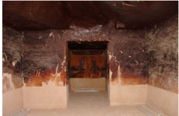
Main chamber (G) as it appeared after interventions (photo 2007).
