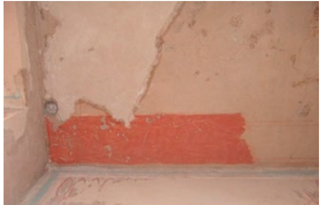
Ceiling in the corridor is unfinished. Setting out lines are visible in one corner but the painting was never finished.
