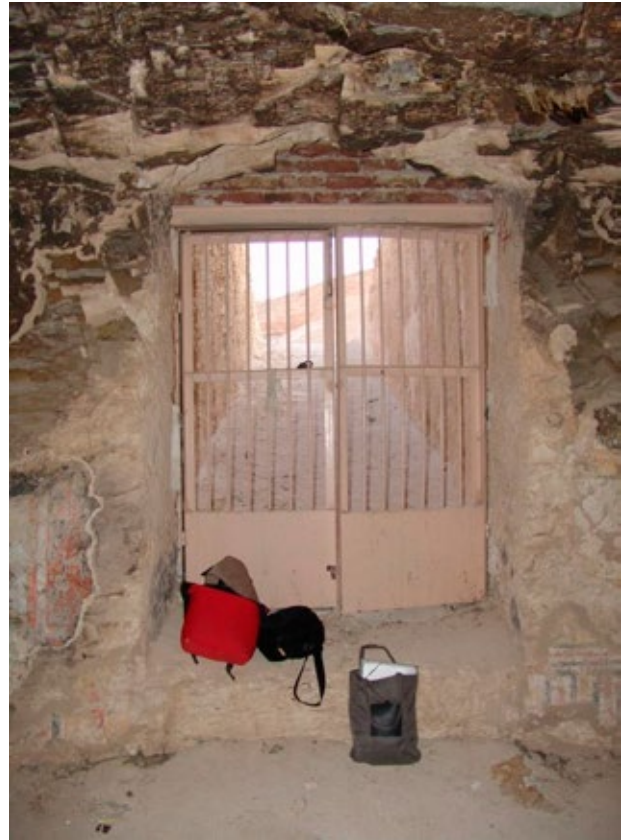
Doorway (B) has a rebuilt fired-brick lintel and metal grill door without mesh.
