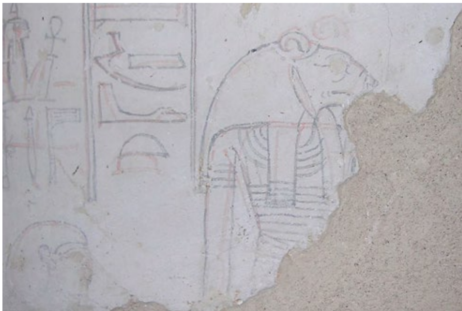
Same area on the north wall, west side of chamber (C) taken in 2006 indicating that the repaired areas have remained stable.
