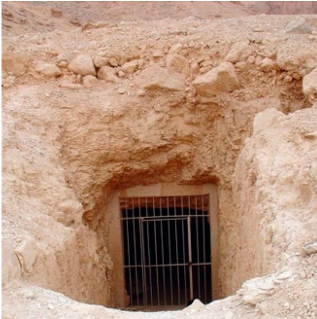
Entrance ramp (A) has heavily weathered marl and a large area of rock loss in the east wall (see also image right). A short overhang of marl rock above entrance doorway (B) exhibits some cracking and disaggregation. Stability of large boulders above entrance and ramp walls is required.
