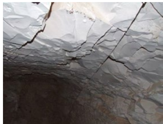
Fracture running through ceiling and wall of chamber (E).
