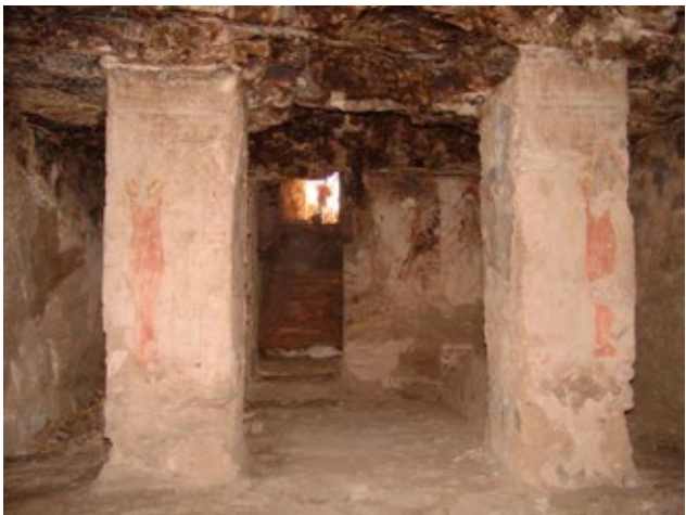
Note extent of surviving painted plaster on pillars of chamber (G) and that fire blackening was only on the upper parts of walls and on the ceiling. The lower parts of the walls and pillars escaped serious fire-related damage.
