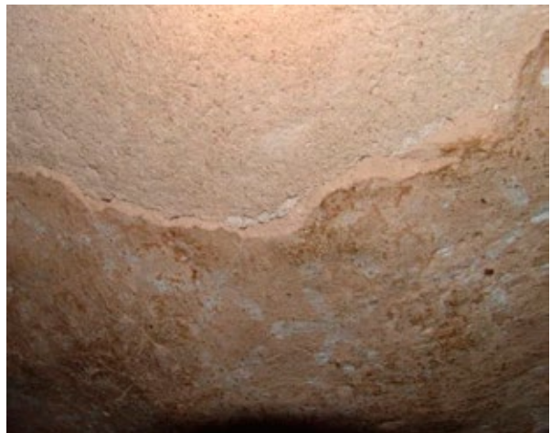
The plaster repairs are slightly recessed from the level of the painting.
