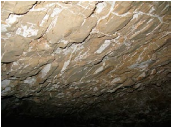
Extensive salt or gypsum deposition (white) in joints of the ceiling.
