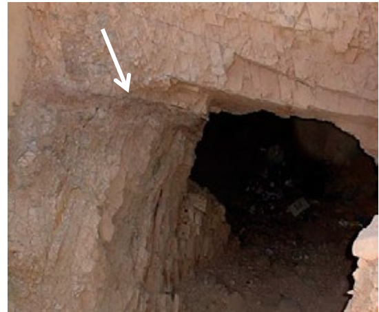
View down shaft with evident marl and shale interface (indicated by arrow).
