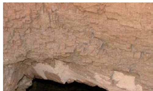
QV 16 entry shaft showing cream-colored fractured marl above grey shale (above); detail of shale (below).
