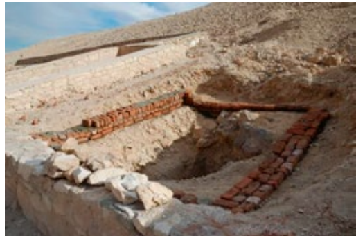
Construction of a new masonry surround by SCA in progress in December 2009.
