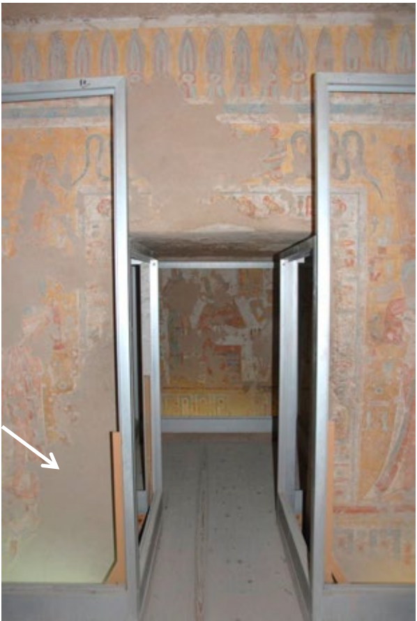
Jamb of doorway (F) in 2008 showing large loss having been reconstructed.
