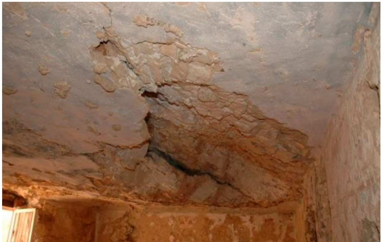
Open diagonal ceiling fracture with adjacent areas of unstained rock, indicating loss in the past.
