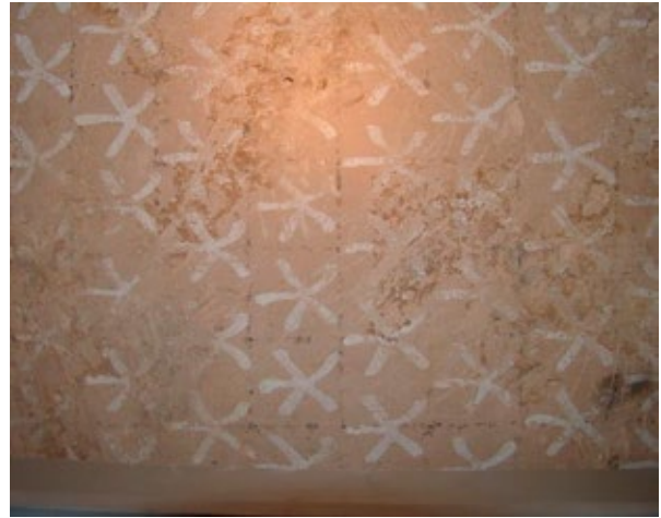
Black snapped lines were used on the ceiling to form a grid for painting the white stars. The beige color of the starry sky ceiling is unusual, a dark blue background color being more typical. It is not known if the effect is intentional, or the result of alteration, or some other cause.
