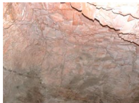
Reddish coloration of heavily jointed ceiling.
