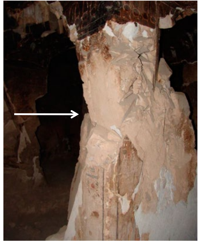
Losses of rock and painted plaster on pillar III in burial chamber (E) can be seen since 1977 photograph (left, Image: CEDAE).
