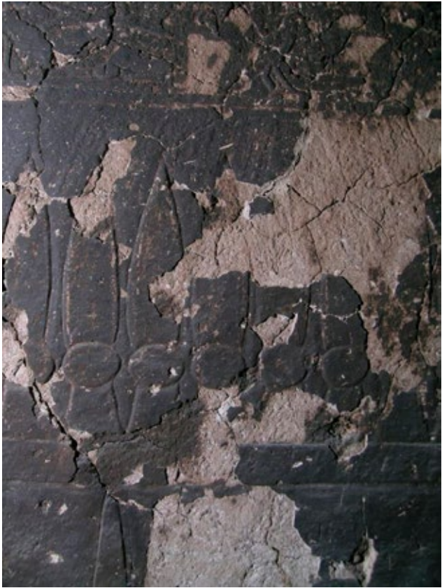
Note cracking and post-blackening losses of the thin upper decorated plaster layer.
