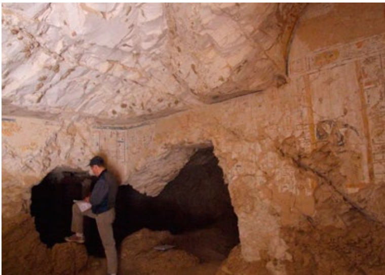
QV 60, shown here, exemplifies some of the severe rock related problems of tombs affecting their structural stability and wall paintings.
