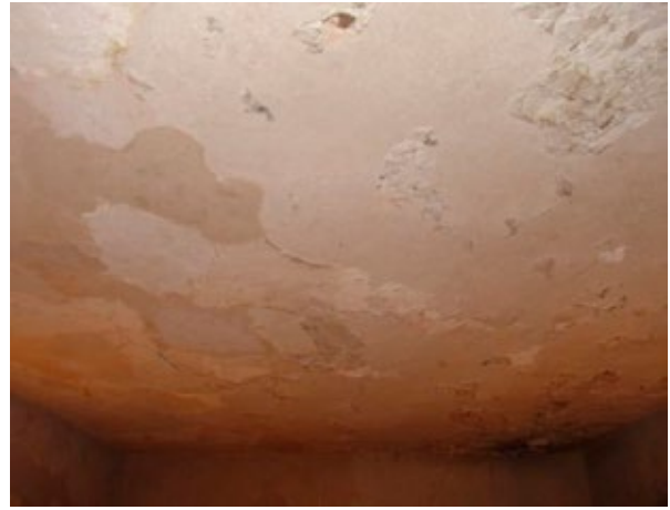
The ceiling of the rear chamber (K) has a number of different types of plaster repairs indicating ongoing losses in this area of the tomb. As the ceiling is extremely low it is recommended that access to the chamber (K) be limited and that the ceiling be monitored.
