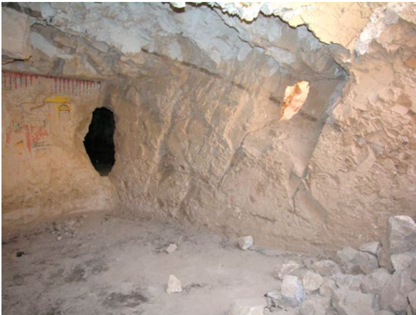
Break in west wall of chamber (C) (right) requiring infill for stability of rock above. Note diagonal band of chert and surface repair plastering of the ceiling rock to prevent further detachment and loss.
