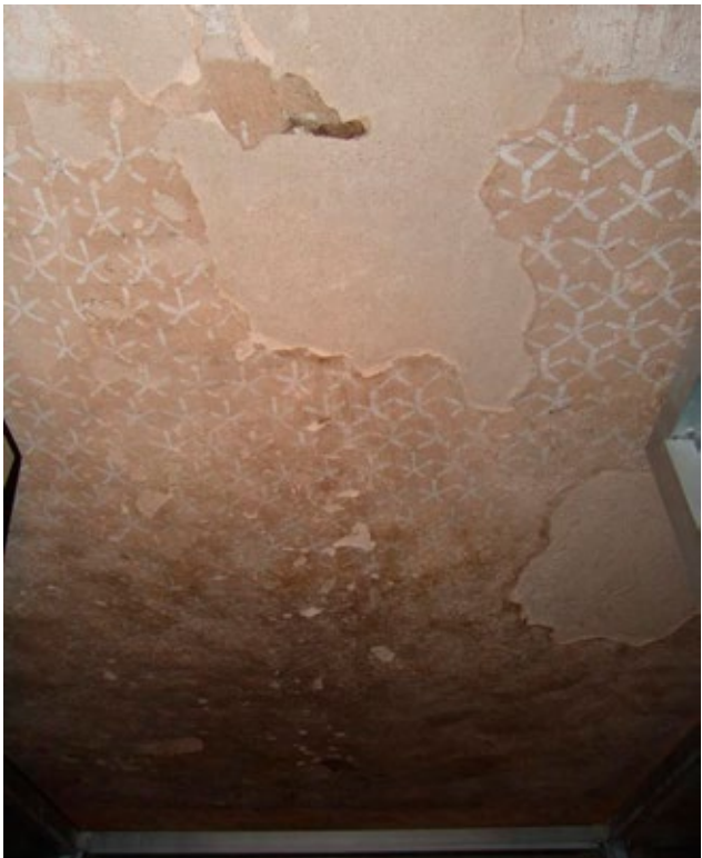
Losses in ceiling of chamber (G) have been filled with plaster repairs.
