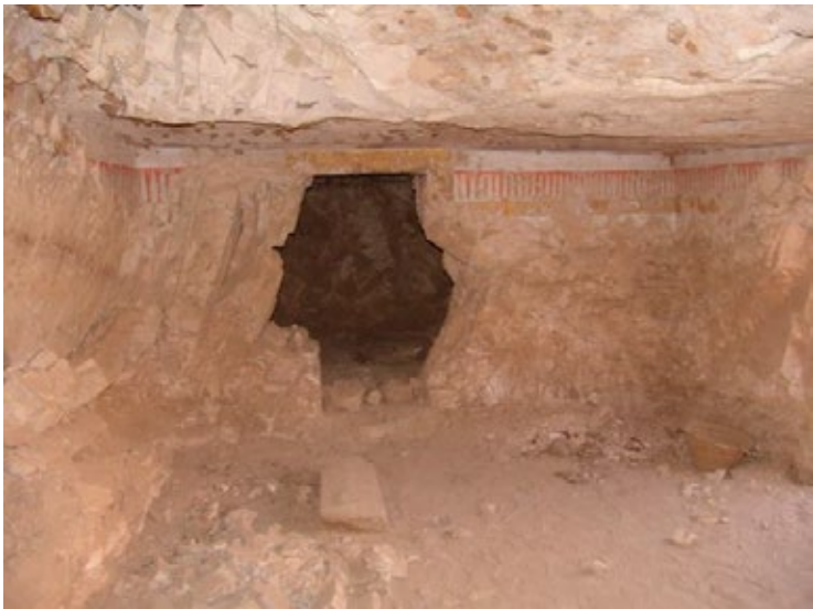
Main chamber (C), view towards doorway (D). Fractures with resulting loss along rear wall of tomb; painting only survives in this chamber along upper portion of wall; a large area of ceiling plaster is also extant (photo 2007).
