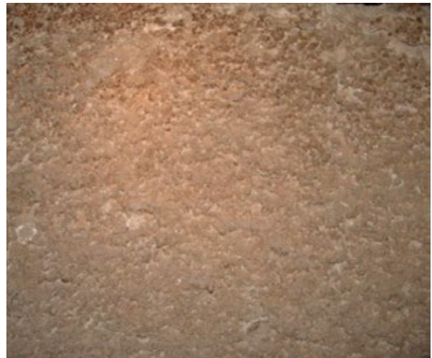
Detail of salt accretions on rear wall of burial chamber (G).
