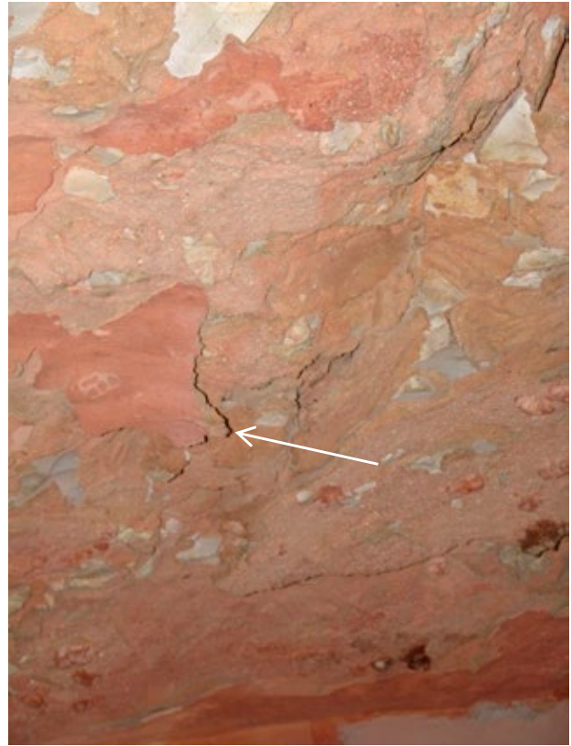
The firing has made the plaster layer rigid and brittle. The upper layer is detaching from the plaster layer below. This lower plaster layer has rock shards set in it to serve as infill material.
