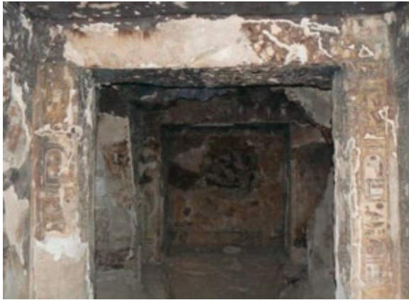
View of doorway (D) into burial chamber (E); jamb loss and repair, and loss of original mortar repair and painted surface since 1977 are visible in foreground; the sunken floor of the burial chamber is in the background.
