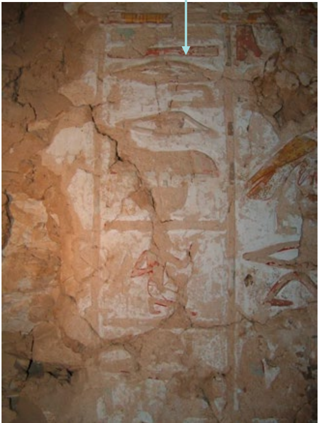
Detail of area of painted plaster on north wall of pillared chamber (C). Note paint loss and cracking in plaster layer.
