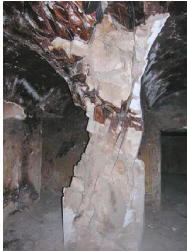
East face of pillar III showing post-fire loss and almost vertical fractures in the remaining rock.
