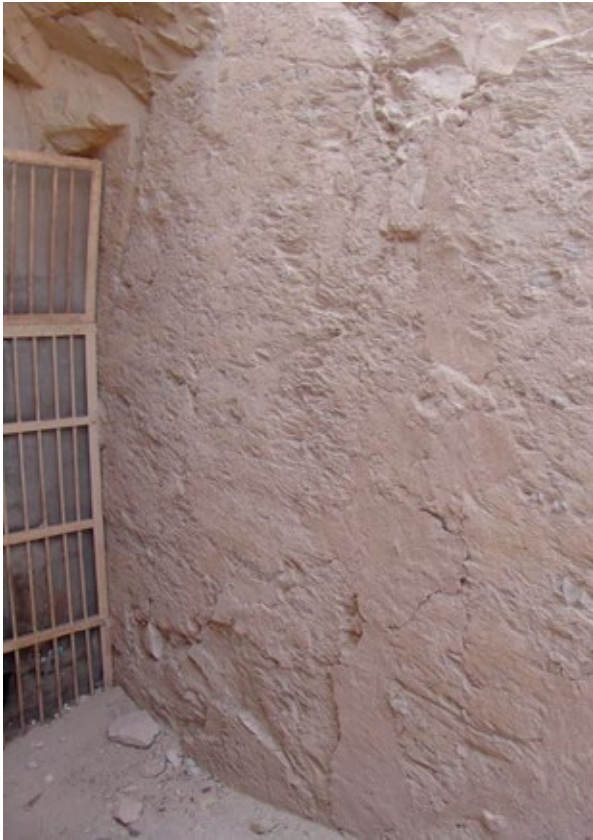
Walls of entry ramp (A) were very finely worked creating a flat, even wall surface. A thin layer of original plaster survives on this wall.
