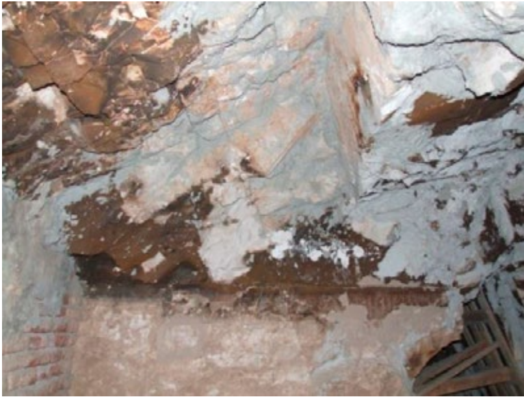
Ceiling of main chamber (C). Note significant amount of post-fire loss. White and gray modern repair plasters are possibly gypsum and cement based.
