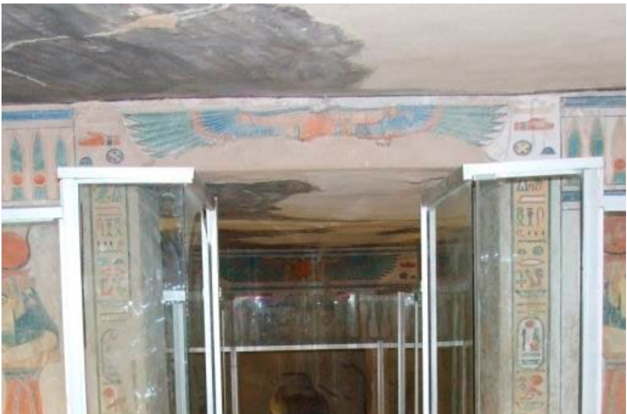
Lintel at doorway (F) is unprotected.
