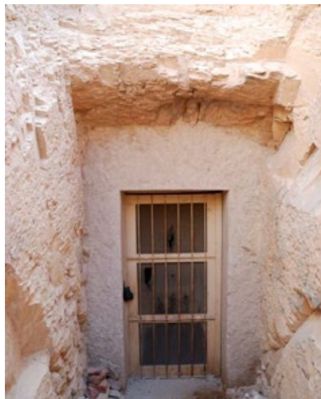
Tomb entrance in 1973 (Image: CEDAE) showing modern ramp walls. The masonry walls were constructed on top of rock-cut wall of the ramp.
