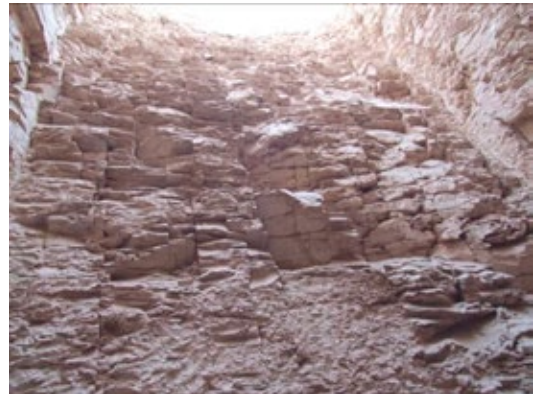
View of shaft from below. Note areas of friable rock.
