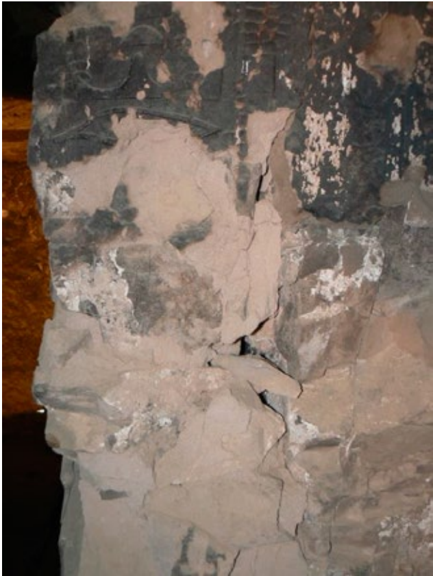
Rock shards were used to construct doorway (H).
