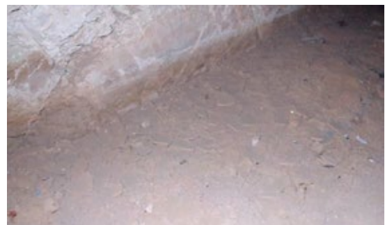
Cracked mud layer on floor with basal staining of wall.
