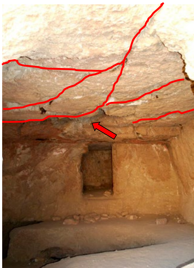
Outer chamber of Chapel F, with red lines indicating locations of structural cracks in the ceiling, and arrow indicating area of substantial rock loss.
