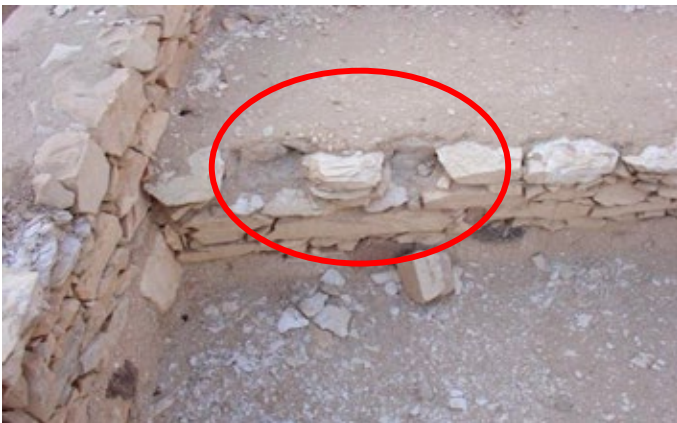
Damage to House 2 where limestone blocks have been displaced from the mortar in which they had been imbedded through CNRS restoration work in the late 1980s.
