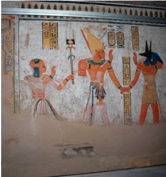
Loss of painted plaster at the wall base of tomb QV 44 (Khaemwaset), presumably due to historic flooding. The tomb is open to general visitation.
