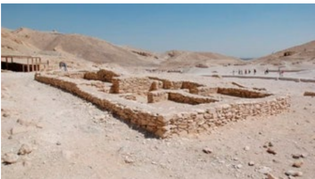
2007 photo of House 1 from northwest.
