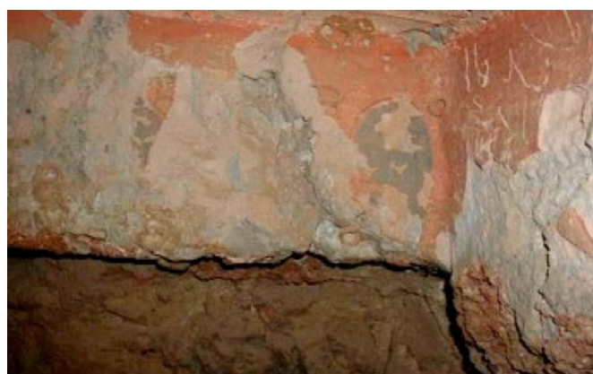
Red painted plaster on the northwest wall of the naos , which has been lost in its lower part.
