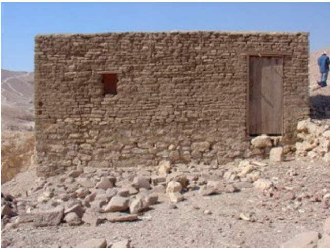
East elevation with door and window.
