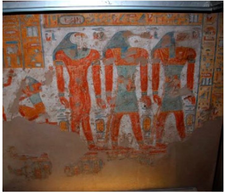
Loss of painted plaster at the wall base of tomb QV 52 (Tyti) presumably due to historic flooding. The tomb, open to general visitation, is in a vulnerable position near the main drainage channel.
