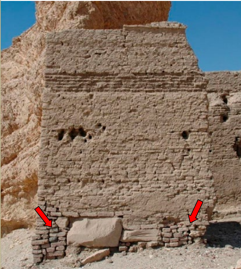
Example of infill of lost foundation stones at wall base with loose fired bricks.
