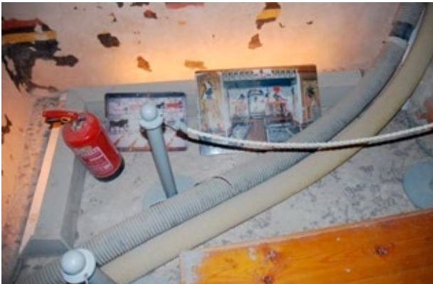
Fire extinguisher and air extraction pipes in upper chamber. Contact of pipes with wall causes abrasion.
