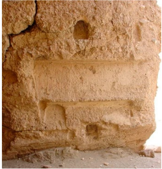
Western wall of Chapel G, which has been extensively damaged by graffiti.
