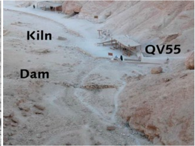
View from upstream side of Dam within context of drainage channel and in relation to QV 55, the adjacent visitor path, and the kiln.
