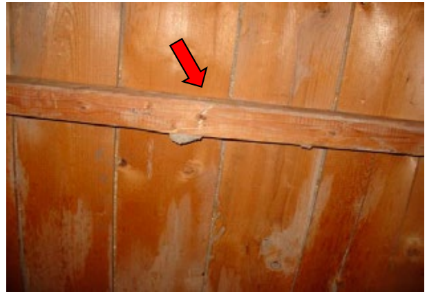
Crack in the middle of the beam supporting the roof in the southeast room. The roof sags in this area.
