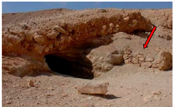
A similar view of QV 1 in 2006 showing loss of stones in the upper part of the masonry wall (indicated by arrow) and around the shelter's opening.
