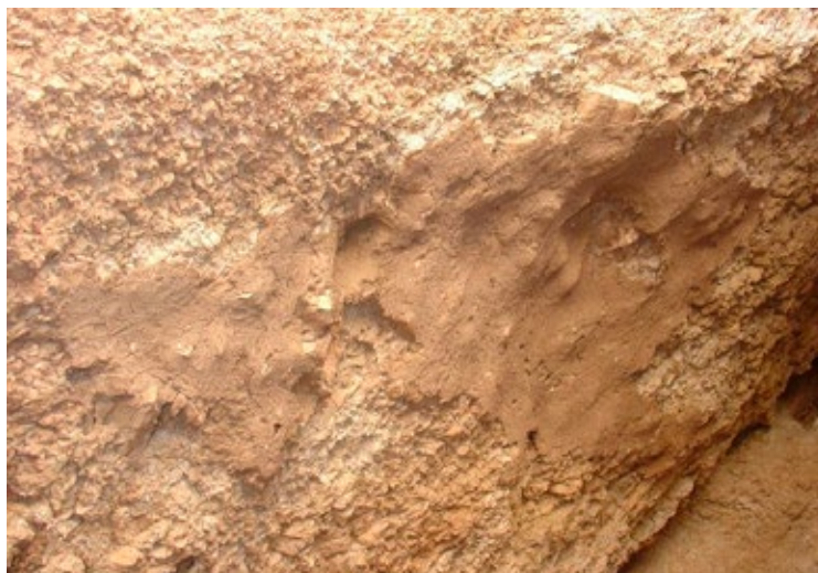
Earthen plaster within QV 1.
