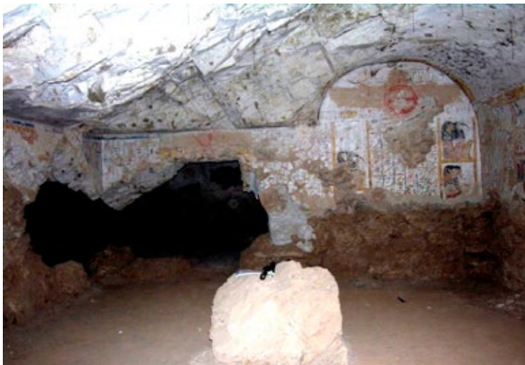
Rock collapse, deterioration, and loss of painted plaster in the lower walls of tomb QV 60 (Nebettau) due to repeated flooding, including in 1994.
