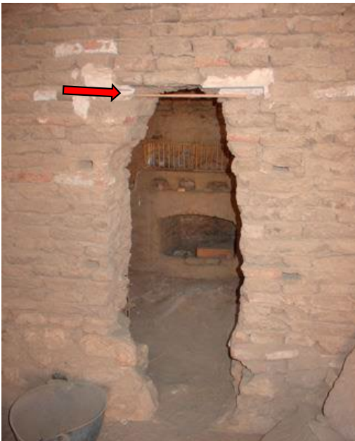
View of missing lintel (arrow) in doorway between the northeast room and the west room.
