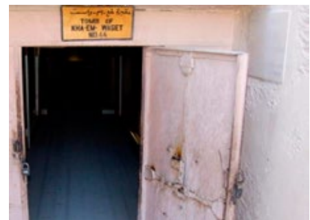
QV 44 modern sign above door and Schiaparelli plaque in wall to right
