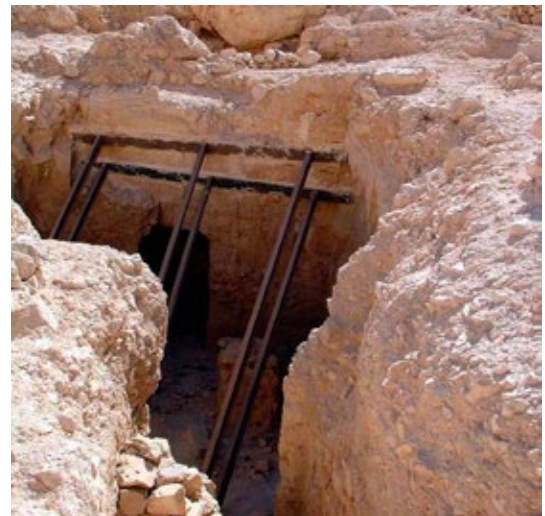
View of roof collapse of tomb QV 34, which is in an area where most tombs contain shale susceptible to water damage.
