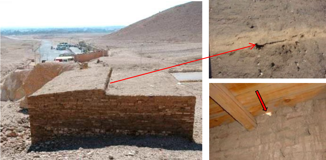
Left: North elevation with site entrance and parking area in background. Upper right: Detail of the hole in the building's roof at the juncture between the two levels. Lower right: Interior view of the hole in roof (arrow), with mud drip lines below providing evidence of water infiltration.
