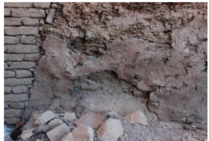
Hermit Shelter 3. Detail view (2007) of exposed mud plaster on the wall of shelter.
