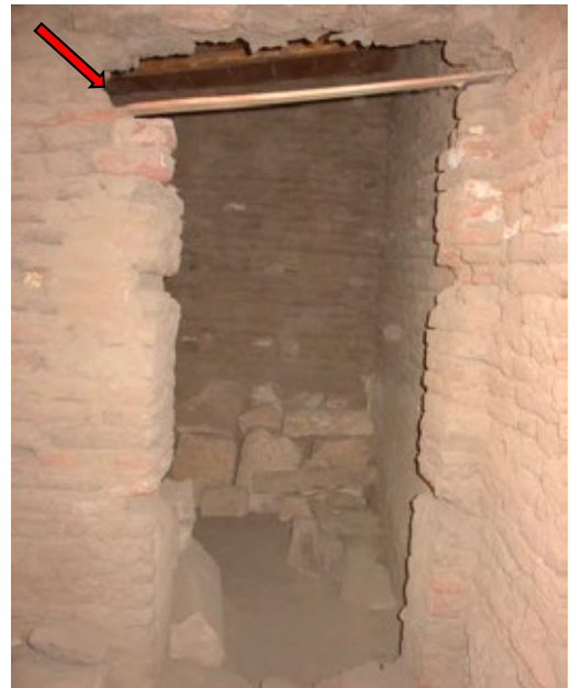
View of missing lintel (arrow) and bricks above it in doorway between the northwest and northeast rooms.
