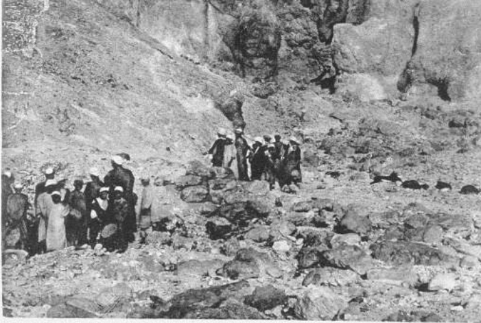
Area of the Dam in the early 20 th century showing workmen of the Schiaparelli mission (Schiaparelli ca. 1903 - 1905). (Image: Schiaparelli 1923)
