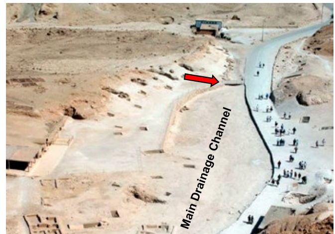
View of main drainage channel looking downstream showing channel narrowing and point of constriction at bridge (arrow).
