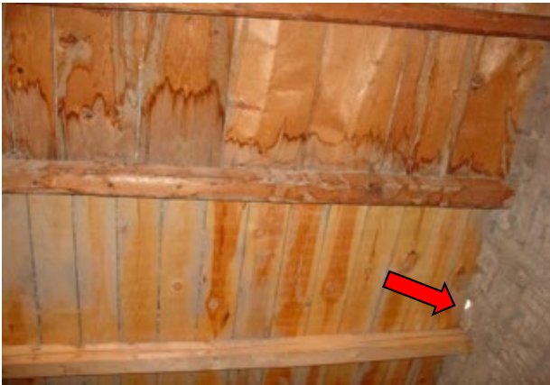
Interior view of water stains on the wooden ceiling adjacent to the hole in the roof (arrow).
