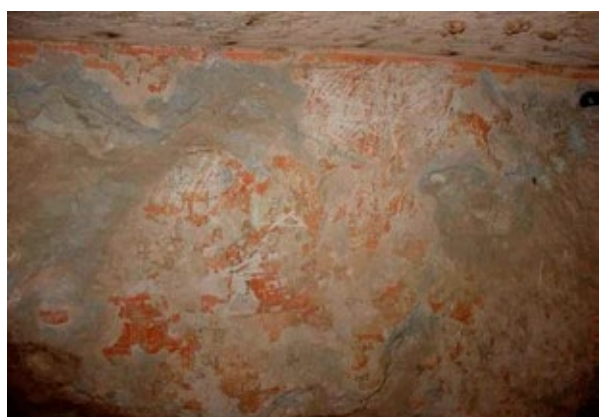
Area of red painted plaster on the west wall of the naos that is substantially degraded, in areas by scratching.
