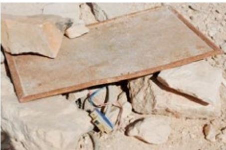
Junction box for electrical cables
