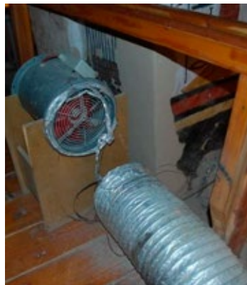
Broken extraction pipe at top of stairs.
