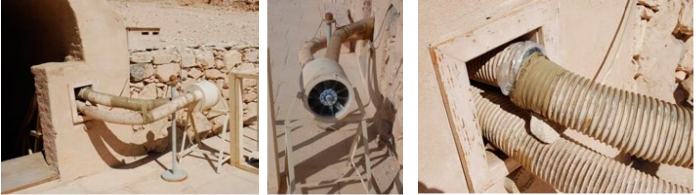
Air extraction pump outside entry to tomb. The pipe exits at the front of the tomb and is a significant visual intrusion. Extraction pipe was broken in several places, occasionally repaired with tape.
