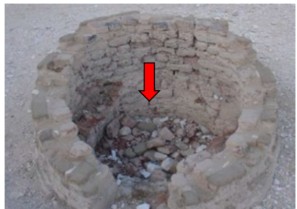
Kiln in 2008. Note bricks that have fallen within the Kiln's interior (arrow).
