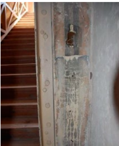
Screen over vent holes is torn and sand-clogged. Door is left open during visitation allowing air-borne particulates to enter tomb.
