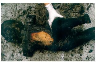
High temperatures during the fire damaged the relief of the four evangelists that decorates the shells of the main cupola. This image shows St. Mark on the left and a charred angel on the right.
