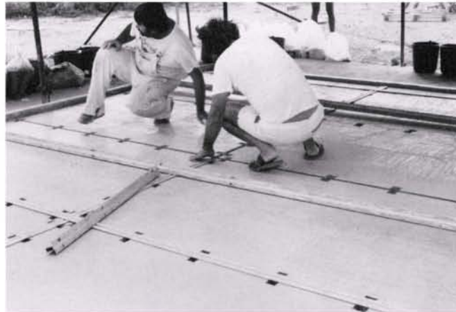
Figure 30 (below right). Roughening the surface of one of the panels.
