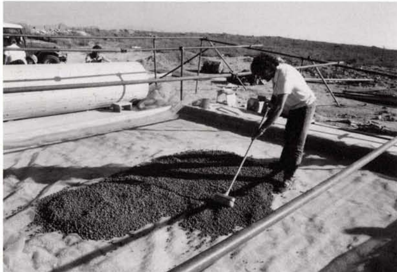
Figure 25 (below right). Structure of scaffolding poles constructed over the mosaic for additional security.
