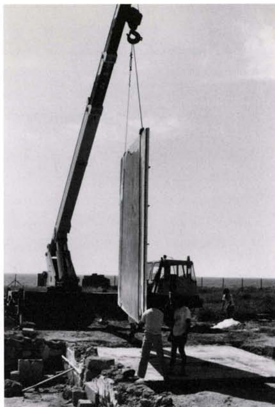
Figure 34. The mosaic, with its new support, being lowered onto its original site.
