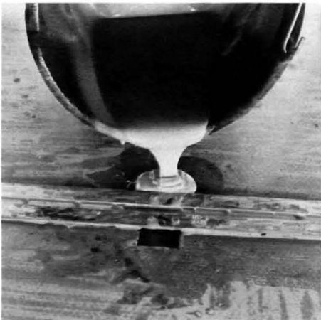
Figure 31 (above). Pouring epoxy into the inserts in the panels.
