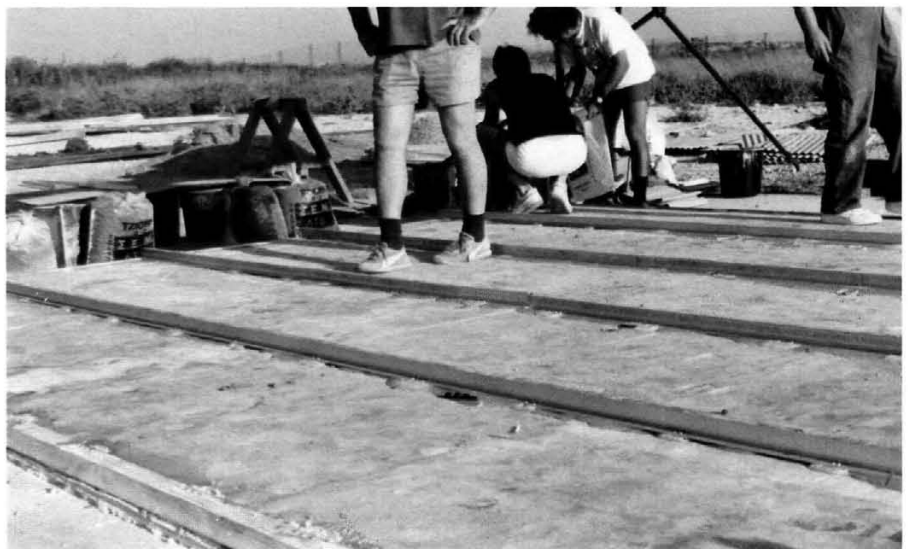
Figure 31 (above). Pouring epoxy into the inserts in the panels.
