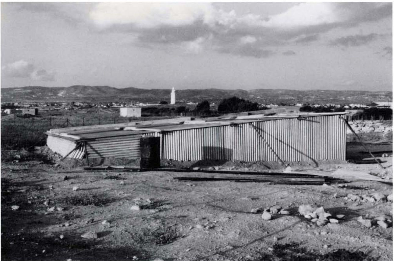
Figure 21. Temporary shelter over the Orpheus mosaic.
