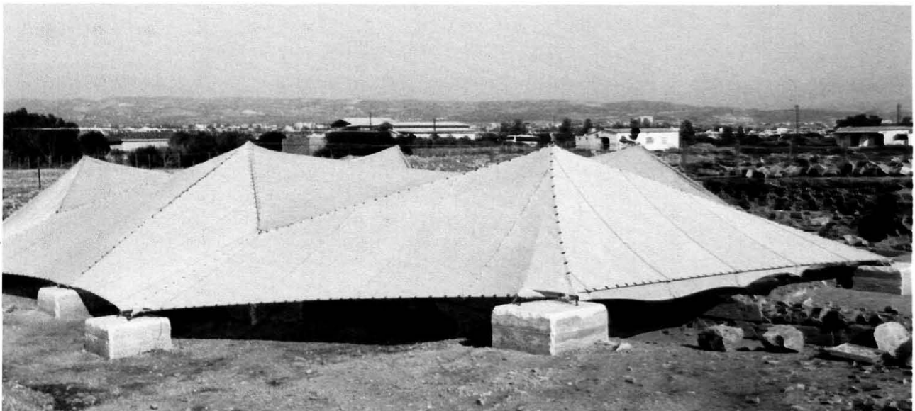
Figure 42. The hexashelter in November 1990 with a new roof membrane and more extensive, overlapping side panels.
