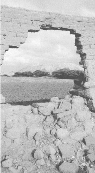
Figure 6 Deterioration and loss of construction materials in the perimeter wall. Photo by Carolina Castellanos.
