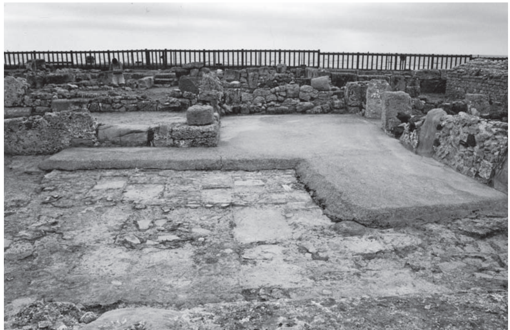
FIGURE 2 The protective contact covering of lime-cement mortar completely isolates the surfaces from contact with the environment. Courtesy Centro di Conservazione Archeologica-Rome (CCA).
