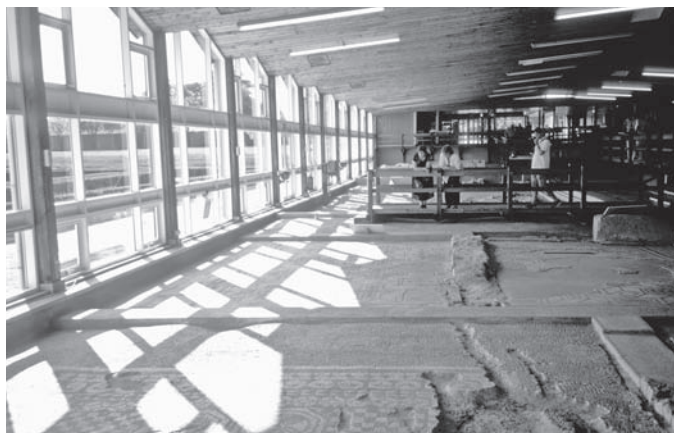
FIGURE 3 Fishbourne Roman Palace. Extensive glazing in the shelter’s original design contributed to major solar gain on adjacent mosaics and high internal temperatures. Photo: John Stewart.
