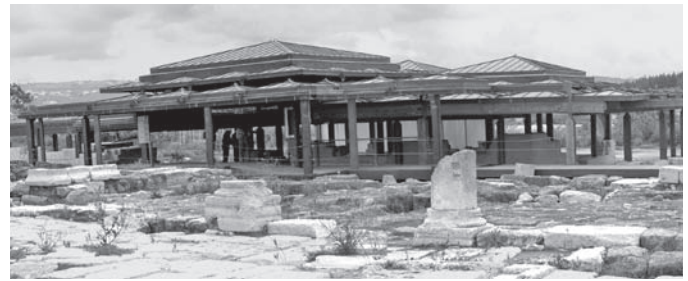
FIGURE 4 The Nile Festival shelter is a complex system of pitched roofs made of fiberboard and copper that rest on a metal-and-timber frame structure. A series of faults in the design and during its construction impaired its protective efficacy. Photo by Y. Alef (2002) © IAA.
