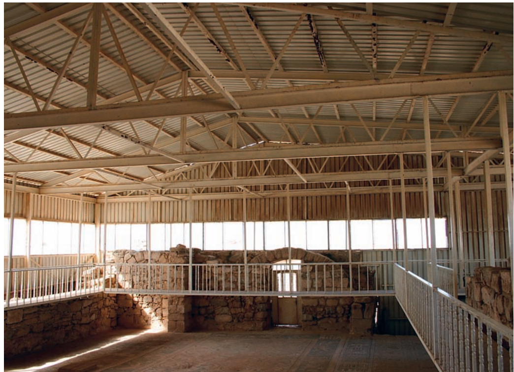
FIGURE 4 The interior of the existing shelter. Photo by Mervat Ma'moun Ha'obsh.
