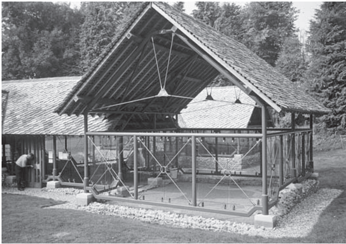
FIGURE 7 Dorchester Roman Town House (1996–99). Steel structural frame with open gables and glass sheets below. Photo: John Stewart.
