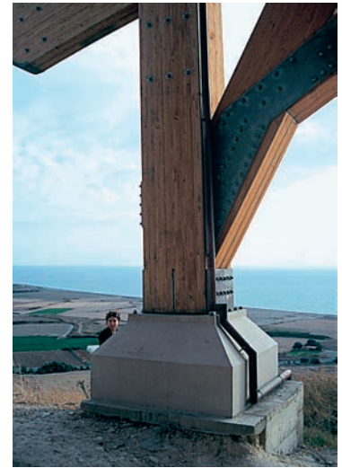
FIGURE 6 The current shelter of the Annex of Eustolios. (Photo by X. Michael 2005)
