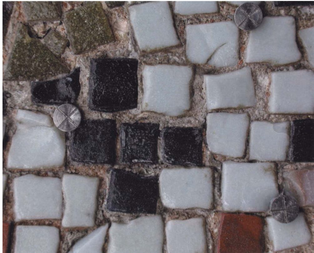
FIGURE 6 Close-up of sector showing position for tripod's leg. Photo: M. Martan.
