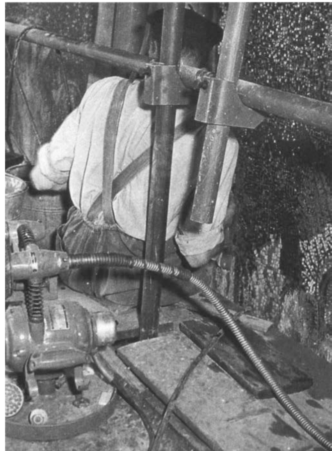
FIGURE 3 (BELOW) The corrosion was removed using wire brushes mounted on an electric motor-driven flexible shaft.
