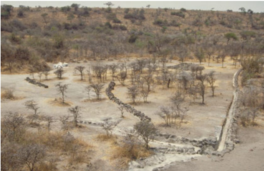
1996. Site-wide drainage was implemented to direct rainfall away from the trackway to the gully north of the site.
