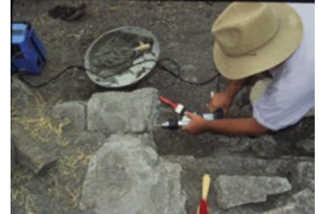
Re-attachment of four collapsed blocks, from left: fallen blocks placed on ledge near where they were found; placement of blocks in original position; re-attachment using fiberglass geo-rods and epoxy adhesive.
