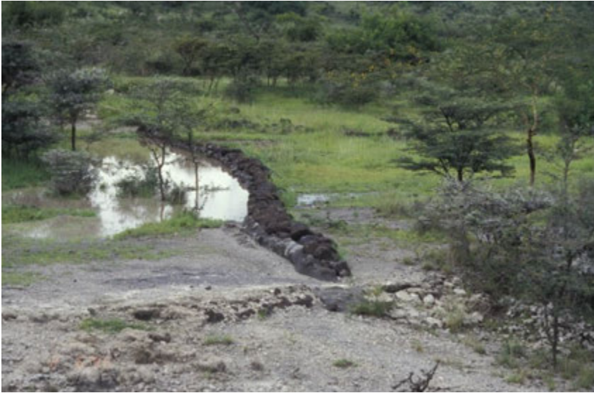
1996. Accumulation of water behind berm in rainy season, prior to completion of drainage plan.
