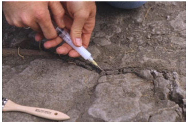
1996. Close-up of consolidation of tuff where disrupted by acacia root penetration.
