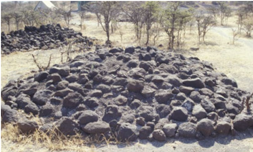
1995. Monitoring trench completed with boulder capping.
