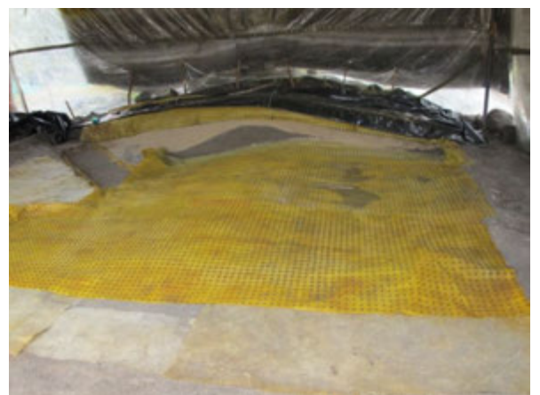
Biobarrier 1 completed.
