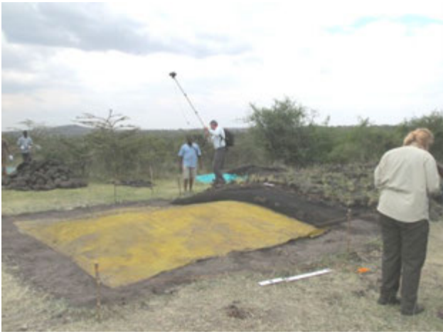
Biobarrier 1 after removal of Layer 4
