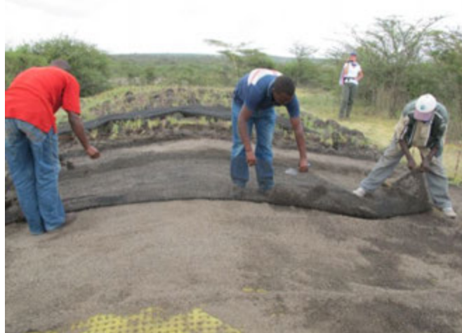
Removal of Enkamat. Biobarrier 1 is beginning to appear in foreground.
