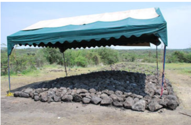
Boulder capping re-instated (temporary shelter still in place).
