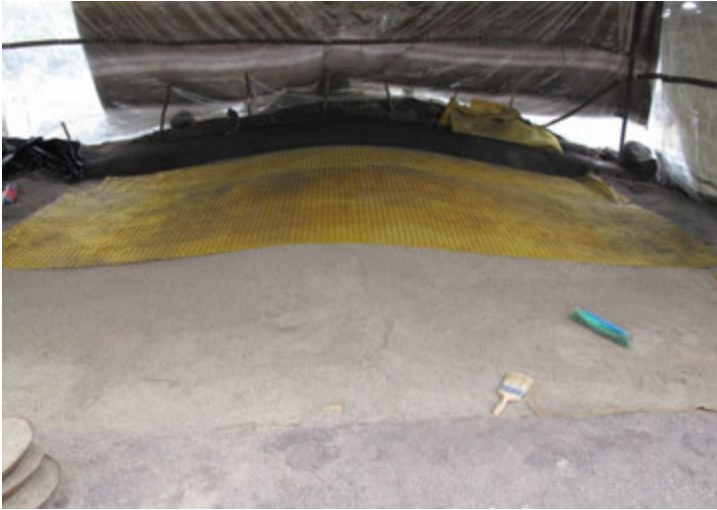
Layer 3 in place with Biobarrier 2 being placed over it.
