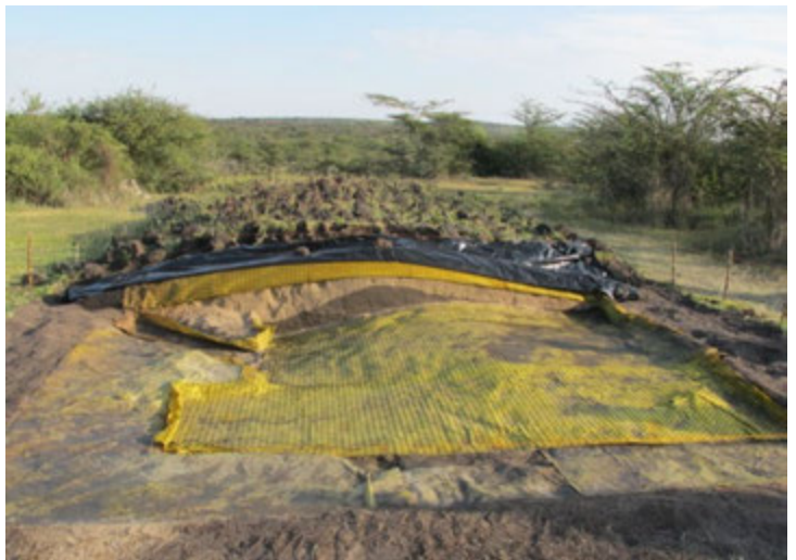
Biobarrier 2 after removal of Layer 3
