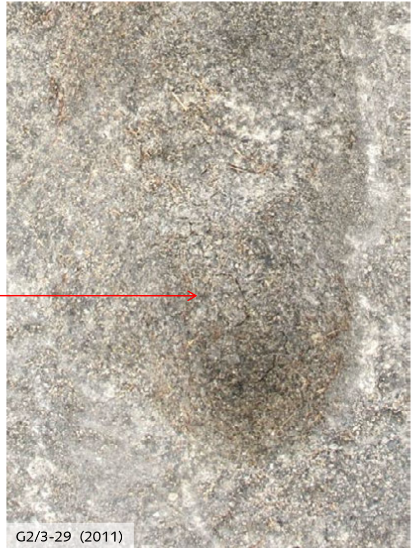
Close-up of heel of G2/3-29 in 1995 and 2011 showing incipient cracking in heel in 1995 slightly enlarged in 2011
