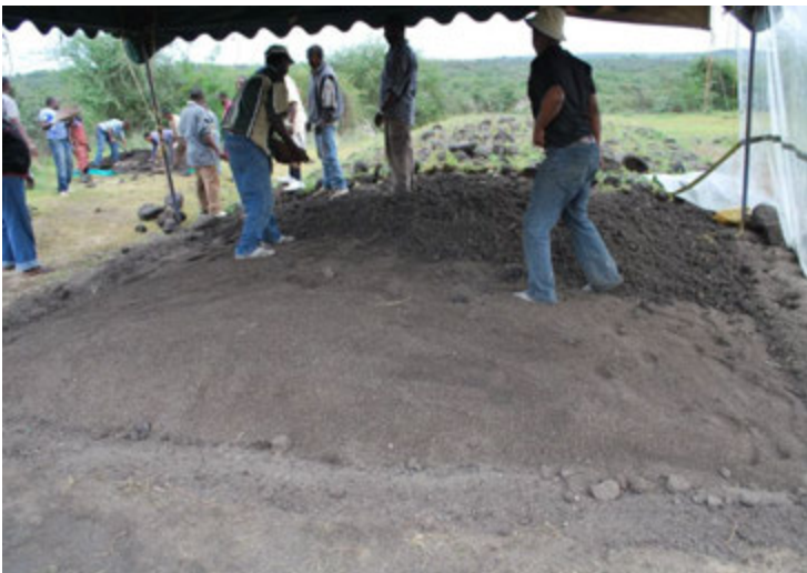
Layer 4 and Enkamat in place with Layer 5 being placed over it.
