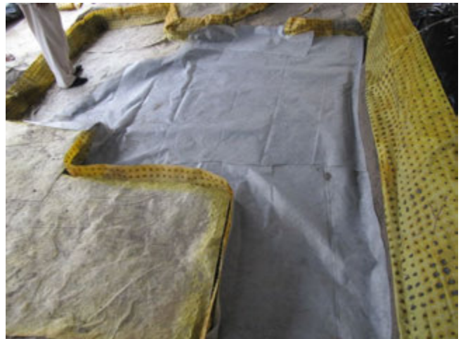
Geotextile in place over Layer 1.
