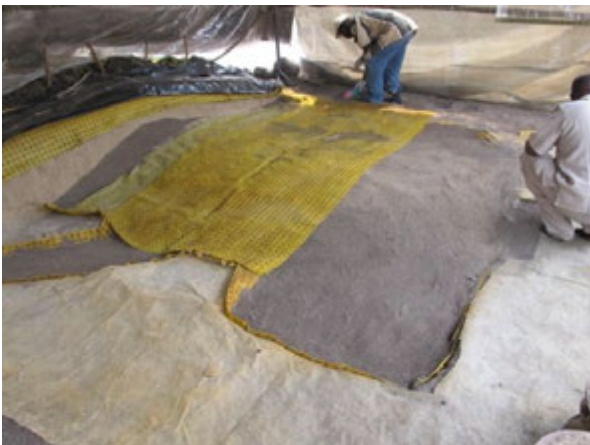
Layer 2 in place with strips of Biobarrier 1 being placed over it.
