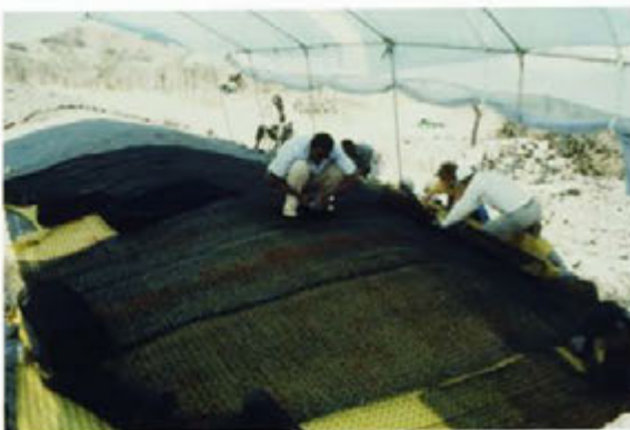
60. Securing strips of Enkamat over Biobarrier, prior to placing Layer 4.
