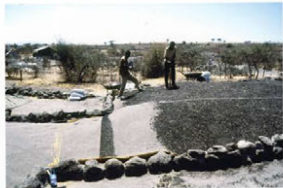
59. Tamping Layer 5 (cotton black soil); looking east.
