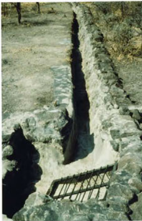
46. Sump with grate and drainage channel associated with Berm 4, looking west.
