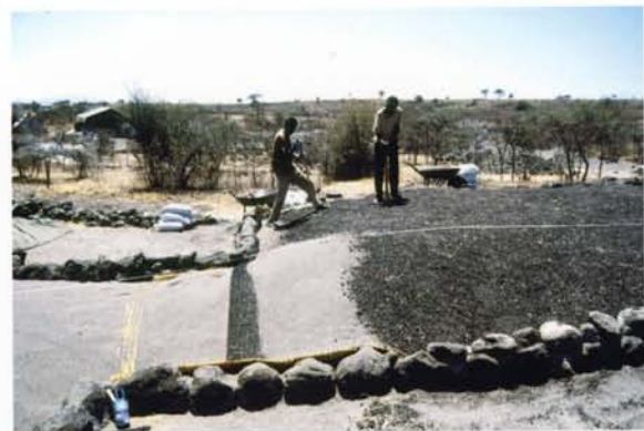
59. Tamping Layer 5 (cotton black soil); looking east.
