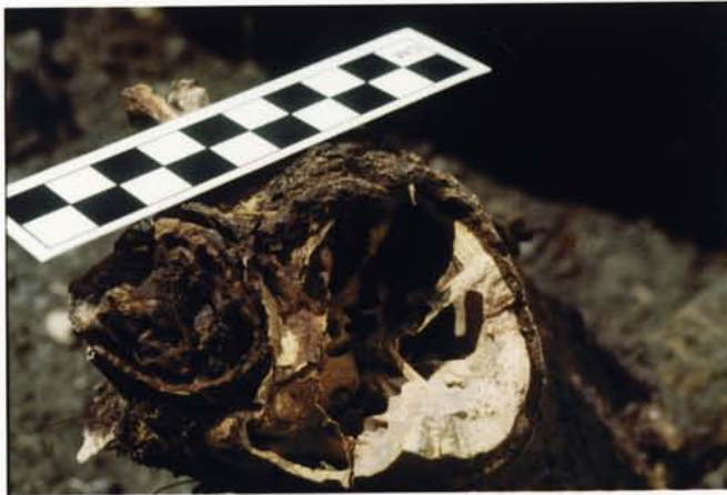
42. Stump killed with herbicide but not treated with PCP, showing evidence of termite galleries and rot.
