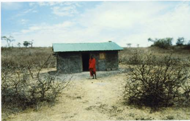
63. Site guard house on slope of the hill south of the site.
