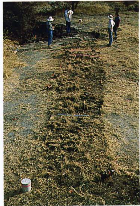
7. Northern and middle sectors of trackway after initial clearing of vegetation and removal of boulders; looking north.
