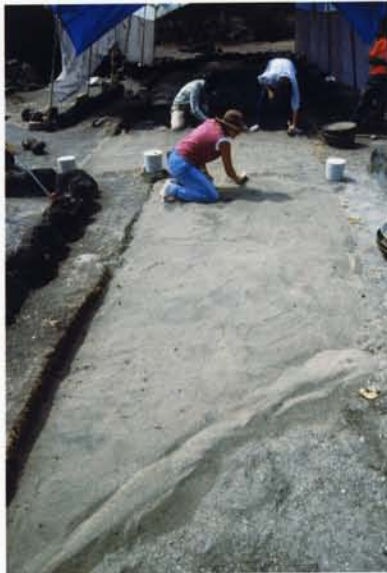
56. Placing the first layer of sand on the middle trackway sector.
