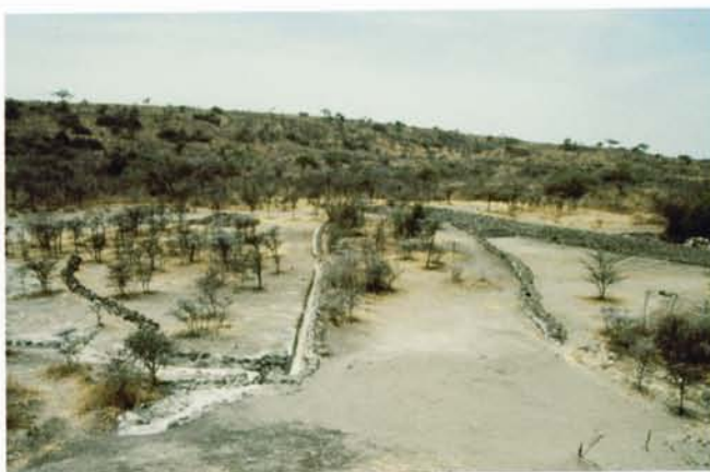
47. Site drainage control after completion: Berm 4 is in the center with Berm 2 on the left and Berm 3 on the right; looking west.
