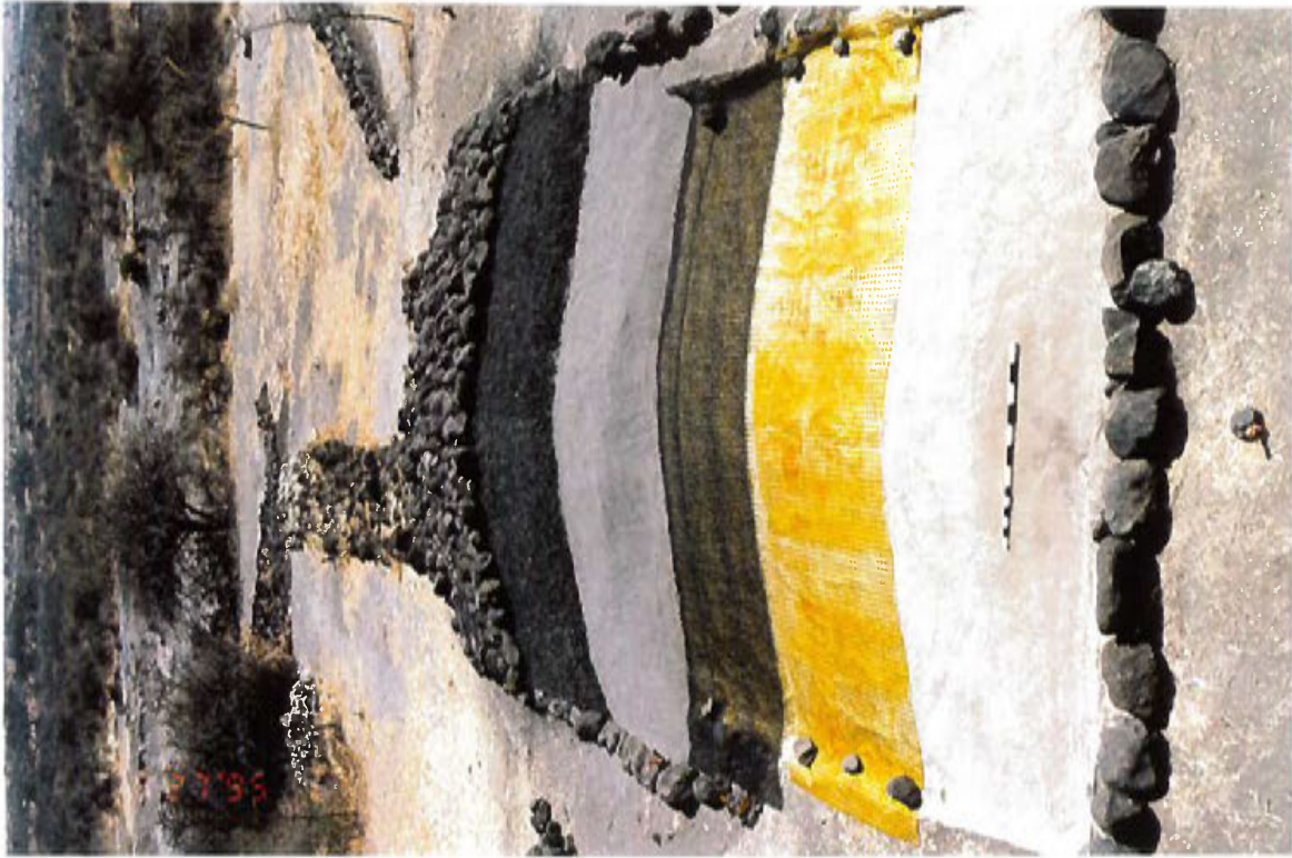
7. Profile of the layers of the reburial mound over the southern trackway. From the south (bottom of photo): Layer 3 (Kakesio sand is visible), 2nd layer of BiobARRIER , Enkamat, Layer 4, Layer 5, boulder capping.
