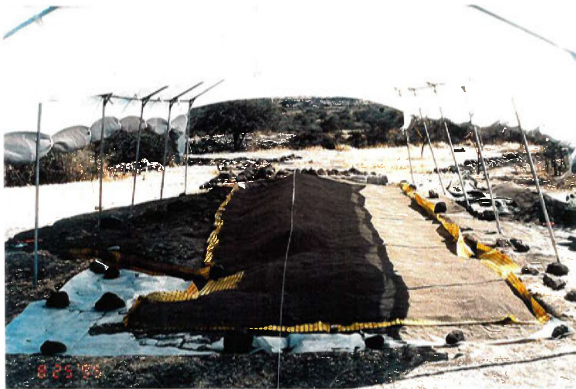
35. Middle stages of the reburial showing upturned edges of 1st layer of Bio barrier partially covered by Layer 3. Layer 3 is in progress: the center of the mound is being established along tape line and geotextile over the 1979 land surface in foreground is not yet covered.
