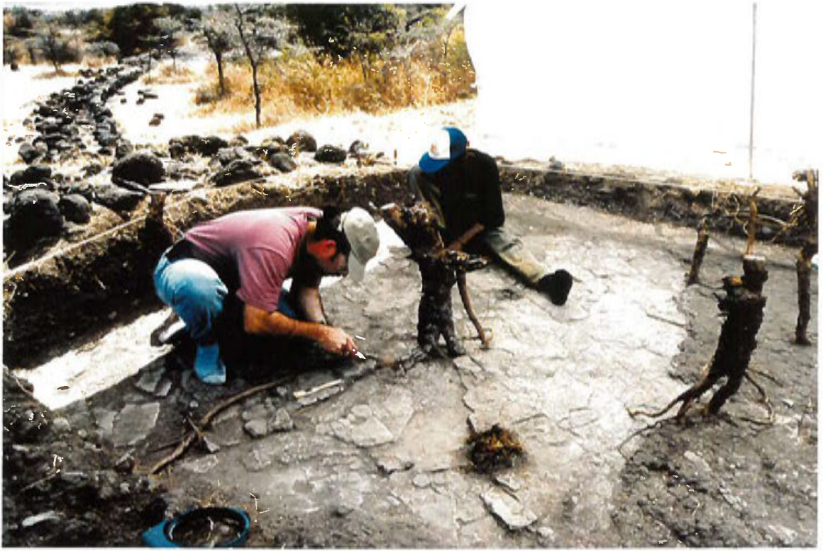
19. Consolidation of tuff disrupted by a lateral root from stump #27, in preparation for its partial removal.
