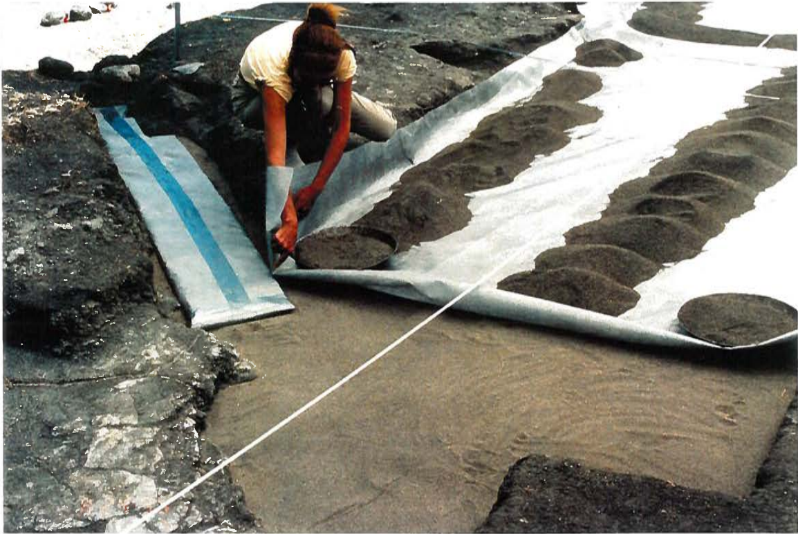
34. Early stage of the reburial showing Layer 1 in place, placement of geotextile above Layer 1 with small mounds of Layer 2 to hold it in place, and geodrain in the 1979 west trench.
