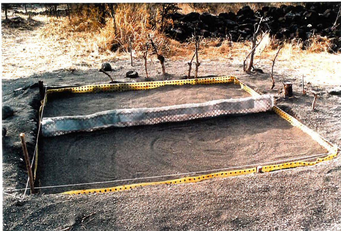
37. Test Site 3. Partial reburial of monitoring trench showing vertical placement of Biobarrier on trench walls, Layer 2 and separator barrier between north and south sections of the trench.
