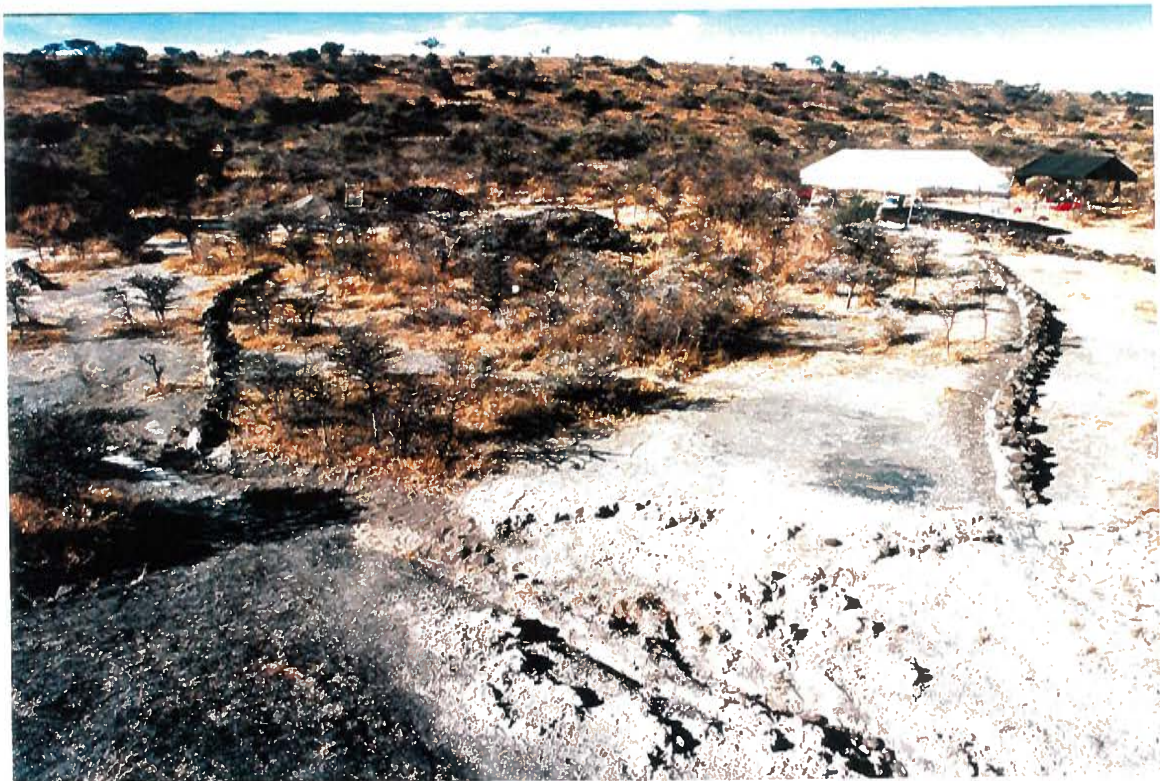
29. Berm 2 (left, center) and newly constructed Berm 3 (right, center). At lower center is the debouchment of Drainage Channel 2.
