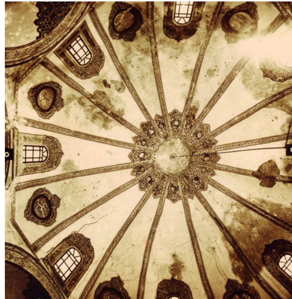
A pair of stereographs of the dome, taken looking straight up. Note the large number of cracks. Photo: A. Alkiş © Küçük Ayasofya Project.
