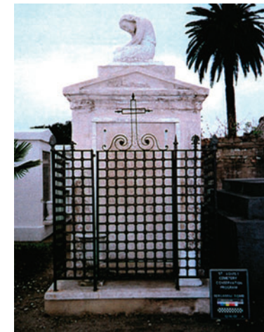
The Bergamini tomb, after restoration. The masonry and associated stone and metalwork were stabilized and conserved. Photo: Frank Matero © University of Pennsylvania Architectural Conservation Laboratory.
