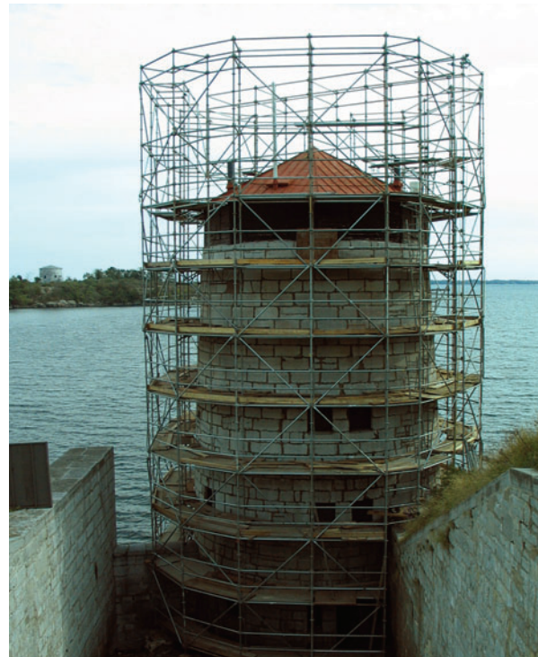
The scaffolded East Branch ditch tower during the restoration project. Photo: © Fort Henry National Historic Site of Canada—Archives.
