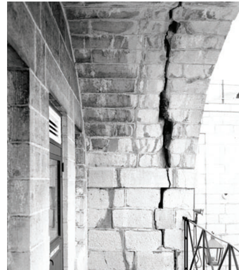
Fractures and spalling of the limestone blocks in an archway of the redoubt. The mortar joints had also deteriorated significantly. Photo: © Fort Henry National Historic Site of Canada—Archives.
