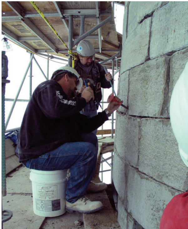
Workers removing deteriorated mortar from the East Branch ditch tower for repointing. Photo: © Fort Henry National Historic Site of Canada—Archives.
