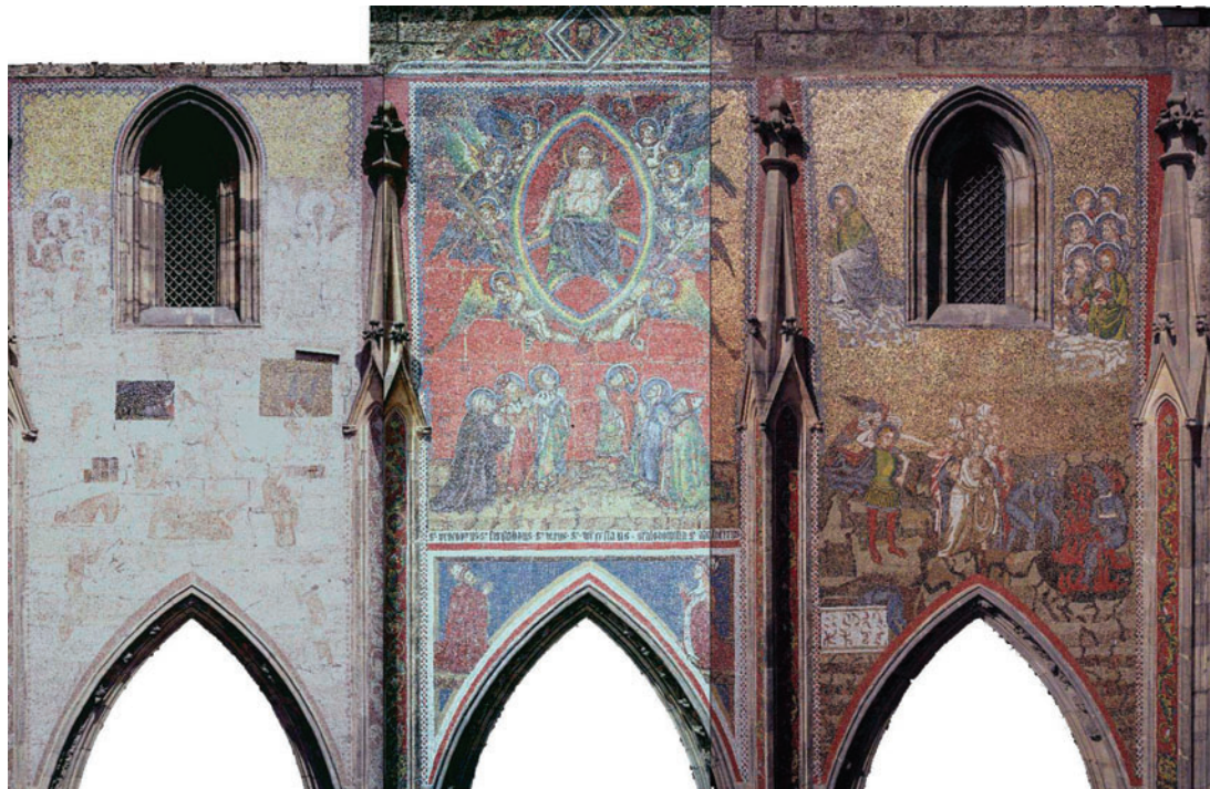
Rectified images of the facade, showing its state before conservation ( left ), after treatment ( center ), and after gilding ( right ). Images: Jaroslav Zastoupil.
