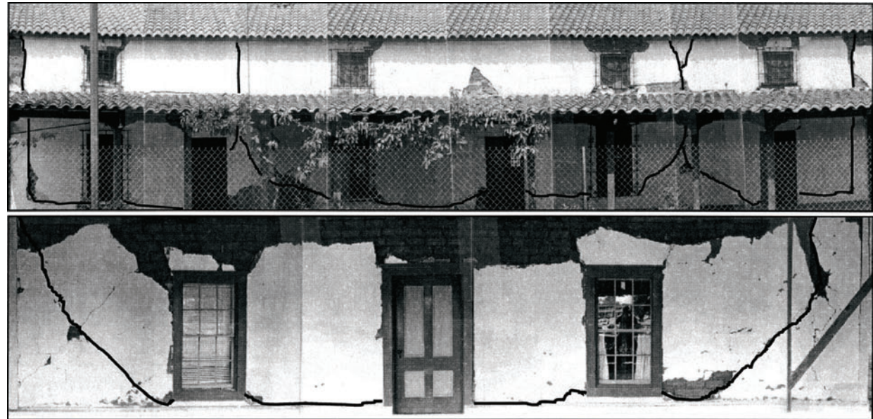
East exterior elevations of the Andres Pico Adobe, after initial structural assessment. Structural failures such as cracks caused by out-of-plane flexure were sketched on top of 35mm film and Polaroid images that were taken perpendicular to the building. This type of on-site assessment allowed engineers and architects to compile the final synthesis analysis and quickly move on to the next building. Photo: E. Leroy Tolles.
