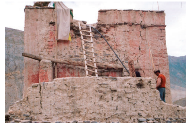
A local worker recording the front elevation of Chango Temple. Manual recording techniques, although labor intensive, are readily available and allow conservators to study buildings in great detail. Photo: © Sandeep Sikka.
