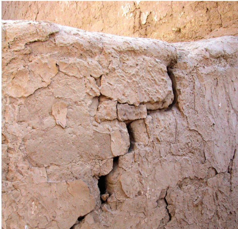
Example of structural damage to the earthen adobe walls of the Tambo complex. Photo: © Alonzo Addison.
