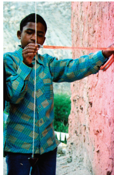
A worker measuring exterior deformation in reference to a vertical plumb line at Chango Temple. Photo: © Sandeep Sikka.
