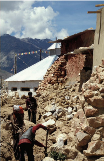
Workers burying perforated drains. Photo: © Sandeep Sikka.
