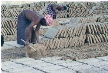
Fig. 26 Workers in Seyoun, Yemen, creating new mud-brick construction. Every step in this traditional building process was recorded on video and screened for the public. Photo: © Caterina Borelli.
