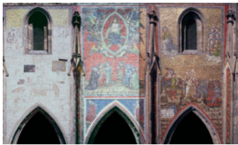
Fig. 16 Rectified images of the Last Judgment mosaic, St. Vitus Cathedral, Prague, showing its state before conservation (left), after treatment (center), and after gilding (right). Recording must accompany each phase of conservation activity. General and detailed photographs before, during, and after treatment are standard procedure in conservation documentation. Photo: Jaroslav Zastoupil, 2002.
