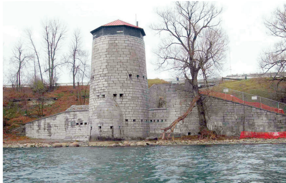
Fig. D.1 The East Branch ditch tower at Fort Henry, overlooking Lake Ontario and the mouth of the St. Lawrence River. Photo: Christian Ouimet © Heritage Conservation Directorate, Canada / Direction de la conservation du patrimoine, Canada.
