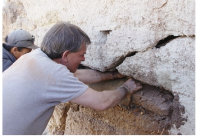
FIGURE 22 Filling the chase.
