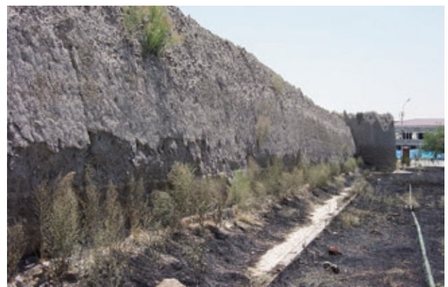
FIGURE 8 City wall with pisé lifts, Armenia. A horizontal turf lift is revealed behind plasters on the lower wall.
