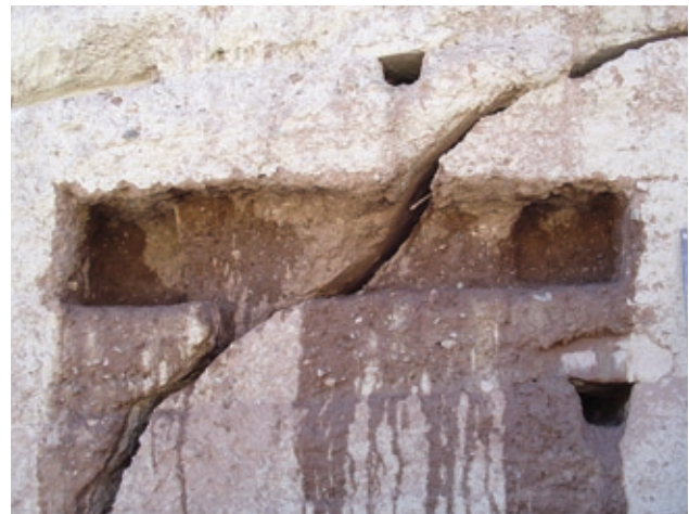
FIGURE 20 Wetting the finished chase.
