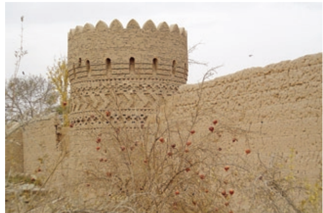
FIGURE 12 Adobe wall with horizontal vegetation mattresses in Yazd, Iran. The tower, which has been rebuilt, has no ring beam.
