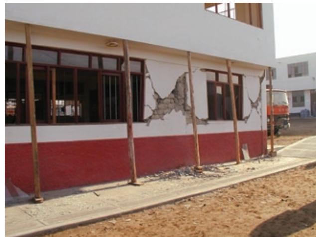
FIGURE 2 Seismic cracks of unreinforced adobe house.
