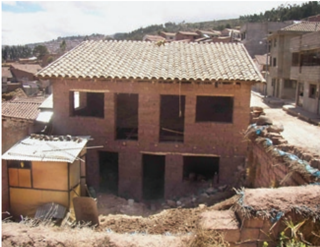
FIGURE 1 Seismically vulnerable adobe house in Peru.
