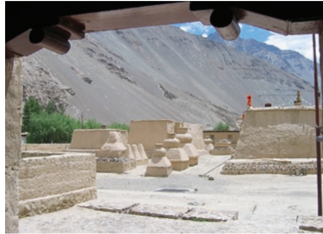
FIGURE 1 The tapered load-bearing adobe walls at a temple in Spiti provide extra stability to the building during seismic vibration.
