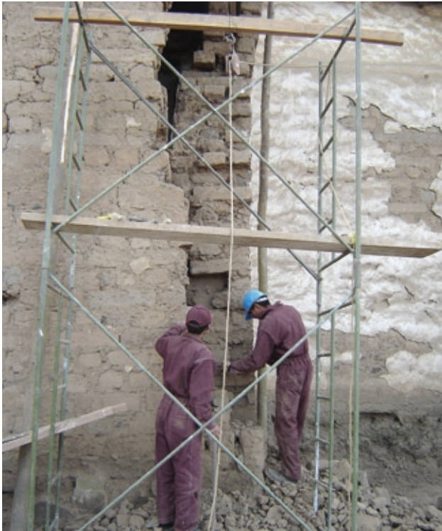
FIGURE 10 Damaged corner in the process of being demolished and rebuilt, San Pedro de Navan.
