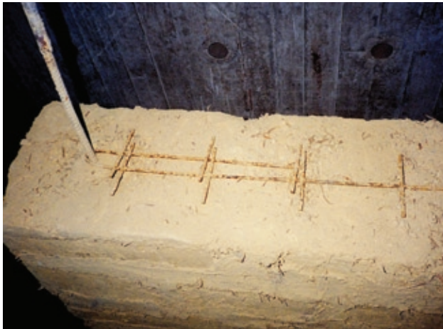
FIGURE 12 Detail of reinforcement, with vertical rods in holes through the adobes and horizontal reinforcement wrapped around the vertical rods. Now geogrid is more typically used for horizontal reinforcement.
