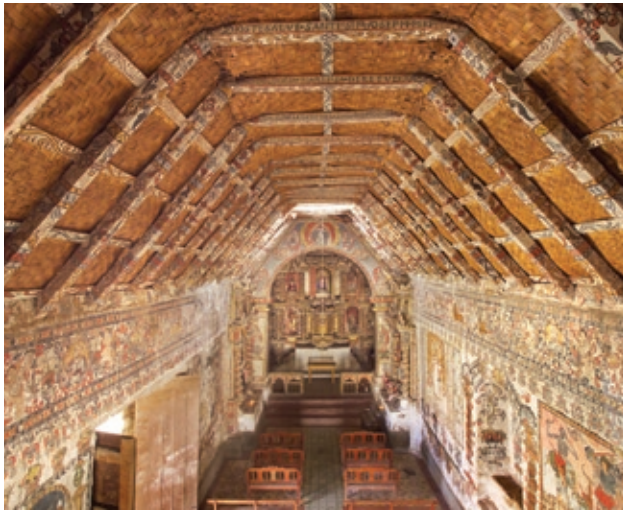
FIGURE 2 Interior of the Rapaz Missionary Chapel showing roof construction. Photo: Daniel Giannoni.
