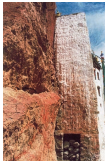
FIGURE 4 Vertical structural crack between buildings and the adjacent hill. This significant detachment was caused by the earthquake.
