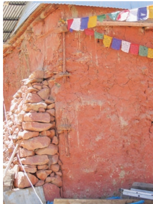
FIGURE 2 The external surface of the temple at Nako village in upper Kinnaur (AD 1025) is fitted with horizontal wooden wall ties and supporting rubble stone buttresses at the corners.
