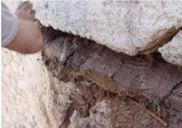
FIGURE 21 Filling the chase with yagtsa and hemp matting.
