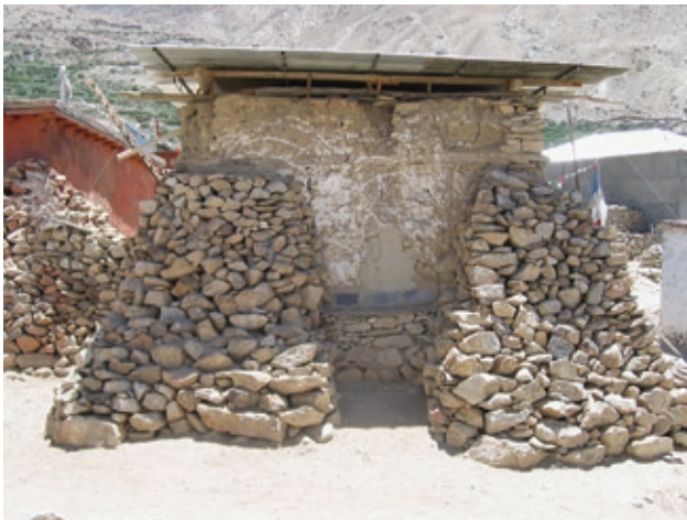
FIGURE 5 Piles of rubble stones stacked against the corners of the buildings after an earthquake in Nako village, to serve as buttresses to halt further outward movement of the masonry walls.
