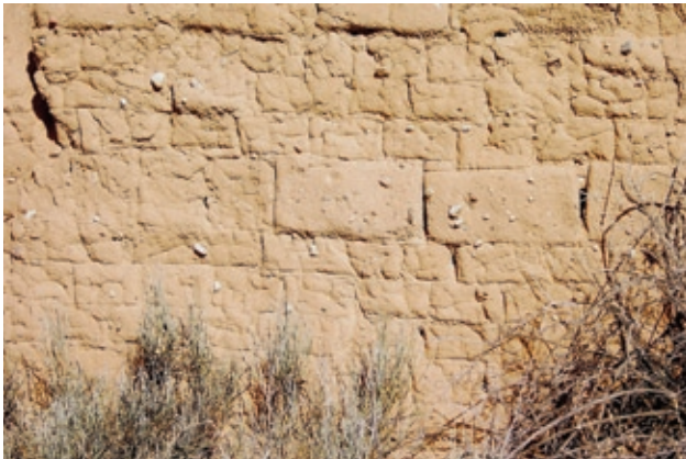
FIGURE 11 Nineteenth-century wall with large-block ring beam, Kyrgyzia. These modern remnants show horizontal changes in block size.
