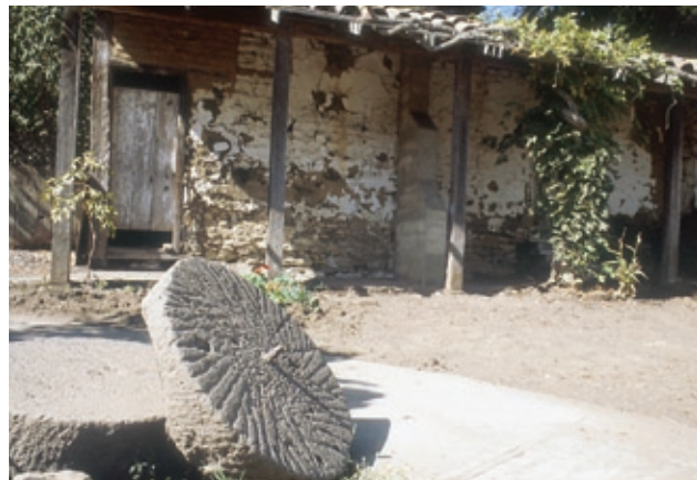
FIGURE 5 Don Jose Antonio Bolcoff Adobe, ca. 1840, Wilder Ranch State Park, near Santa Cruz, California. The Bolcoff Adobe's deteriorated condition is the result of deferred maintenance. Photo: California State Parks, © 1988.
