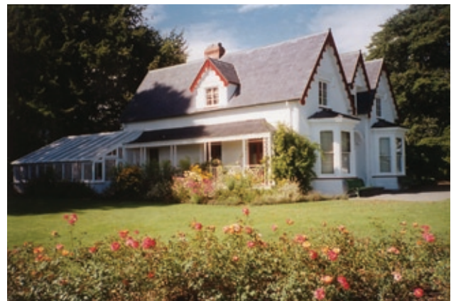
FIGURE 4 Broadgreen House, with lower-story cob walls. Photo: Richard Walker.
