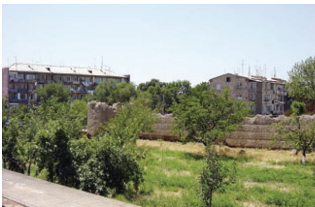
FIGURE 7 Pisé city wall, Yerevan, Armenia. There are regular horizontal lifts, each lift line concealing a turf lift.
