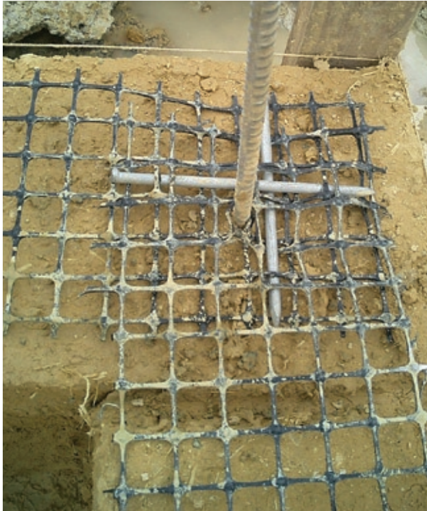
FIGURE 9 Geogrid reinforcement at corner joint. Photo: Richard Walker.
