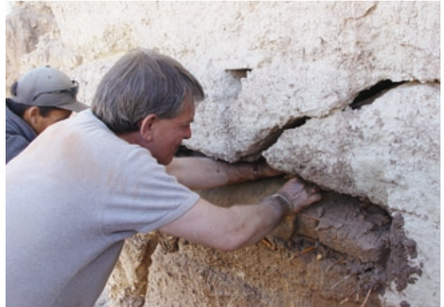
FIGURE 22 Filling the chase.
