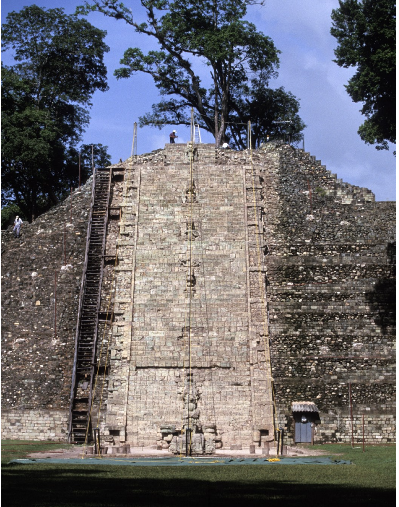
Figure 10 The Hieroglyphic Stairway during the temporary removal of its shelter. July 2003.
