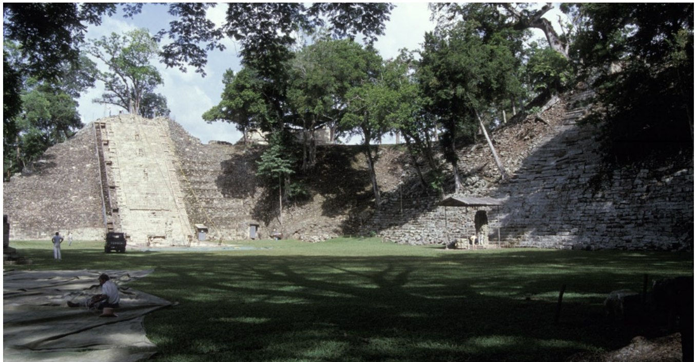
Figure 8 Court of the Hieroglyphic Stairway looking southeast, with Structure 26 and the Stairway, temporarily without its shelter, on the left. July 2003.
