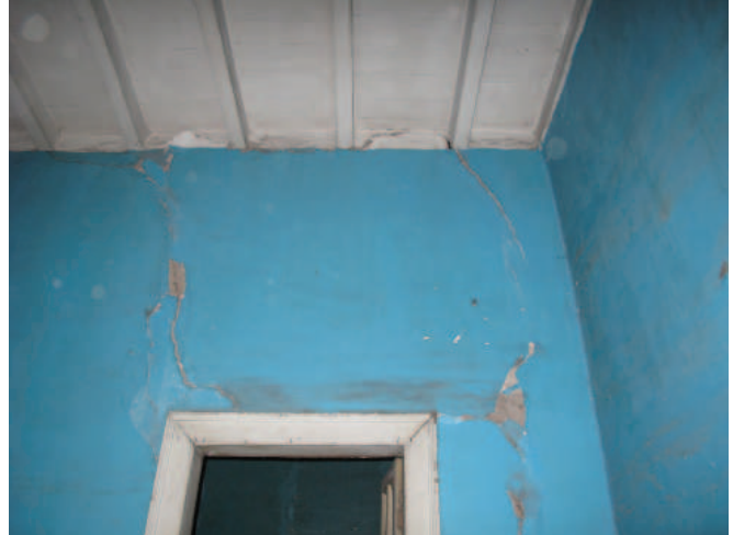
FIGURE 3.49 Typical crack pattern at openings in quincha walls. Image: Claudia Cancino.
