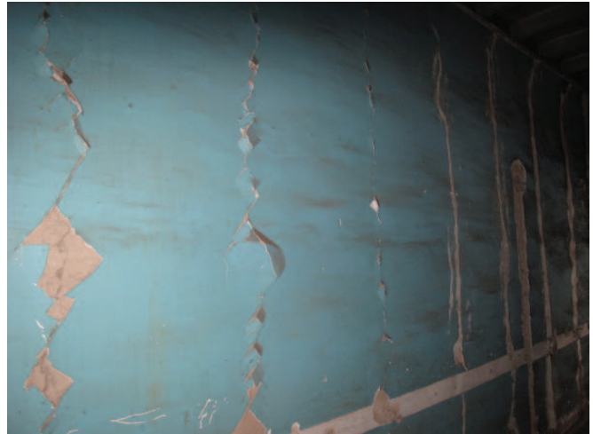
FIGURE 3.51 Vertical cracks corresponding to quincha post locations, southeast wall of corridor 246, sector C. Image: Amila Ferron.
