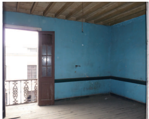
FIGURE 3.17 Typical third floor room (room 306), with doors providing access to the balcony. Image: Mirna Soto, for the GCI.
