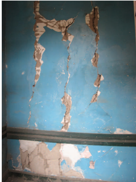
FIGURE 3.50 Typical crack pattern, corresponding to the quincha post locations. Image: Claudia Cancino.
