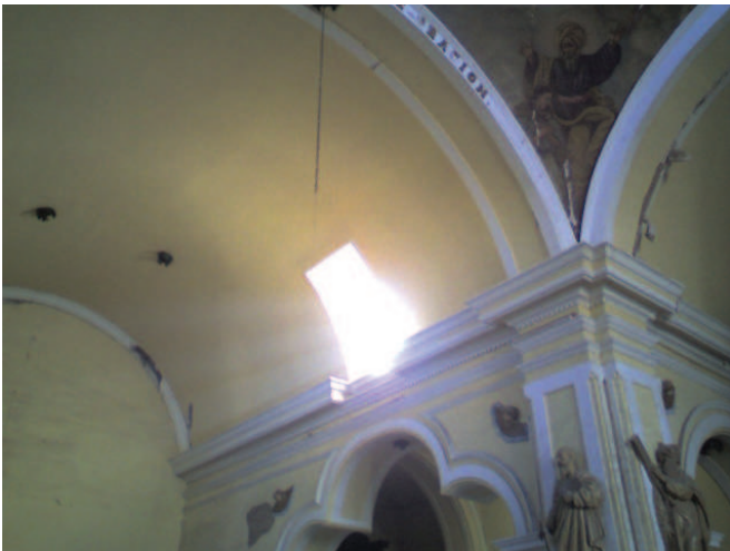
FIGURES 2.22 (LEFT) AND 2.23 (RIGHT) Barrel vault over altar at the Cathedral of Ica: photograph (left) and thermal image (right) of the same sector, indicating the location of the internal wood ribs or arches. Images: Claudia Cancino.
