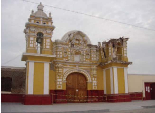
FIGURE 1.3 The earthen Church of El Carmen, Chinchipe, Peru. The bell tower collapsed during the 2007 Pisco earthquake. Image: Philippe Garnier, for the GCI.
