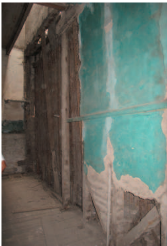
FIGURE 3.52 Northwest wall of room 243. Image: Claudia Cancino.
