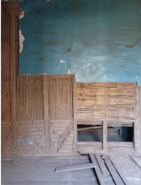
FIGURE 3.25 (ABOVE) Typical quinchá wall at the second floor, showing the mud and fired brick infill at the bottom of the frame (prospection IIS-2). The horizontal canes at the right have been used to infill an earlier door opening. Image: Mirna Soto, for the GCI.
