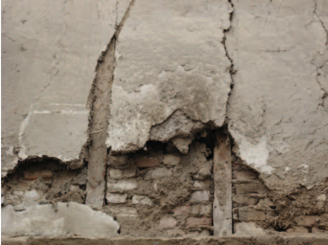
FIGURE 3.48 Typical plaster detachment at quincha wall bases and posts. Image: Claudia Cancino.
