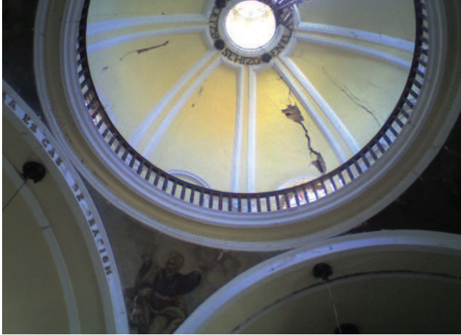
FIGURES 2.20 (LEFT) AND 2.21 (RIGHT) Dome of the Cathedral of Ica: photograph (left) and thermal image (right) of the same sector, indicating the location of the internal wood ribs or arches. Images: Claudia Cancino.
