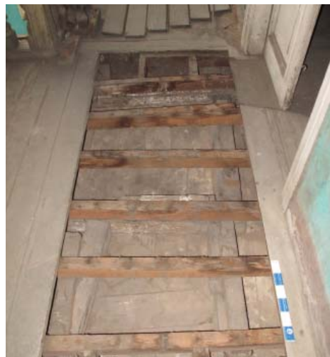
FIGURE 3.36 (FAR RIGHT) Typical finish ceiling at the underside of the floor construction. Image: Amila Ferron.
