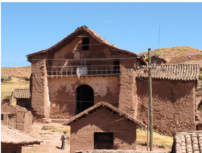
FIGURE 5.6 Primary façade at south side of church, with the baptistery wing to the right. Image: Sara Lardinois.
