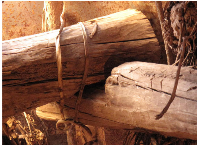
FIGURE 5.29 Half-lap joint at intersection of roof rafters over main church. Image: Claudia Cancino.
