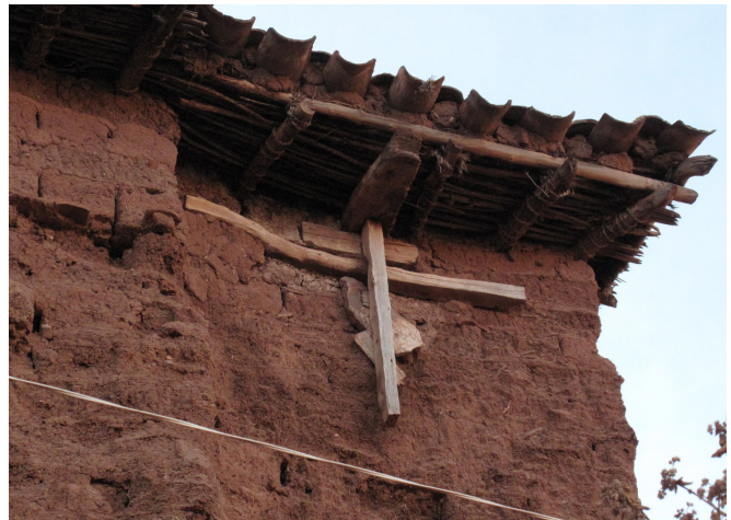
FIGURE 5.43 Wood key at south end of west lateral wall. Image: Claudia Cancino.
