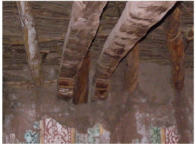
FIGURE 5.32 View of the pair of tie beams over the nave. Image: Mirna Soto, for the GCI.
