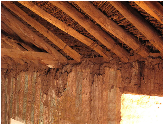
FIGURE 5.31 View of rafters and wall plate at the lateral wall of nave. Image: Claudia Cancino.
