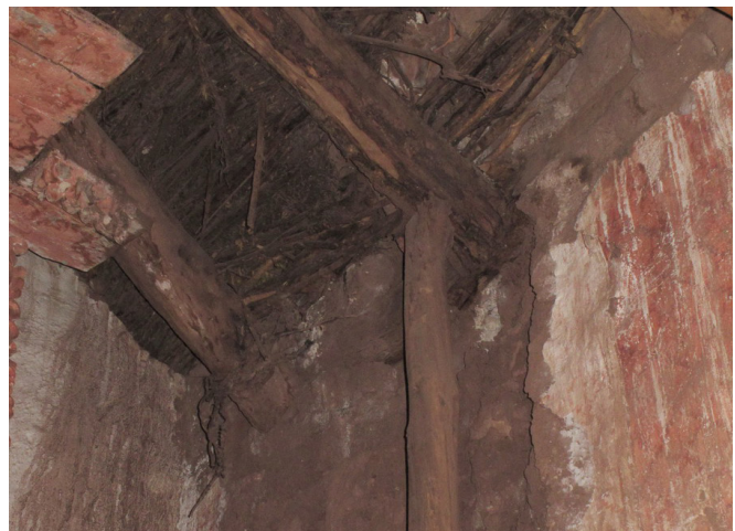
FIGURE 5.42 Erosion at the top of the mud brick wall in the northeast corner of the altar has led to failure of the roof rafter. A wood post has been installed to temporarily support the rafter end. Image: Sara Lardinois.
