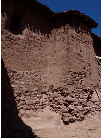
FIGURE 5.12 View of erosion at east side of church. Image: Mirna Soto, for the GCI.
