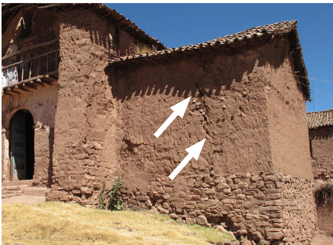
FIGURE 5.41 Crack in the south façade of the baptistery wing. Image: Wilfredo Carazas, for the GCI.
