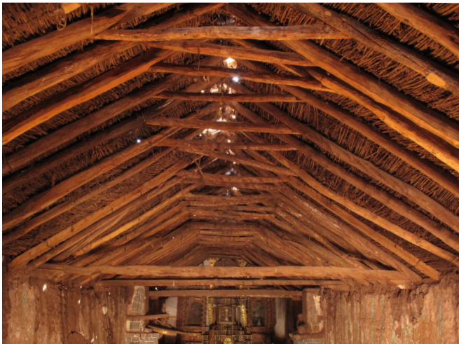
FIGURE 5.28 View of pares y nudillos framing and tie beams over the nave. Image: Claudia Cancino.
