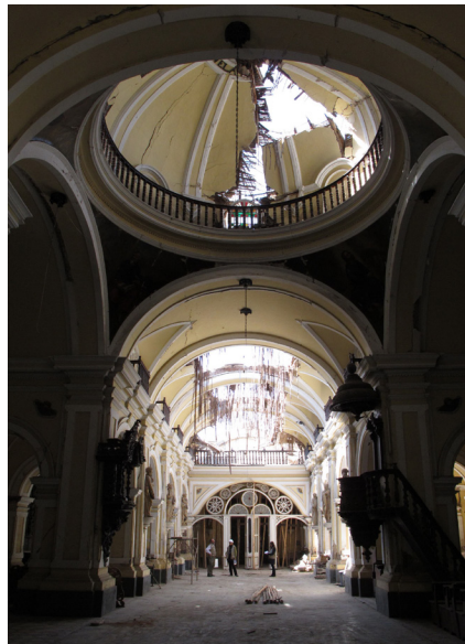
FIGURE 4.57 Sector E: Interior view, looking east, showing the partial collapse of the dome and barrel vault. Image: Sara Lardinois.
