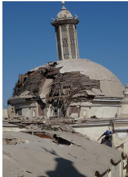
FIGURE 4.56 Sector E: View of partial collapse of quincha dome. Image: Mirna Soto, for the GCI.
