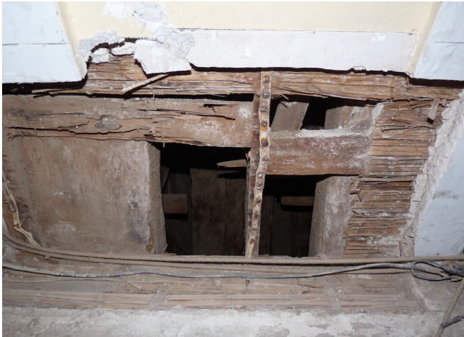
FIGURE 4.32 (ABOVE LEFT) View of plaster and caña chancada (flattened cane reeds) at the interior side of the vault. Image: Mirna Soto, for the GCI.
