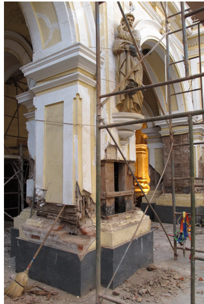
FIGURE 4.23 View of quincha pillar. Image: Sara Lardinois.
