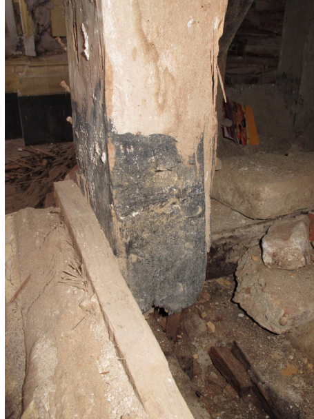
FIGURE 4.53 (NEAR RIGHT) Sector C: View of pillar base, showing deterioration of the wood post and sill. Image: Sara Lardinois.
