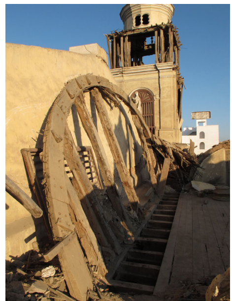
FIGURE 4.34 View of semicircular end panel that once formed the end of the barrel vault above the choir loft, which collapsed during the 2007 earthquake. Image: Sara Lardinois.
