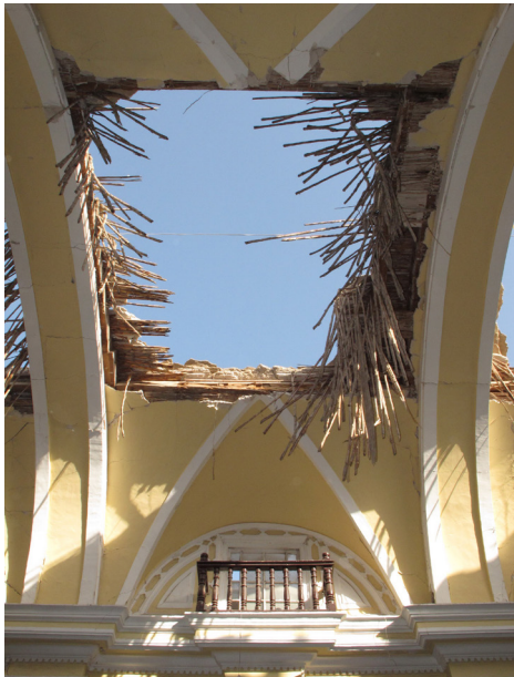
FIGURE 4.50 Sector C: View of a collapsed bay of the nave barrel vault. Image: Sara Lardinois.
