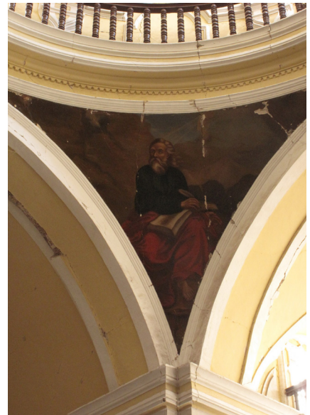
FIGURE 4.58 Sector E: View of the vertical cracks in a pendentive at the main dome. Image: Claudia Cancino.
