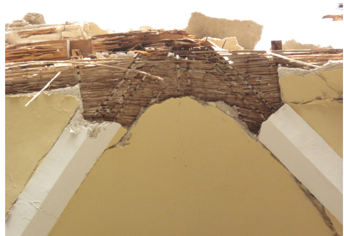
FIGURE 4.51 (TOP) Sector C: Damage to wood arches forming the nave barrel vault, with corrosion at the nails connecting the arch segments. Image: Claudia Cancino.
