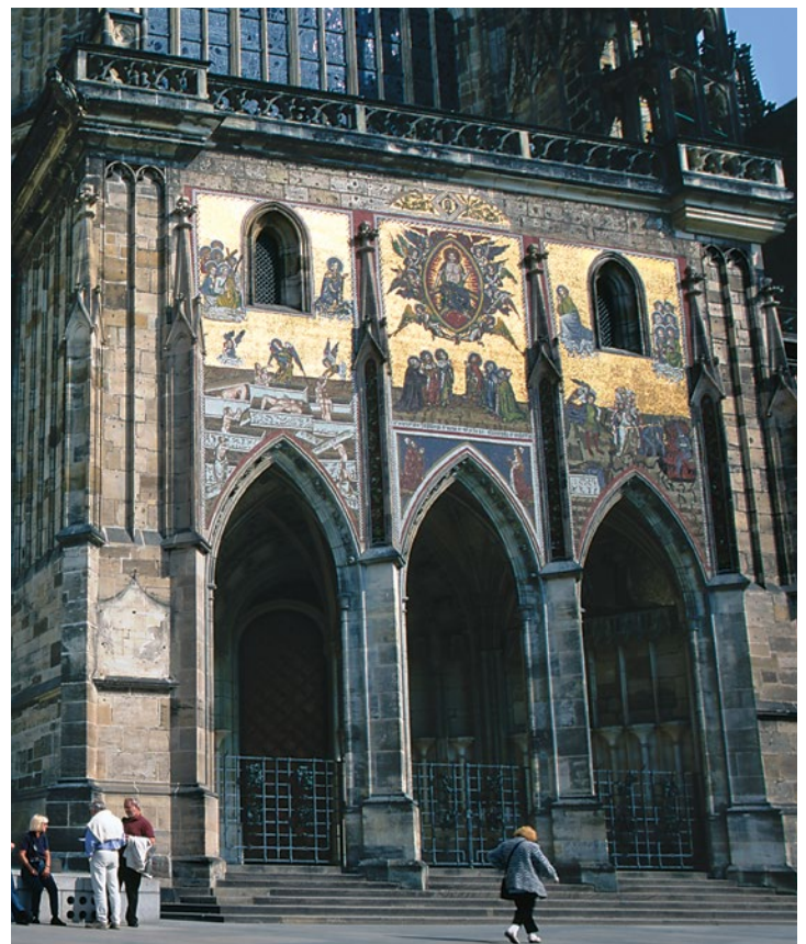
The fourteenth-century mosaic on St. Vitus Cathedral in Prague. Working with Czech authorities and conservators, the GCI studied the causes of the mosaic’s deterioration, developed a conservation strategy and a system for its protection, restored and conserved the mosaic, and developed a long-term maintenance plan. Photo: Dusan Stulik, GCI.
