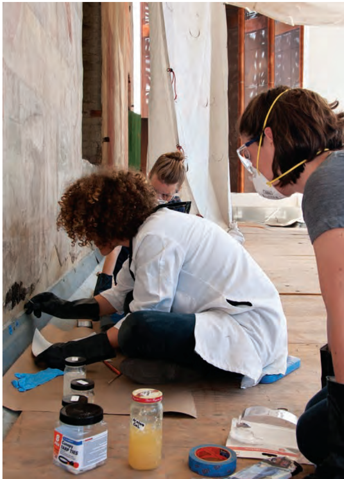
Conservators testing solvent gels to reduce and remove tar stains. Tar, which was applied to the wall, caused extensive damage along the wall's base. Part of final conservation was removing or reducing remaining tar and tar stains. Photo: Stacey Rain Strickler, for the GCI.
