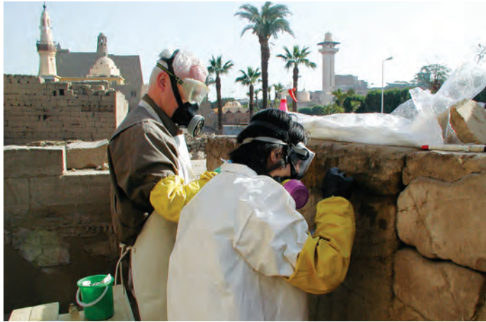
Field conservators John Stewart (left) and Hiroko Kariya (right) in protective clothing testing alkoxy silane stone consolidant for the block yard conservation project, Luxor Temple, Egypt. Photo: Sue Lezon, courtesy of the Epigraphic Survey, Oriental Institute, University of Chicago.
