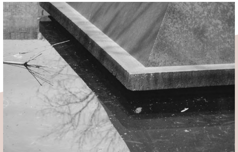
Detail of the support pyramid of Broken Obelisk , prior to the sculpture’s conservation. The sculpture’s location over a pool (in accordance with the artist’s wishes) exacerbated deterioration problems. Photo: Laramie Hickey-Friedman, The Menil Collection. Courtesy of the Rothko Chapel, Houston. ©2007 Barnett Newman Foundation, New York/Artists Rights Society (ARS), New York.
