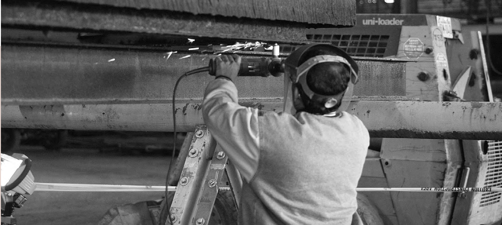
Contractor removing severely corroded steel from the footing of the sculpture in order to replace it with a stainless steel footing. Photo: Laramie Hickey-Friedman, The Menil Collection. Courtesy of the Rothko Chapel, Houston. ©2007 Barnett Newman Foundation, New York/Artists Rights Society (ARS), New York.
