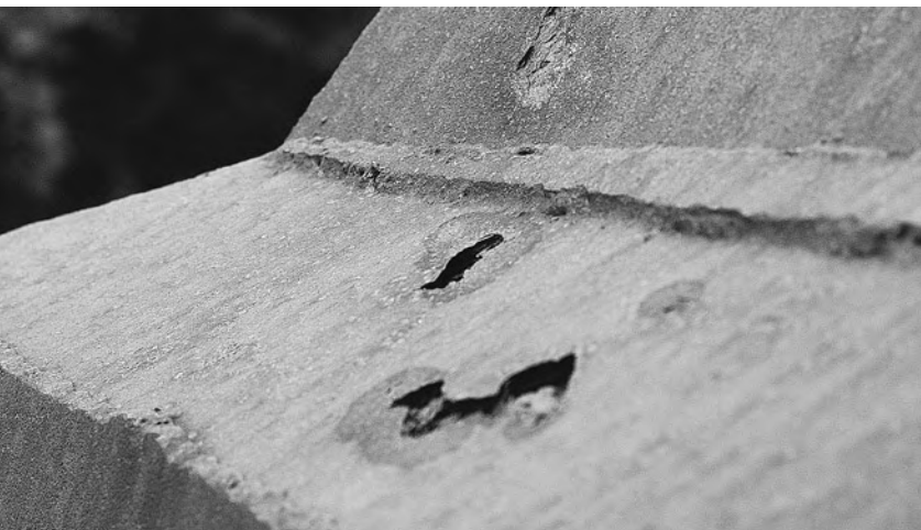
Extensive pitting at the top of Broken Obelisk in 2004. The pitting was caused by expandable foam that was sprayed into the top of the obelisk during conservation treatment in the 1980s, and the unintended result was that the interior walls of the obelisk were continually exposed to moisture. The metal in this section needed to be replaced. Photo: Laramie Hickey-Friedman, The Menil Collection. Courtesy of the Rothko Chapel, Houston. ©2007 Barnett Newman Foundation, New York/Artists Rights Society (ARS), New York.
