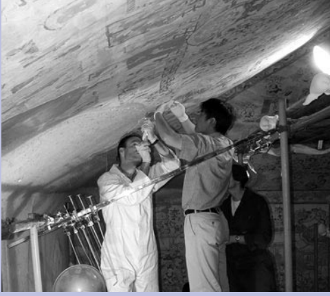
Cave 85 at the Mogao grottoes. Project team members Stephen Rickerby and Yang Jinlian inject earth-based grout behind painted plaster to re-adhere plaster to the underlying rock. Photo: Lorinda Wong.
