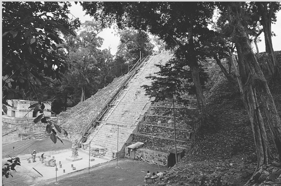
The hieroglyphic stairway at the Maya site of Copán in Honduras, during the repair of the tarp protecting the stairway. Photo: Elsa Bourguignon.
