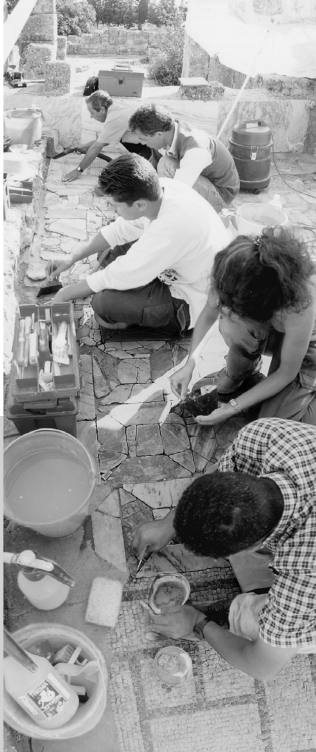
Trainees and instructors performing cleaning and stabilization treatments. Stabilization work utilizes different lime mortar mixes to reset and fill gaps between the individual elements of two different types of Roman pavements— opus tessellatum (foreground) and opus sectile (center). Photo: Richard Ross.
